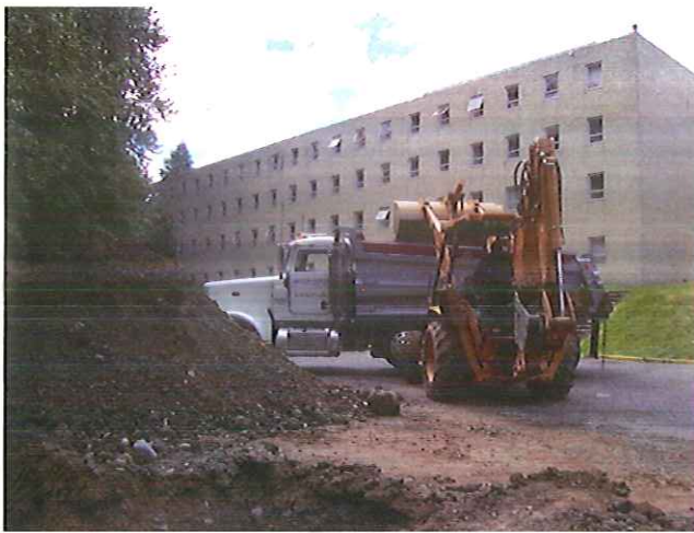
Photograph 7. Petroleum contaminated soil directly loaded onto truck for offsite disposal (June 25, 2007).
