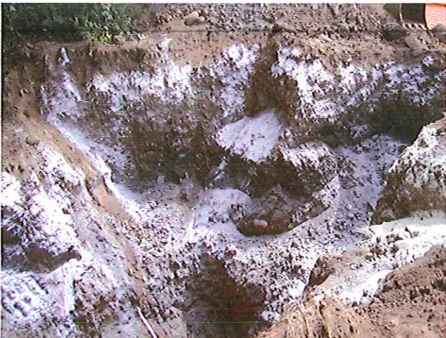
Photograph 11. White Oxygen Release Compound applied to excavation before backfilling (June 27, 2007).
