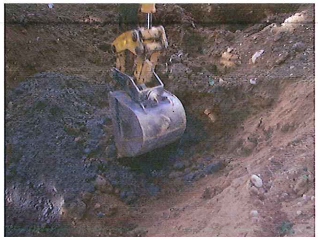
Photograph 6. Removing gray petroleum stained soil from excavation floor (June 25, 2007).
