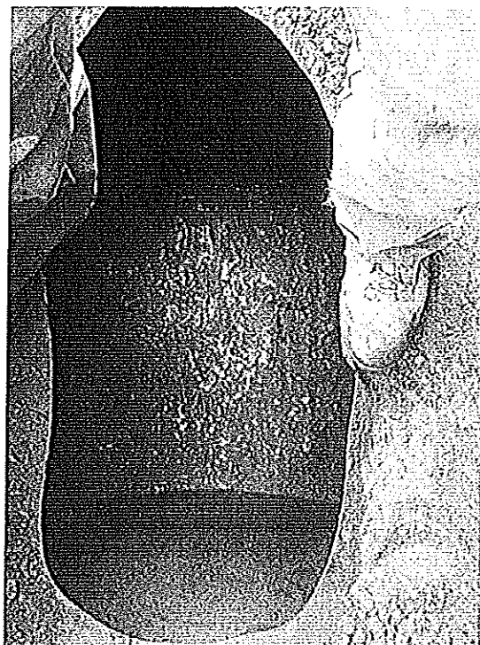
A portion of the top of the tank was exposed and cut open. All of the tank contents were removed and the tank interior was thoroughly pressure-washed.
