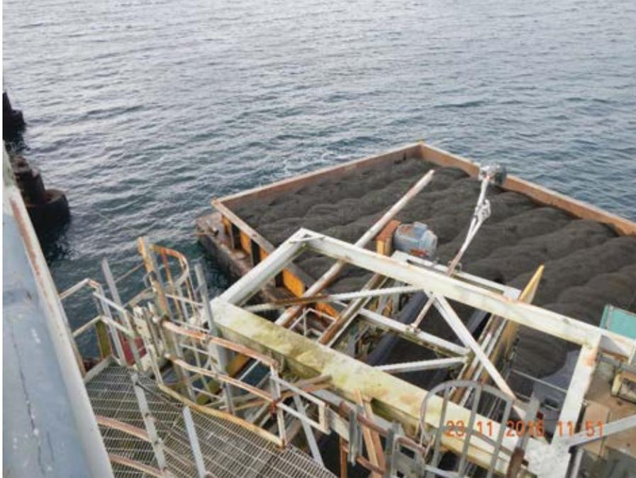
2016-11-23 10.51.43 Gravelly sand + AC being loaded onto the KP-2 barge.
