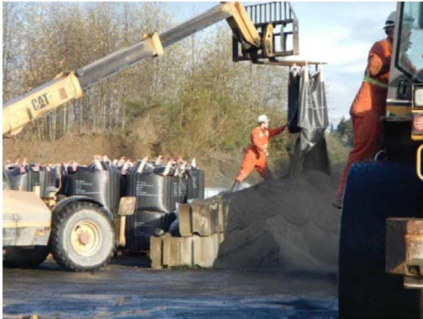
Photo 5 500-kilogram bulk bag of AC being emptied into feed pile by CalPortland employee prior to blending with ENR.
