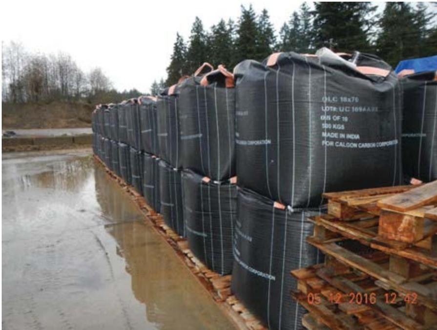
2016-12-05 11.42.24 AC placed on pallets to keep the super sacks out of the standing water.
