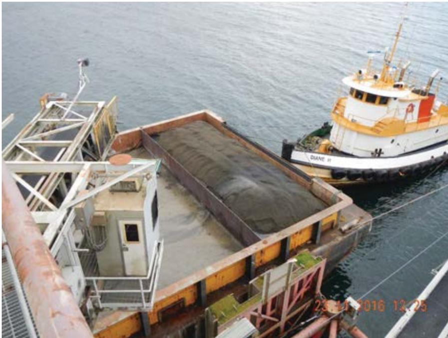
2016-11-23 11.25.28 Sand + AC was loaded at the stern of the KP-2 barge. CalPortland loaded the material so that just the toe of the windrow was against the bulkhead between the two materials.
