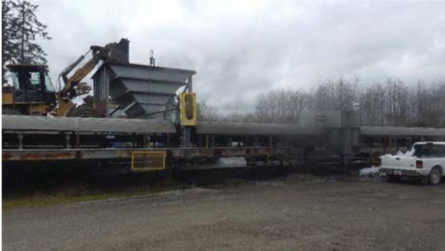
**20161213\_124124** Activated carbon being loaded into the feed hopper and placed onto the Gravelly Sand material.
