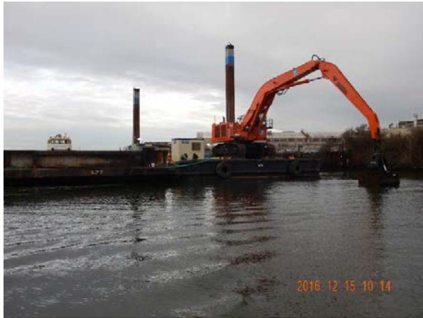
Photo 19 Placement of material in the intertidal plot.
