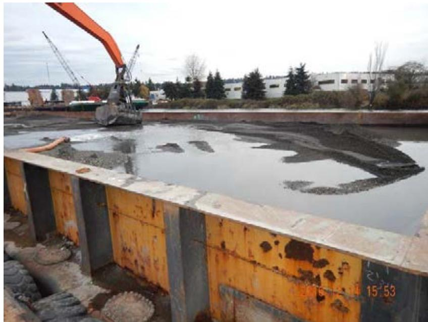
Photo 16 Pumping of water into the barge to soak ENR+AC material overnight. Excavator is knocking down wind rows and leveling material.
