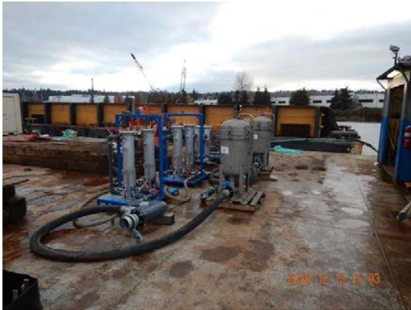
Photo 29 Water treatment plant for all water that is pumped out of the barges.
