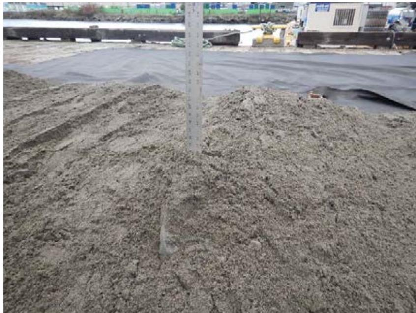
Photo 14 Thickness measurement (~14 inches) after placing third bucket using modified overlapping bucket placement pattern.
