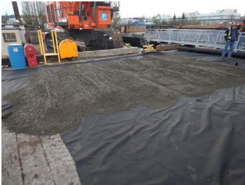
Photo 10 Placement test on deck. Note hummocky surface.
