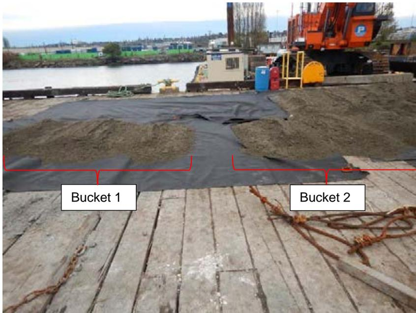
Photo 12 Modified overlapping bucket placement pattern after first two buckets placed.
