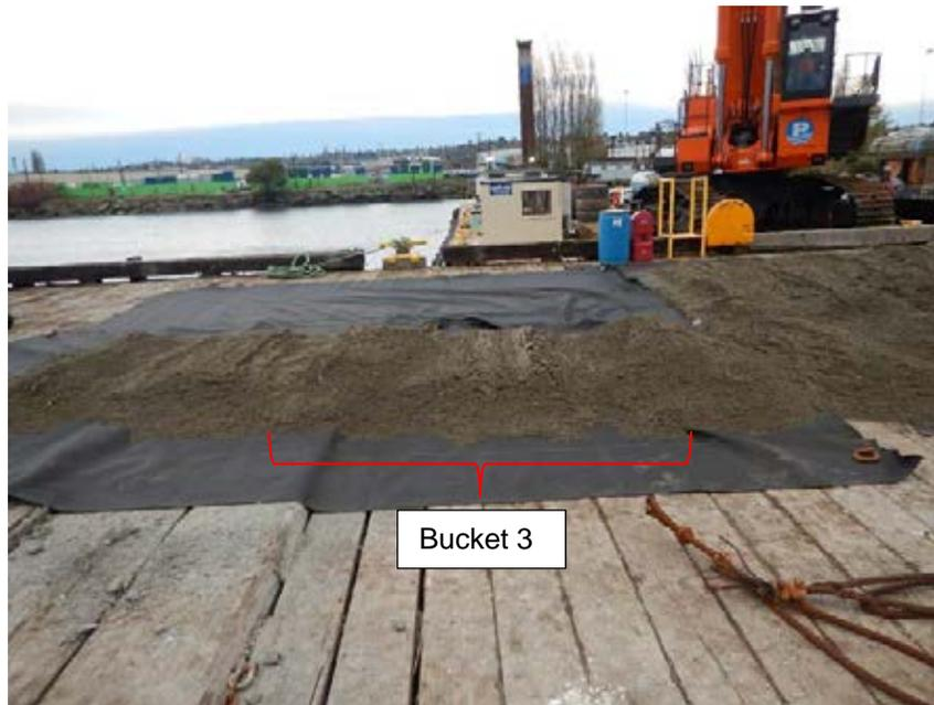
Photo 13 Modified overlapping bucket placement pattern after third bucket placed.
