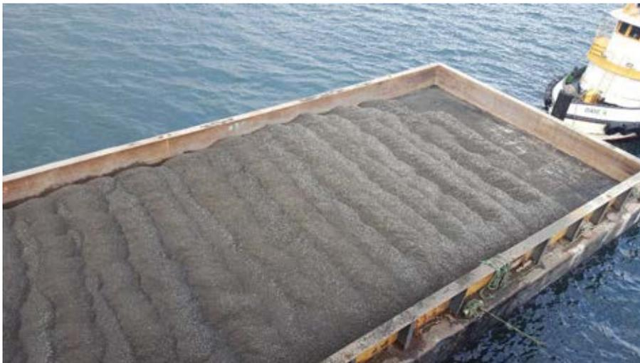
**20161213\_130734** Gravelly Sand + AC loaded onto the KP-2 barge.
