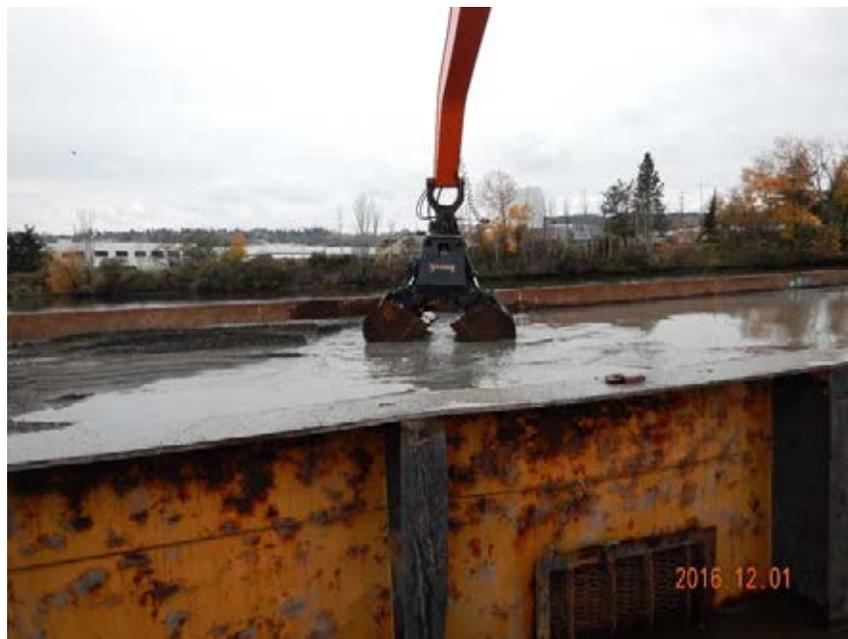
Photo 20 Excavator grabs a bucket of submerged ENR+AC material.
