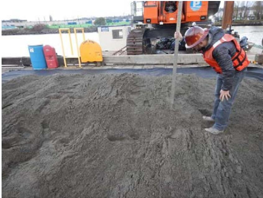
Photo 11 Thickness measurement (~17 inches) after placing offset overlapping fifth bucket.
