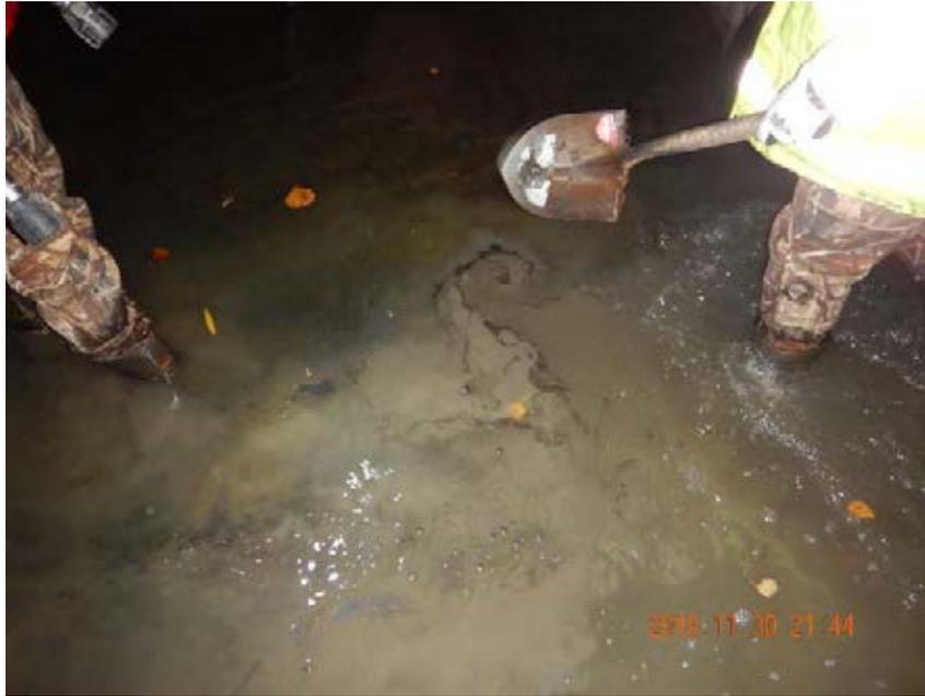
Photo 27 Fine-grained AC floating to the surface after the underlying ENR+AC material was disturbed by the shovel.
