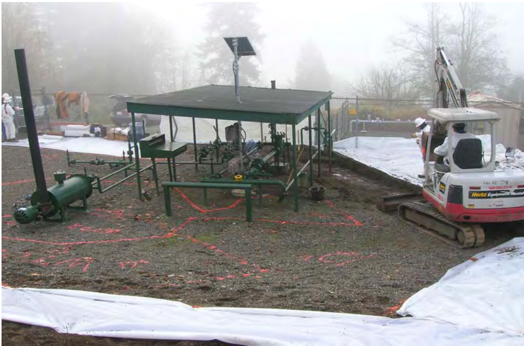
Photo SNMS-1 Pre-Remediation Site Preparation
