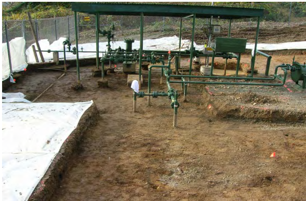
Photo SNMS-2 Remediation in Progress
