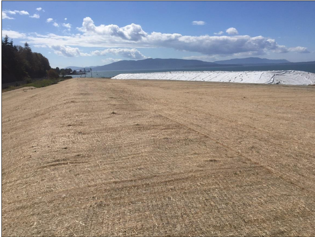
36. Looking south from top of northern stockpile. Grass seed has not been successful.
