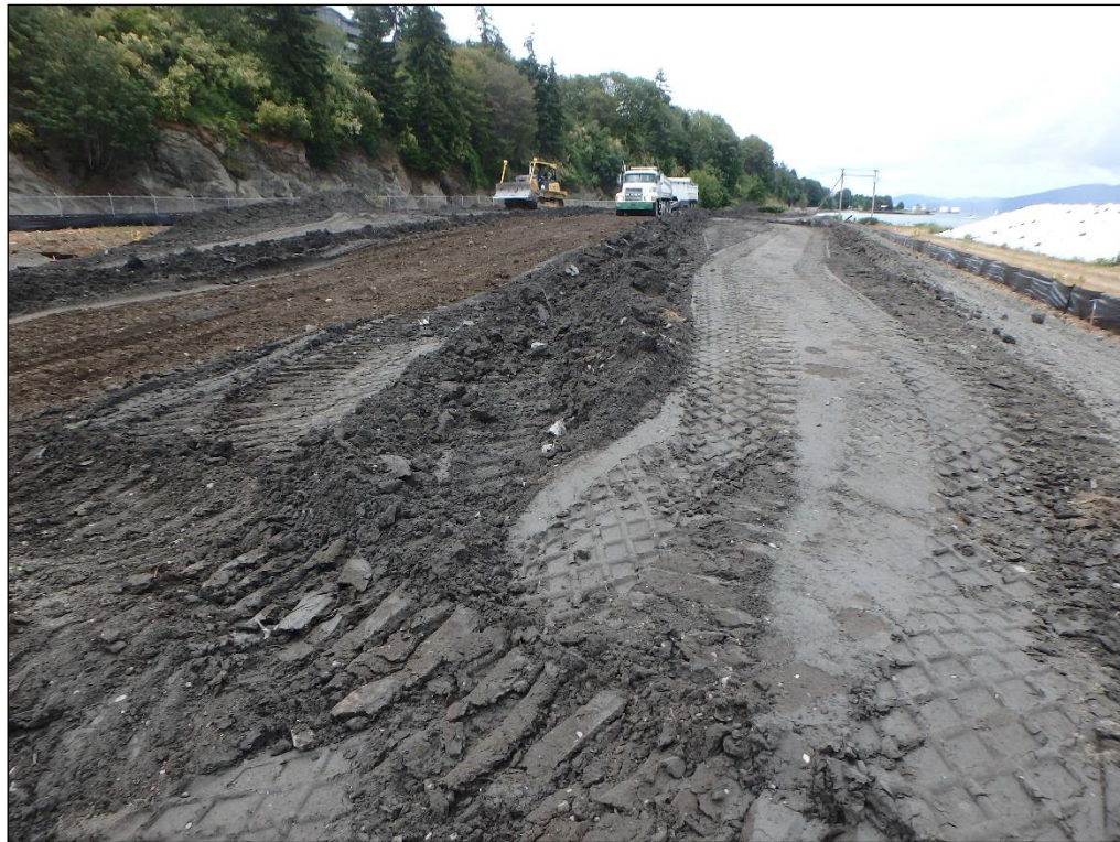
20. Construction of southern stockpile.
