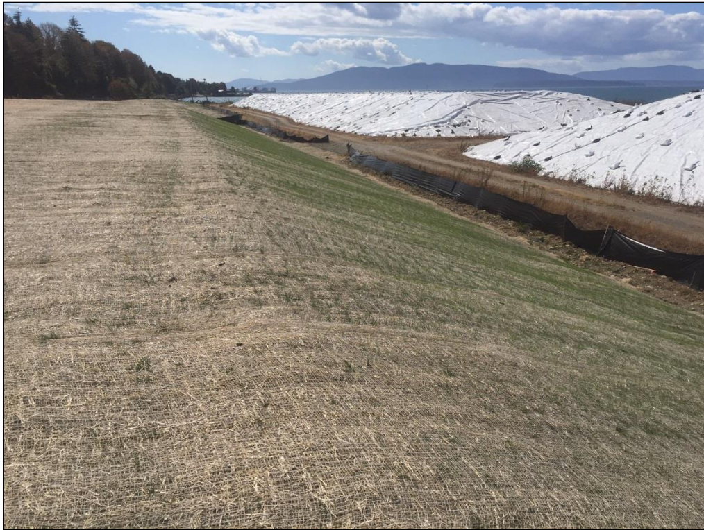
35. Looking south along the west edge of the northern stockpile.
