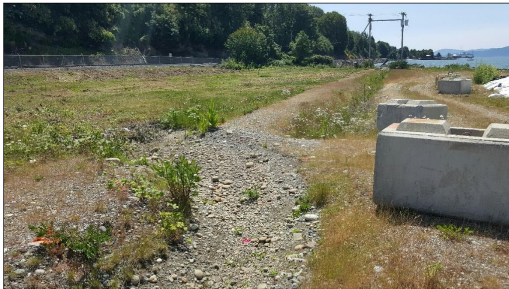
4. Looking south from southwest end of site. Vegetation has been mulched and left in place.
