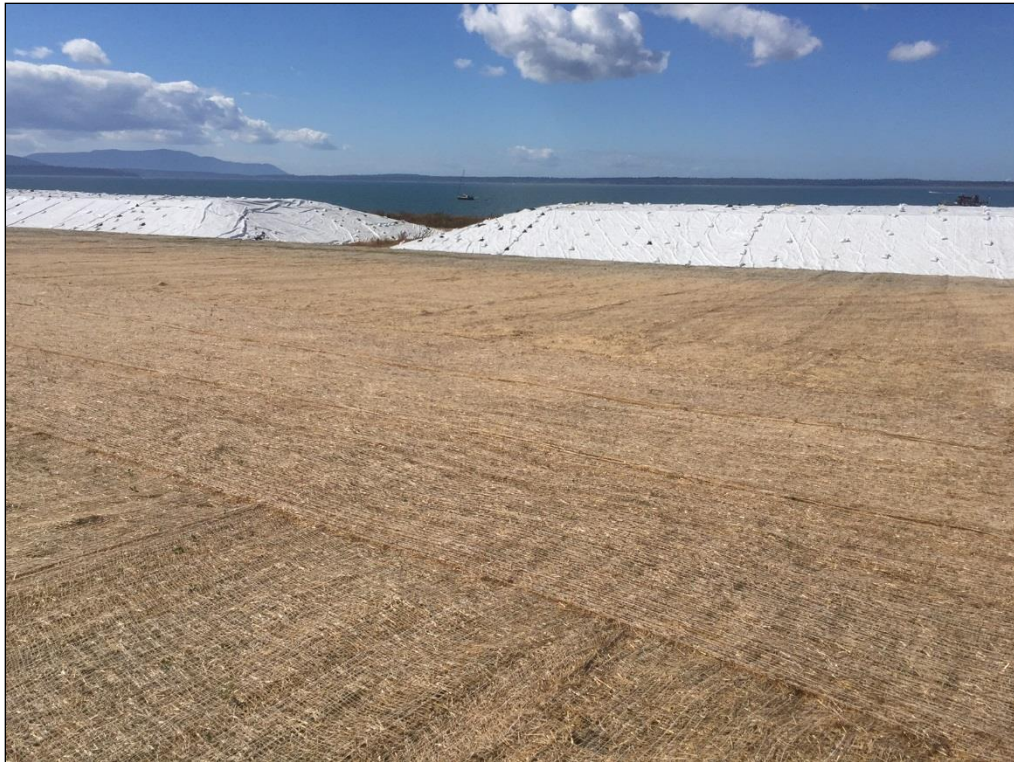
37. Looking west from top of northern stockpile.
