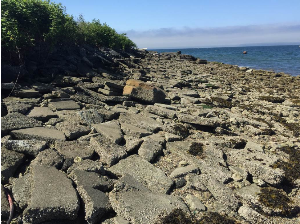
Photograph 8. Extensive coverage of angular concrete below the MHHW within the middle of the Site.
