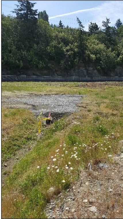
5. Temporary culvert installed between the two stockpiles.
