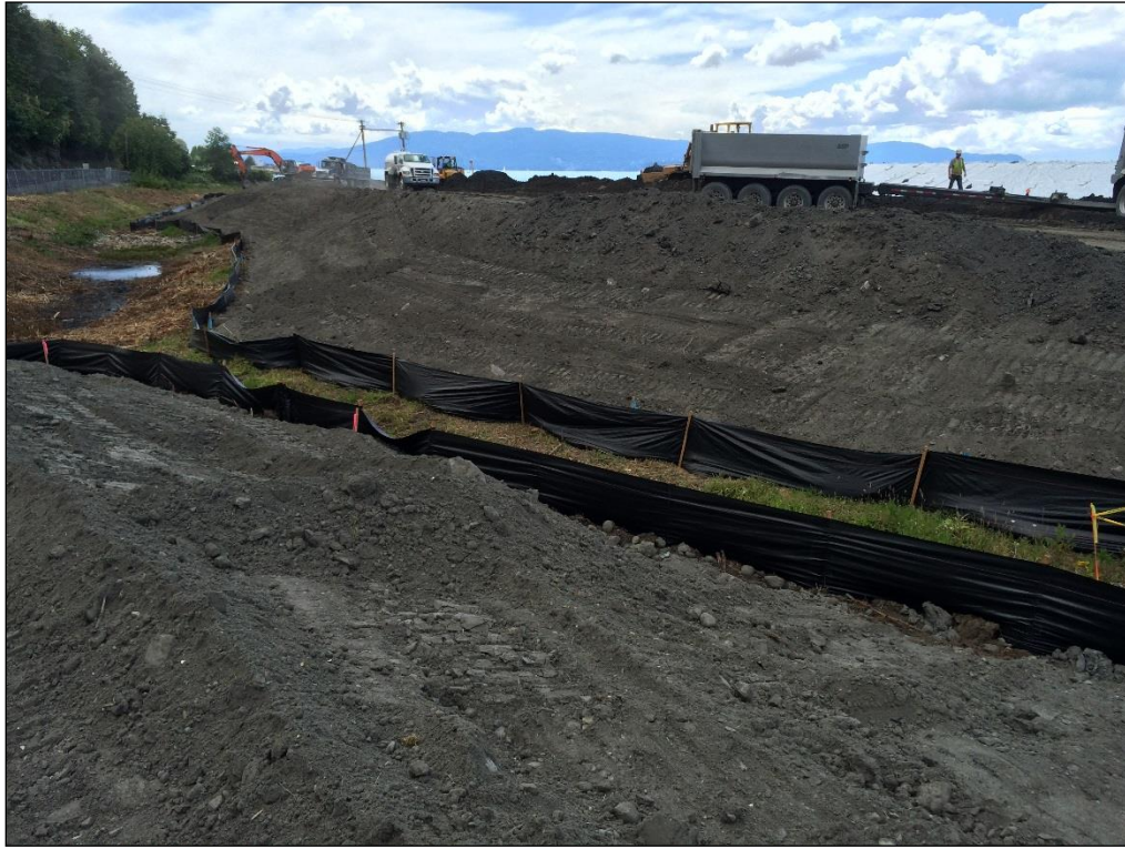
21. Looking south from top of north stockpile.
