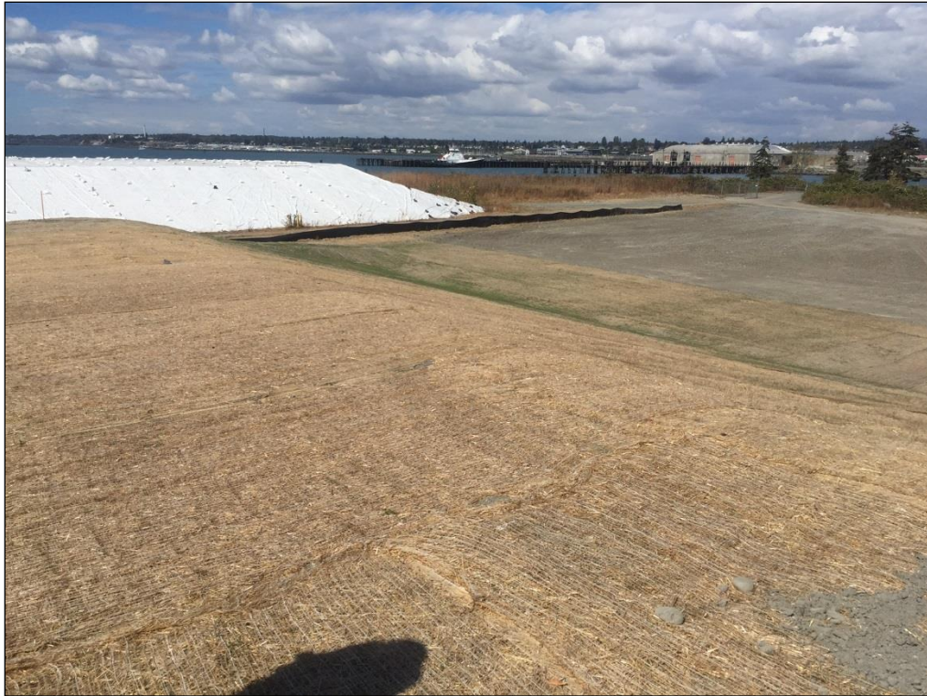
34. Looking northwest from top of northern stockpile.
