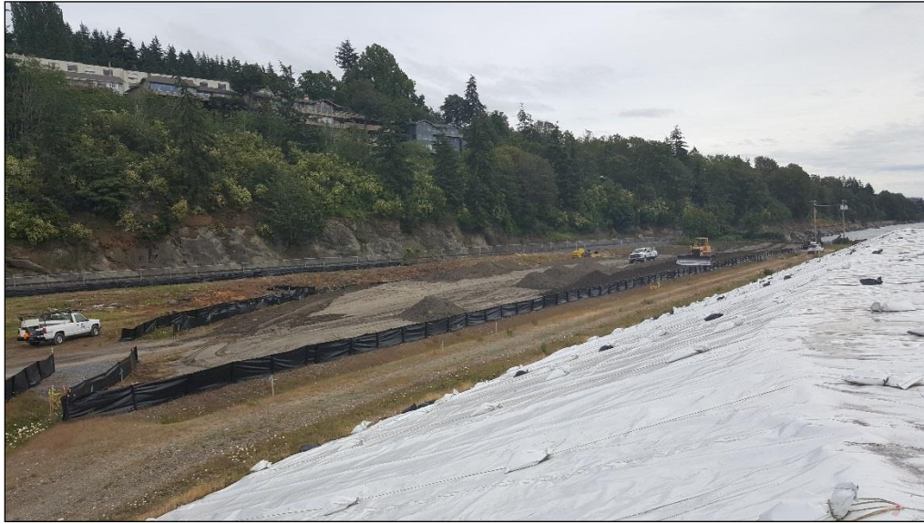
11. Looking from existing stockpile toward the southern new stockpile.
