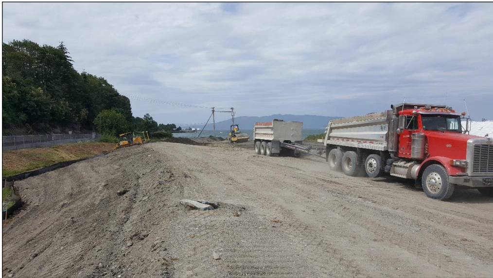
16. Construction of southern stockpile. Note oversized piece in foreground.
