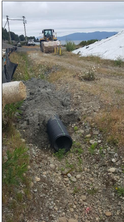
24. Incomplete culvert. Looking to the south.
