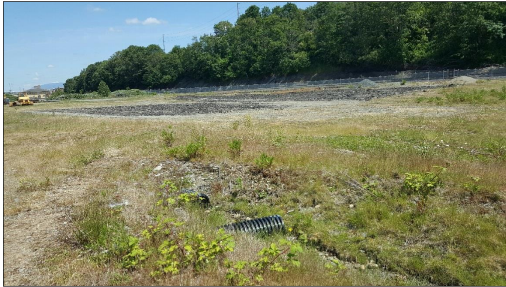
3. Looking north from southwest end of site. Asphalt has been ripped and vegetation has been mulched and left in place.
