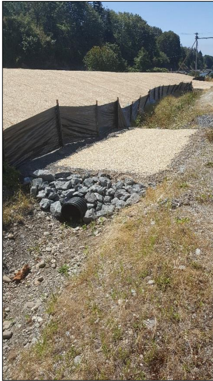
29. Previously incomplete culvert has been completed.
