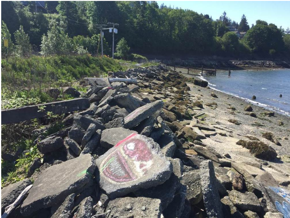
Photograph 6. Weedy grasses and forbs and extensive coverage of angular concrete between the upland and the MHHW along the southern extent of the Site.
