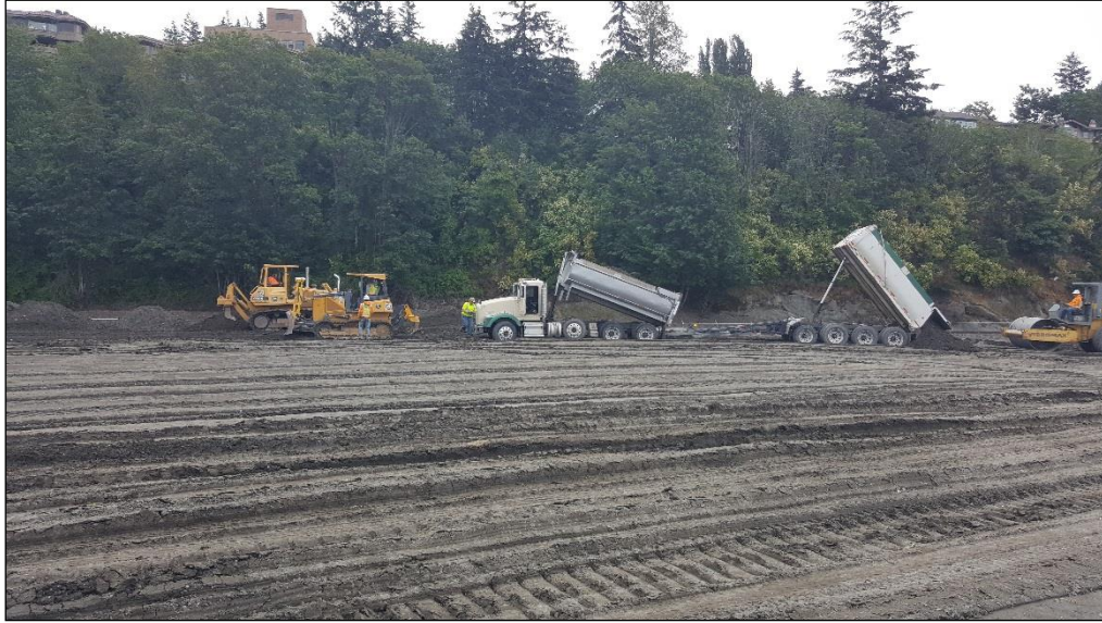
15. A stuck truck being pulled out by bulldozer.
