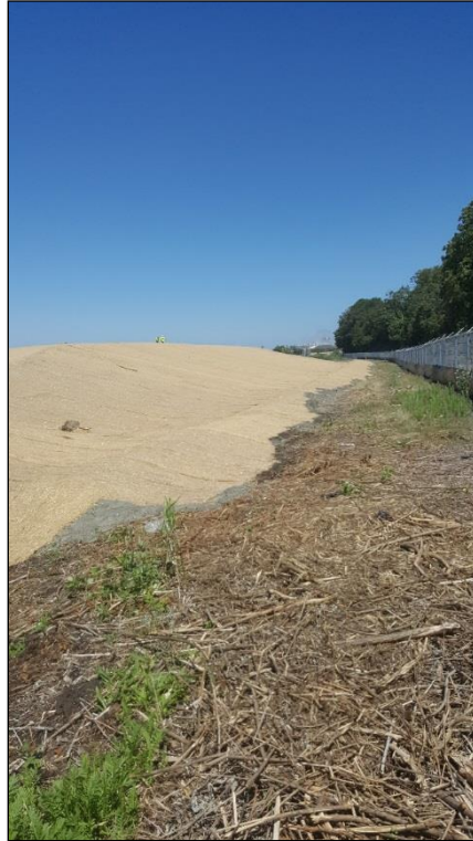
27. Drainage berm has been constructed and covered with erosion control matting.
