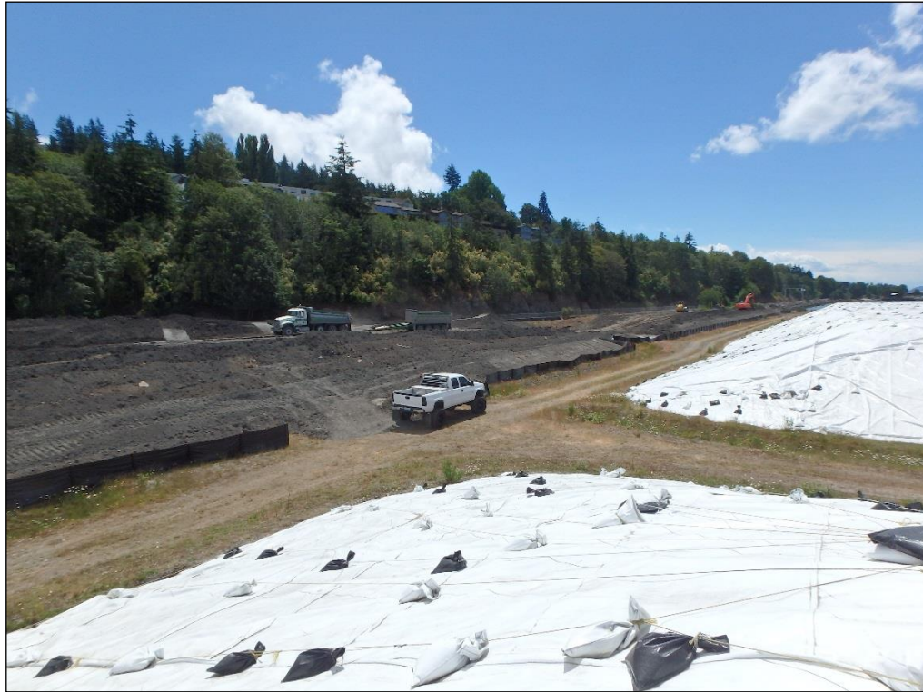
19. Both stockpiles viewed from top of north existing stockpile.
