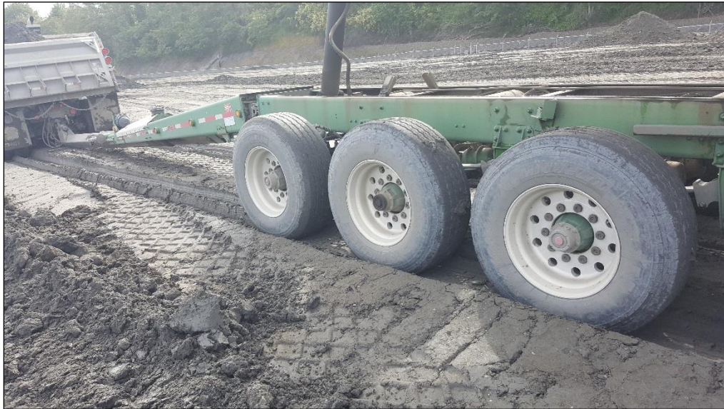
18. Trucks getting stuck in compacted fill material.
