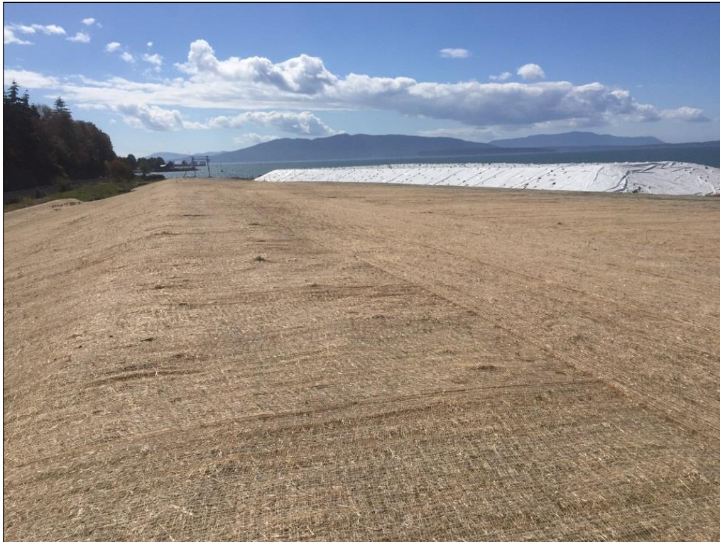
2. Top of pile looking southwest. Southern IPA in background.
