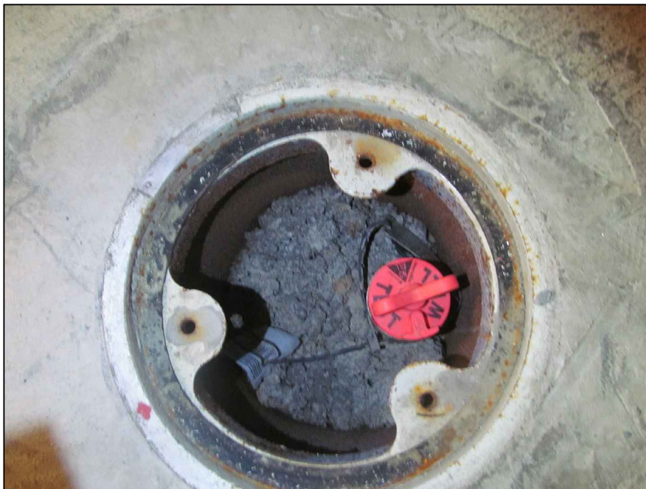
Photograph 10: View of well MW6 without the well cover.
