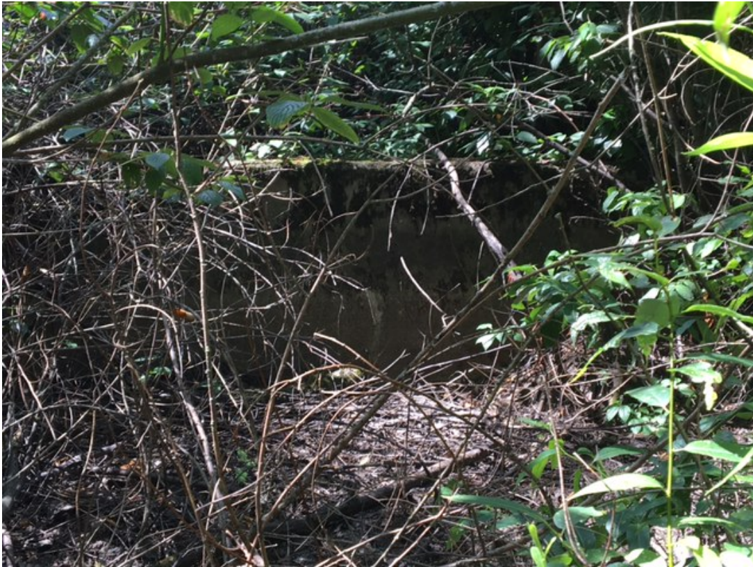
Photo 3 - concrete wall in detention basin used to separate treatment cells.
