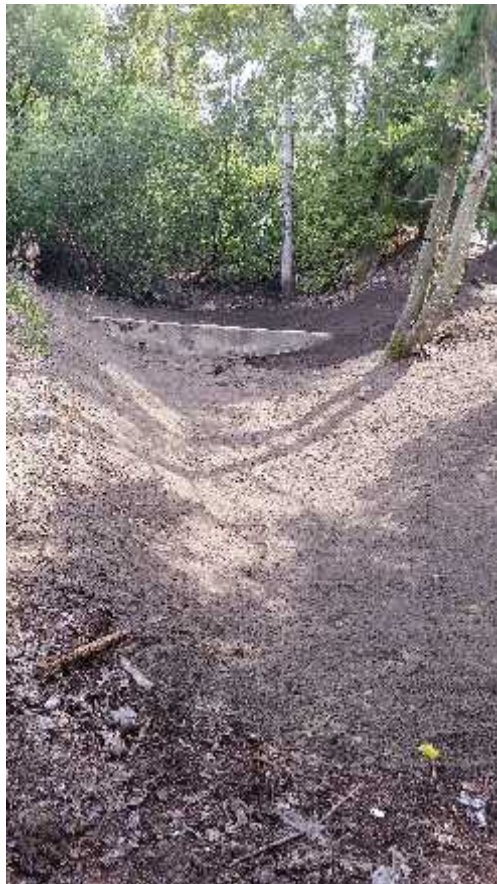
Photo 5 - View of the backfilled excavation, from the western edge of the stormwater retention basin, facing northeast.
