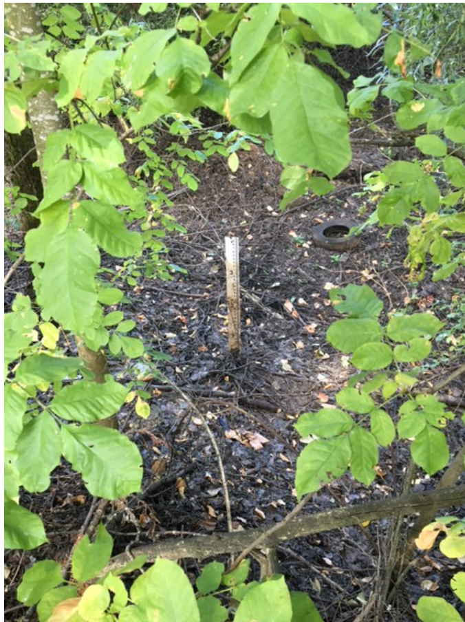
Photo 4 - water gage in detention facility.
