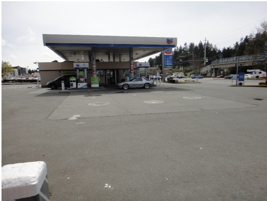
Site looking south from the southwest corner of the old vapor extraction blower assembly (see Site figure below). Both photos taken by Kim Wooten on 4/18/18.
