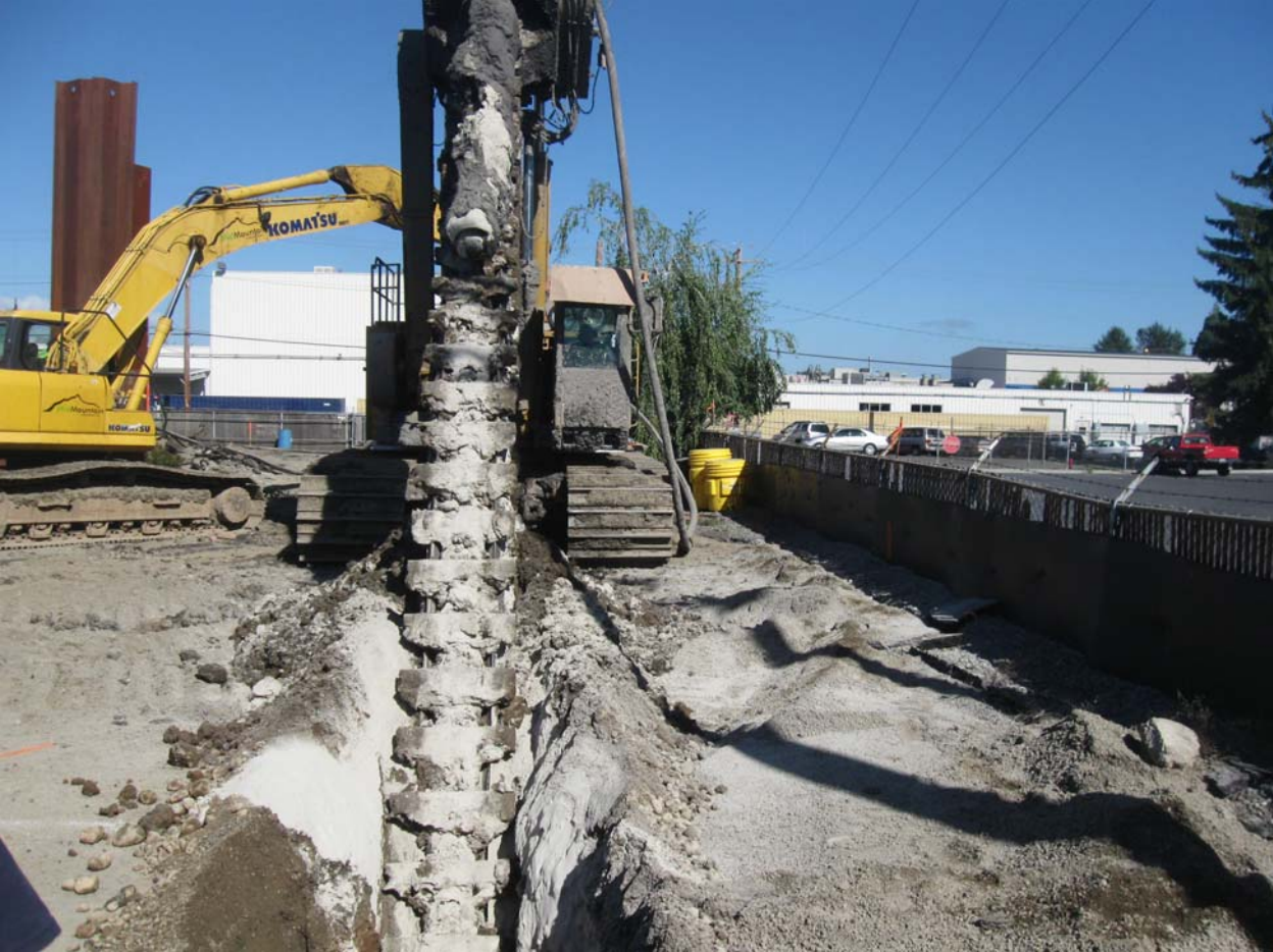
Pilot hole 11+18 looking north.
