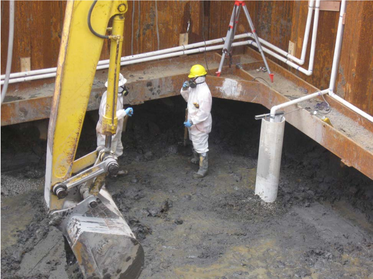
Excavation at grade (9.75) in NE corner.
