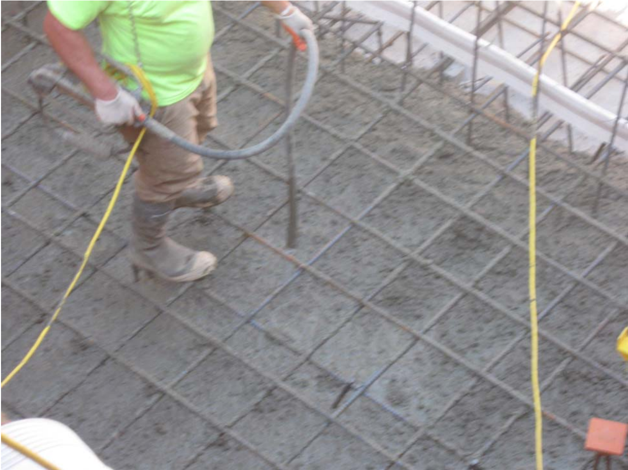
Vibrating first lift of concrete.
