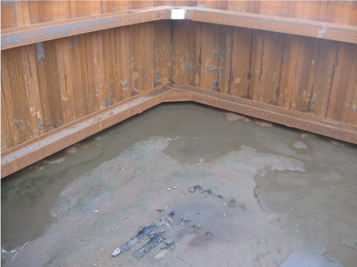
Excavation after removal of stormwater.
