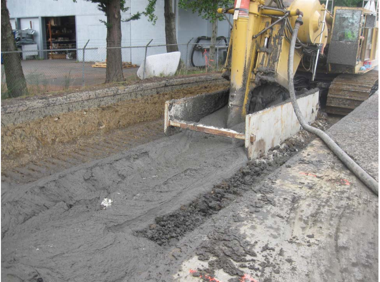
Initial mix in slurry wall trial.
