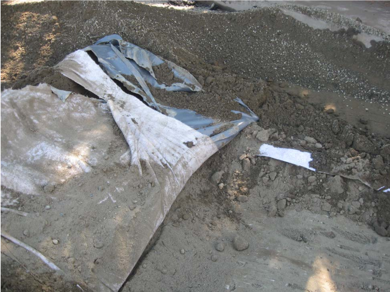
PVC liner over clean sandy soil southeast corner of site.
