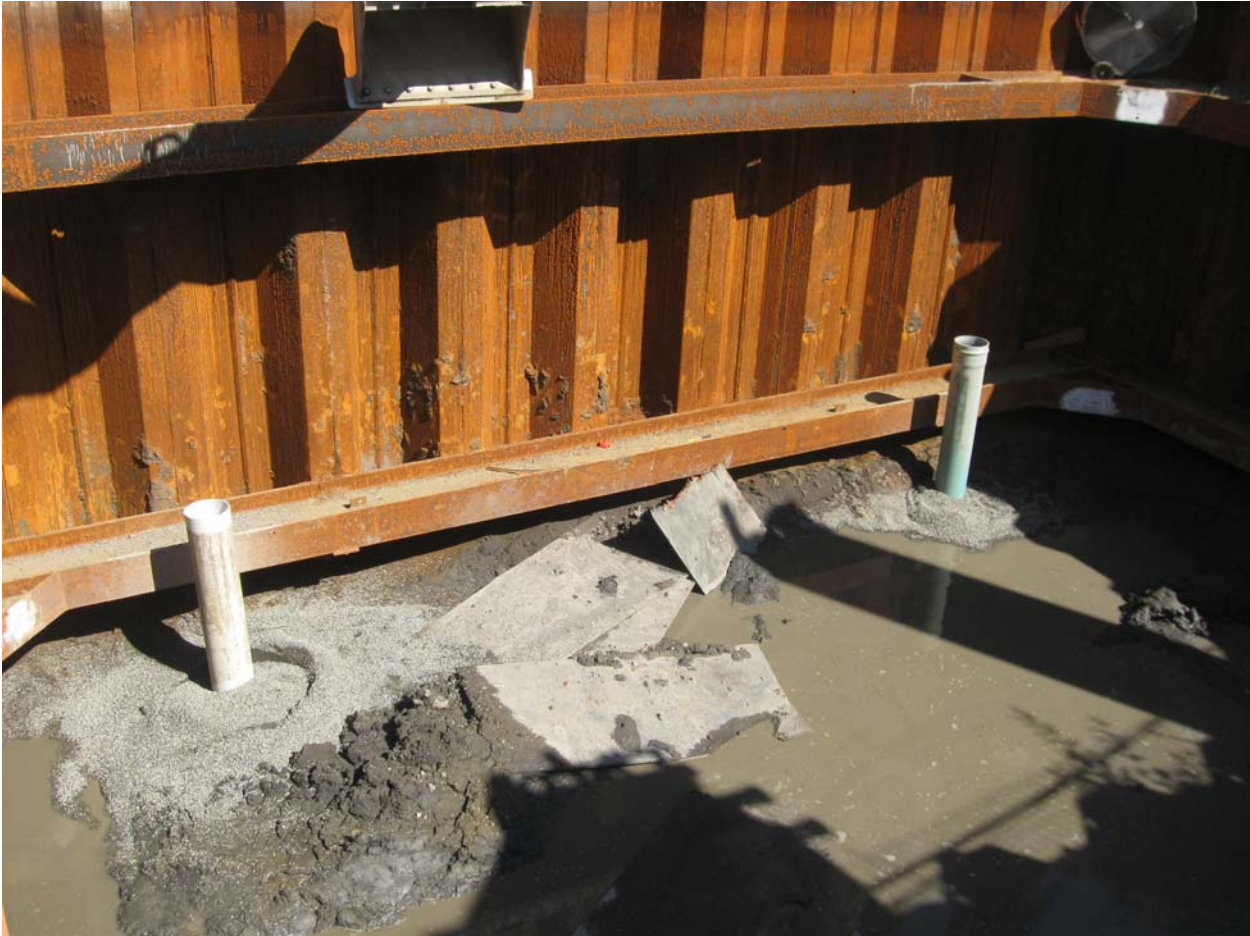
East side wells with pea gravel in place and casing pulled.
