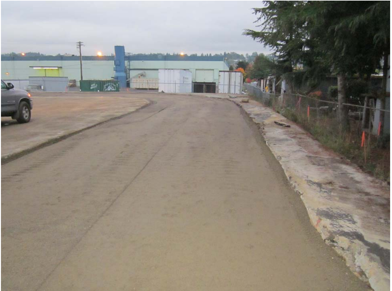
Backfilled key trench with crushed rock in place station 14+50.
