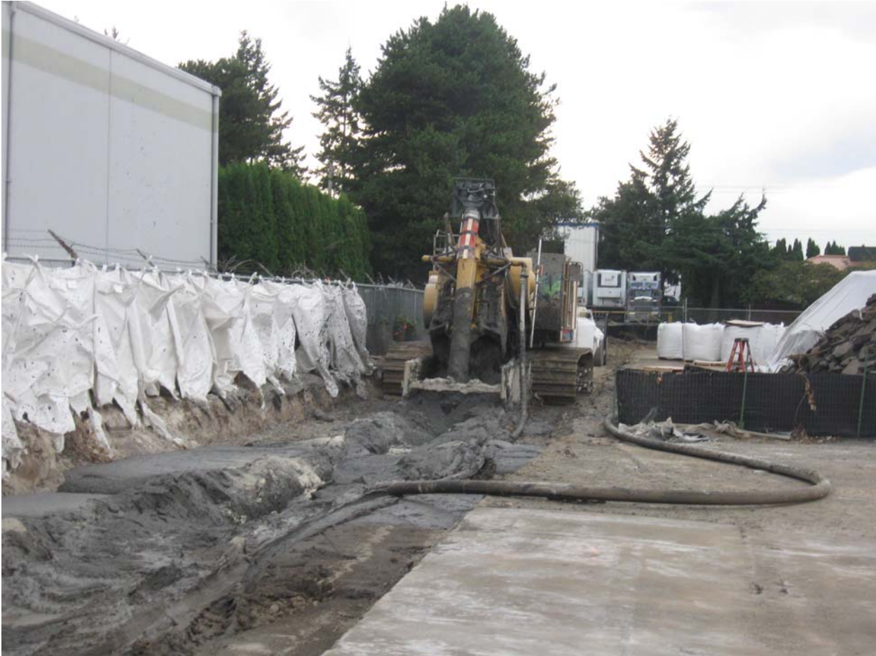
Progress as of 6:00 PM.
