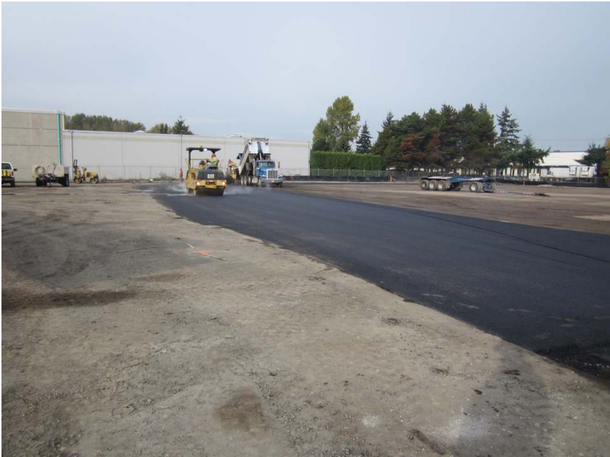
Paving tie-in to existing pavement.
