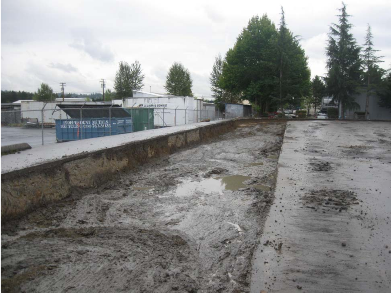
Slurry spread in key trench at station 13+00.
