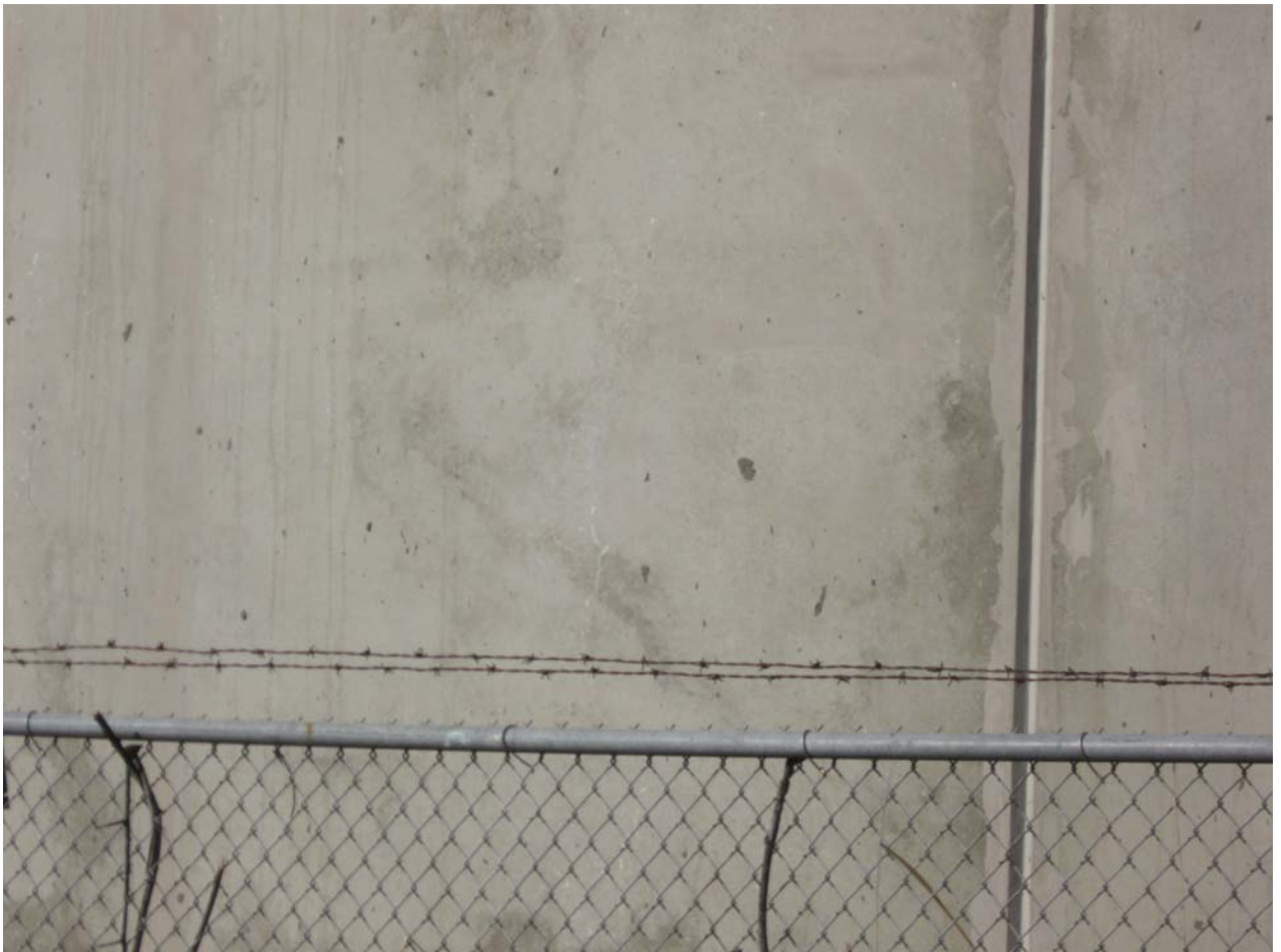
Slurry mix on painted wall.
