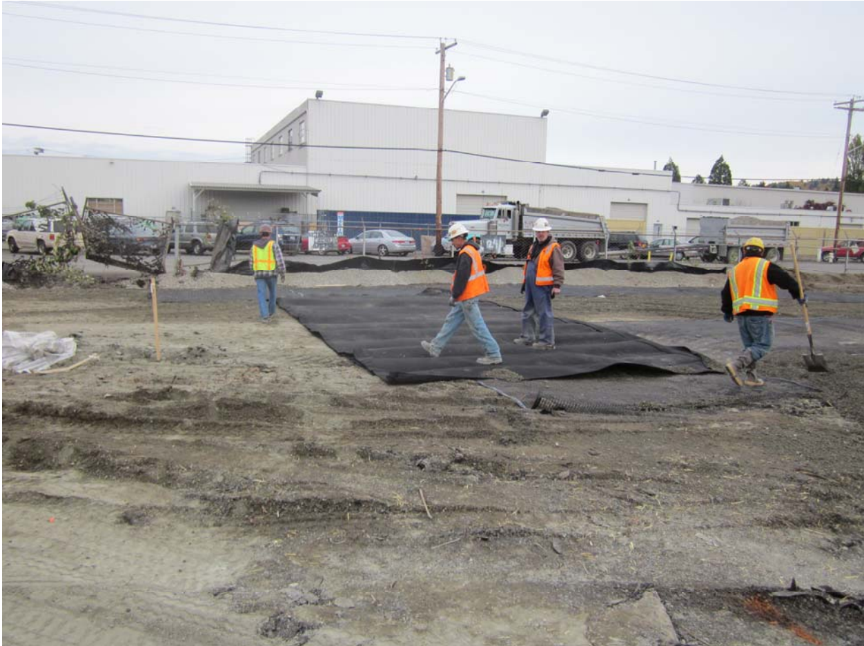
Geocomposite over geogrid at proposed new entrance.
