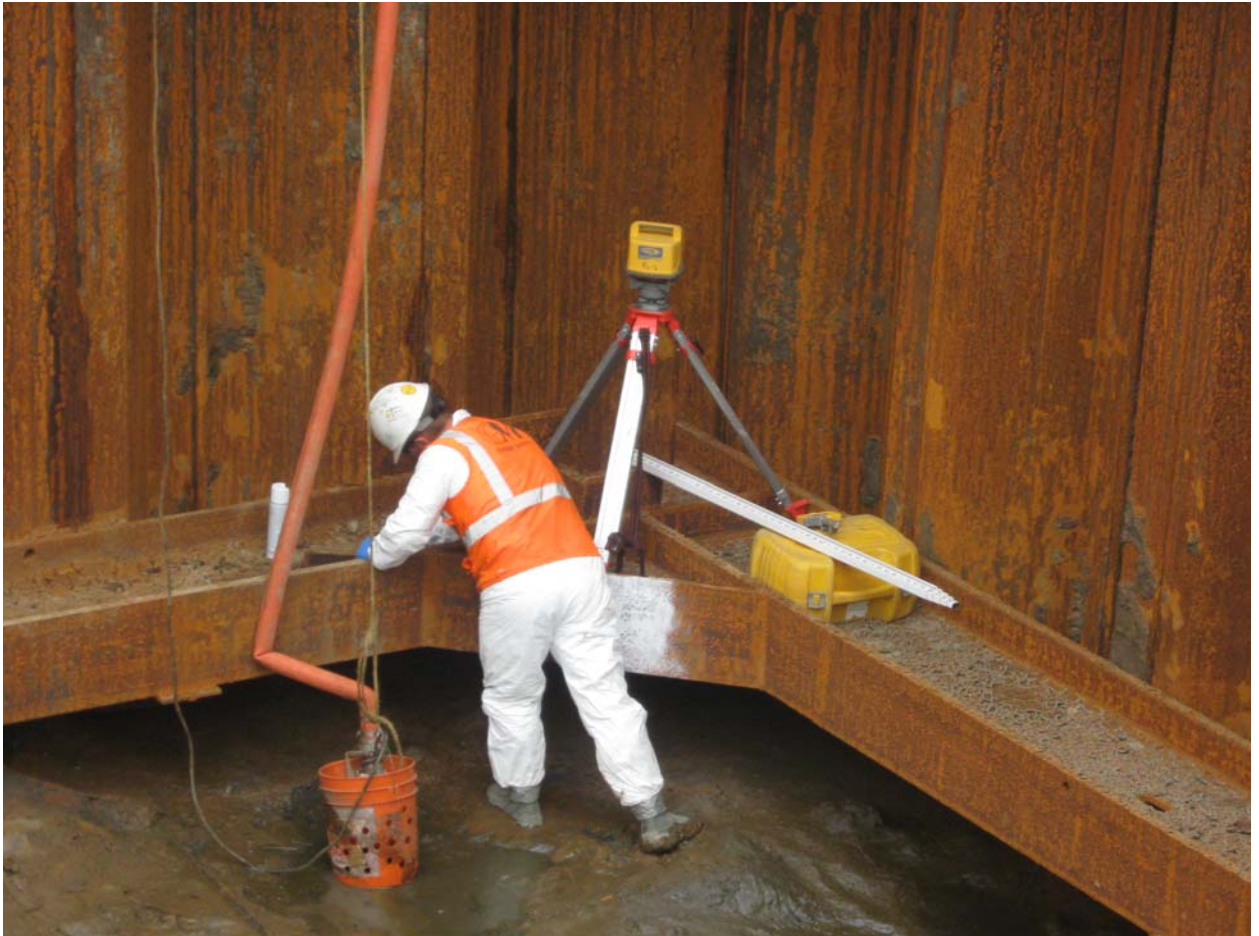
Establishing grade control with laser in excavation.
