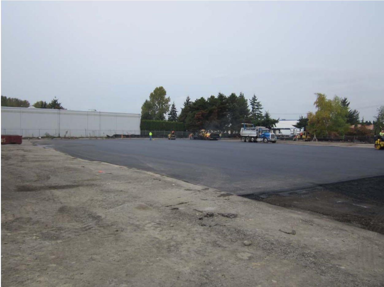
On-going paving in northwest quadrant of site.
