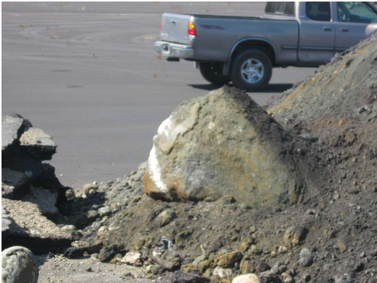
Example concrete debris found at approximately 13+00 in the exploratory trench.
