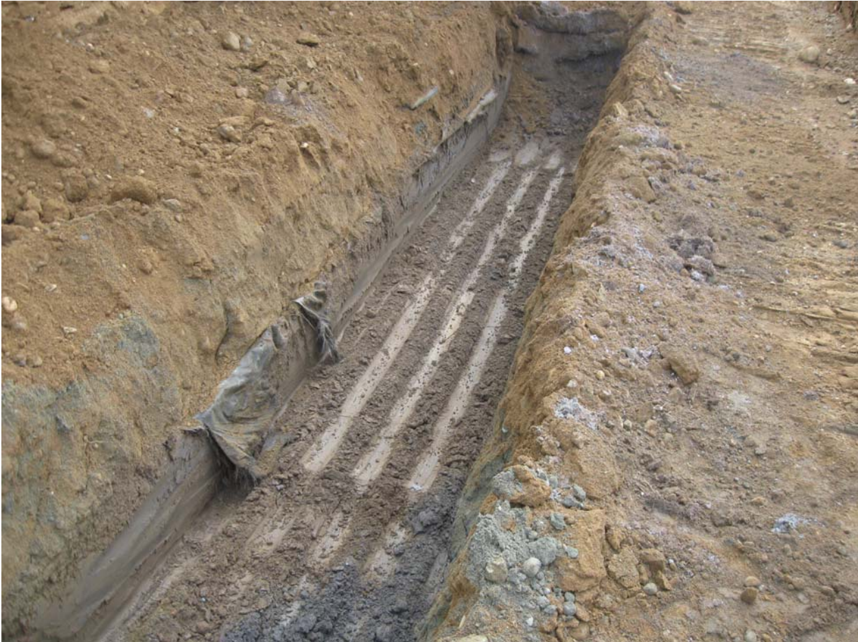
Continued excavation of exploratory trench through sludge.
