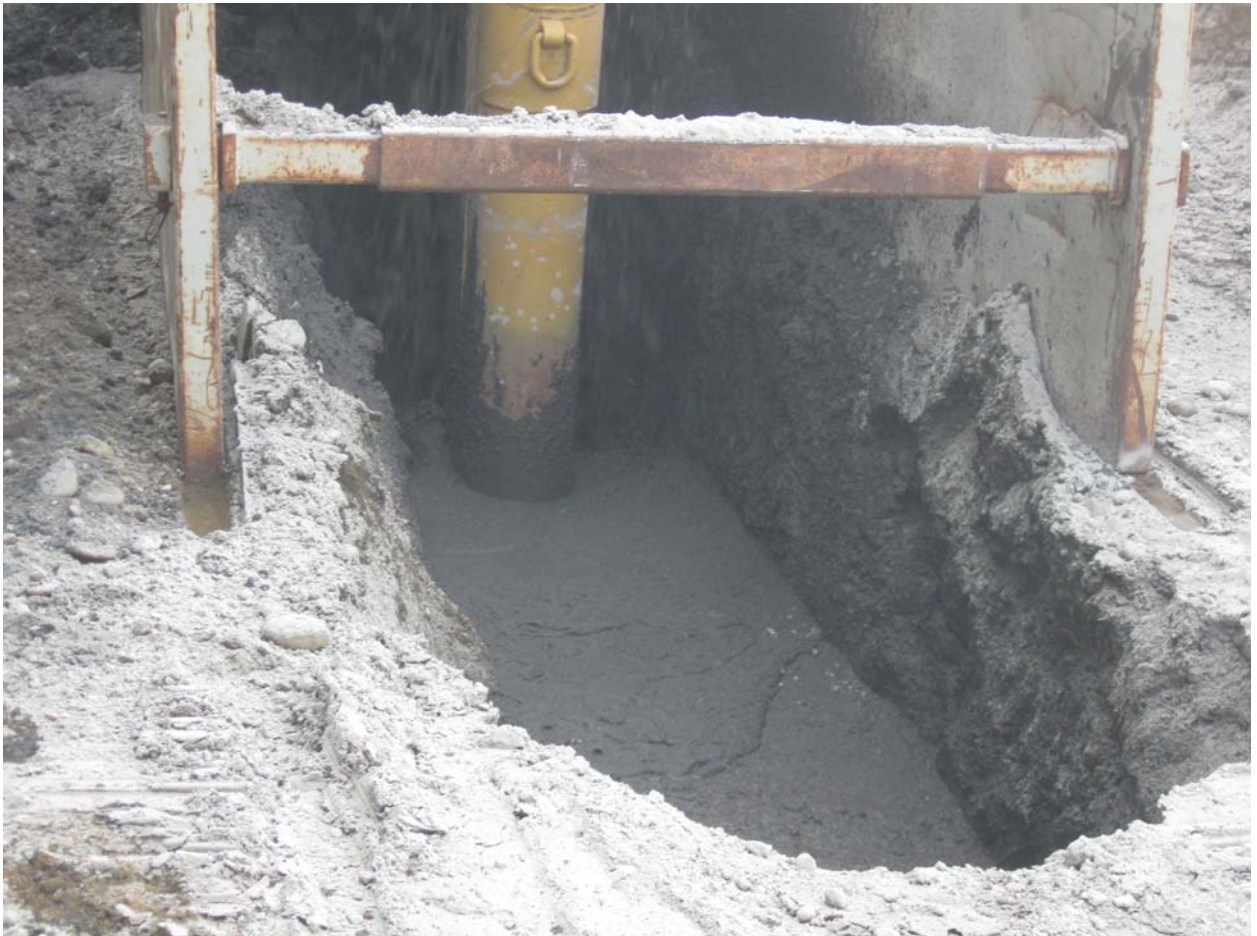
Pilot hole at start of slurry wall work.
