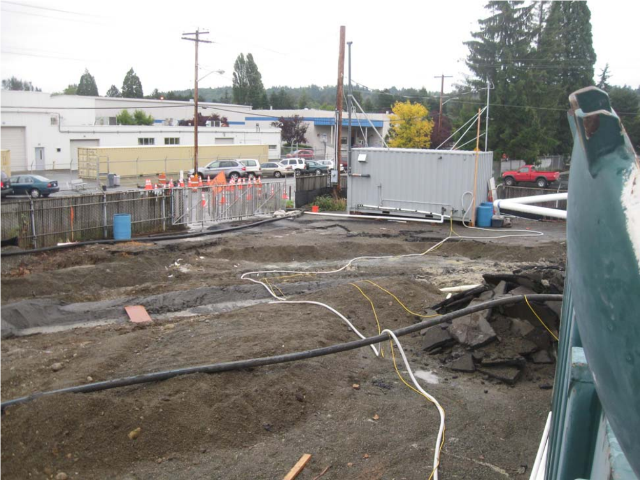
General site conditions as of 10/03/11.
