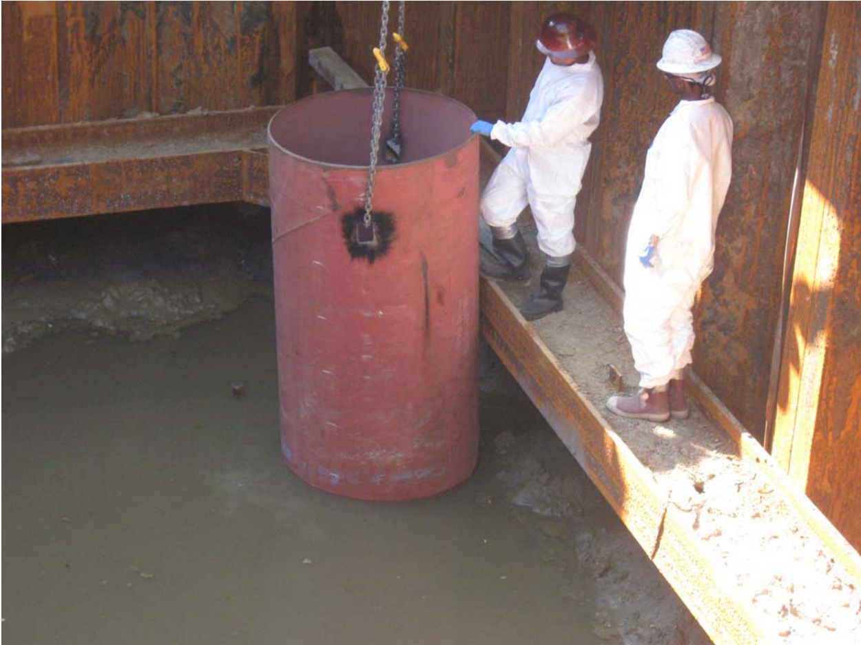
Lowering steel casing into NE corner of excavation.
