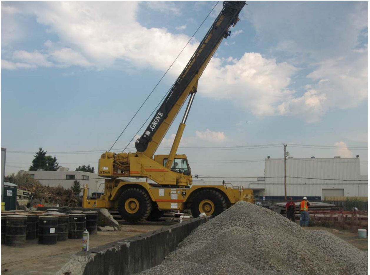
70-ton crane used for lifting and setting vertical rebar and forms.
