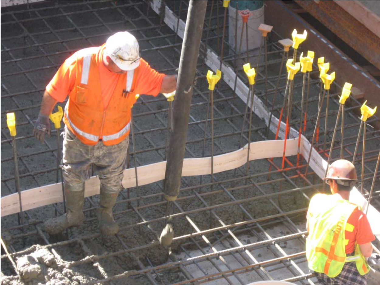
Water stops, and steel reinforcing as concrete pour begins.
