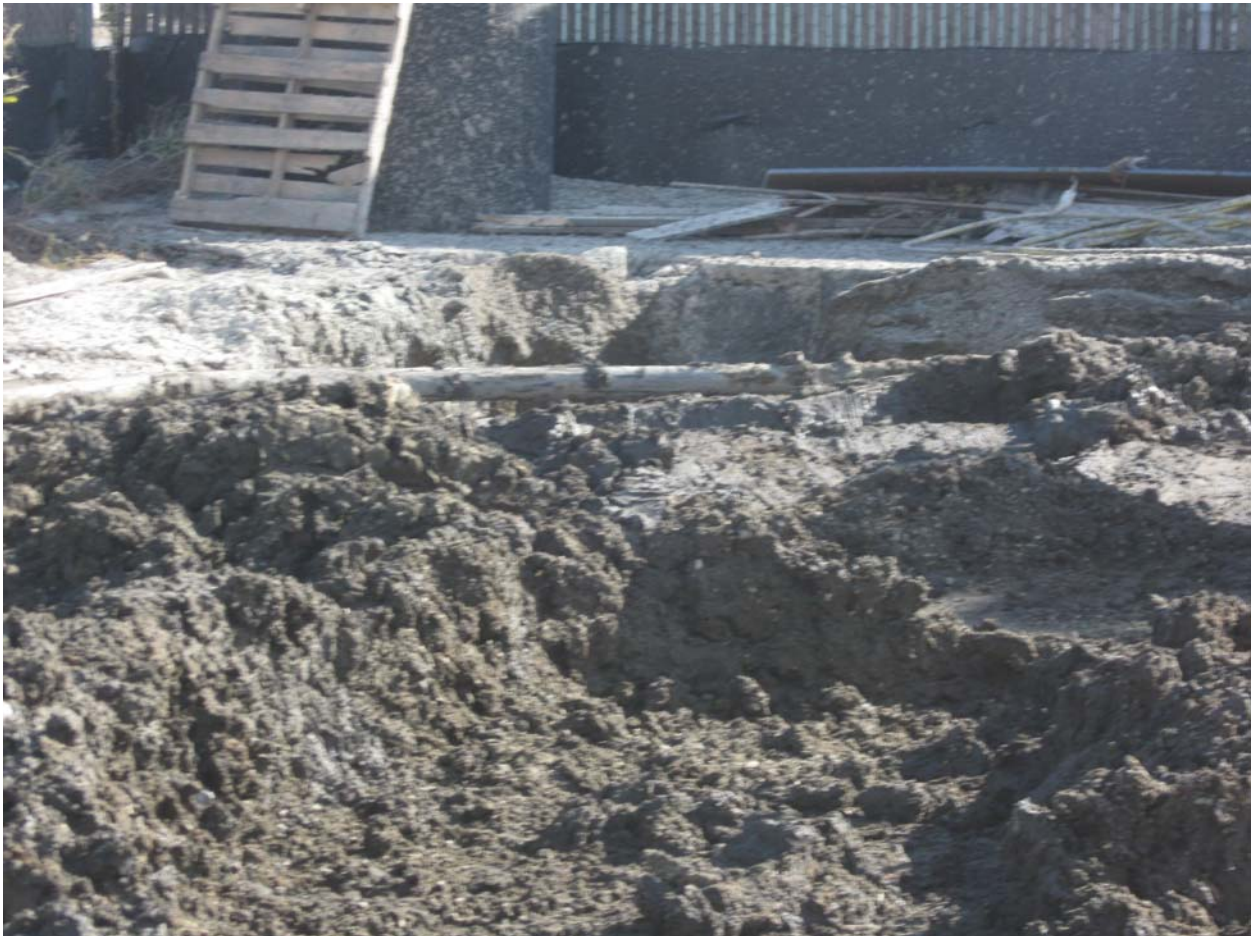
Completed square corner at station 11+18.
