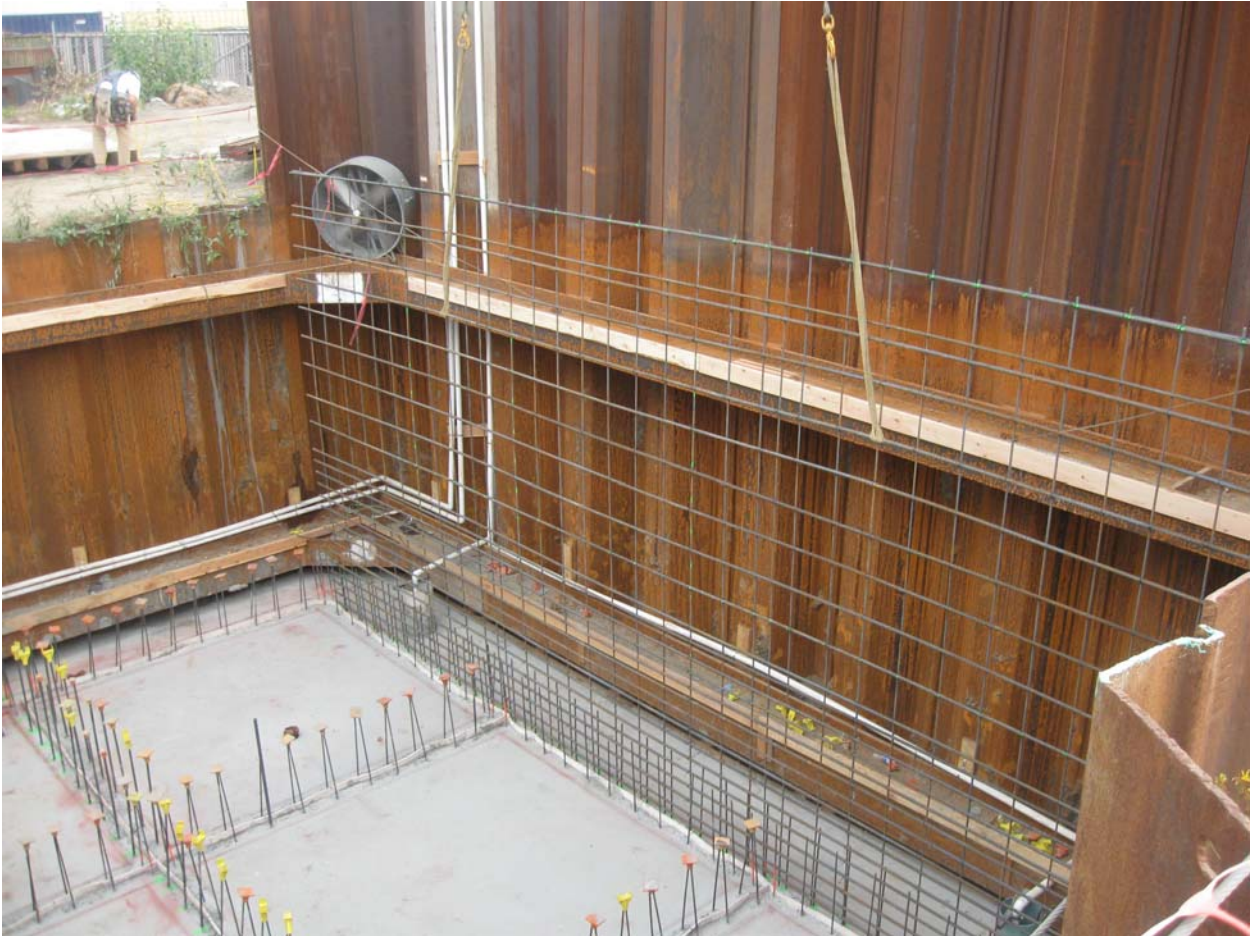
Initial set of east wall rebar.
