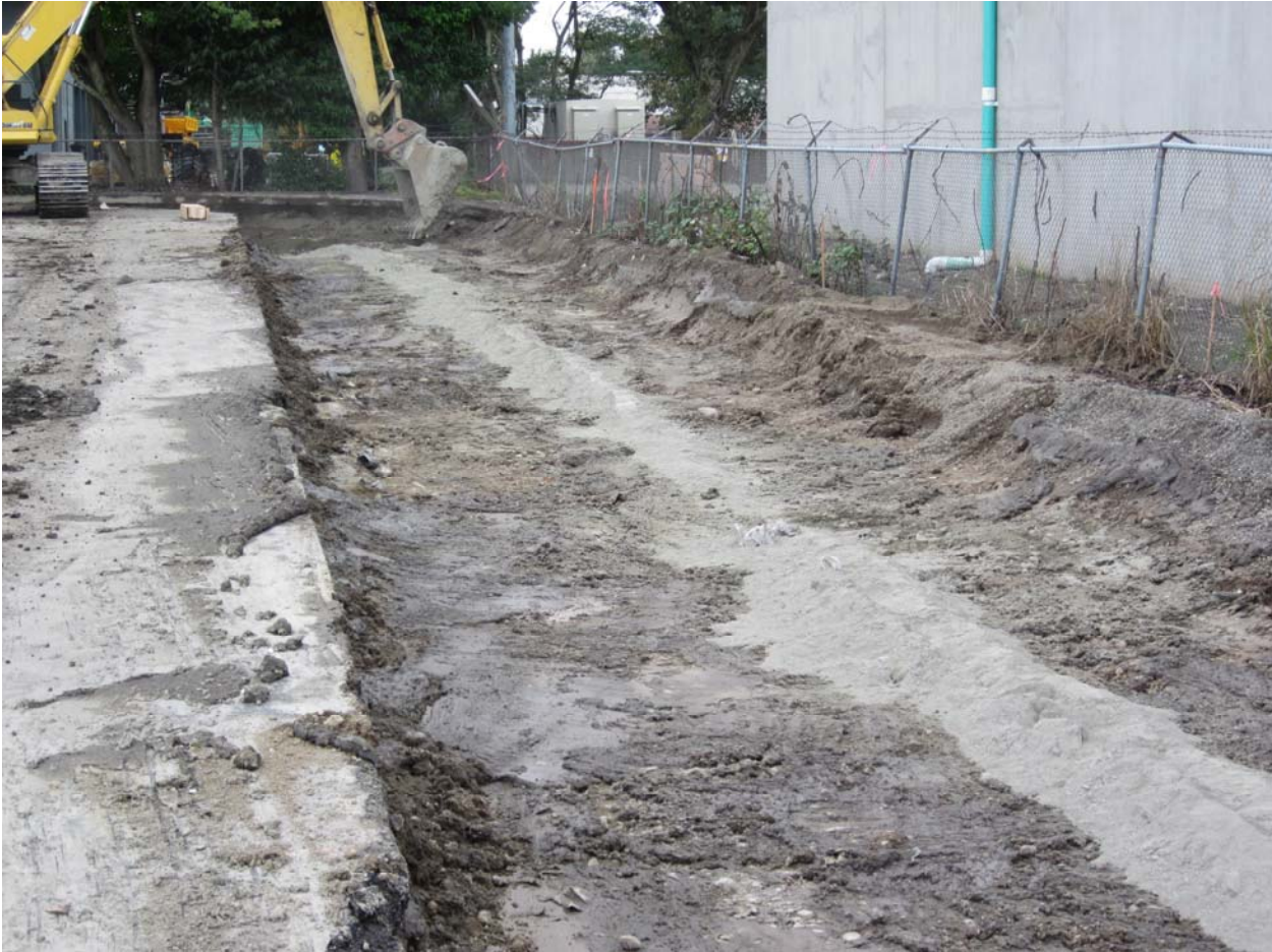
Preparing for cement stabilization of top of slurry wall station 1+50 to 2+50.
