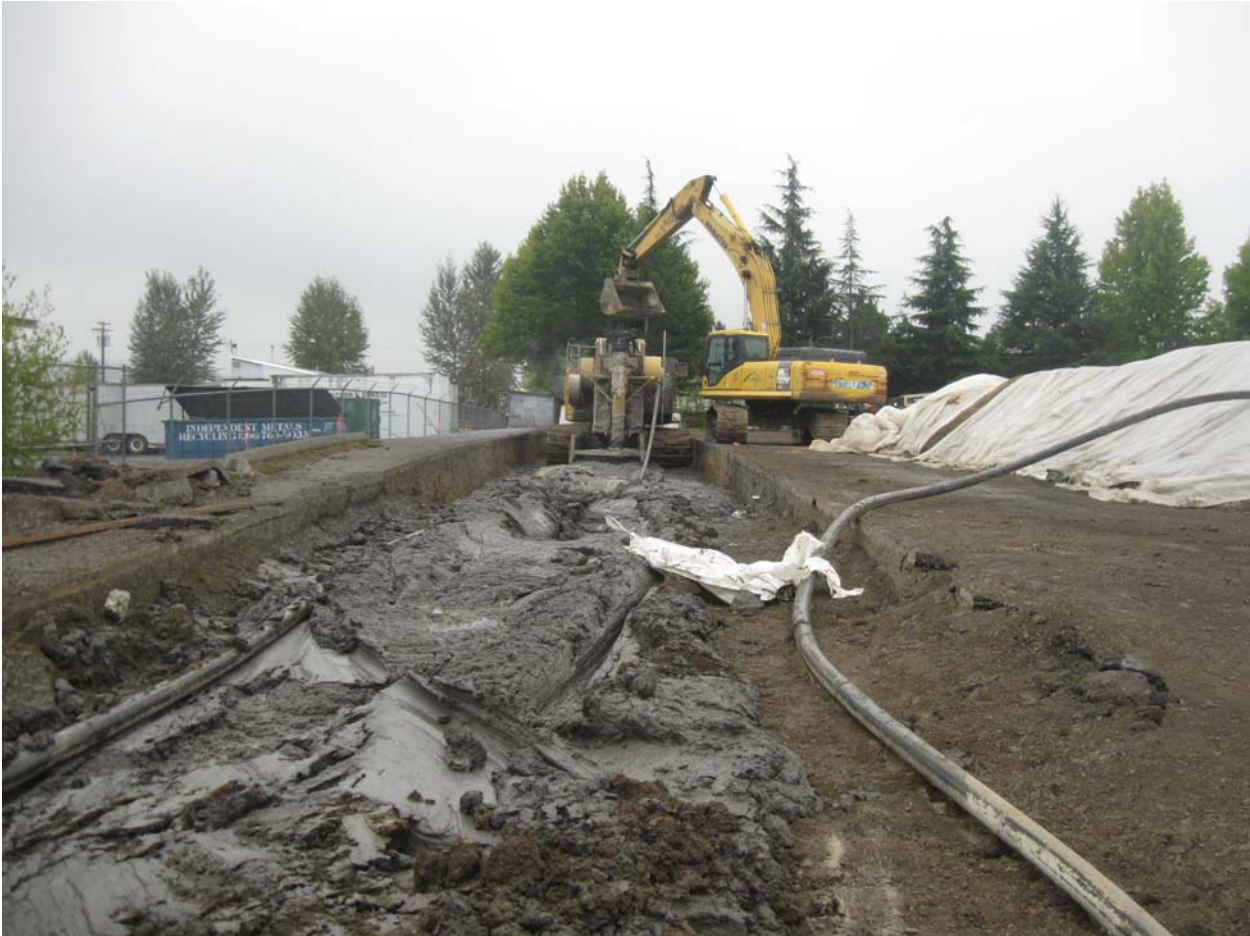
Wall from about station 12+20 to 13+20.
