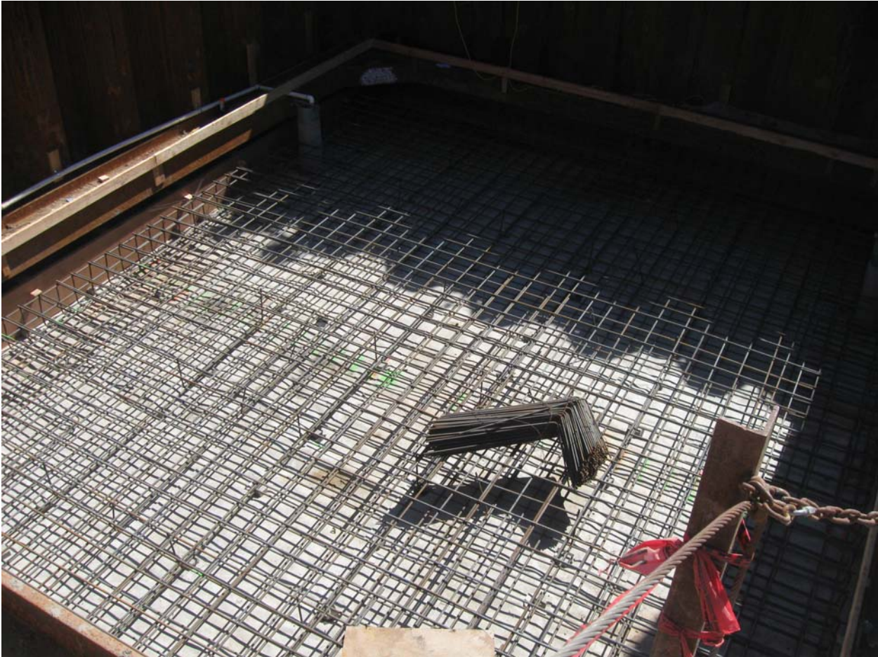
Steel progress as of 1:00 PM Friday.
