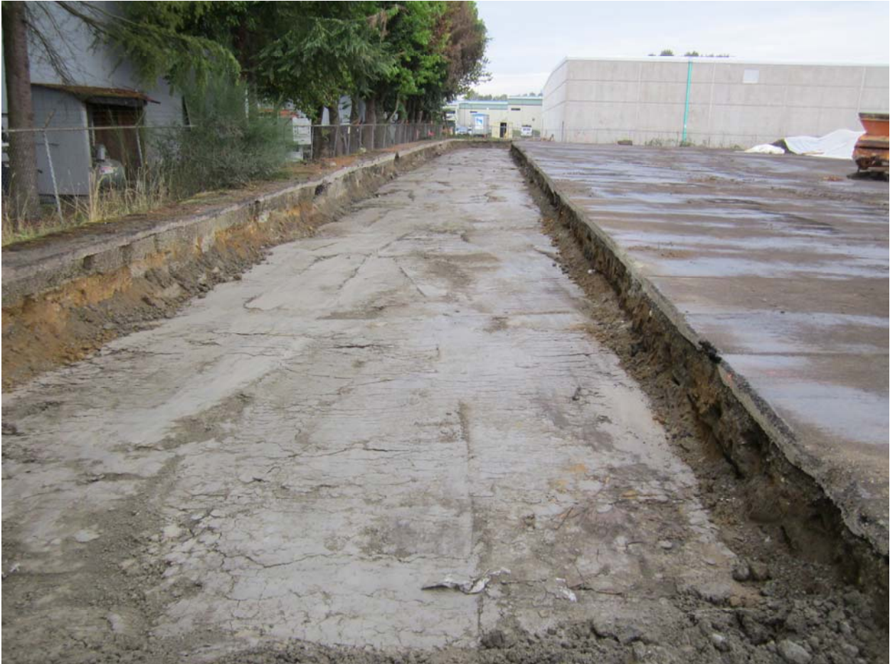
Key trench 0+00 to 1+50 prepared and ready for PVC liner installation.
