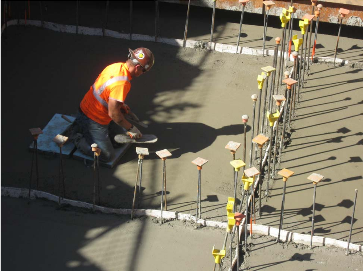
Hand finishing last poured chamber.
