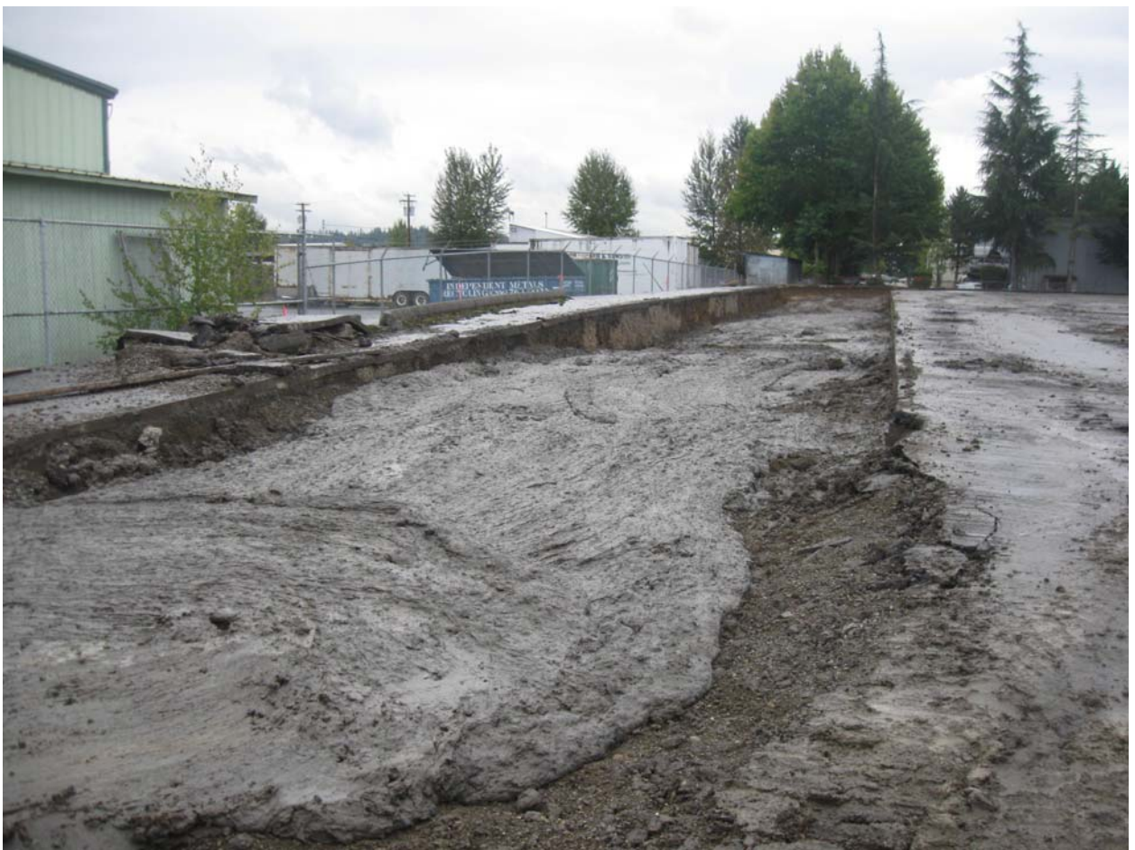
Slurry spread in key trench at station 12+25.
