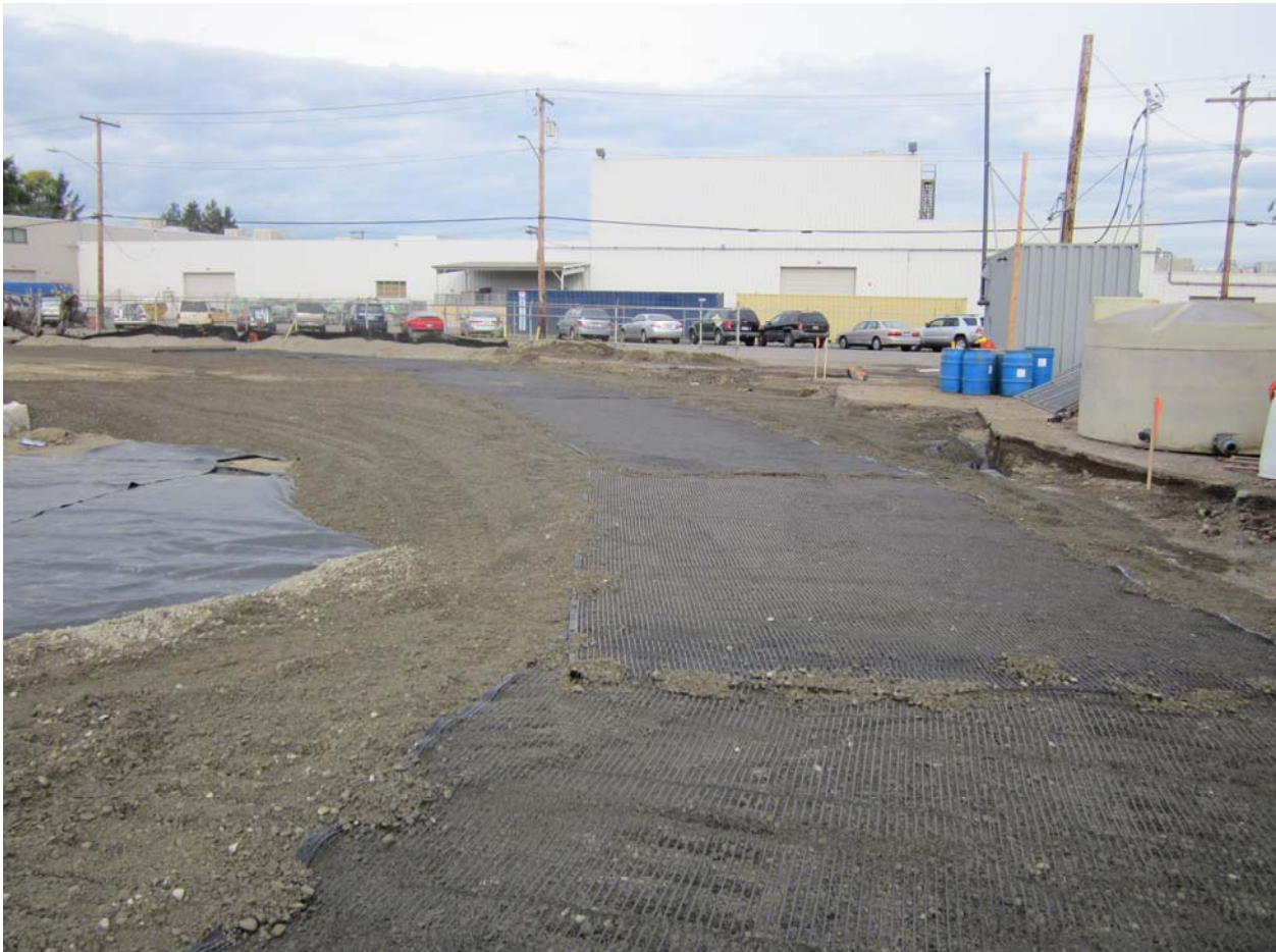
Geogrid over slurry wall
