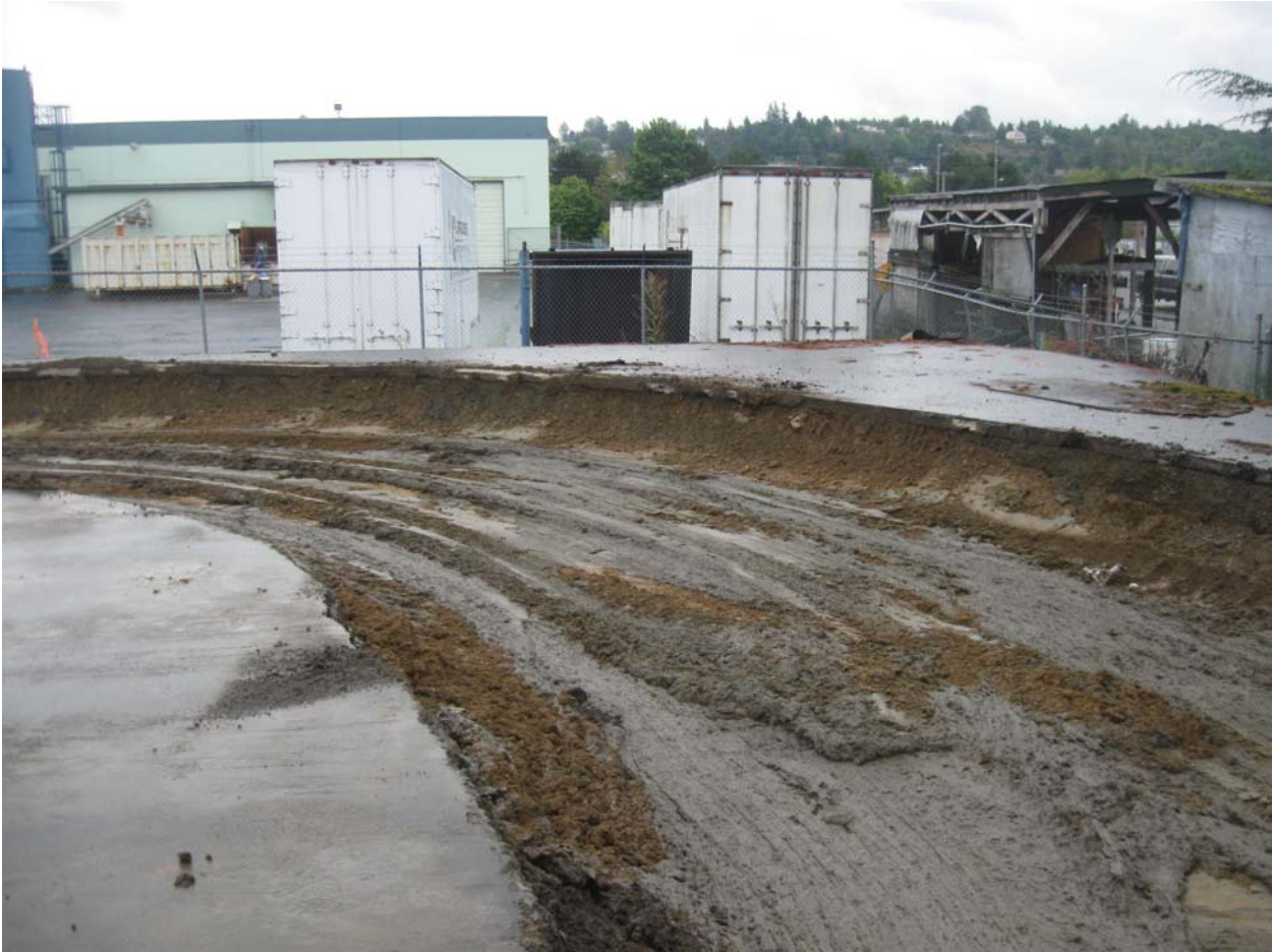
Slurry spread in key trench at southeast corner.
