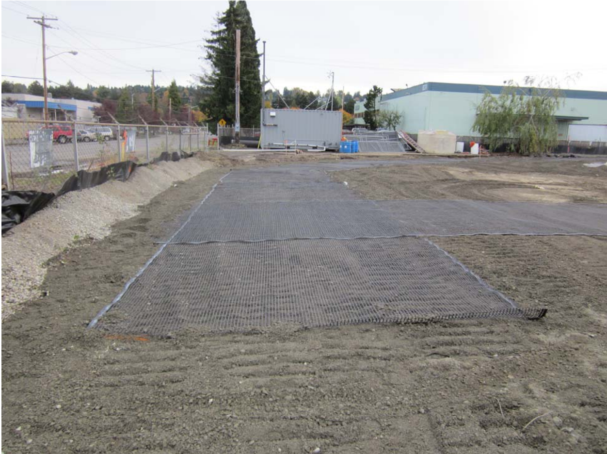
Geogrid over slurry wall.
