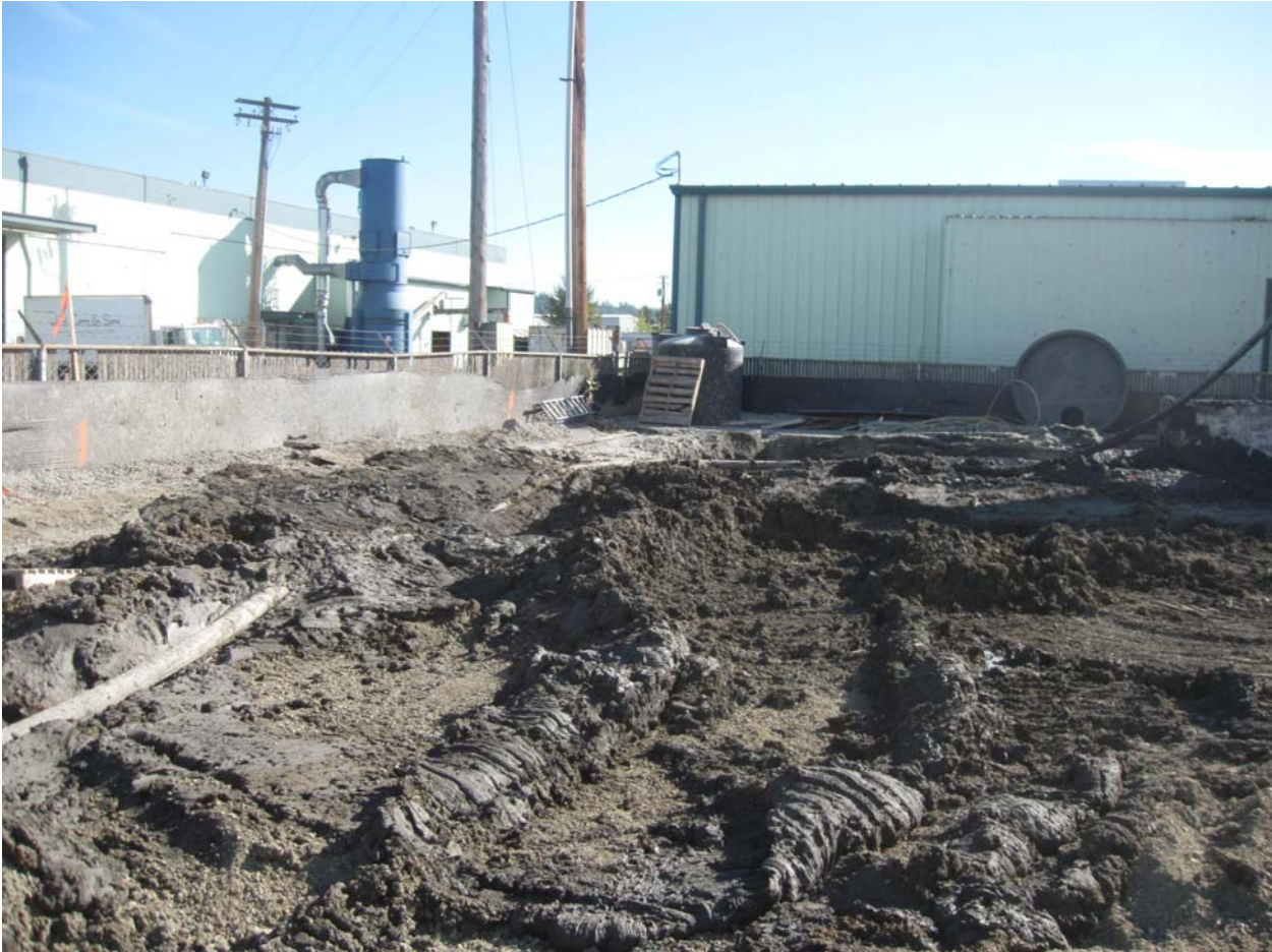
Wall at station 10+75 to 11+18.
