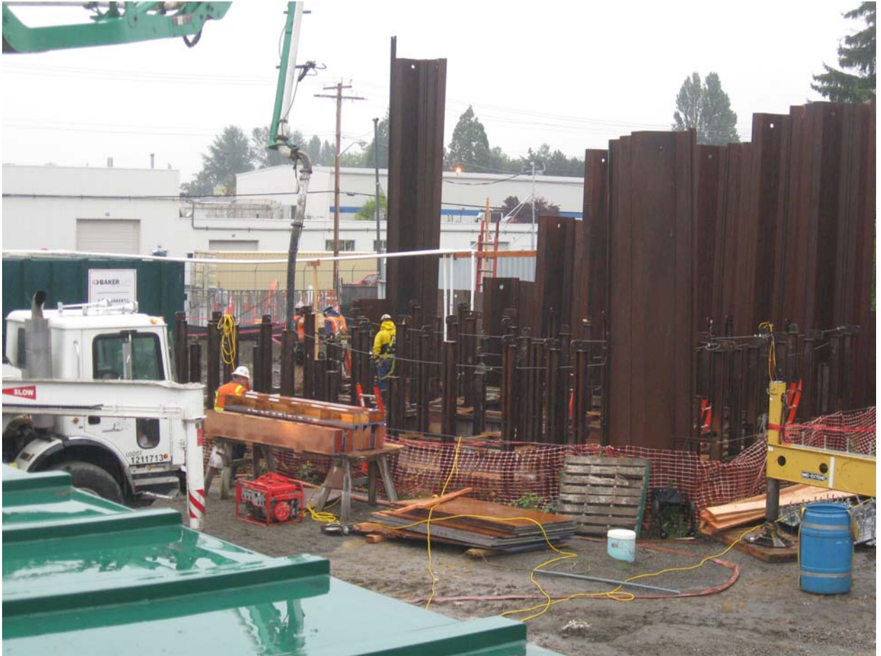
Ongoing concrete placement for vault walls.
