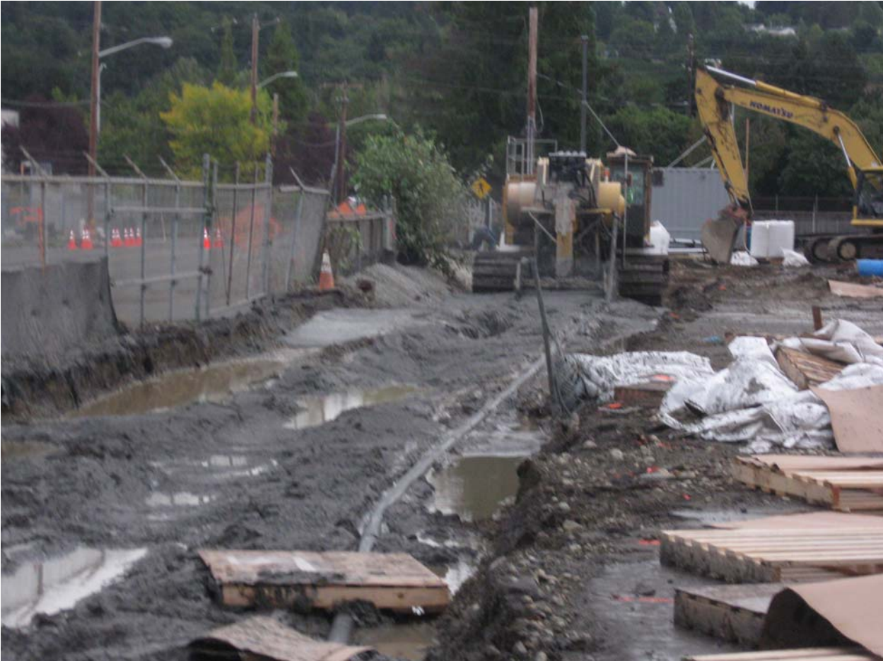
Progress as of 6PM 9/26.
