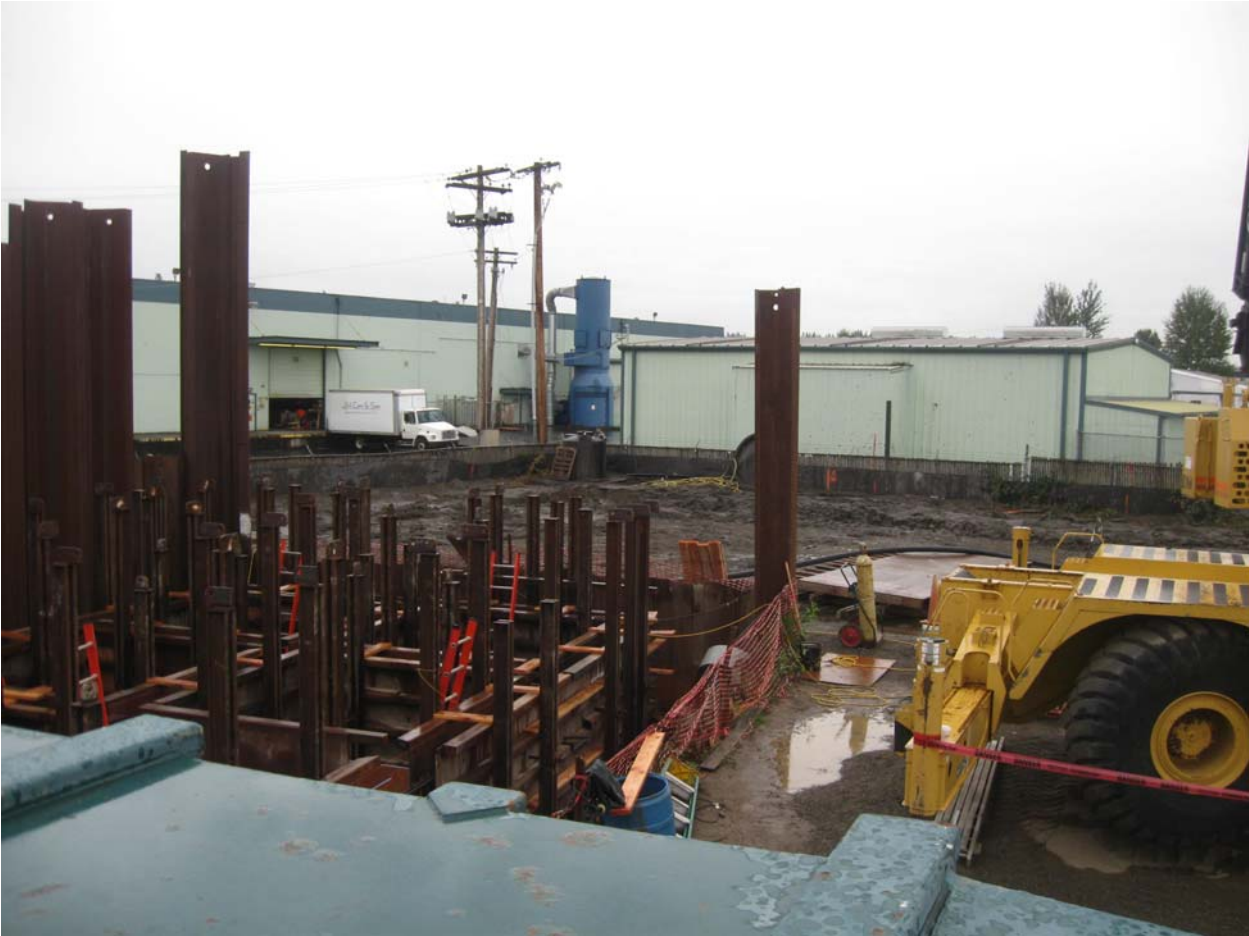
Vault forms nearing completion.
