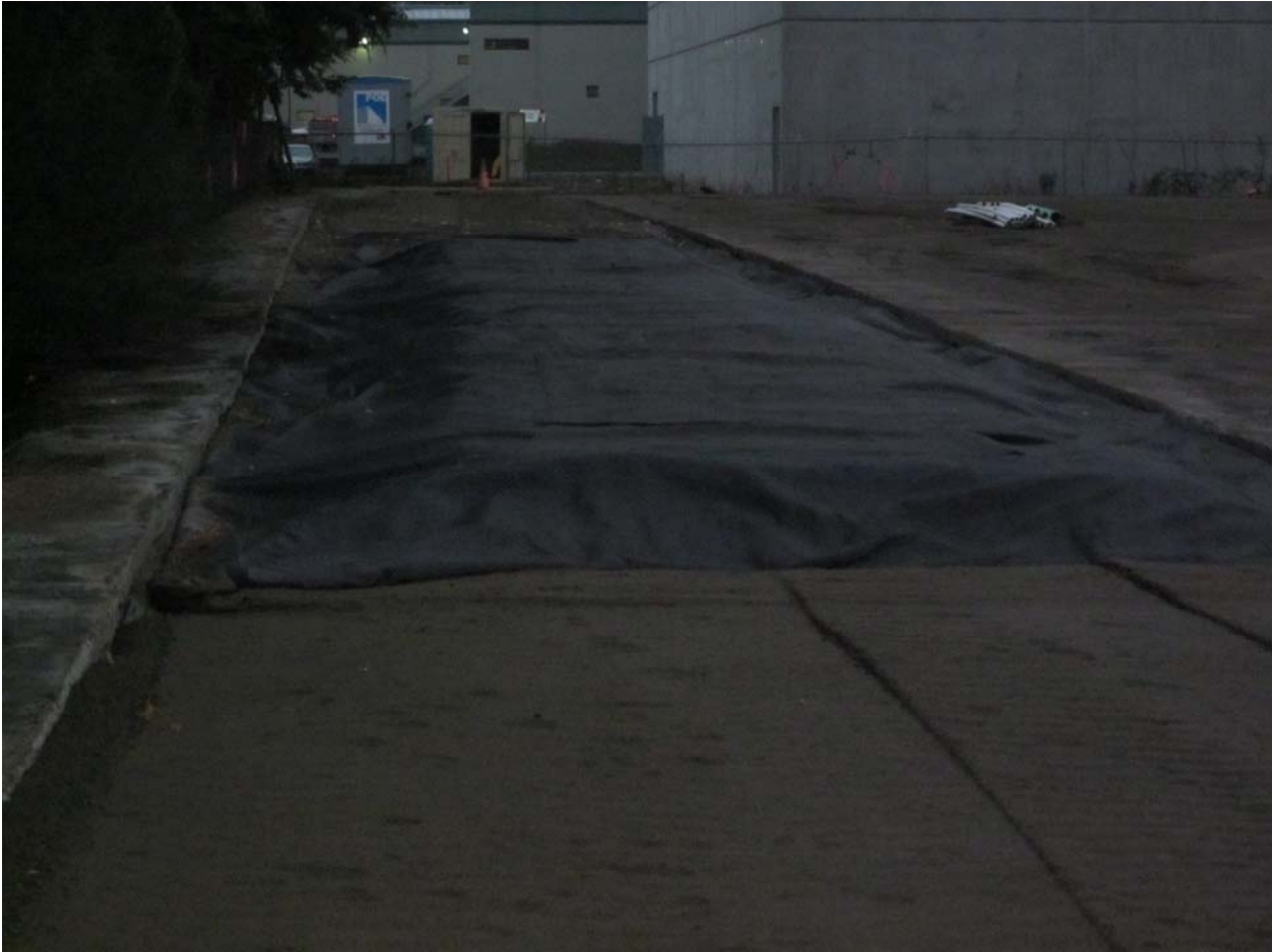
Raised area of burrito at about station 0+00.
