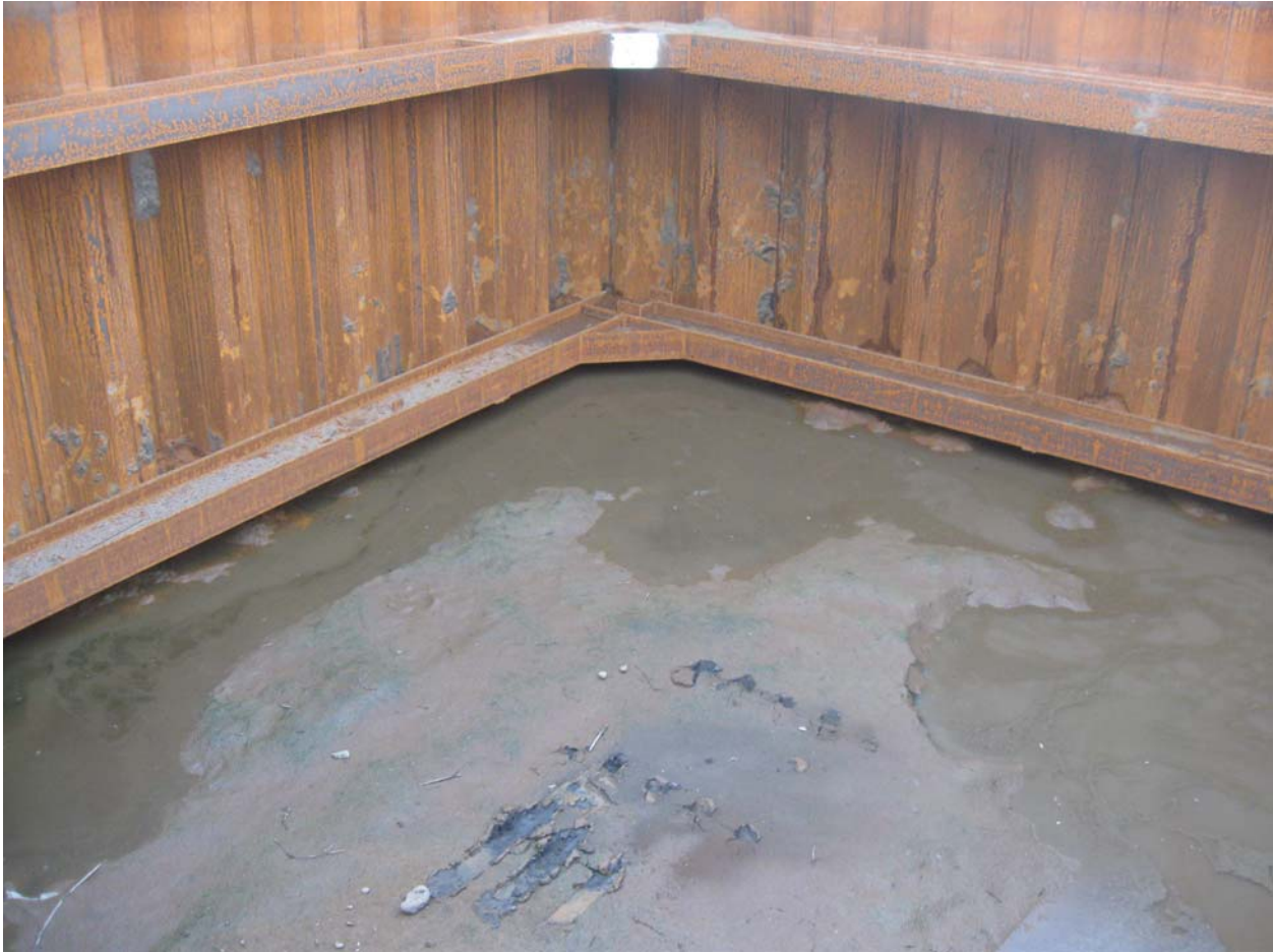
White paint on top whaler is where elevations were established.
