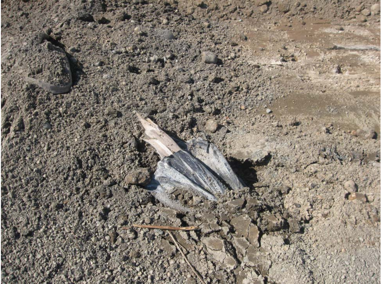
PVC liner at Station 3+65 + or -.
