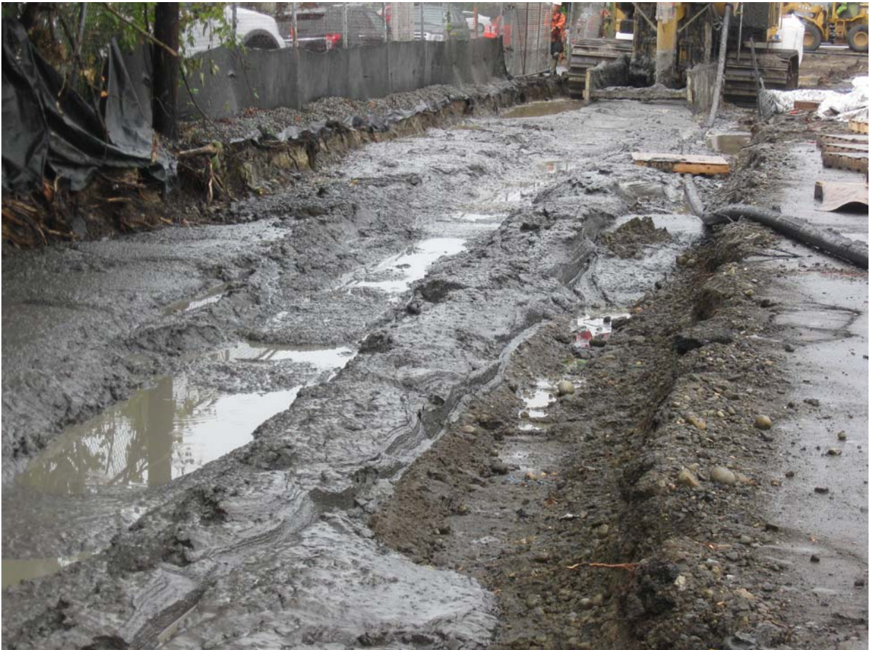
Installing slurry wall in rainy conditions.
