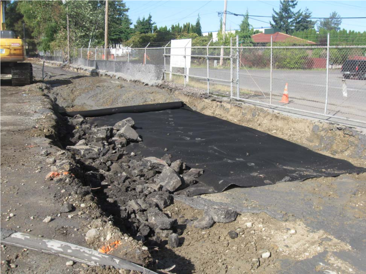
Start of road crossing construction at west gate.
