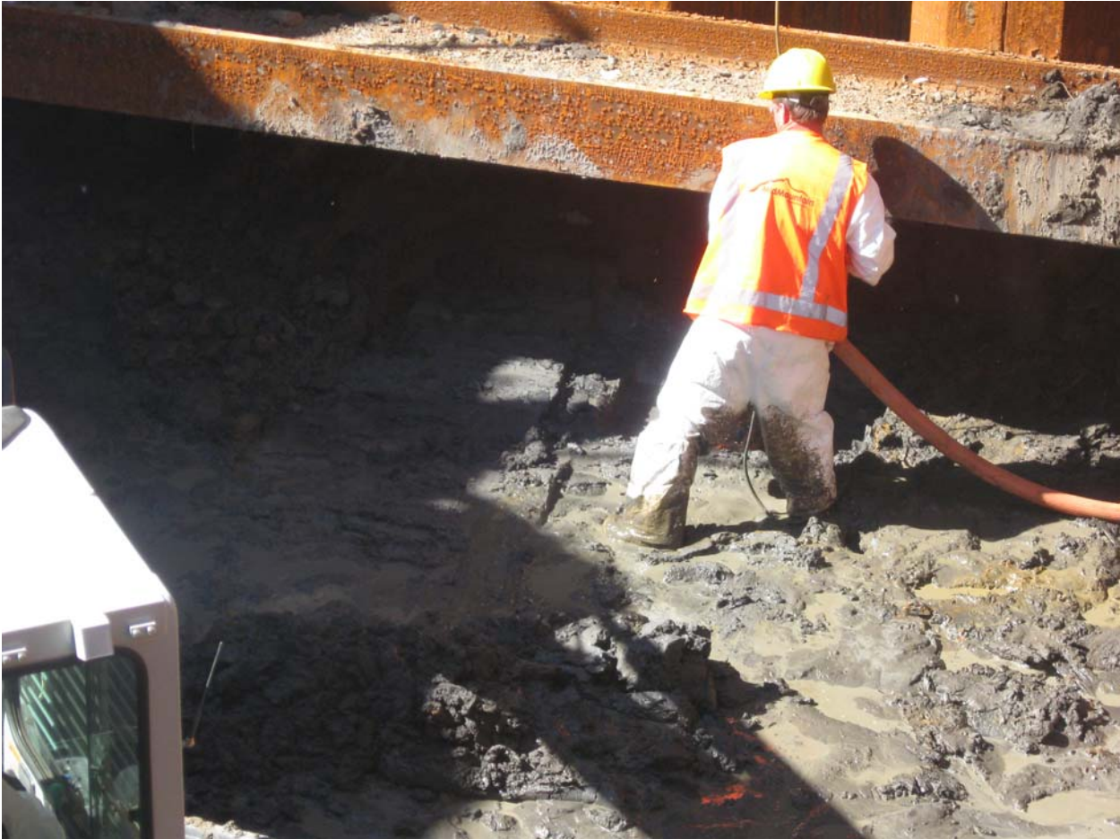
Setting sump pump in excavation.
