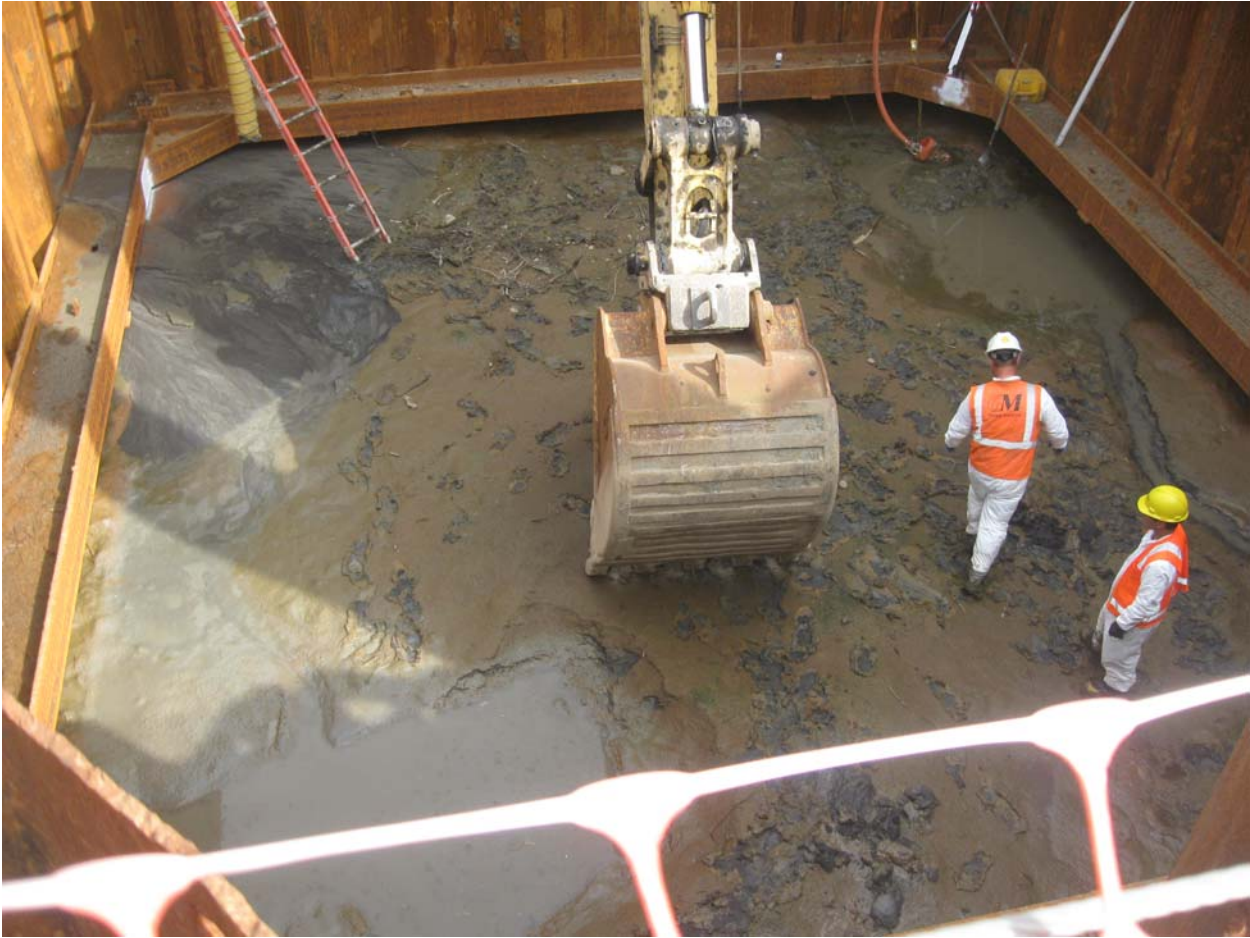
Beginning excavation to elevation 9.75.
