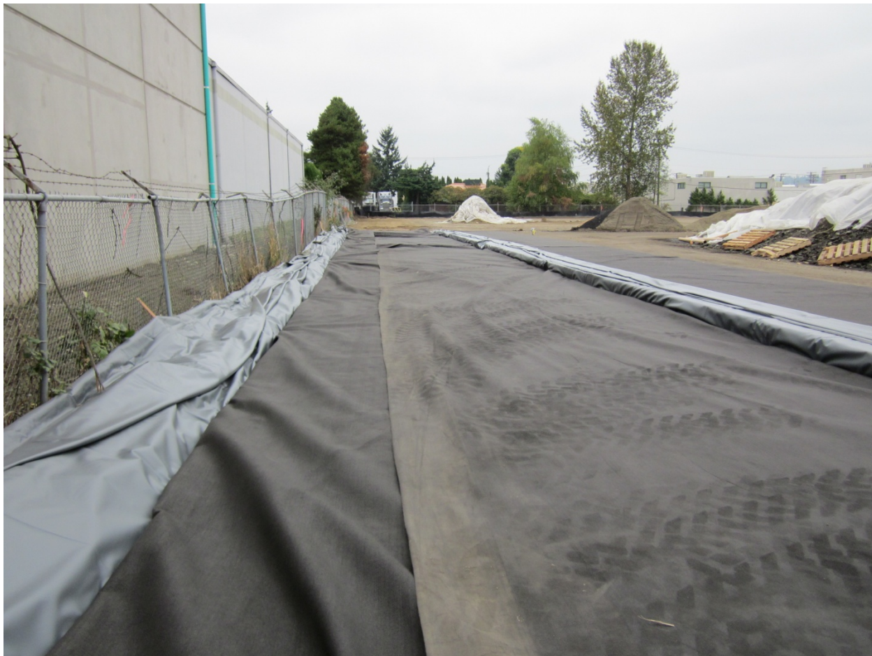
Backfilled burrito with geotextile covering cement stabilized sludge.
