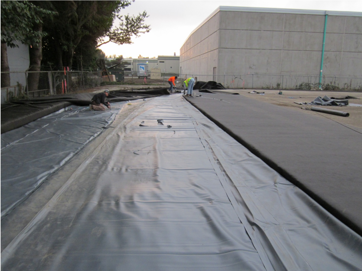
• Top layer of PVC burrito at southwest corner.
