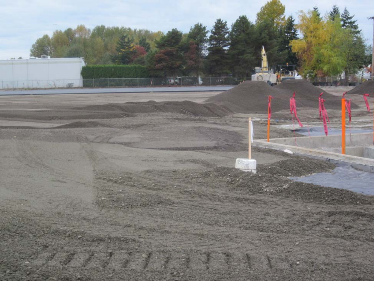
Ongoing placement of aggregates around vault area.
