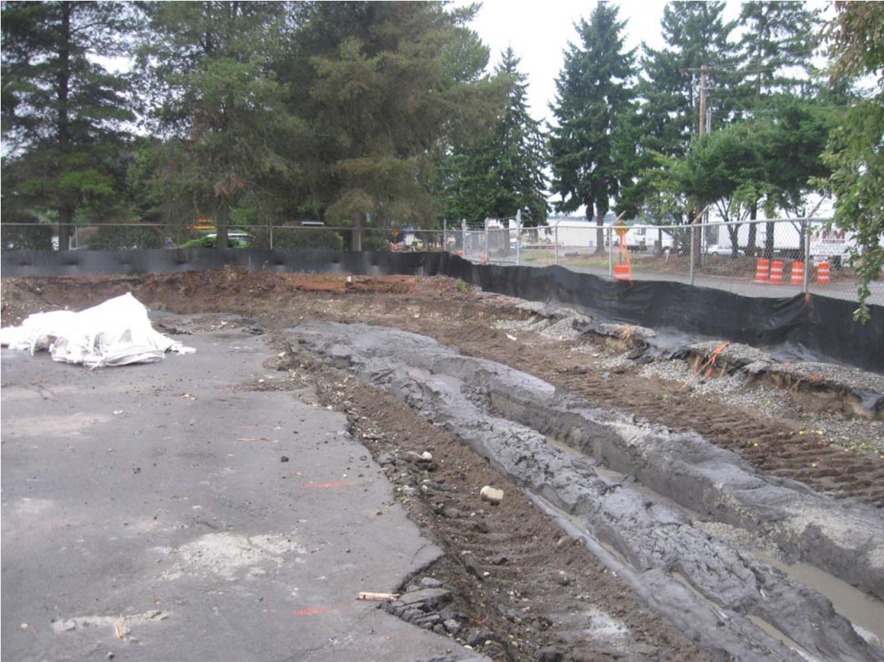
Slurry wall at northwest corner of site.
