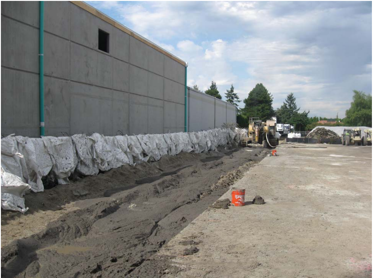
Trench completed to approximately 3+00.
