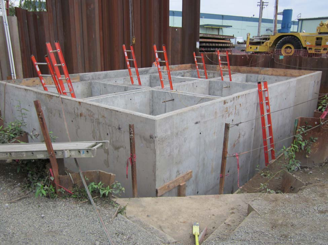
Key trench with crushed aggregate placed station 3+70 to 1+75
