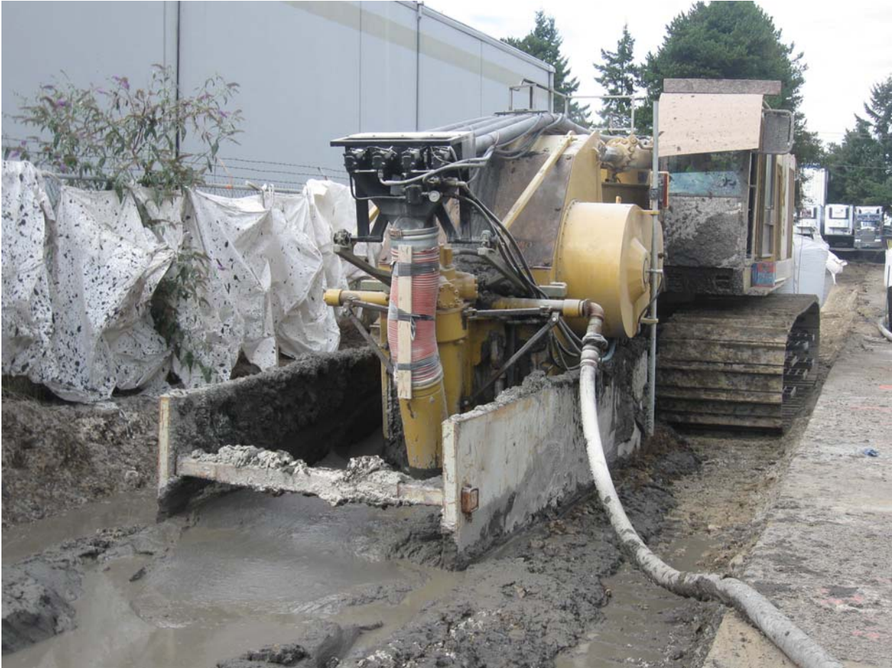
Trencher working at maximum cutting depth.
