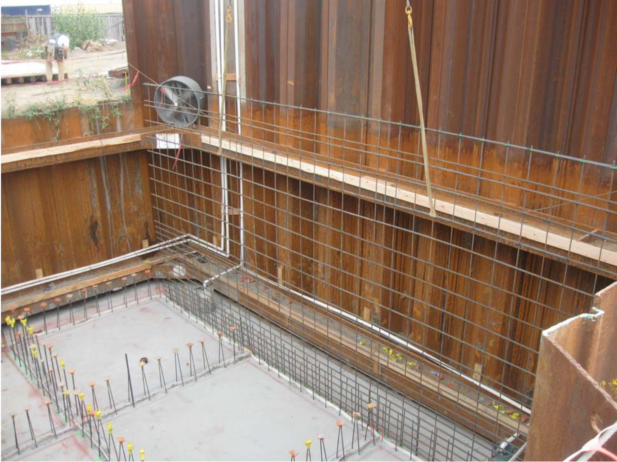
Initial set of east wall rebar.
