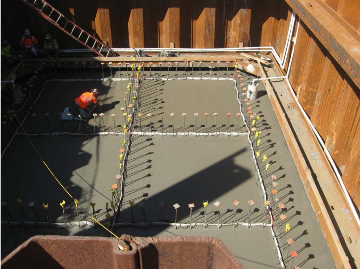
Nearly completed base slab pour.
