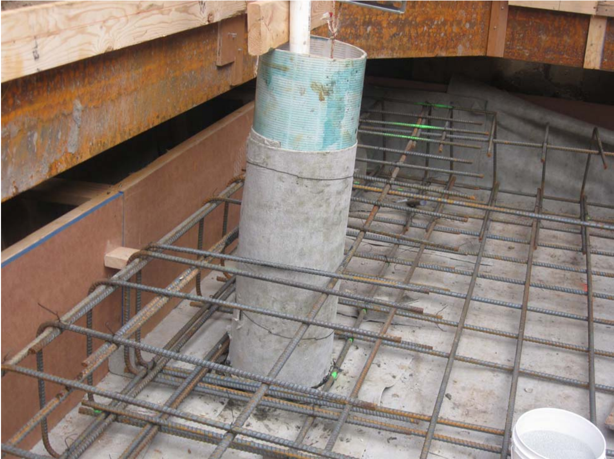
Water stop extended up side walls of vertical well casings.
