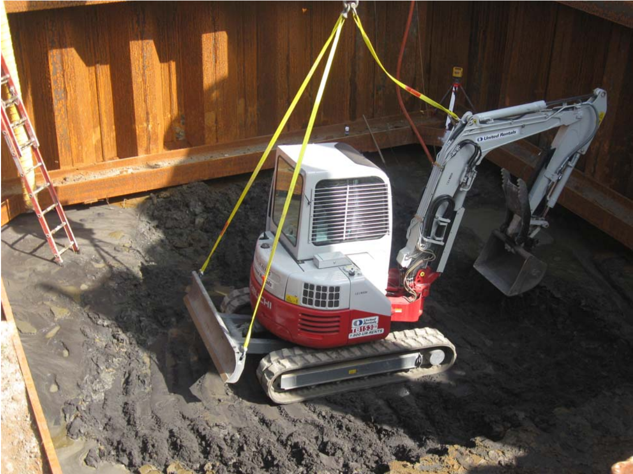
Lowering mini-excavator into excavation to assist with excavation.
