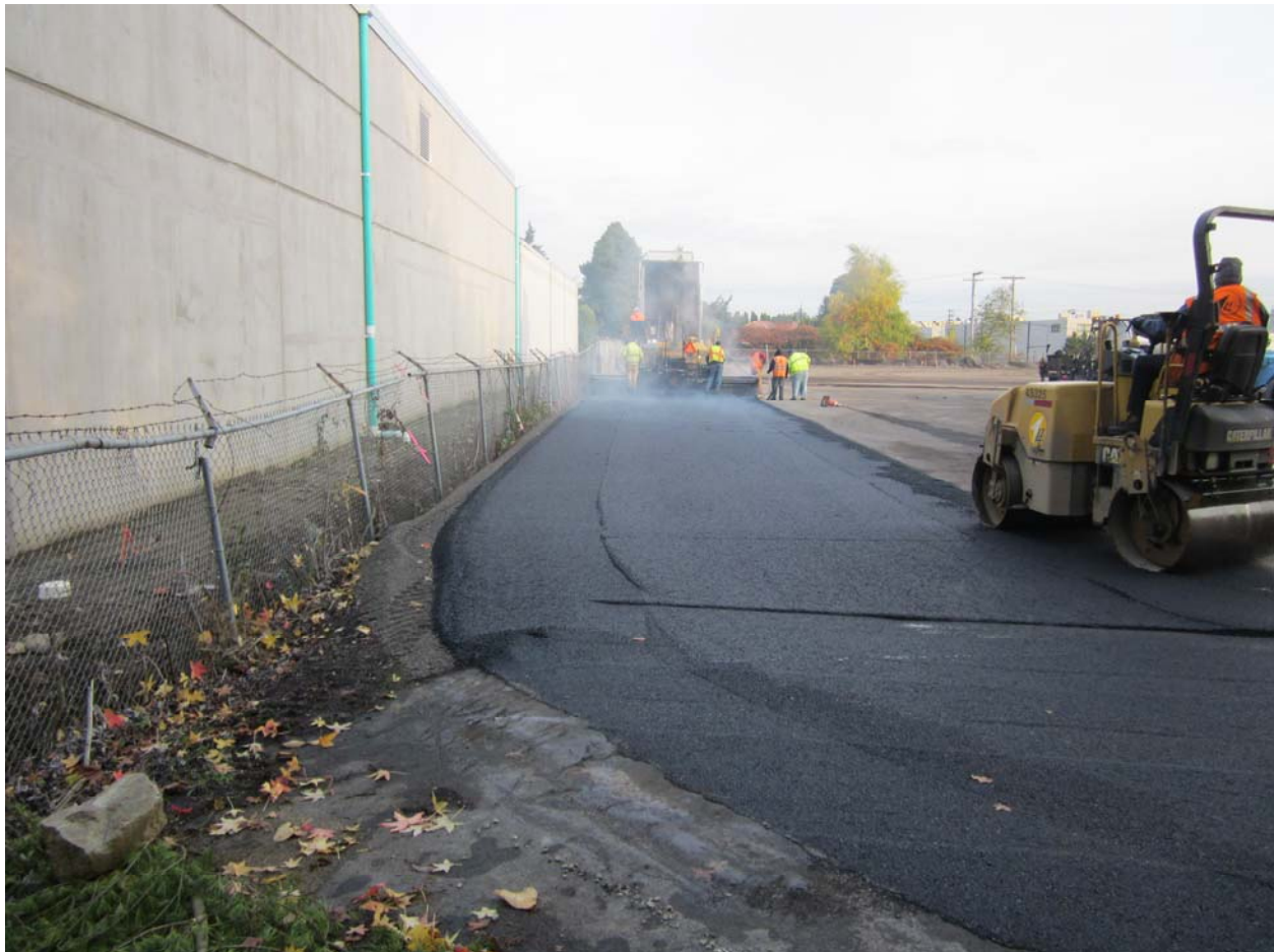
Paving key trench southwest corner.
