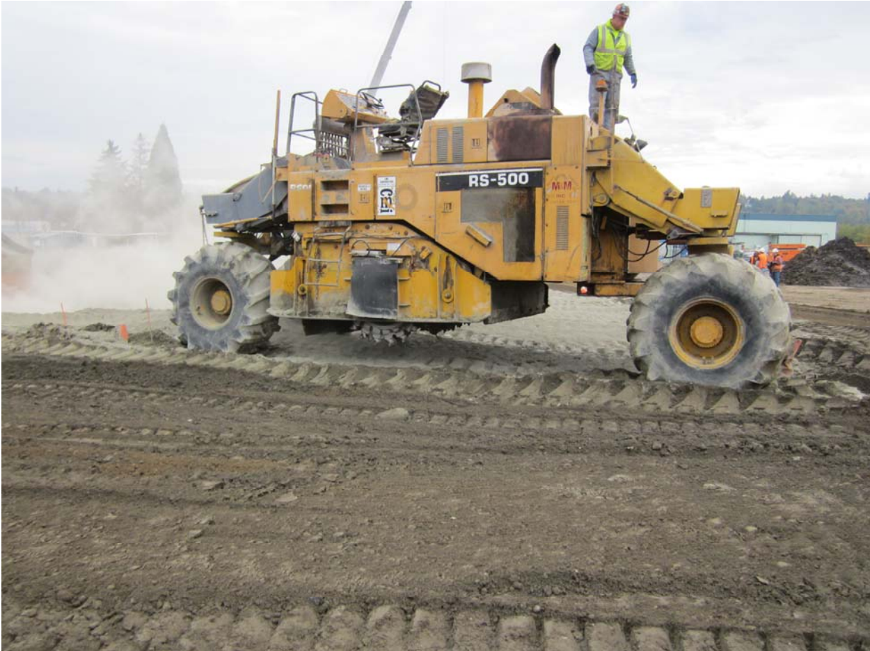
Machine used to mix cement with soft subgrade soil.
