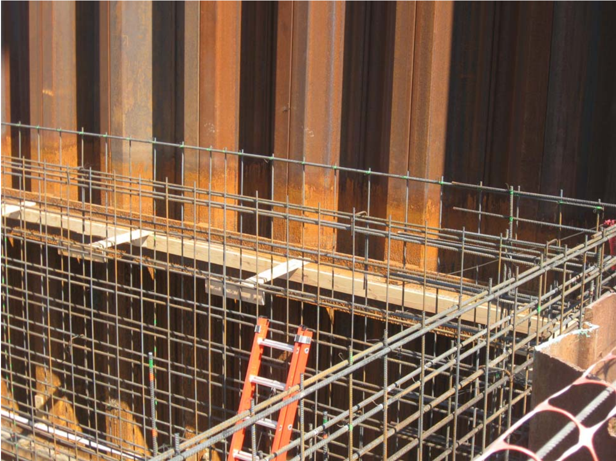
Interior and exterior steel on southeast corner of vault.
