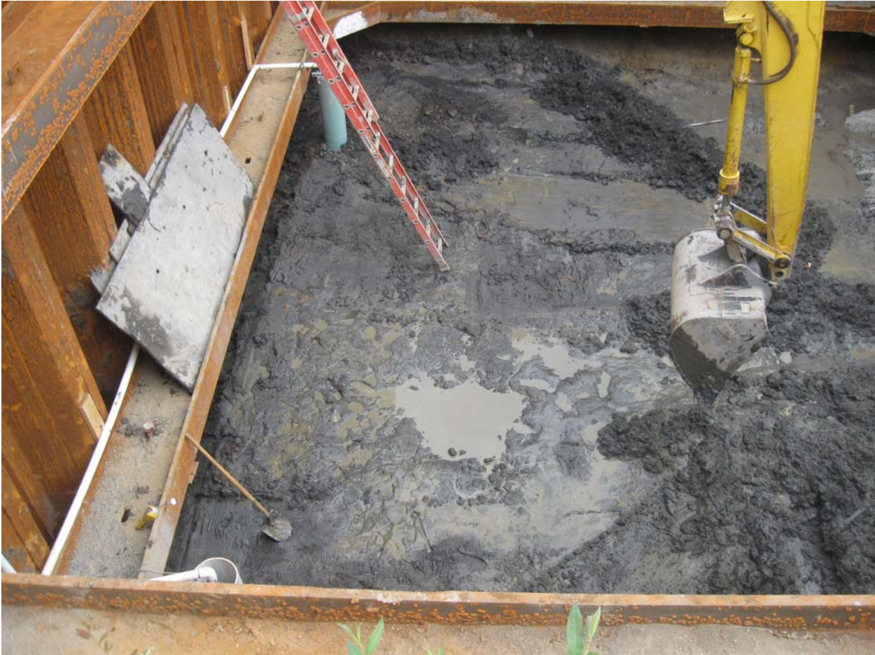
Continued excavation following dewatering well installation.
