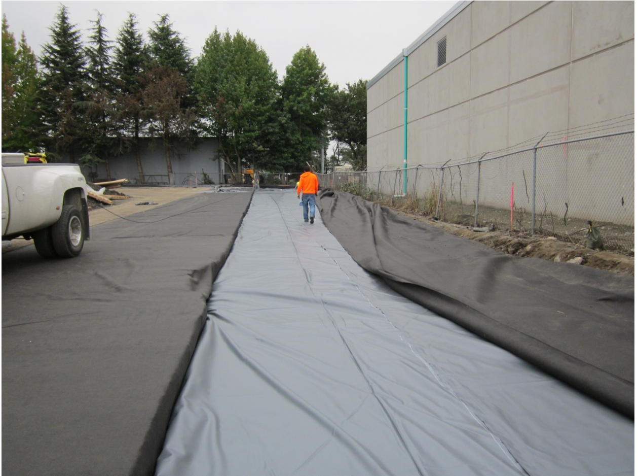
PVC covered waste before placing top layer of geotextile.
