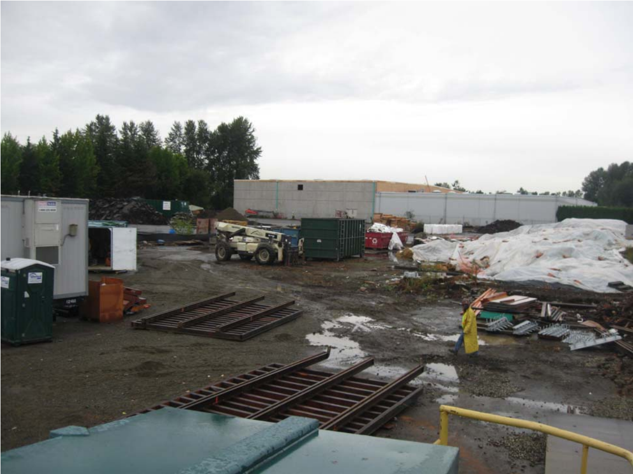
General site conditions 10/03/11.
