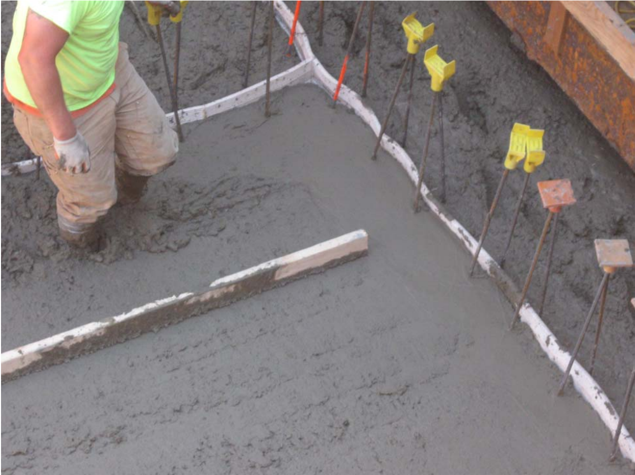
Roding final lift of concrete to grade.
