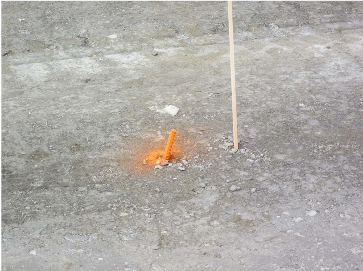
Example rebar on south side of buried well.
