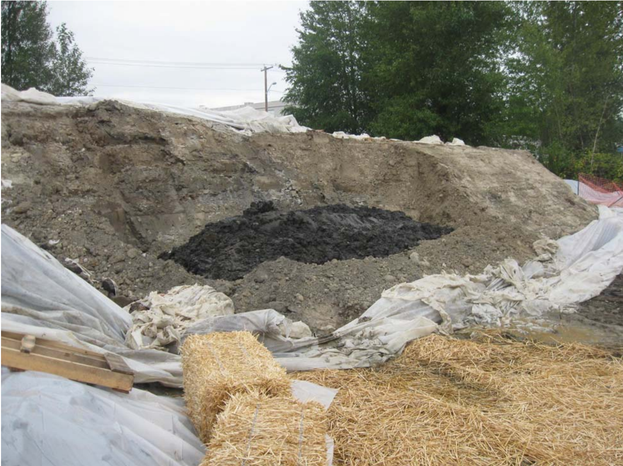
Excavation spoils inside soil berm.
