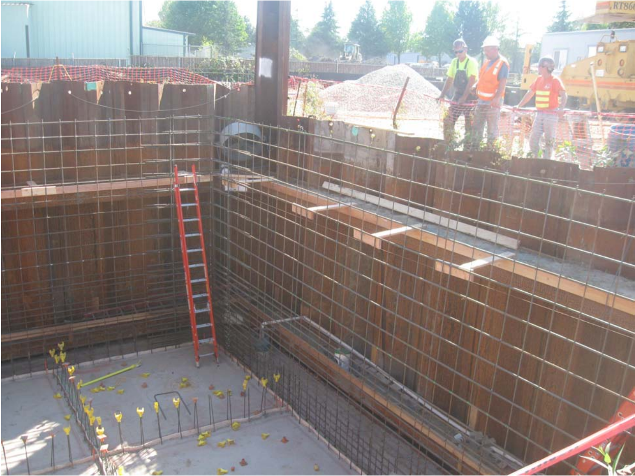
Continued steel erection for vault exterior walls.
