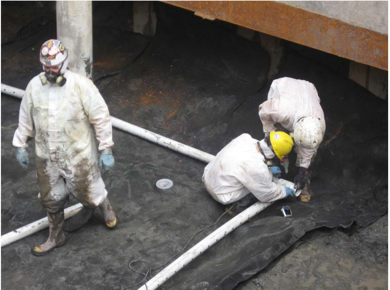
Perforated pipe being installed over geocomposite.
