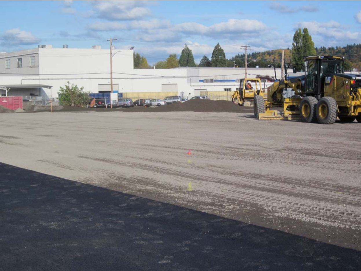
Ongoing Type 1 aggregate grading.
