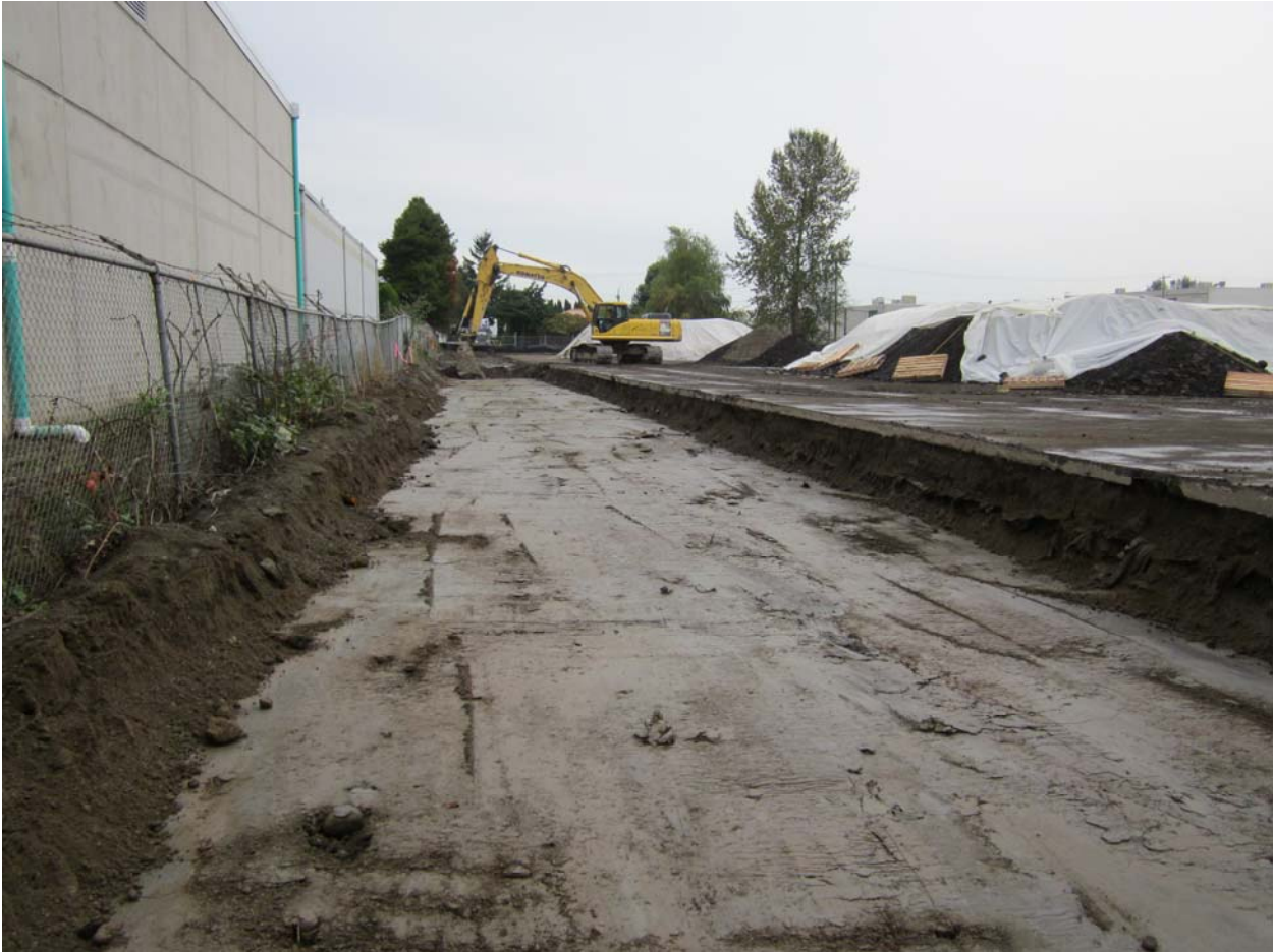
Key trench 1+50 to 3+70 prepared and ready for PVC liner installation.
