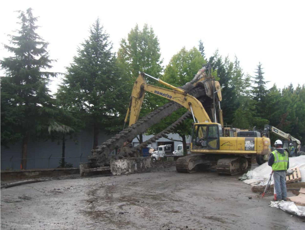
Pulling out of trench after completing wall.
