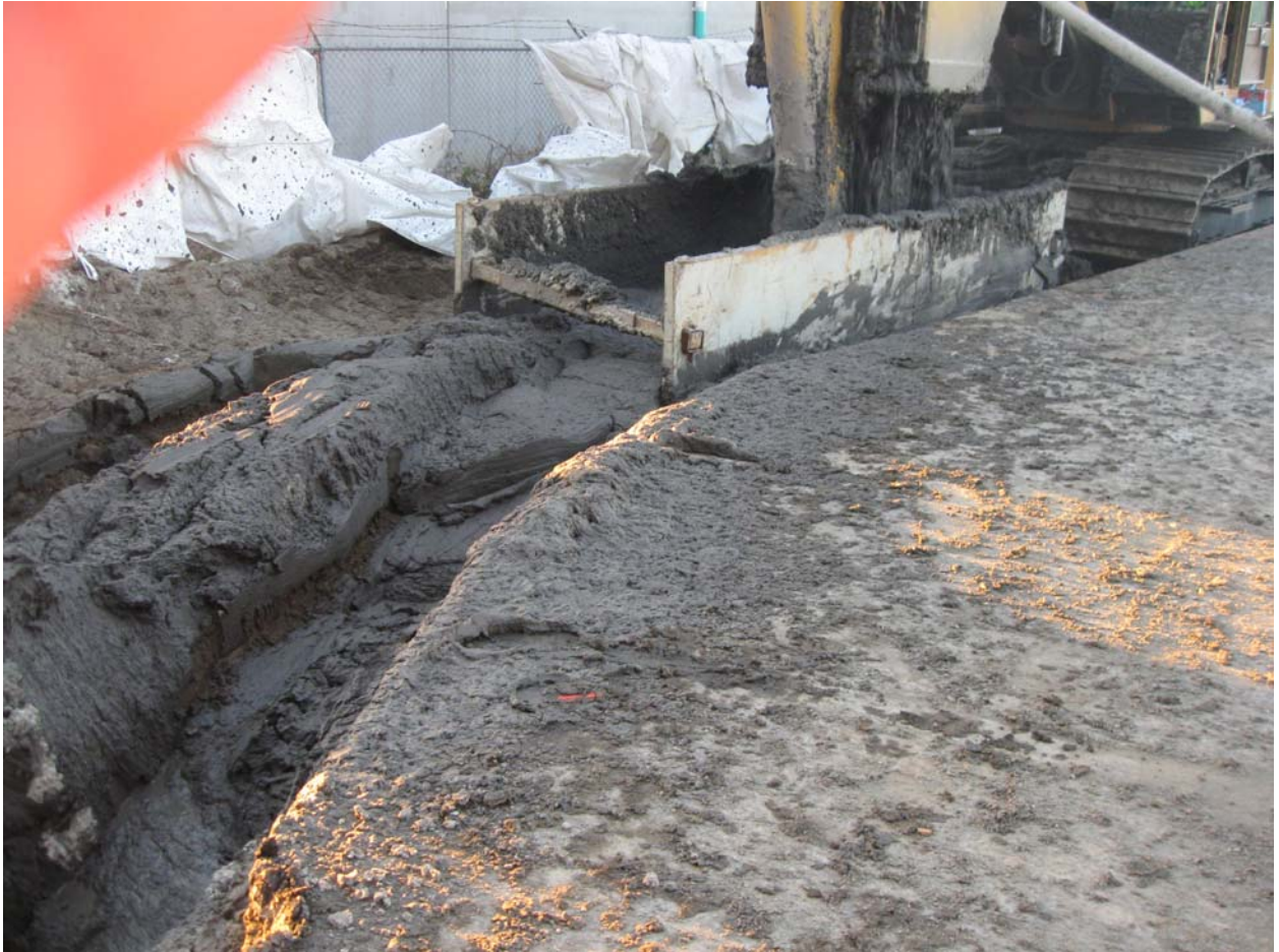
One pass trencher completing southwest corner.
