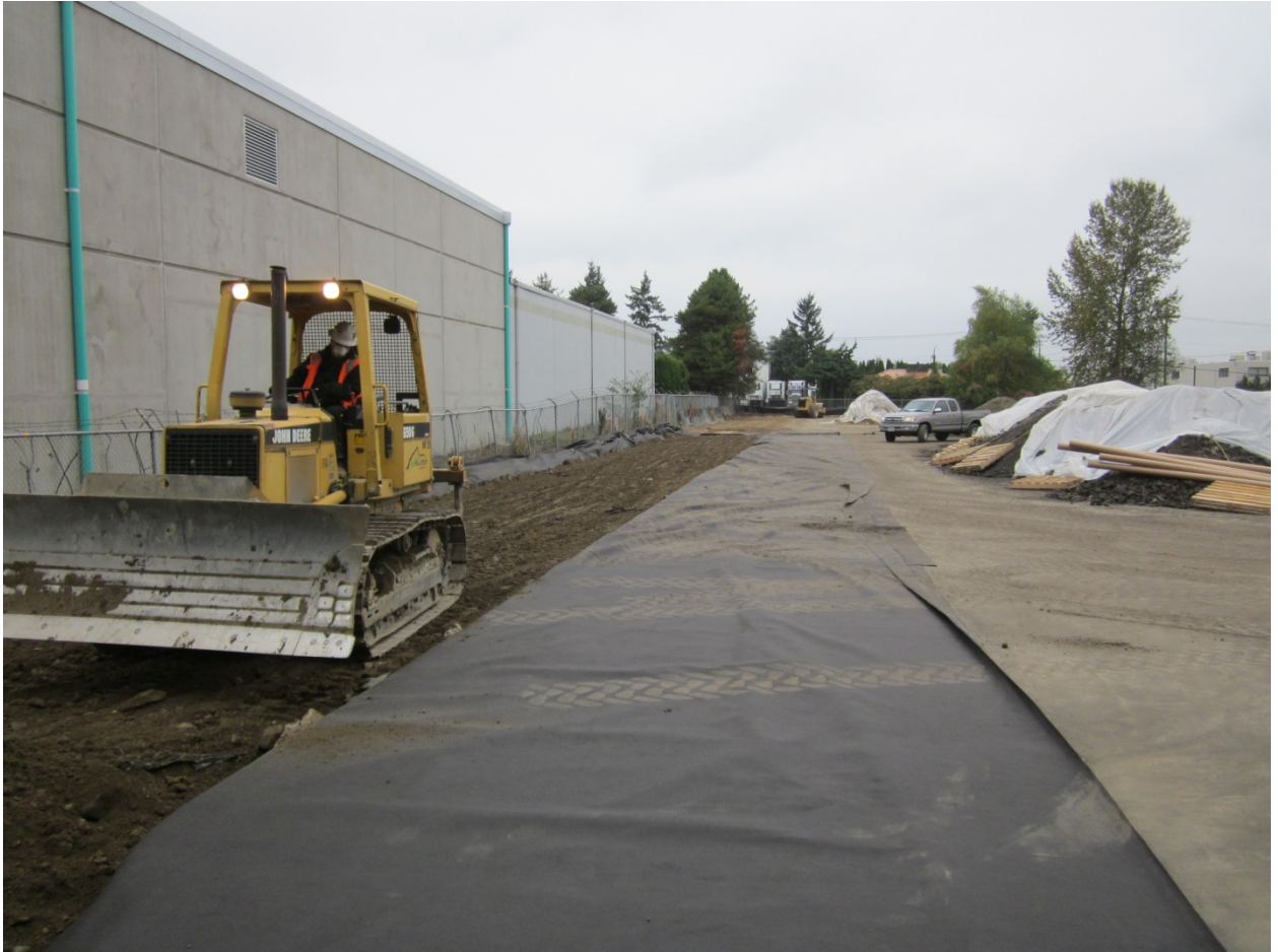
Placing cement treated waste into burrito.
