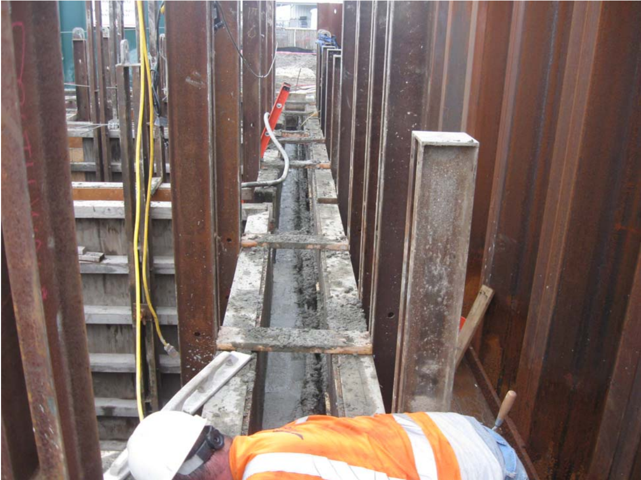
East wall floated to elevation of Nelson Studs.
