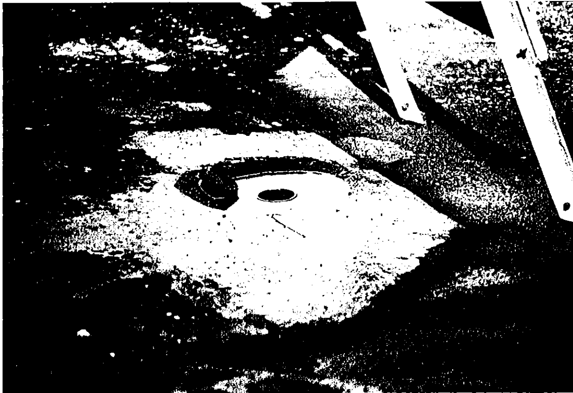
Waste Oil Underground Storage Tank (UST) Fill Receptacle
