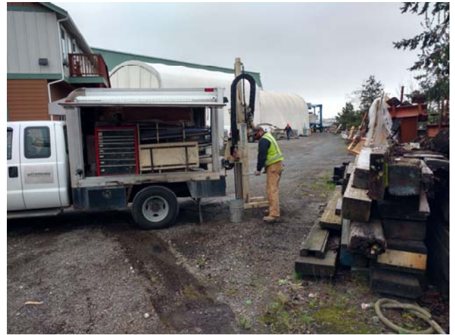
Direct Push Drilling at SB03 Location
