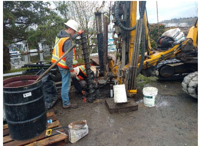
Hollow Stem Auger Drilling at MW4 Location
