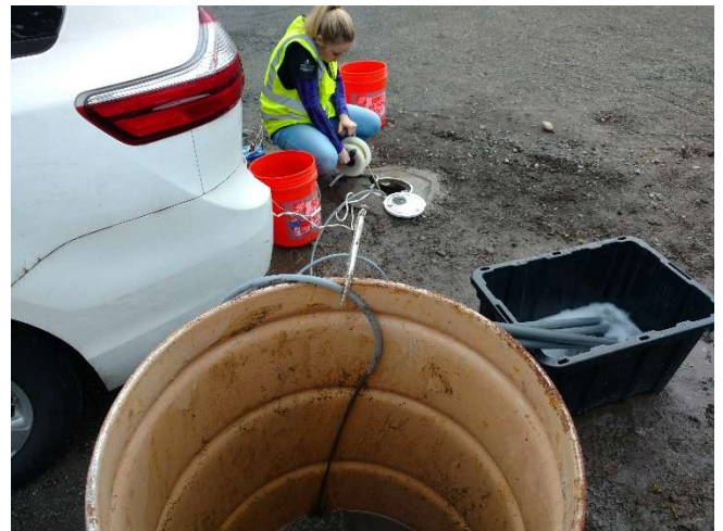
Gauging Well During the Development Process
