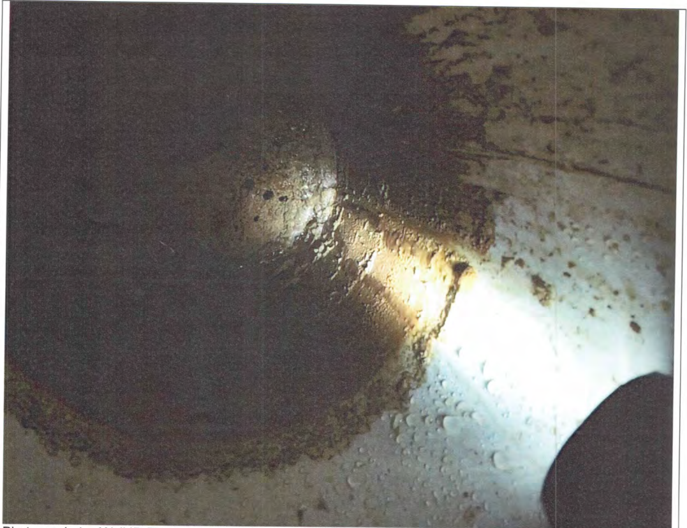
Photograph 4 Well ID EW-2, casing. May 18, 2016.
