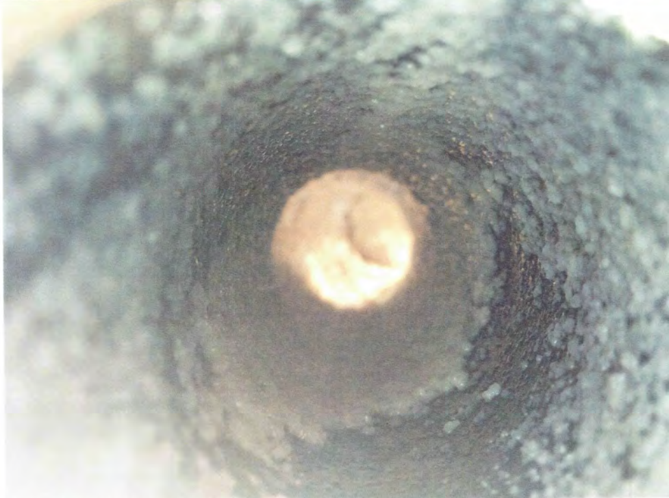
Photograph 1, extraction hose with biological growth
