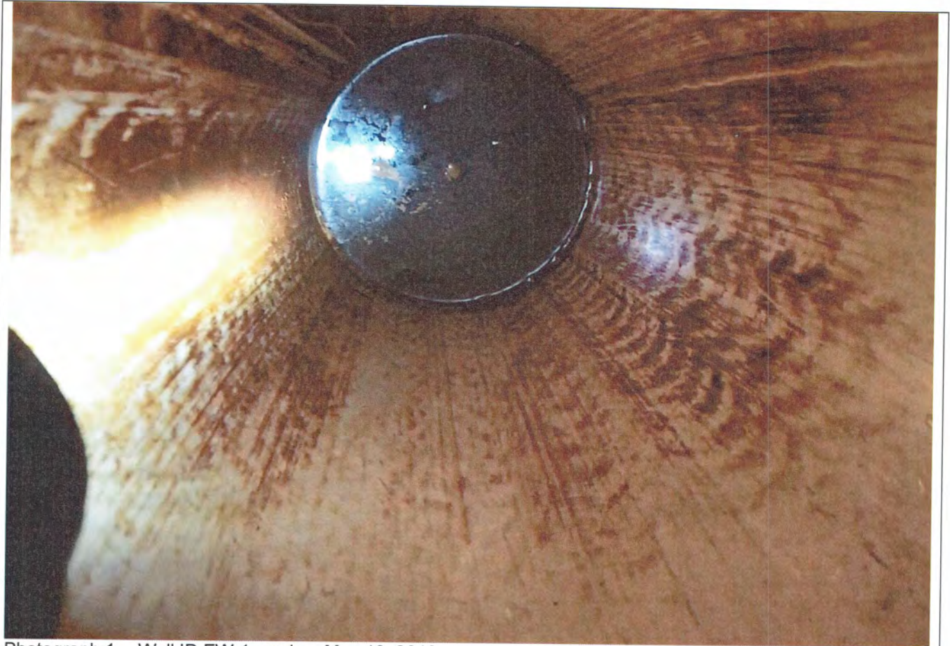
Photograph 1 Well ID EW-1, casing. May 18, 2016.
