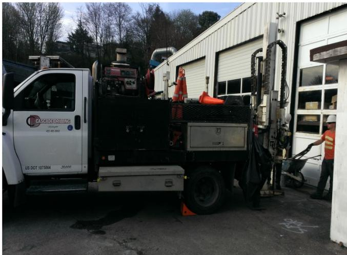
Photograph 1. Installing soil gas point B370.
