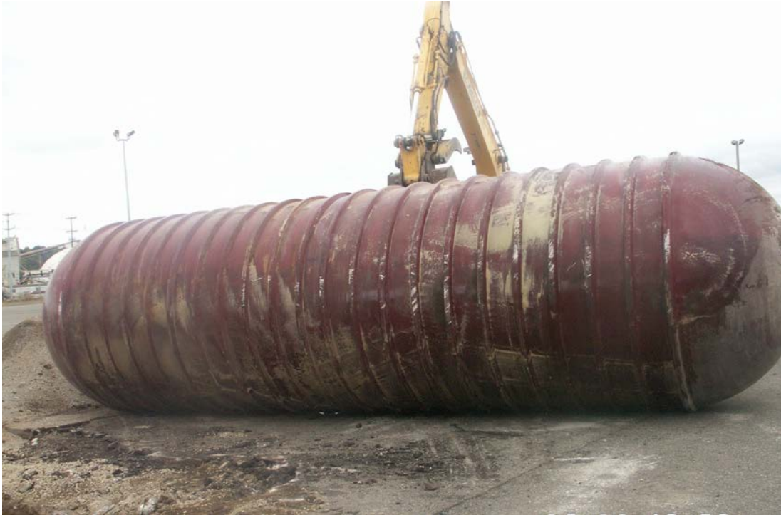
Photograph 5: Bottom of removed UST.
