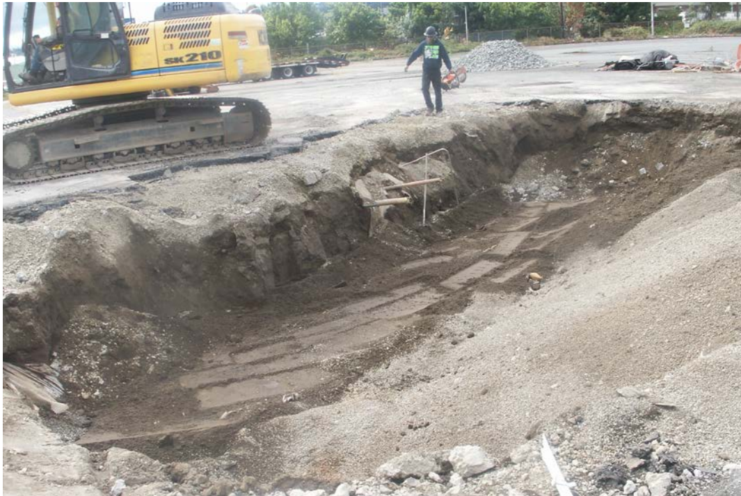
Photograph 7: Partially backfilled UST excavation, looking southwest.
