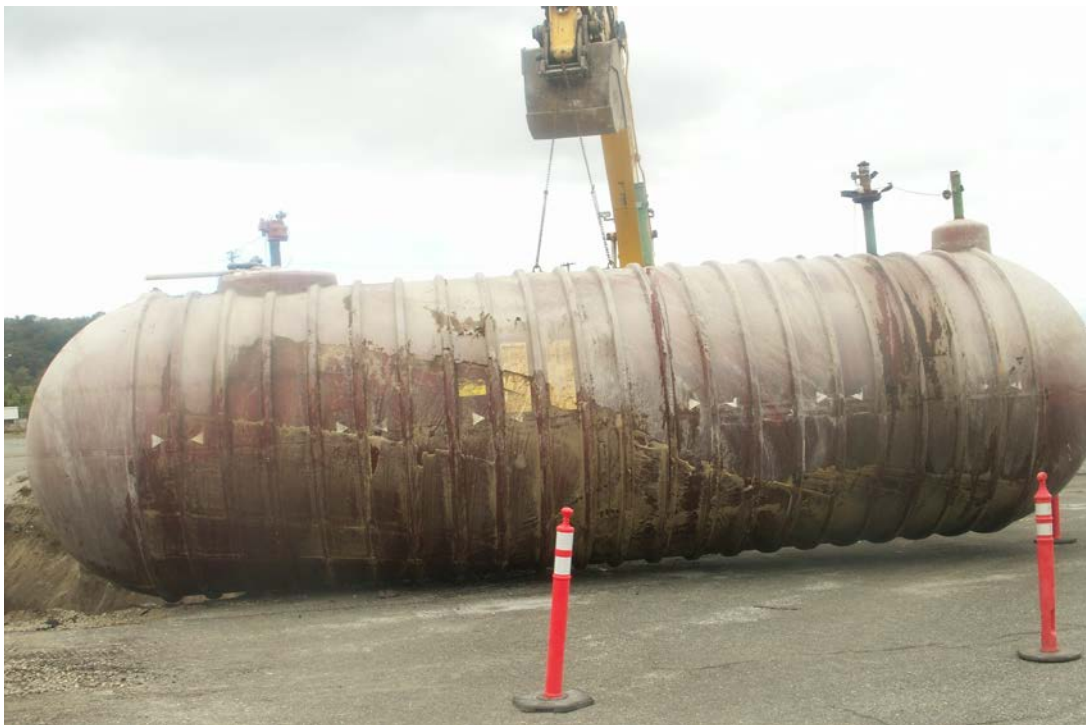
Photograph 4: Southern side of removed UST.
