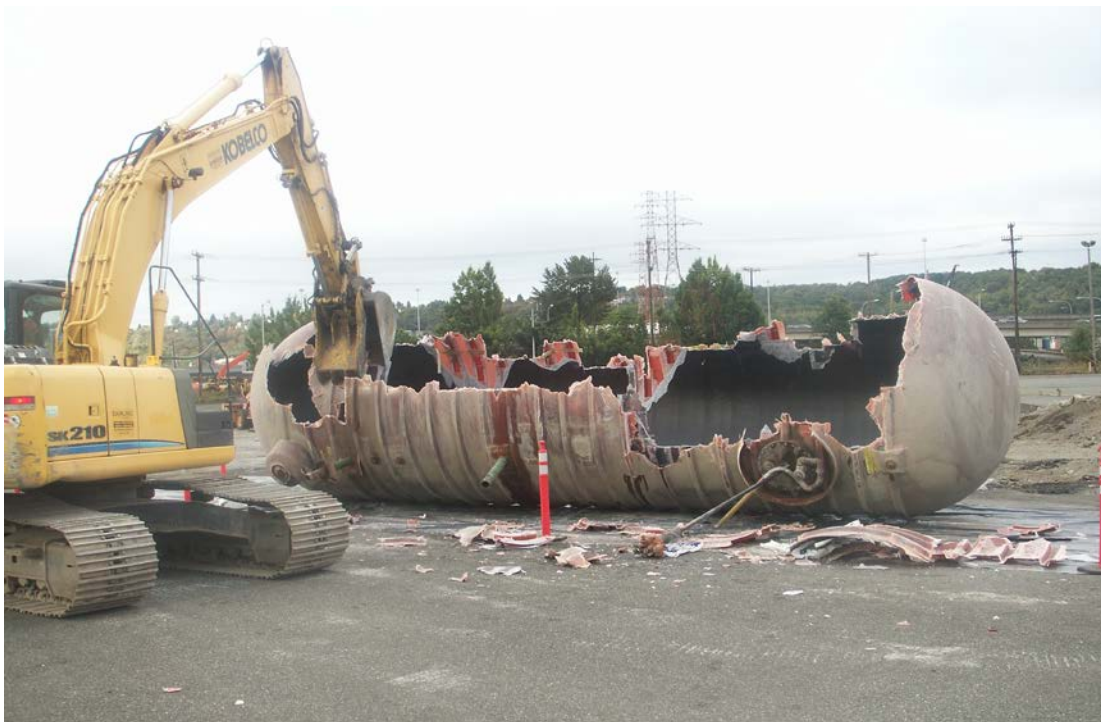
Photograph 6: Track hoe breaking up the UST for disposal.
