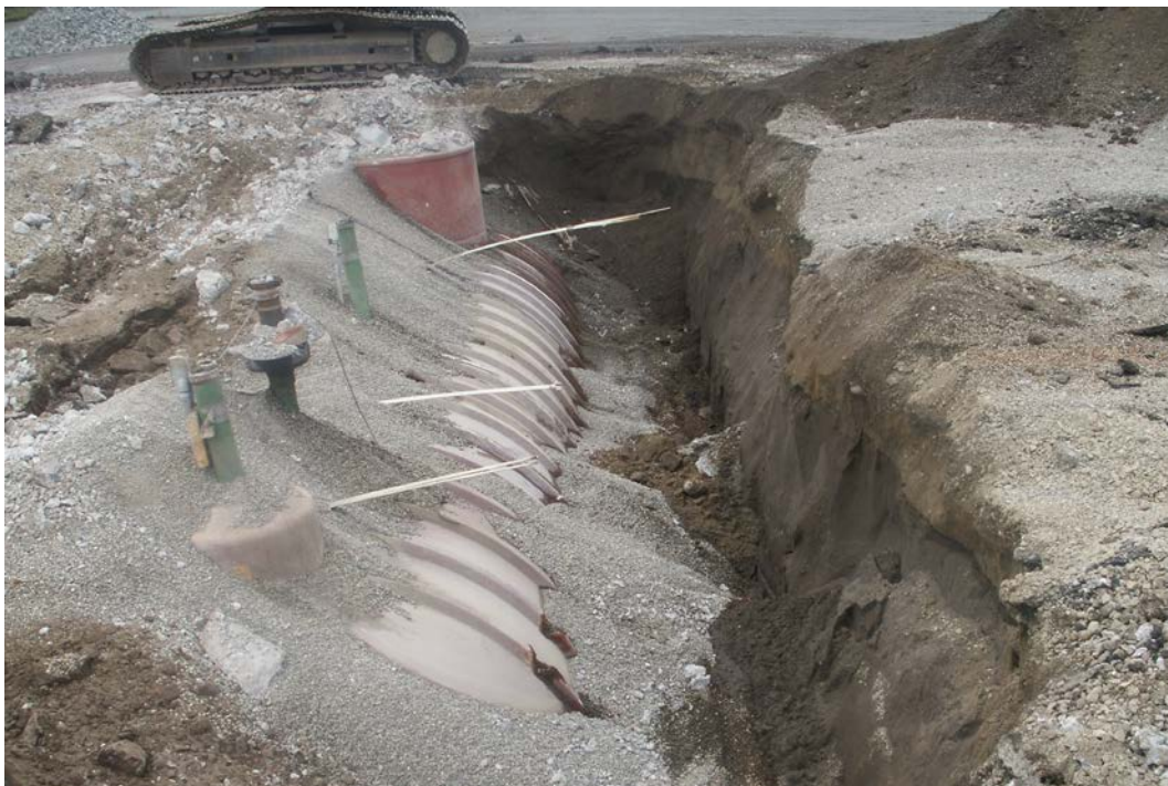
Photograph 2: Partial excavation of northern side of UST hold, looking west.
