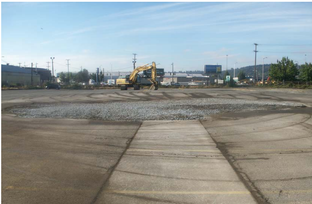
Photograph 8: Completed surface of backfilled and compacted UST excavation, looking south.
