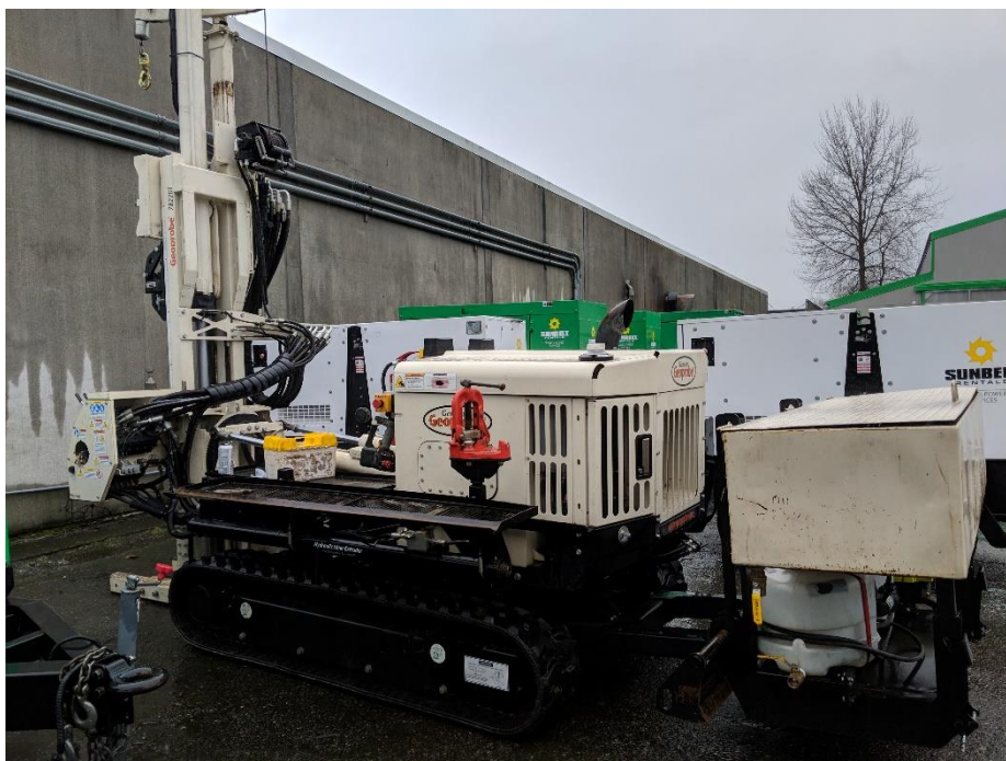
Photo 1. Drill rig set up at location B2.
