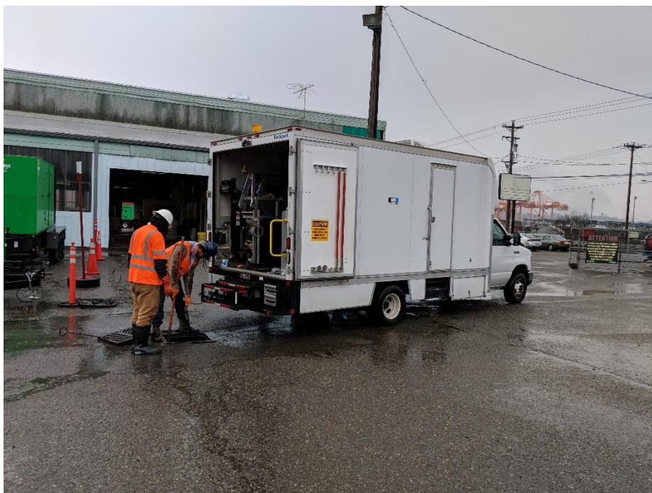
Photo 8. CB-7 CCTV operations.
