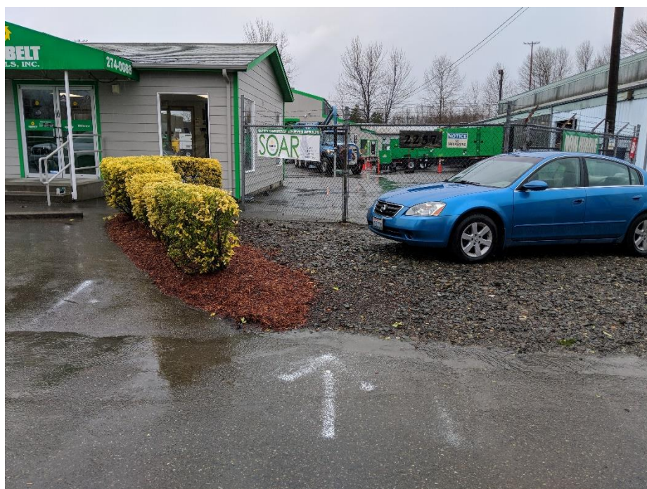
Photo 6. Marking shows approximately location and orientation of storm water "T"-junction.
