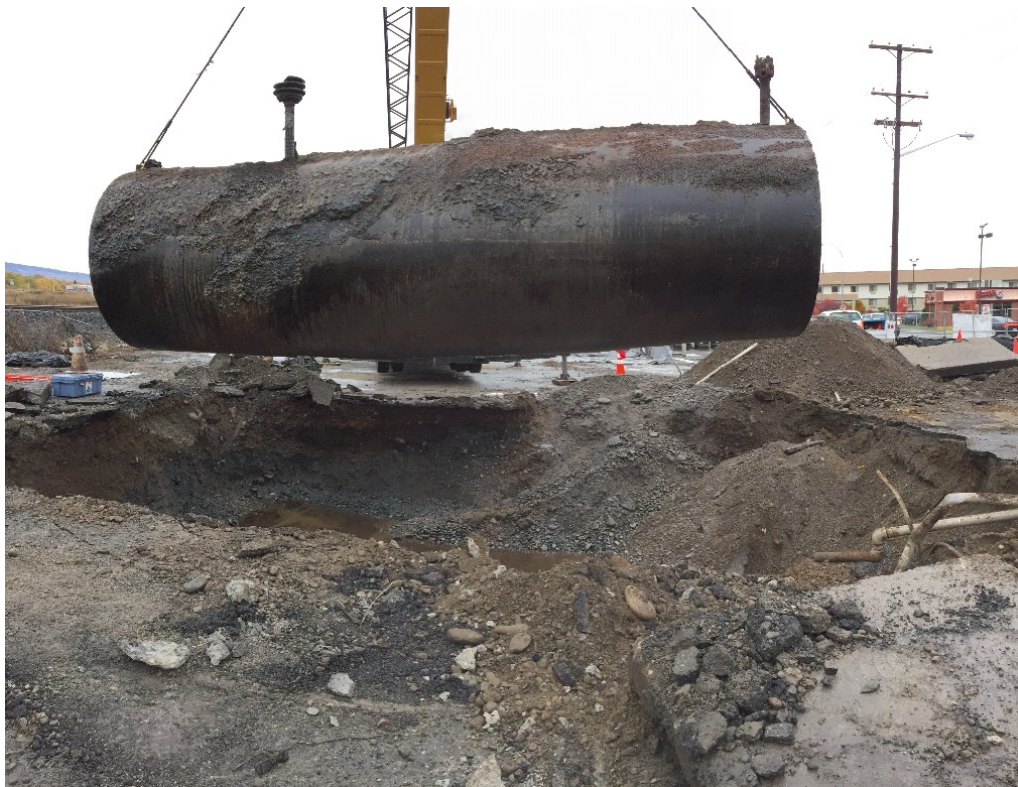
Photograph 4. Southern 10,000-gallon diesel UST removed from the northern UST pit.
