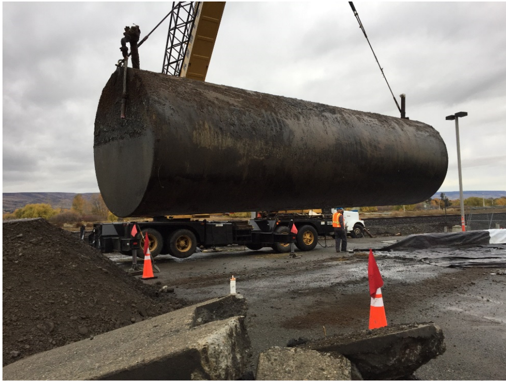
Photograph 3. Northern 10,000-gallon diesel UST removed from the northern UST pit.
