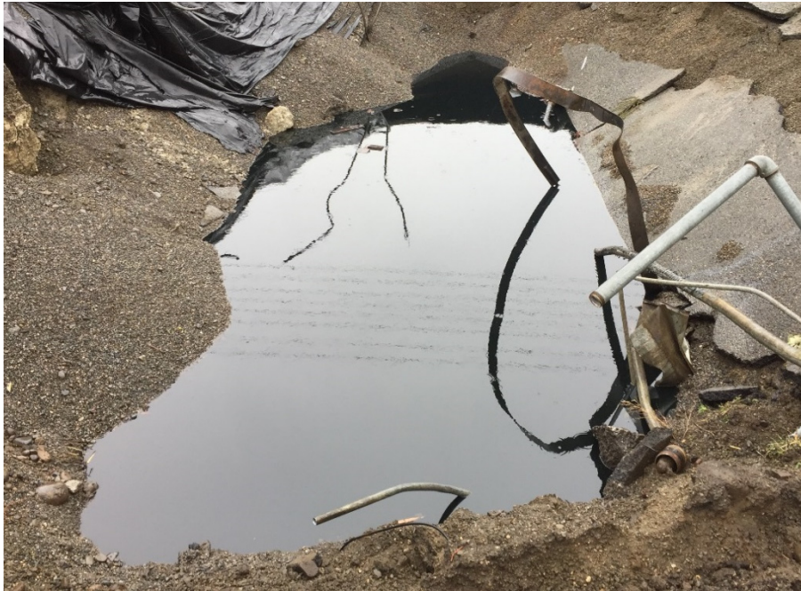
Photograph 12. Southern UST pit and LNAPL, pre-remedial activities (October 28, 2016).
