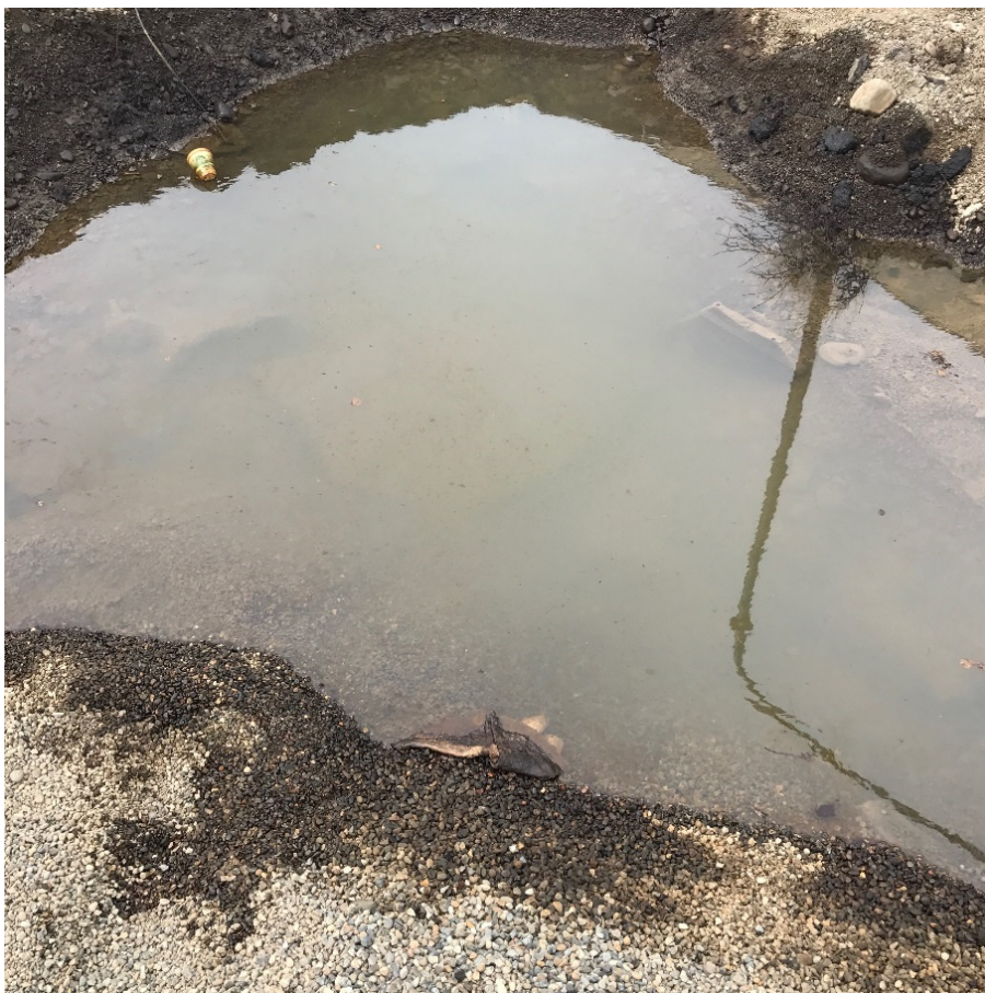
Photograph 13. Southern UST pit and LNAPL, post-system startup (April 4, 2017).
