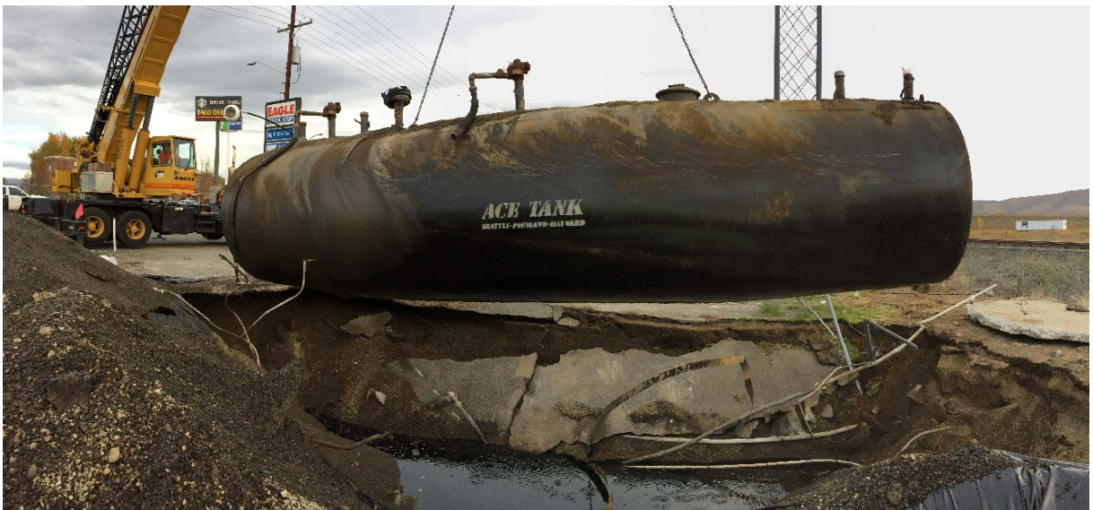
Photograph 2. 12,000-gallon baffled UST.
