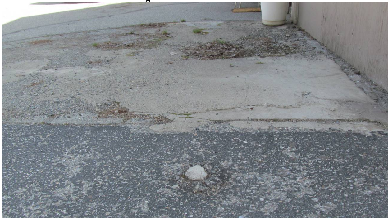
Photo 4: 2011 Phase II ESA Boring Locations West of Store- from the north
