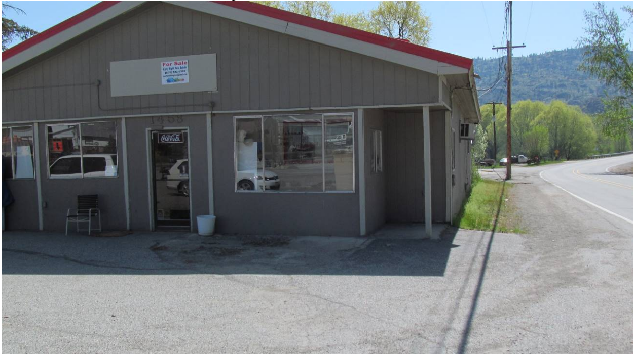
Photo 1: Former Arden's Country Store - from the west
