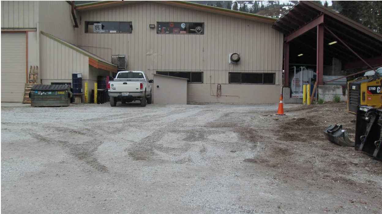
Photo 3: Maintenance Facility Site – from the north
