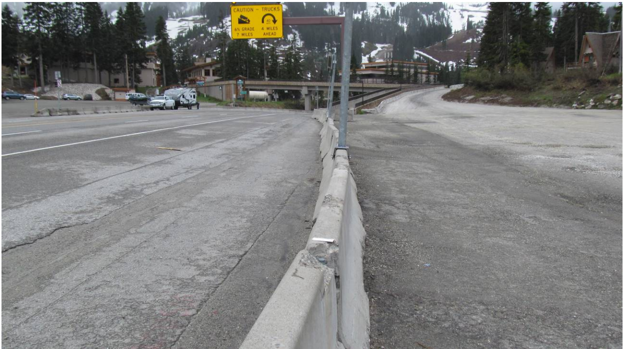
Photo 2: Mini Mart Site and US 2 – from the east
