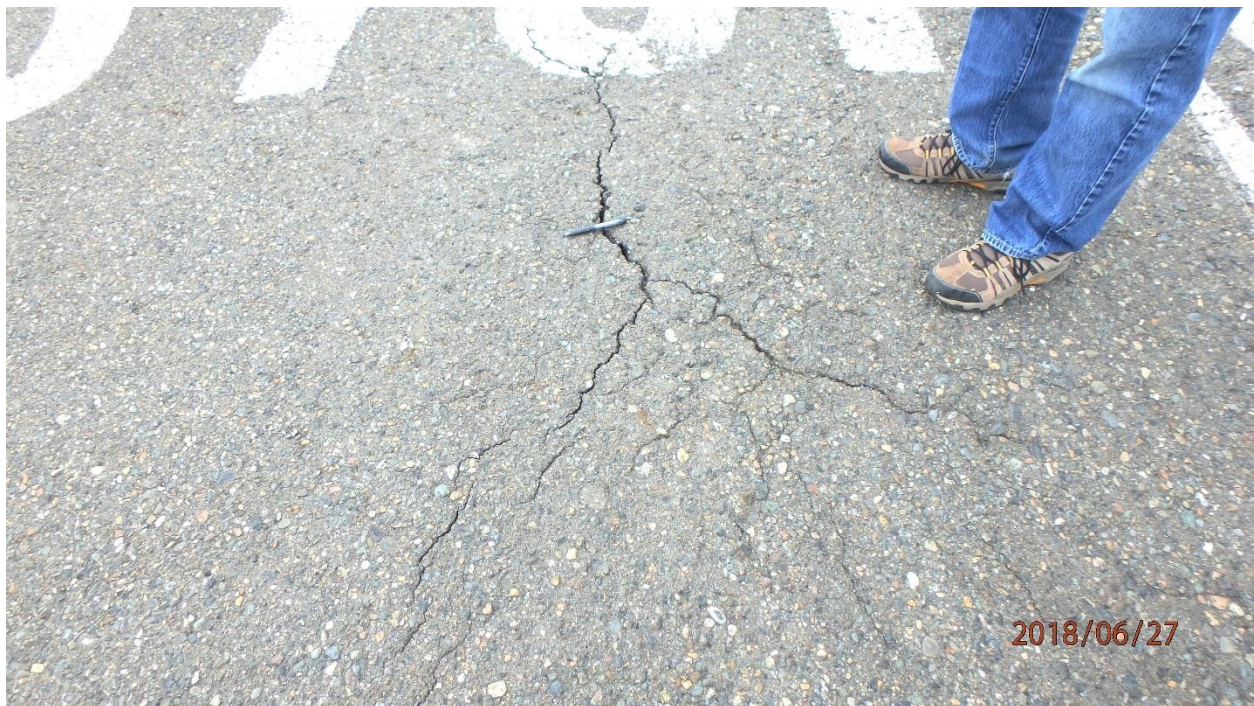
Photo 6. Mound in pavement with cracks as wide as ½ in.: RA-3 (map note 4)
