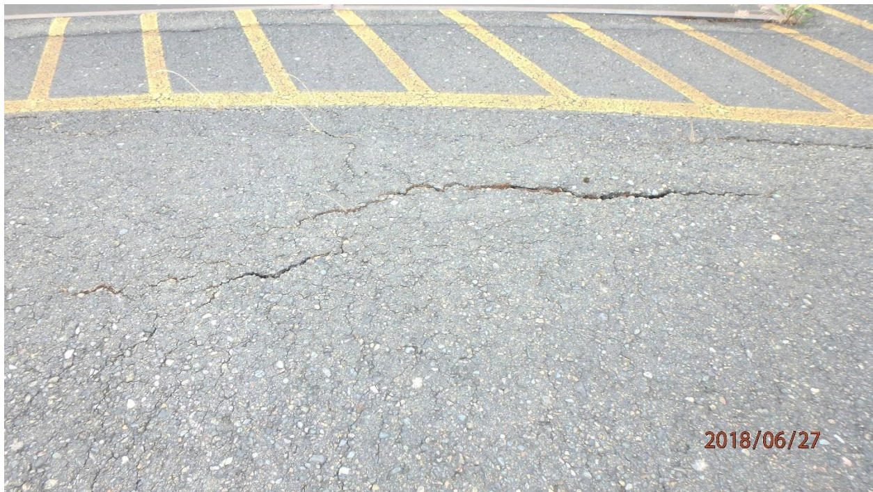
Photo 4. Mound in pavement with cracks as wide as 1 in.: RA-2 (map note 3)
