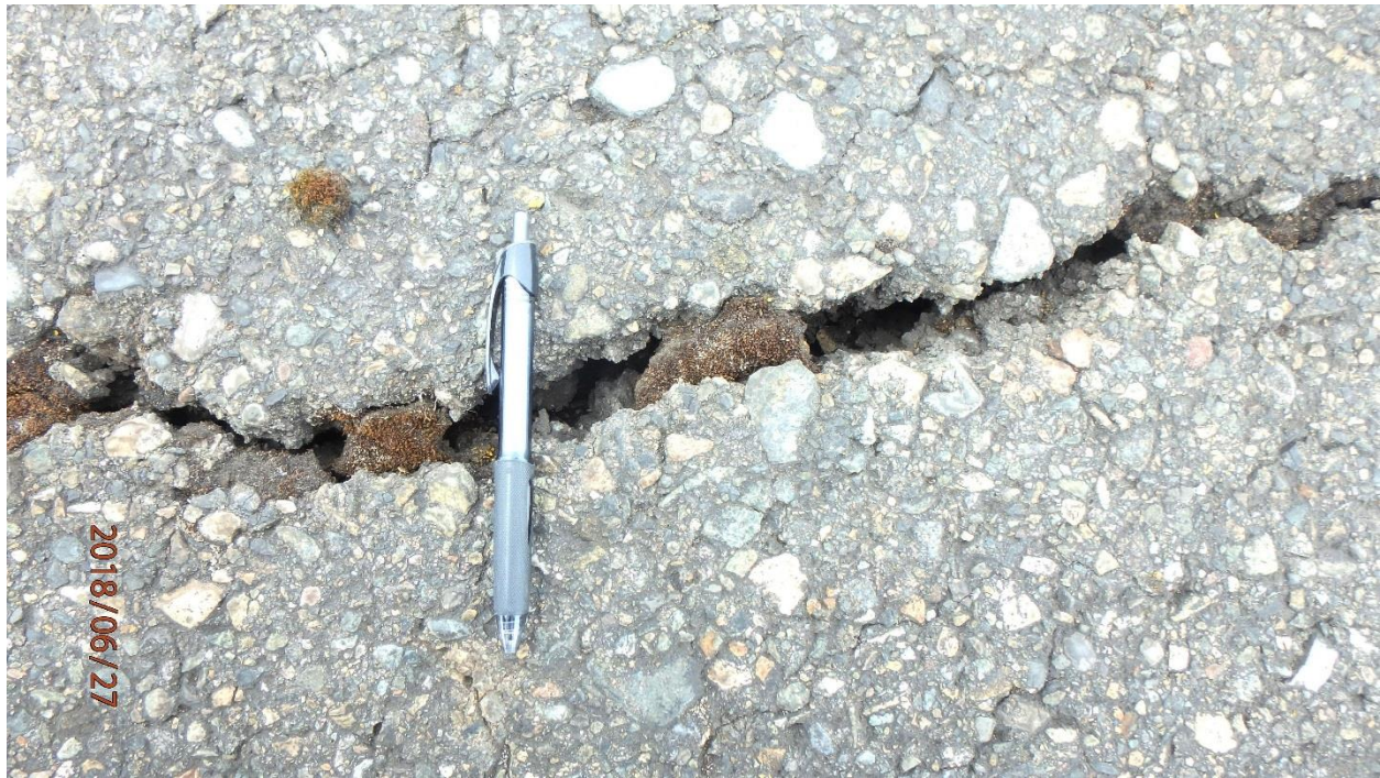
Photo 5. Close-up of mound in pavement with cracks as wide as 1 in.: RA-2 (map note 3)
