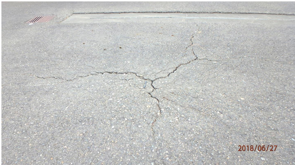
Photo 2. Mound in pavement with cracks as wide as 1 in.: RA-2 (map note 2)
