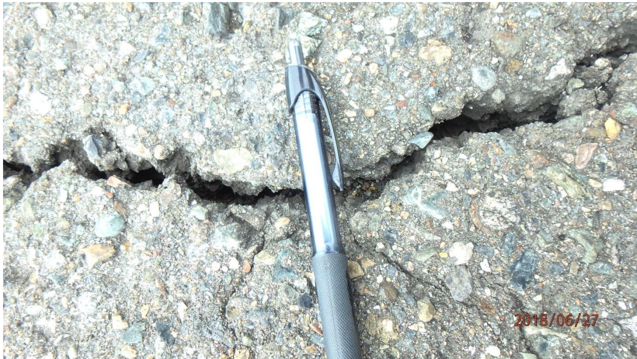
Photo 7. Mound in pavement with cracks as wide as ½ in.: RA-3 (map note 4)
