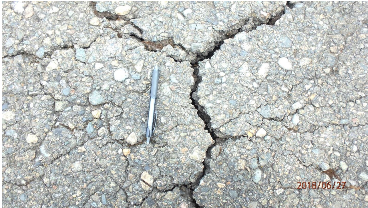
Photo 3. Close-up of mound in pavement with cracks as wide as 1 in.: RA-2 (map note 2)
