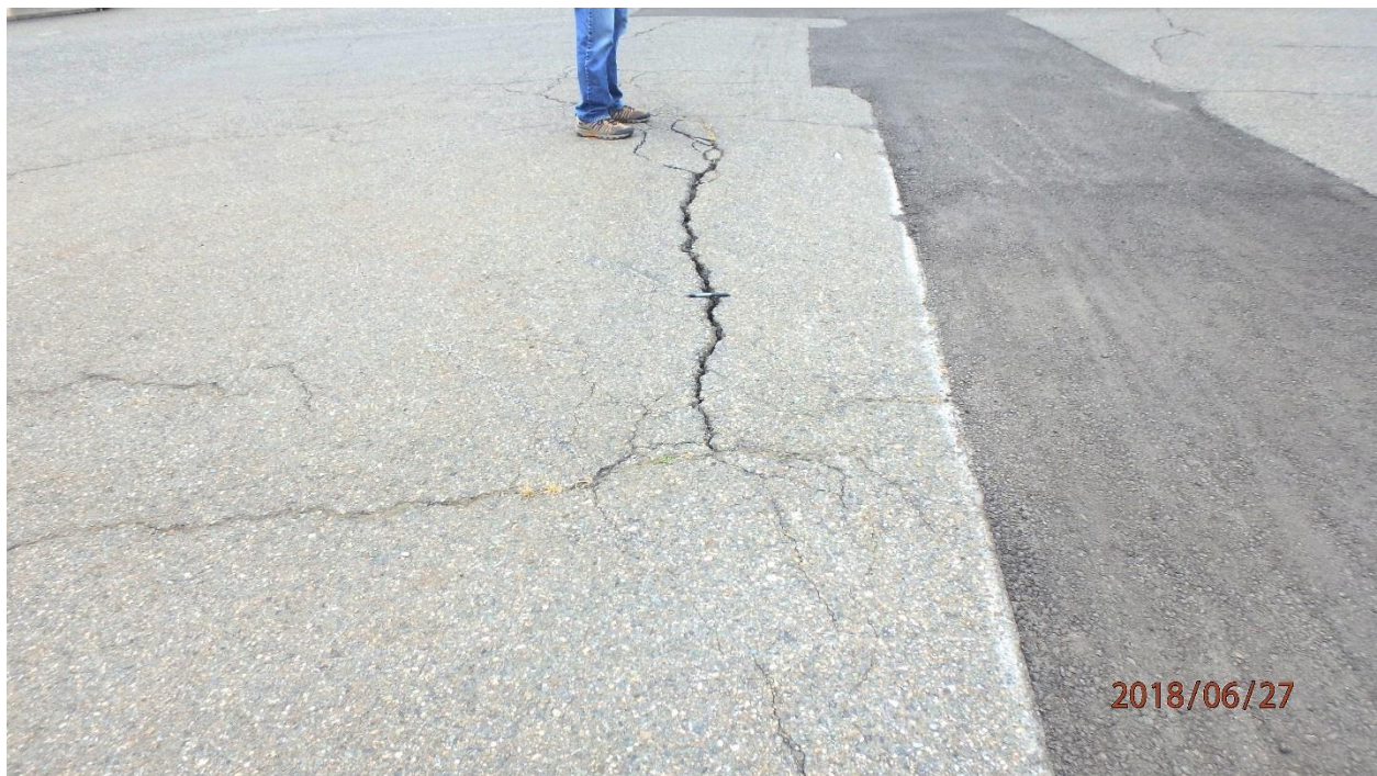
Photo 8. Elongated mound in pavement with cracks as wide as 1 in.: RA-2 (map note 5)
