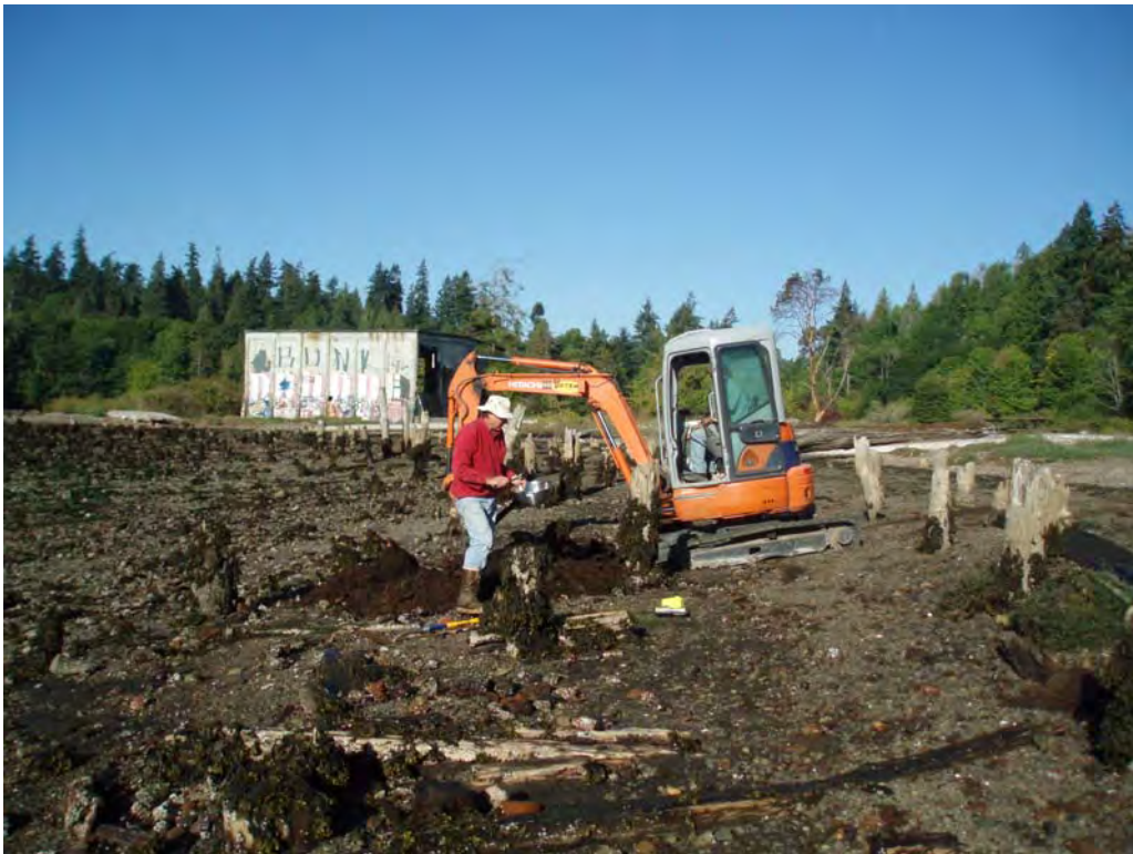
Photograph 8 – Test pit excavator at Test Pit 2
