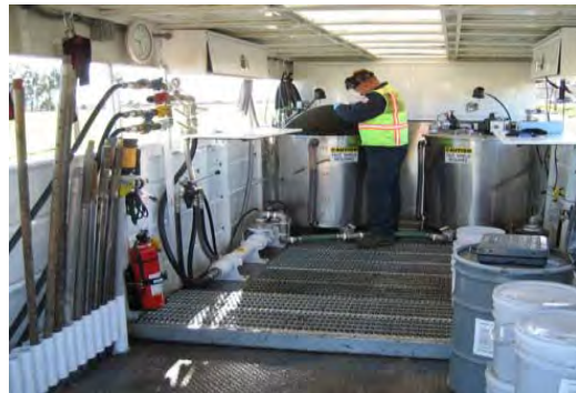
4. Injection Rig Interior
