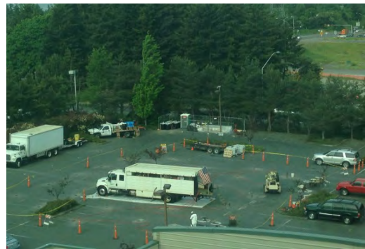
6. Aerial Site View
