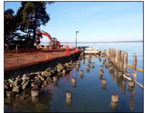
Public pier removal, October 2017
