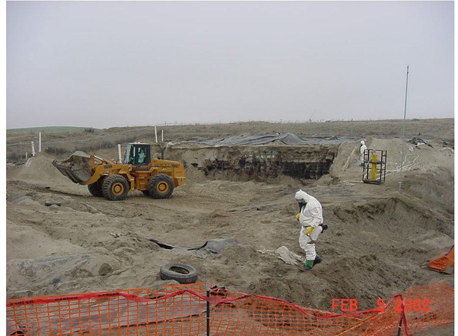
Zone B Removal Action February 5, 2002
