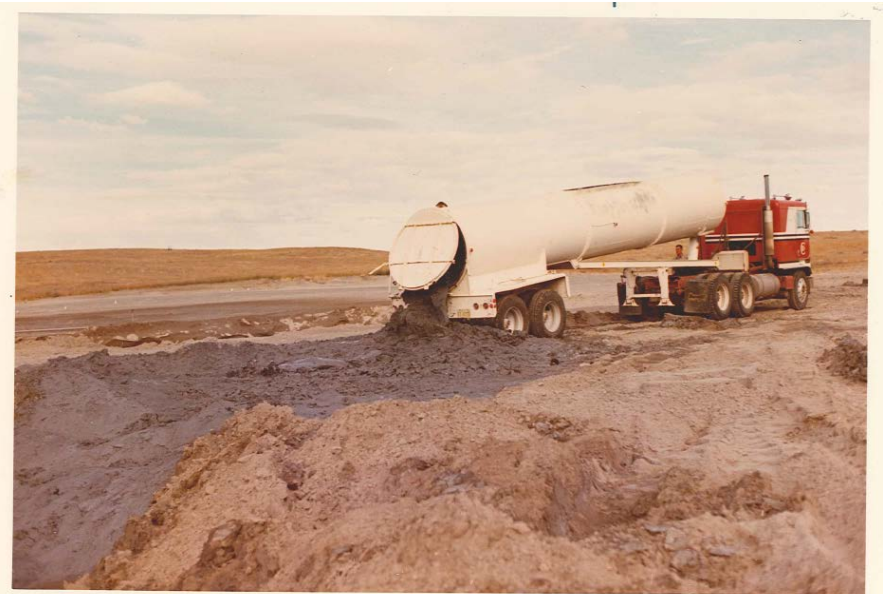
Landfilling toxic sludges into Zone E in 1973 or 1974
