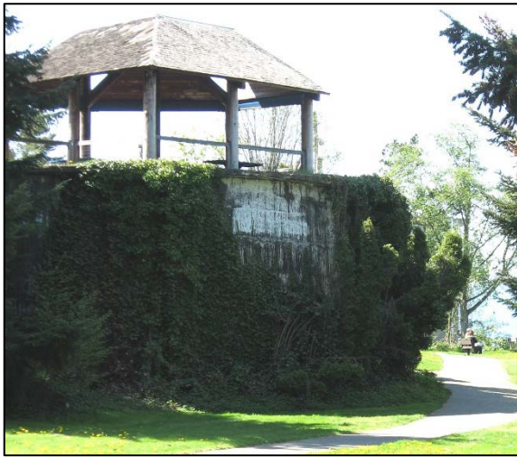
Figure 4: Concrete gas-holding tank near South State Street, upper Boulevard Park
