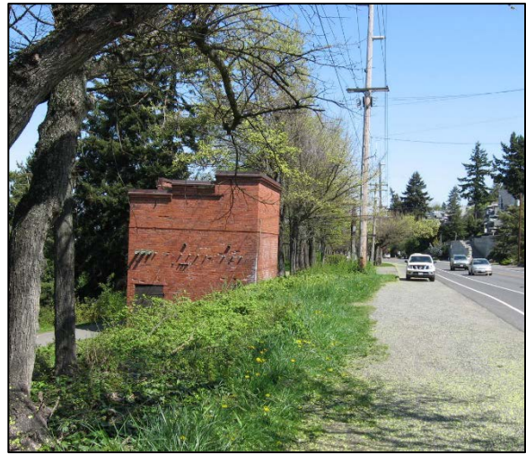
Figure 5: Small brick building near South State Street, upper Boulevard Park
