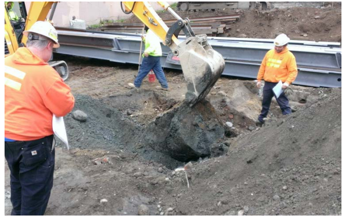
Photograph 2. Taken January 8, 2016, looking northeast. Removal of UST01.
