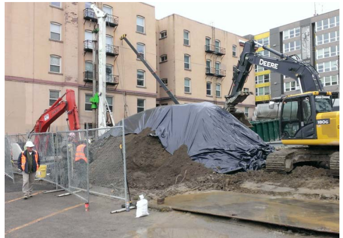
Photograph 8. Taken January 27, 2016, looking northeast. PCS stockpile covered with plastic. Kulchin installing H-piles along north Property boundary.
