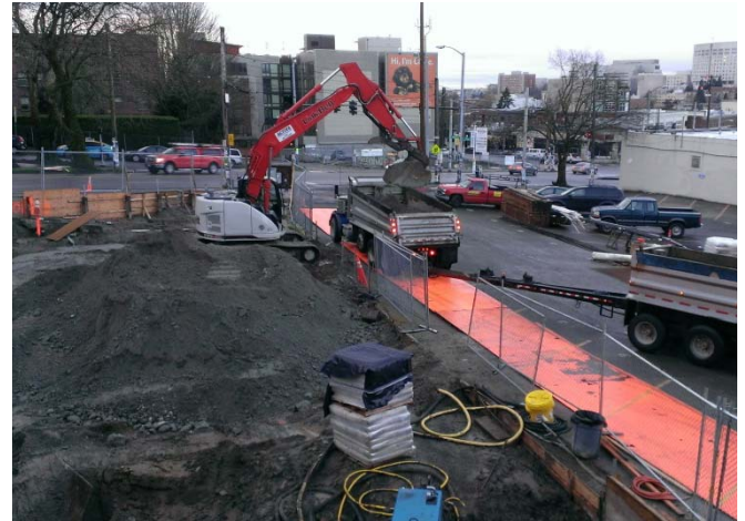
Photograph 12. Taken February 18, 2016, looking south. Loading PCS stockpile into haul truck.
