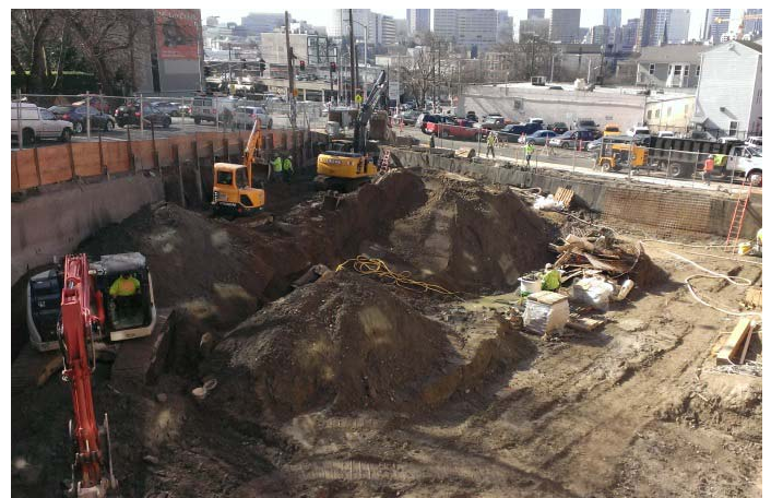
Photograph 16. February 25, 2016, looking southwest. Kulchin completing first lift of perimeter shoring.
