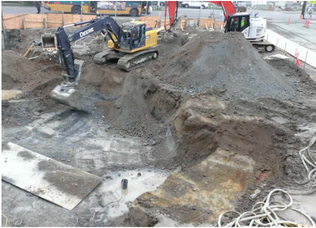
Photograph 11. Taken February 17, 2016, looking south. Excavating and stockpiling PCS.
