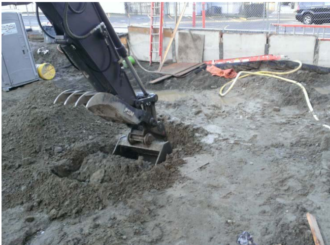
Photograph 13. Taken February 20, 2016, looking west. Digging test pit TP102.
