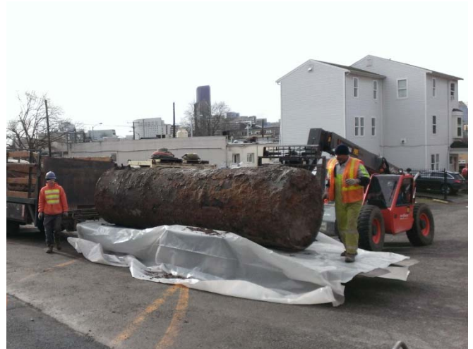
Photograph 6. Taken January 20, 2016, looking southwest. UST03 removed and placed on trailer.
