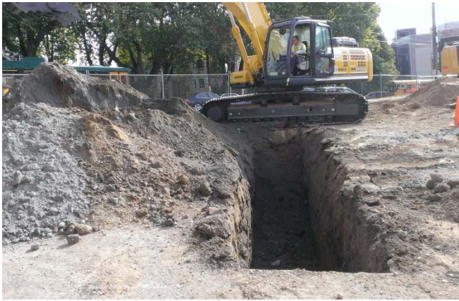
Photograph 1. Taken October 5, 2015, looking south. Note TP04 and soil stockpile.
