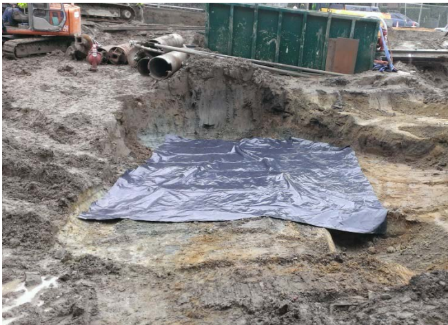
Photograph 7. Taken January 26, 2016, looking south. Plastic sheeting laid down over PCS.
