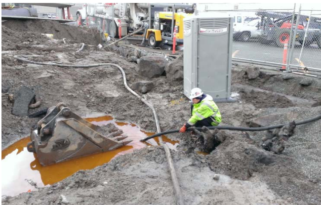
Photograph 5. Taken January 18, 2016, looking southwest. MarVac pumping out displaced contents of UST02.
