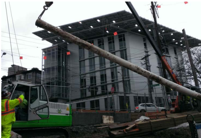
Photograph 9. Taken February 6, 2016, looking southeast. Kulchin installing dewatering well DW01.
