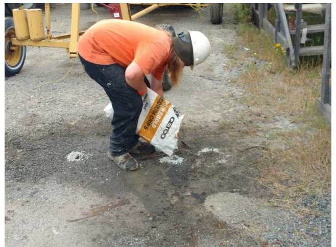
Backfilling soil borings with bentonite to surface
