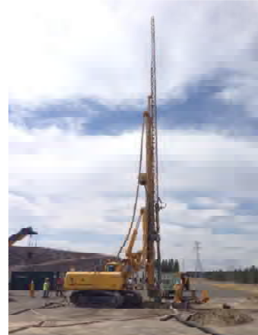
Figure 3: KB6 Drill Rig
