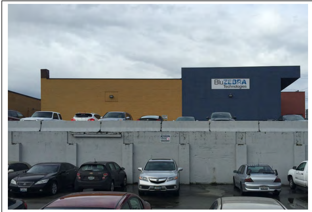
Photo 7: 615 Dexter Avenue North, Seattle, Washington – The parking area on the east side of the parcel looking west. This area used to be a part of the building but burned down around 2005. The building foundation is used as parking.
