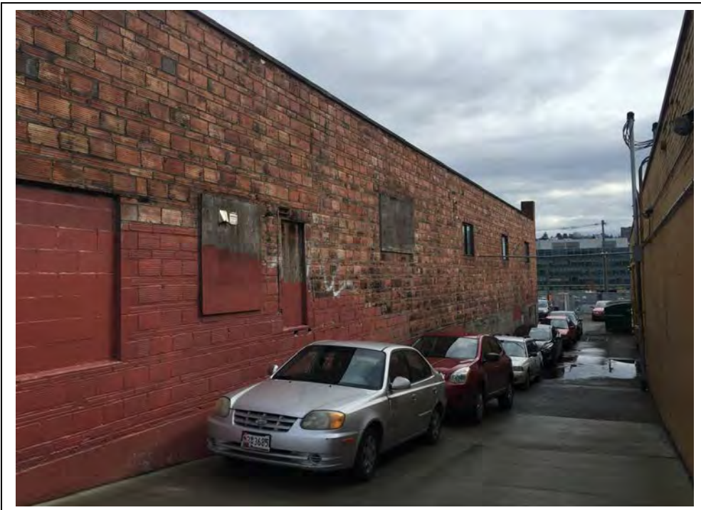
Photo 4: 615 Dexter Ave N, Seattle, Washington – The south side of the building looking east.
