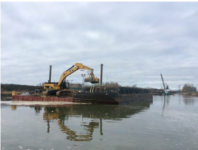
In-water ENR Sand Placement with Young's Bucket.
