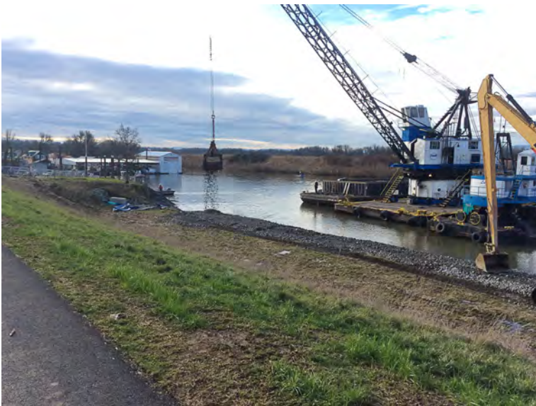
Upstream Fish Mix Placement.
