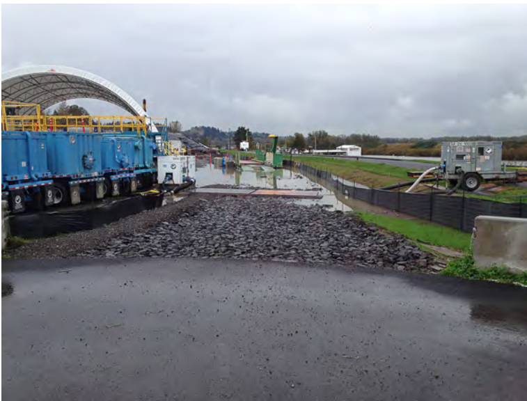
Pumping stormwater accumulated in the MHA to treatment system.
