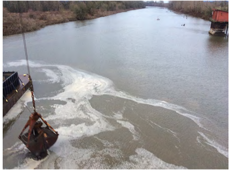
In-water ENR Sand Placement
