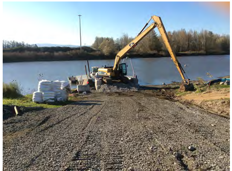
Fish mix and excavator placed in off loading facility.
