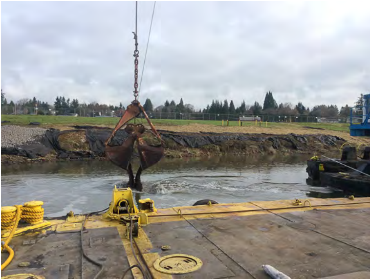
In-water ENR Sand Placement
