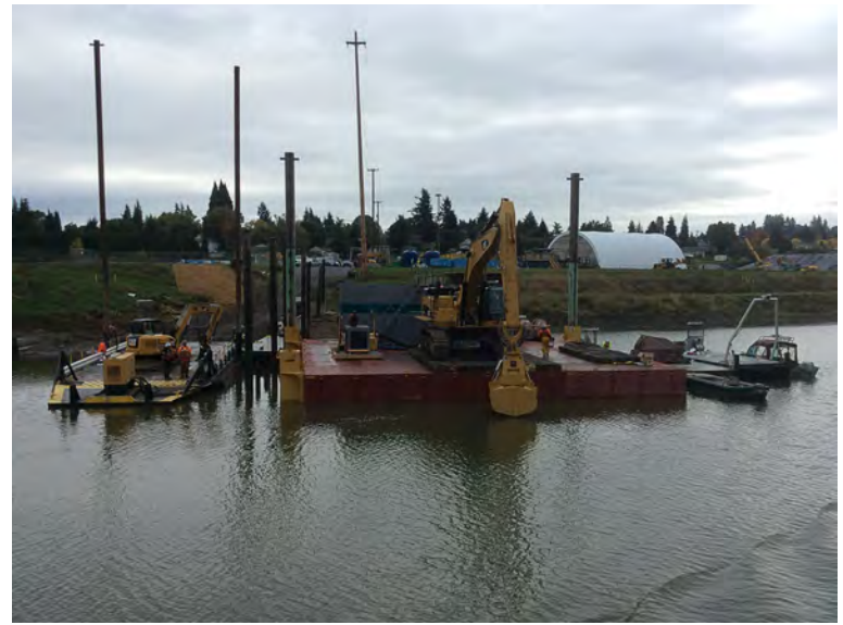
In-water equipment for pile removal and dredging.
