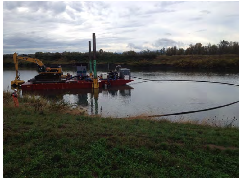
Dredge barge and pipeline
