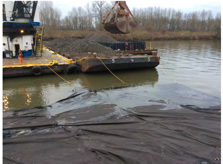
Fish Mix Placement on filter fabric.
