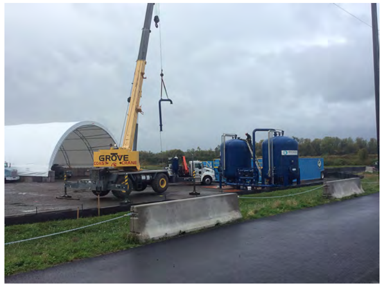
Assembling Water Treatment Equipment in MHA
