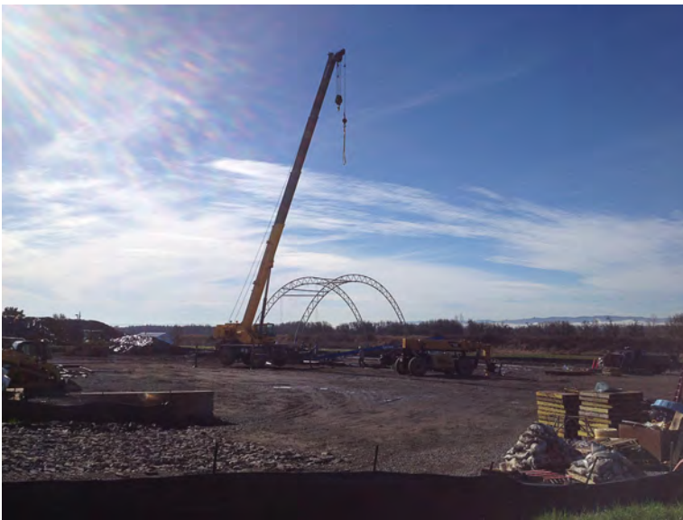
Dismantling tent structure within MHA.
