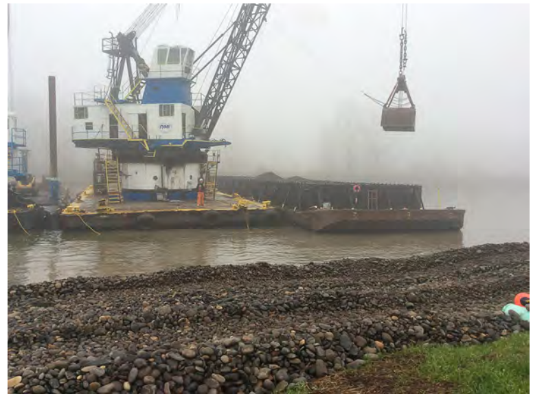
Over water crane placing fish mix in water.
