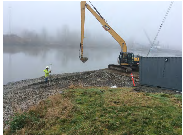
Fish Mix Grading at kayak launch
