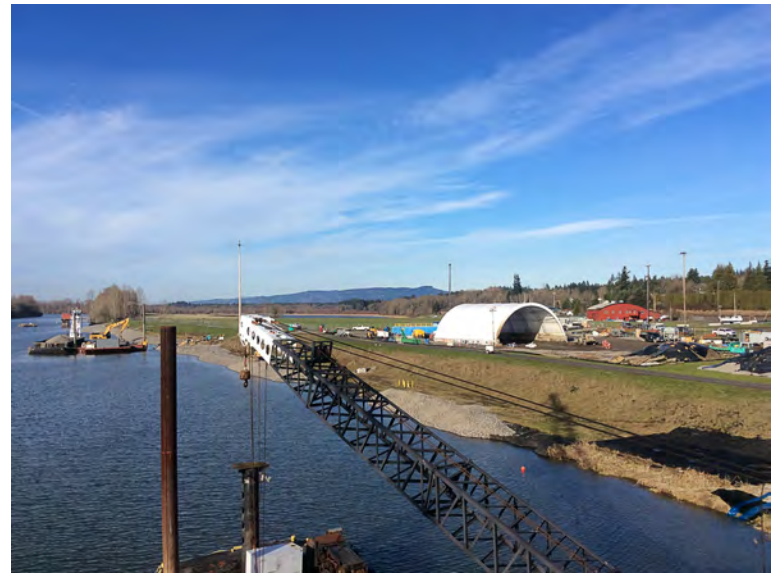
View of MHA and dredge barge.
