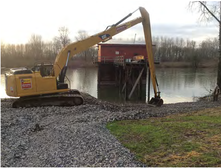
Long reach excavator grading fish mix.
