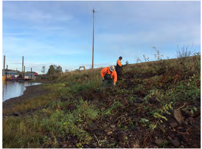
Vegetation and debris removal on shoreline south of Division St.
