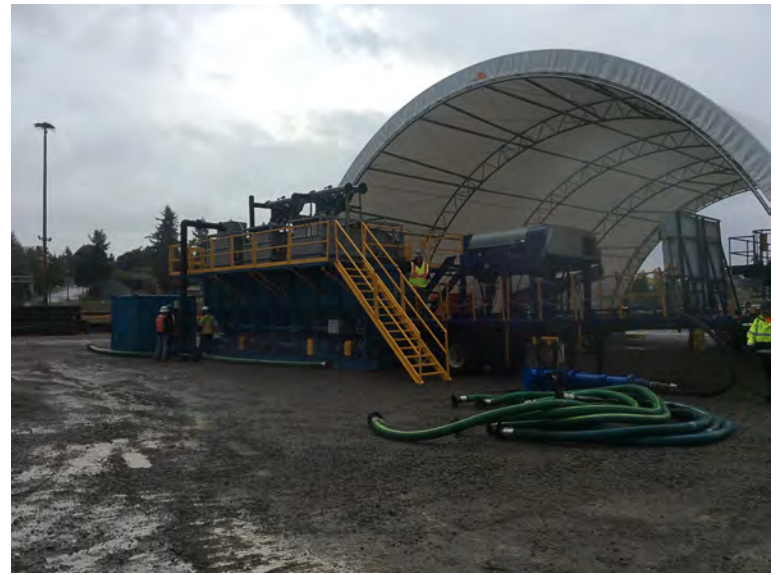
Setting up water treatment system in MHA.
