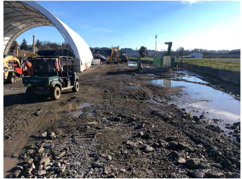
Rock removed from MHA exit.
