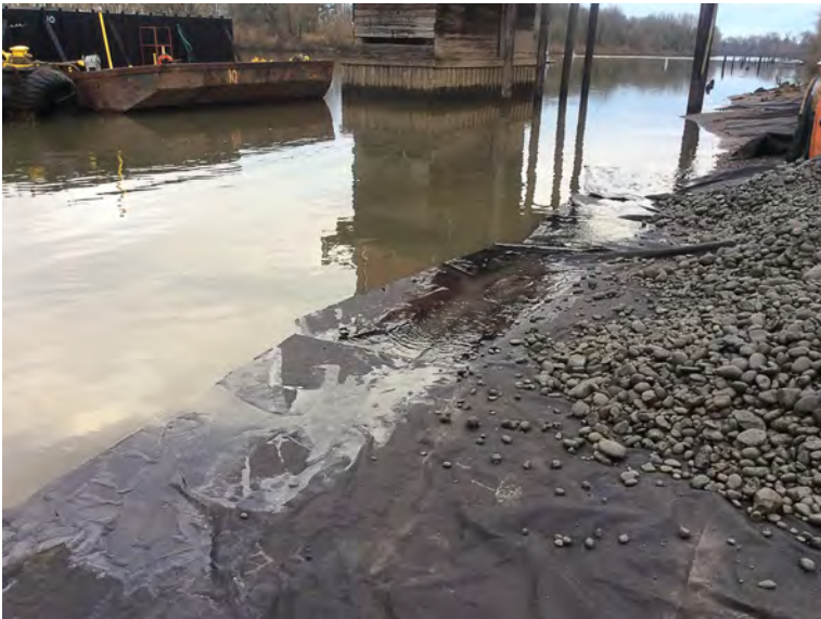
Fish Mix Placement on filter fabric.
