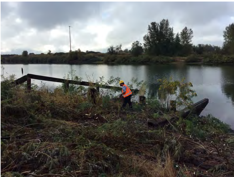
Using chainsaw to cut vegetation to grade along shoreline.
