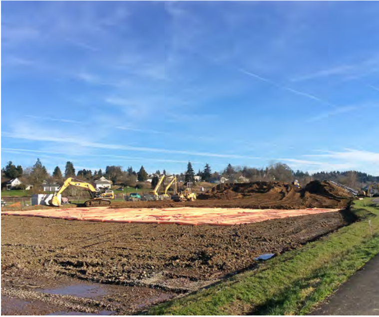
Clean soil cap placement progress.
