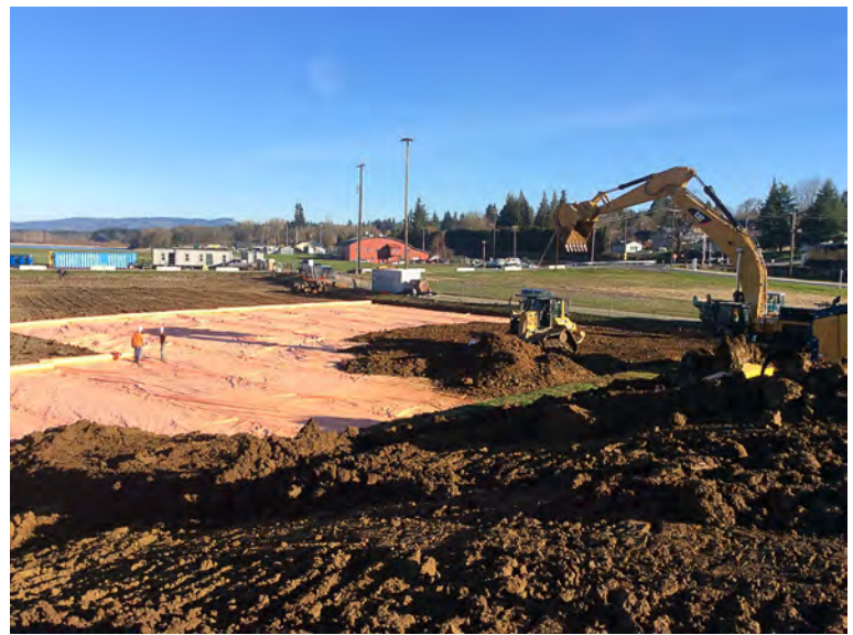
Clean soil cap placement.
