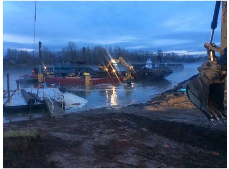
In-water ENR Sand Placement
