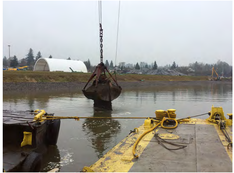
ENR sand placement near Division Street.
