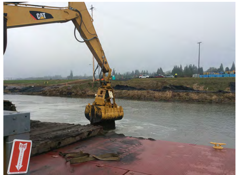
In-water ENR Sand Placement
