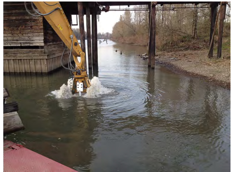
Dredging in shallow water.
