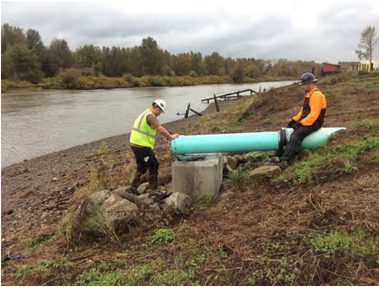
Building stormwater extension north of Division St.
