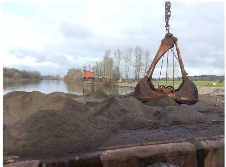
Crane operator grabbing sand.
