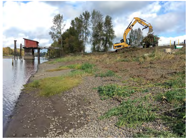
Excavator loading vegetation removed from the shoreline to the track truck, which transfers it to the MHA.
