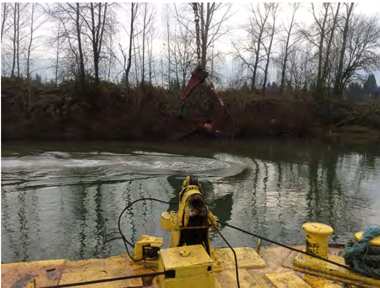
In-water ENR Sand Placement
