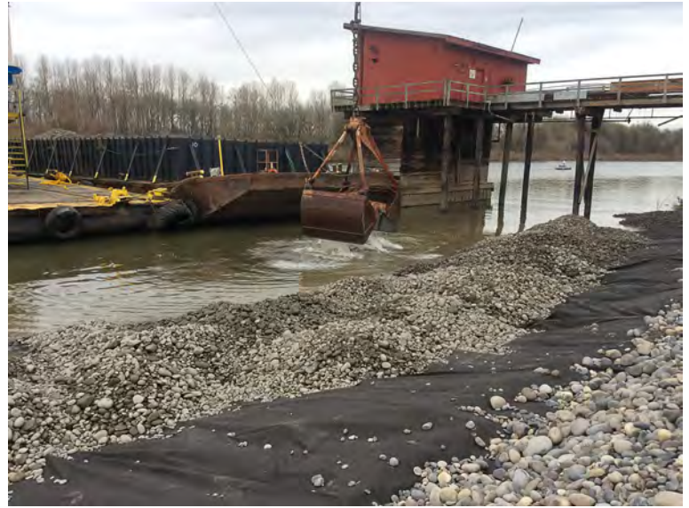
Fish Mix Placement from in-water.
