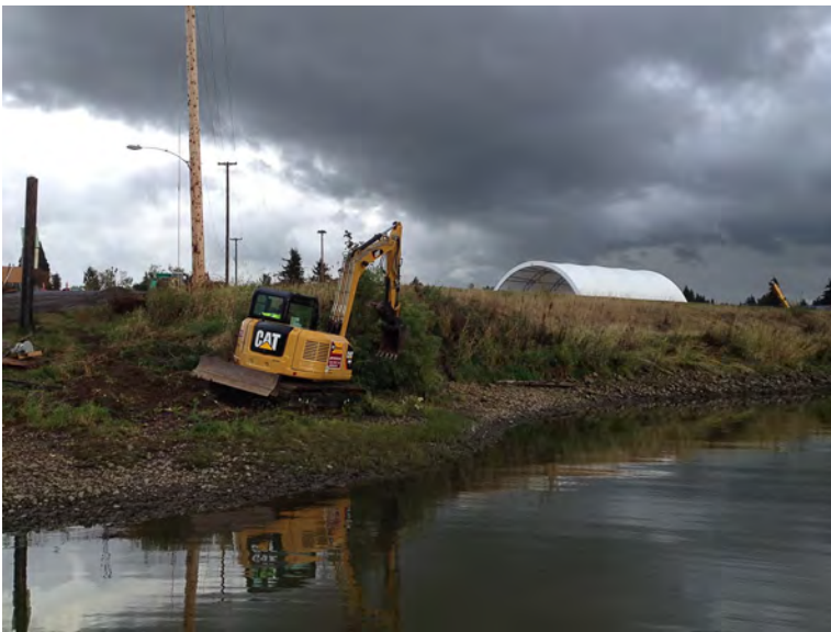
Limited vegetation removal near Division St.
