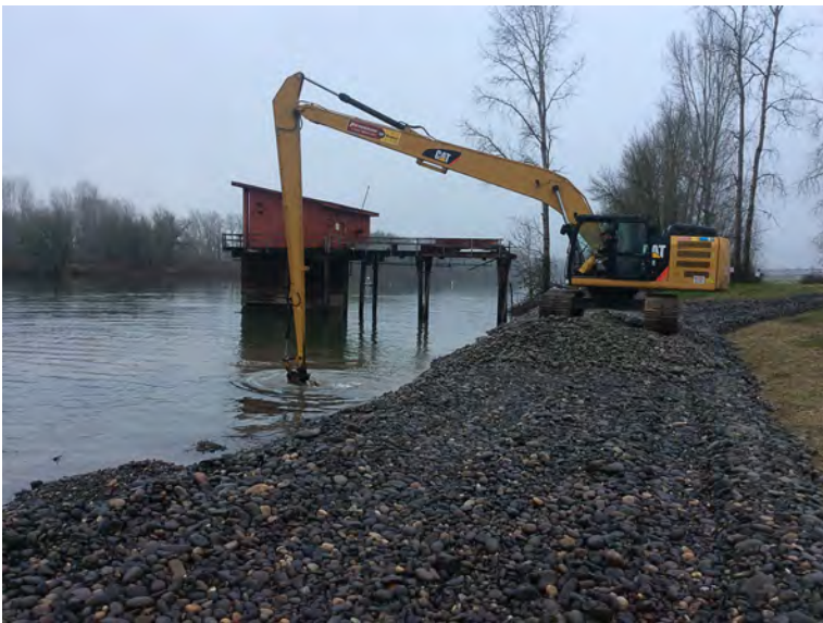
Excavator grading fish mix in water.
