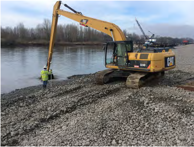
Fish Mix Placement in water at kayak launch.
