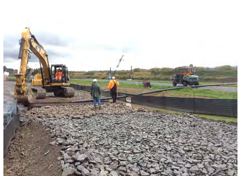
Constructing pathway for pipeline in MHA.
