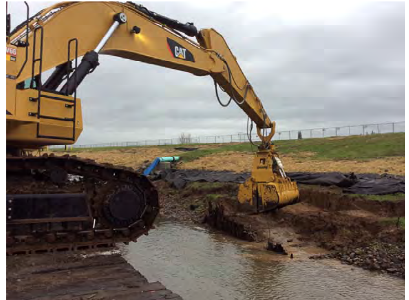
Dredging on shoreline to achieve desired grade.
