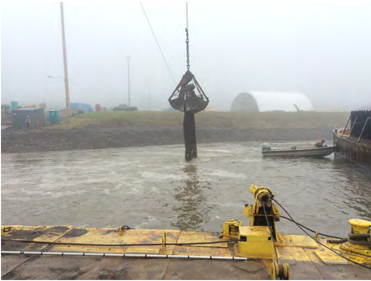
ENR sand placement below power lines.
