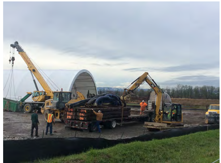
Demobilization of crane mats and piping.
