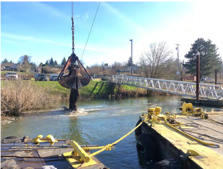
In-water ENR Sand Placement next to dock.
