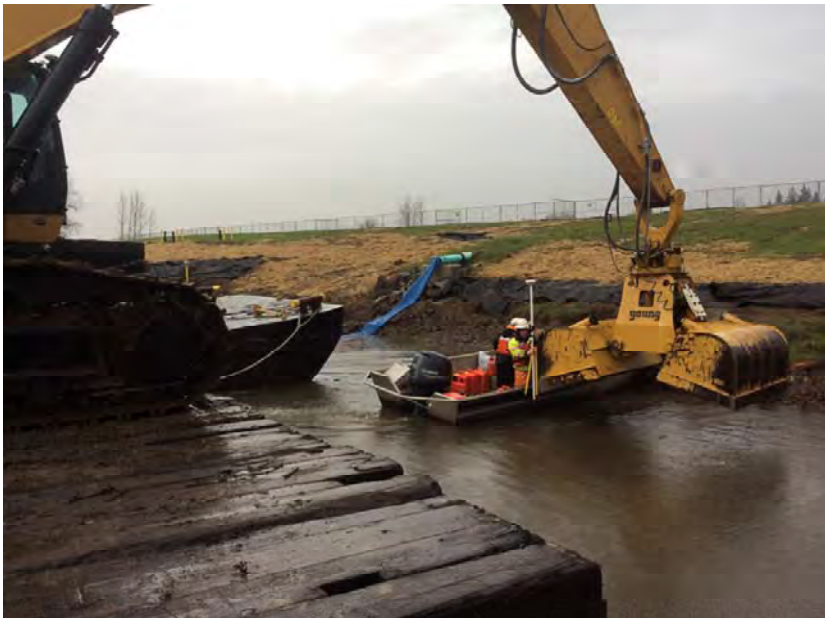
Measuring to ensure the Young bucket alignment is accurate.
