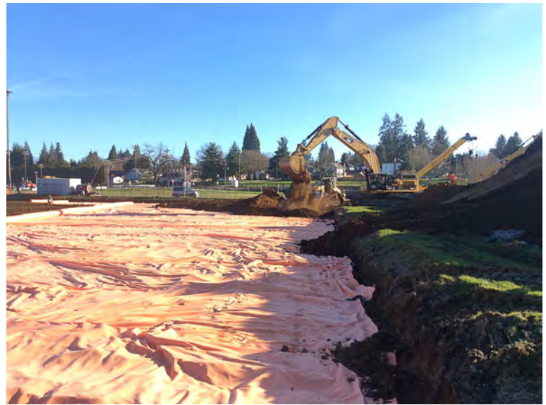
Clean soil cap placement.
