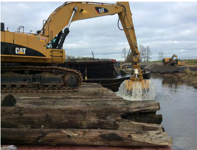
Dredging in shallow water.
