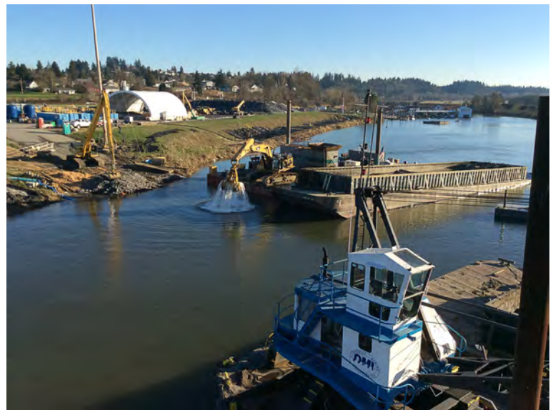
Dredging near transload operation.
