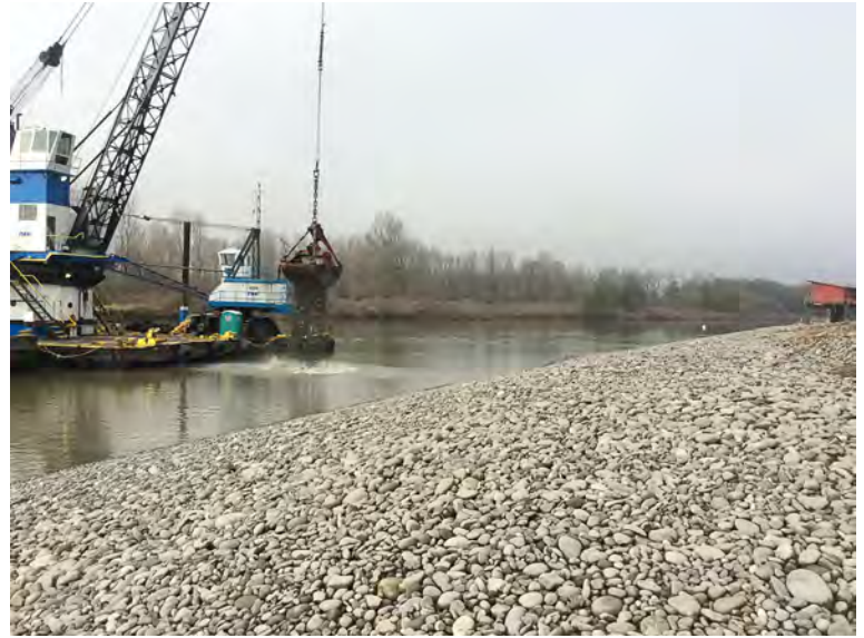
Fish mix placement north of Division St.
