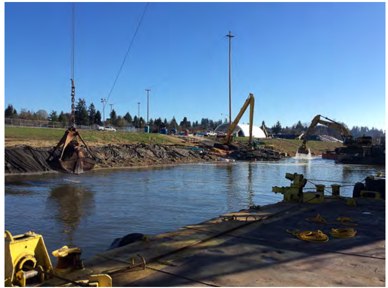
Sand placement and dredging near transload operation.
