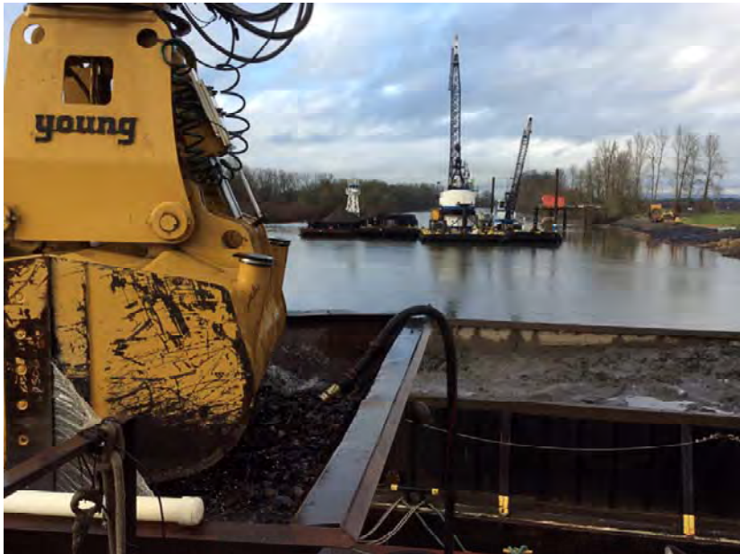
Dredging, placing sand, and laying fish mix on shoreline.
