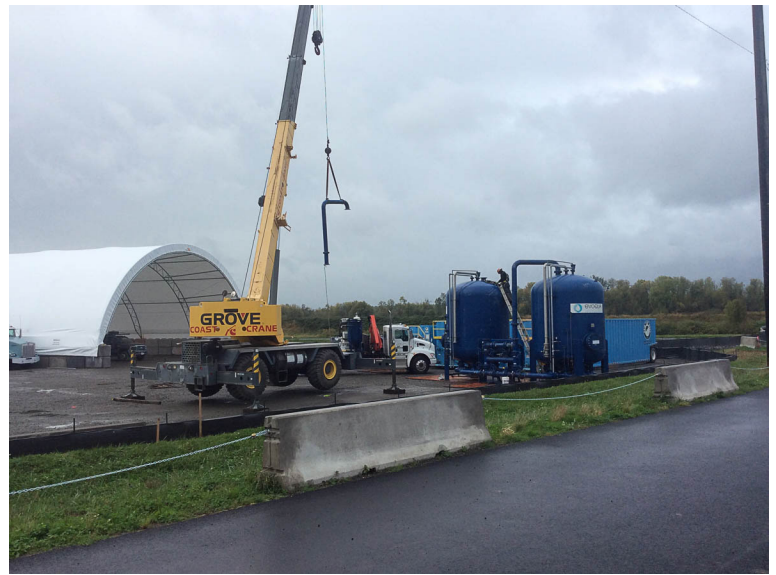
Assembling Water Treatment Equipment in MHA
