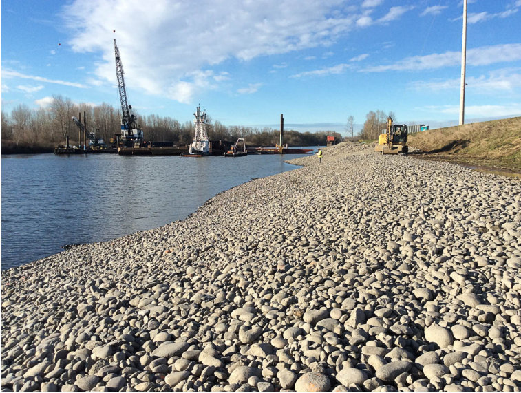
Grading fish mix along shoreline south of Division Street.
