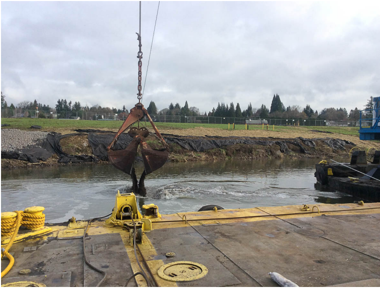
In-water ENR Sand Placement
