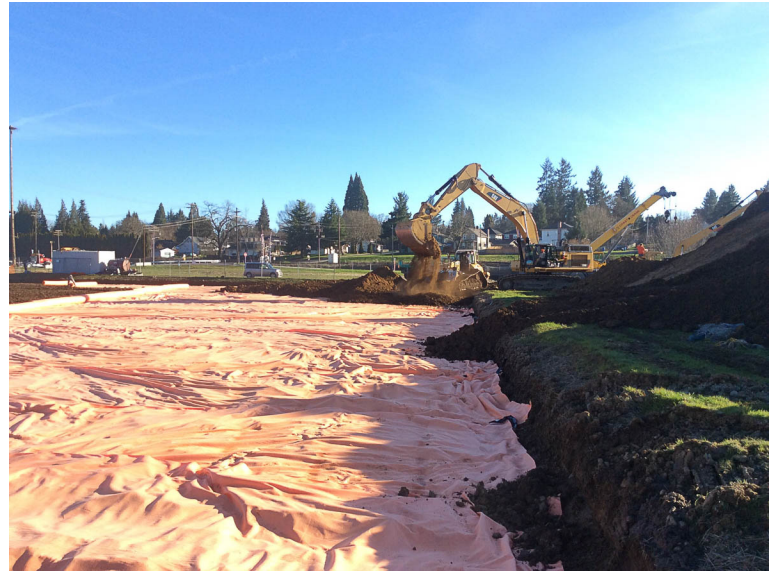
Clean soil cap placement.
