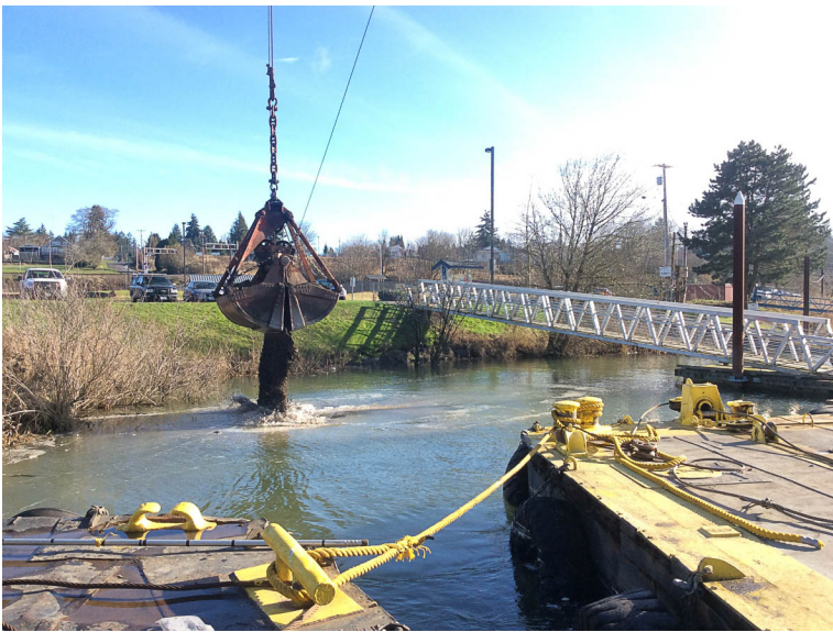
In-water ENR Sand Placement next to dock.
