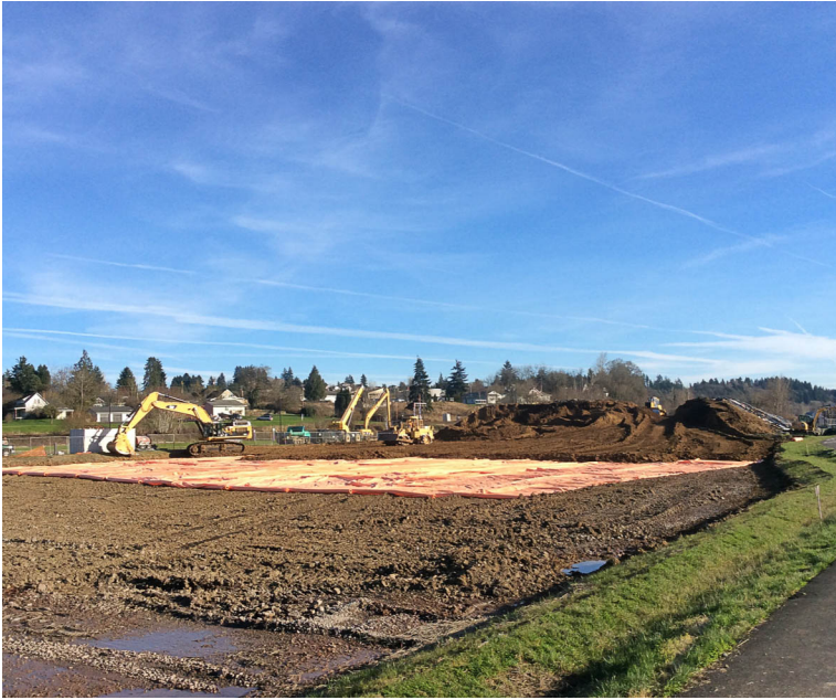
Clean soil cap placement progress.
