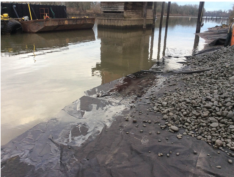
Fish Mix Placement on filter fabric.
