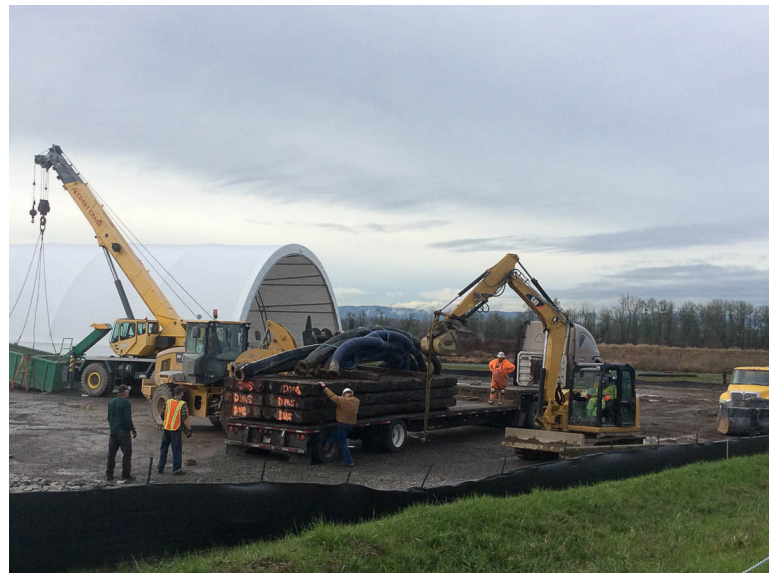
Demobilization of crane mats and piping.
