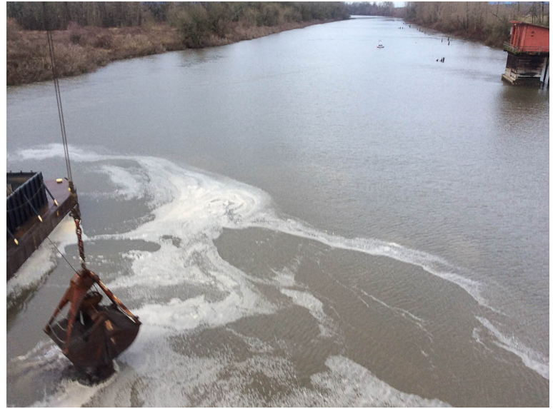
In-water ENR Sand Placement
