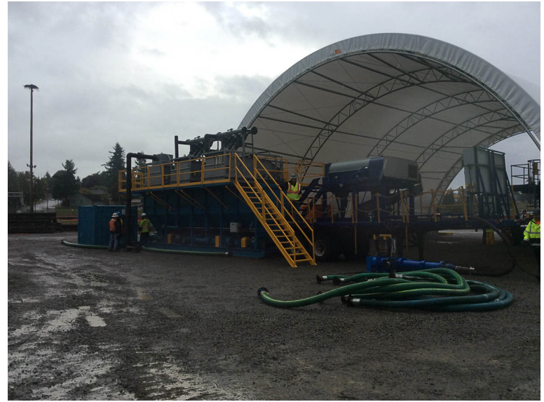
Setting up water treatment system in MHA.
