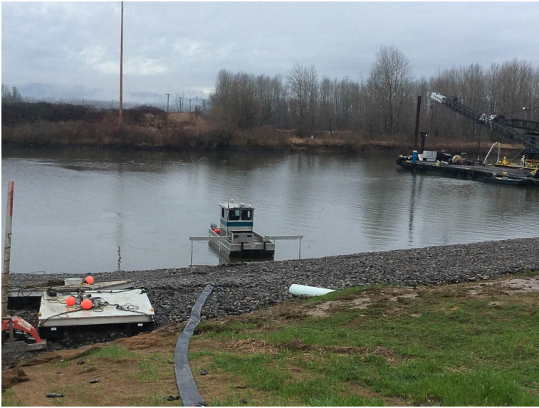
Survey of Fish Mix Placement near kayak launch.
