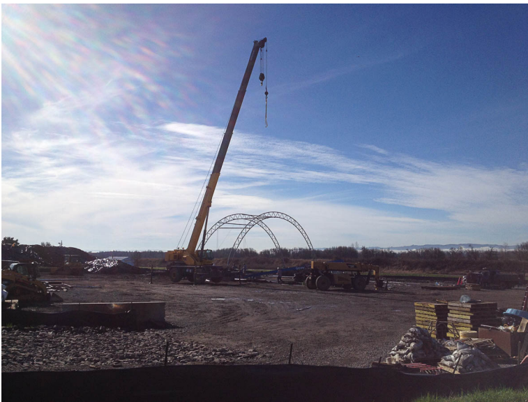
Dismantling tent structure within MHA.
