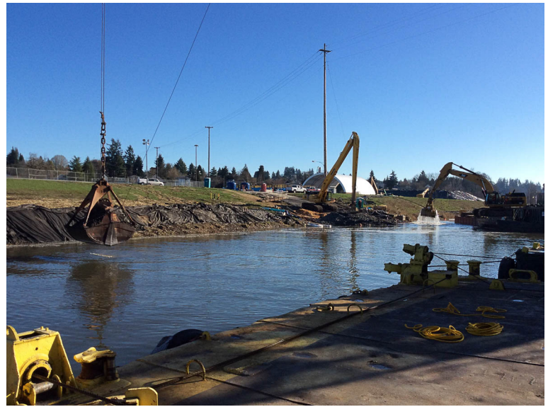
Sand placement and dredging near transload operation.
