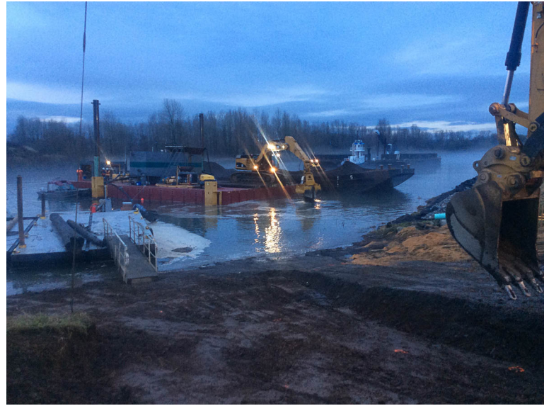
In-water ENR Sand Placement
