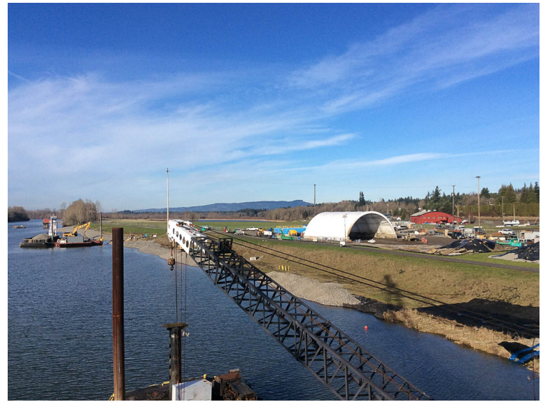
View of MHA and dredge barge.
