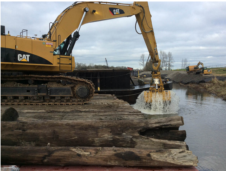
Dredging in shallow water.
