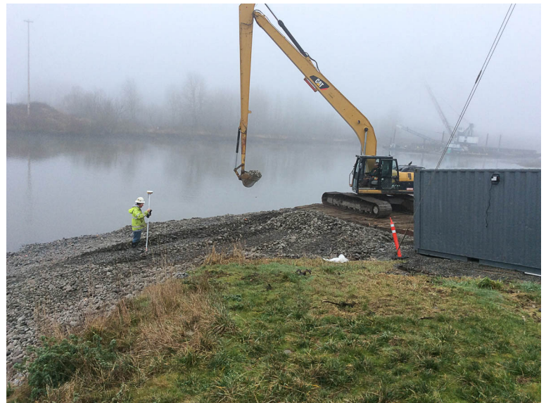
Fish Mix Grading at kayak launch
