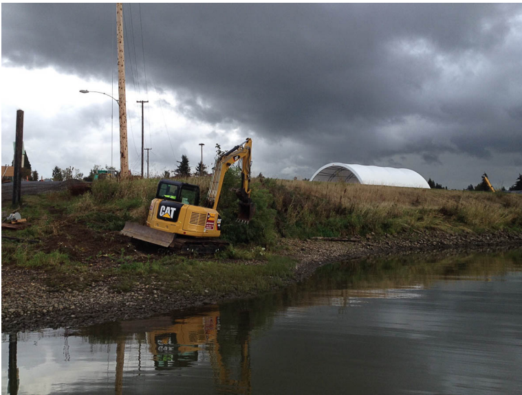
Limited vegetation removal near Division St.
