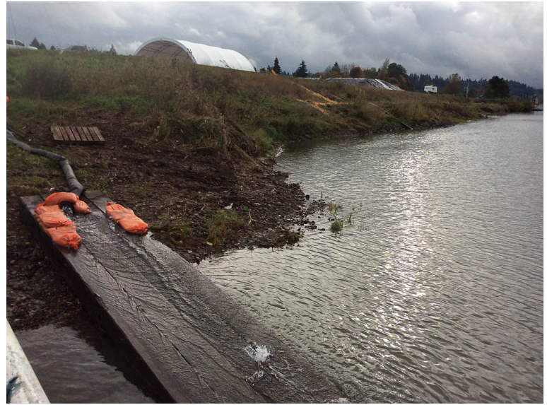
Treated dredge water discharged back to Lake River.
