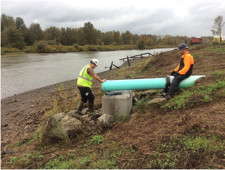
Building stormwater extension north of Division St.
