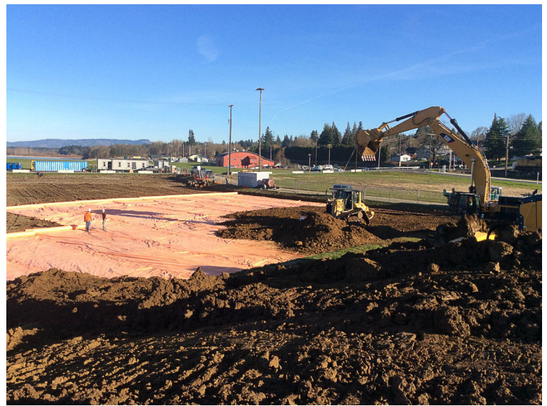
Clean soil cap placement.
