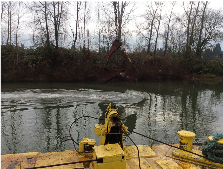
In-water ENR Sand Placement
