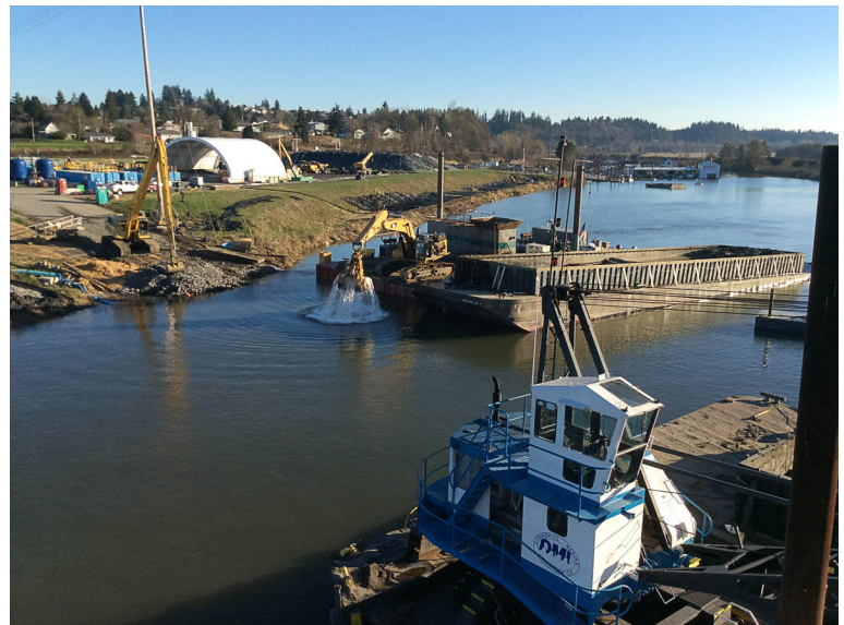
Dredging near transload operation.
