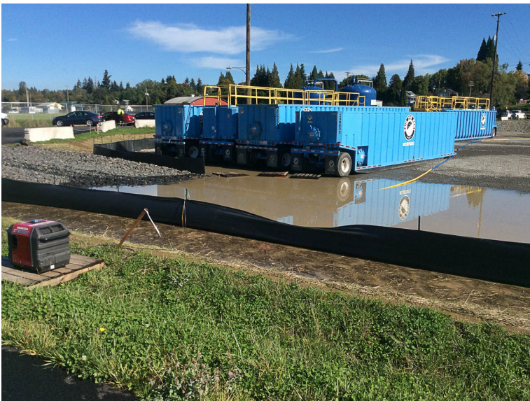
Pumping MHA stormwater into holding tank from 10/15/14 rainfall event.
