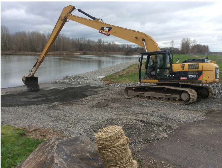
Long reach excavator grading rock at the kayak launch.
