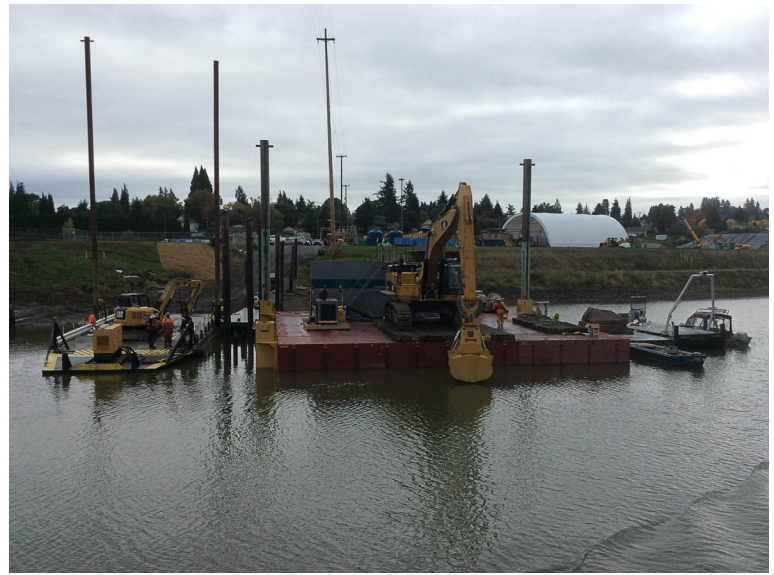
In-water equipment for pile removal and dredging.
