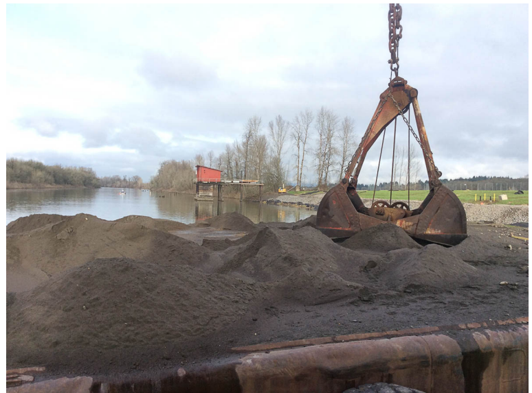
Crane operator grabbing sand.
