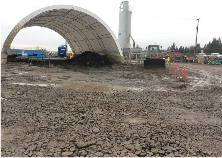
Remaining material at MHA.
