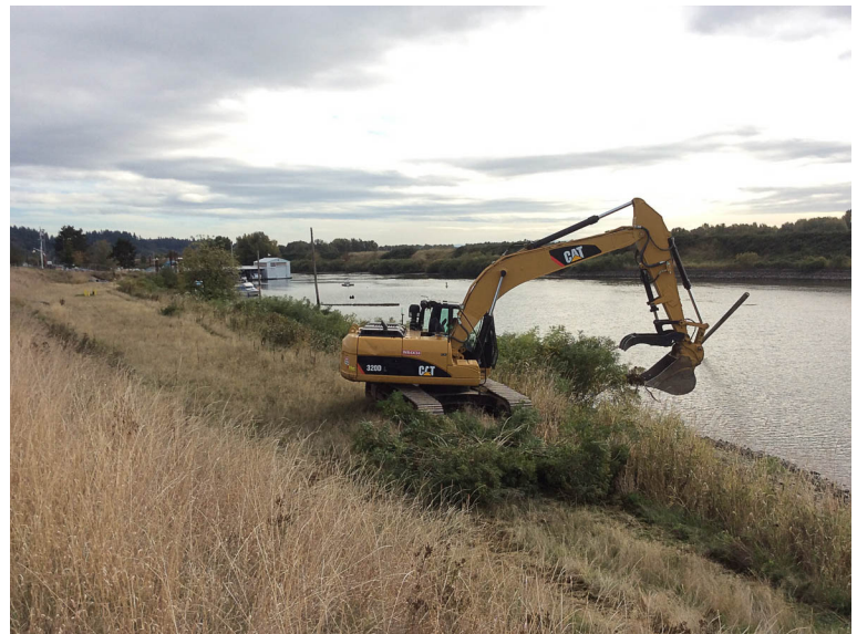
Removing vegetation along shoreline south of Division Street.
