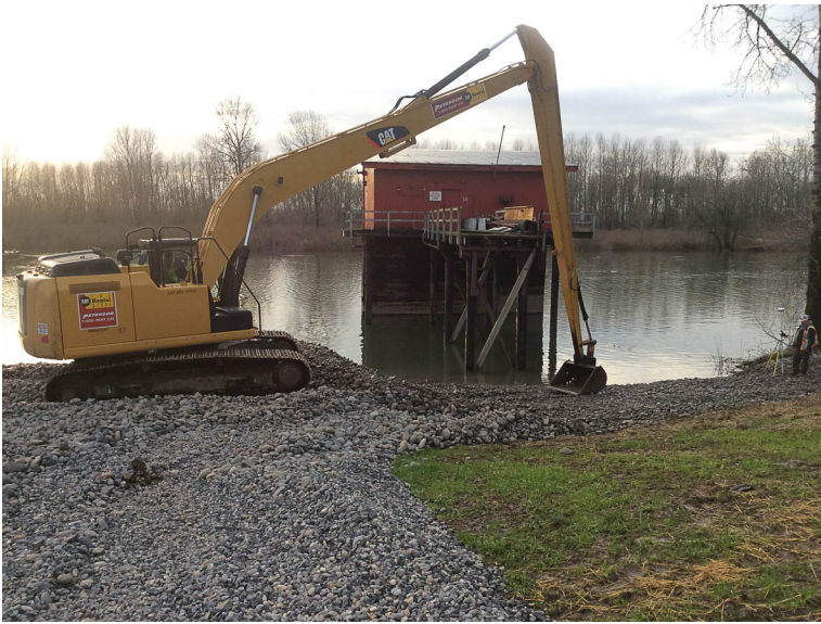
Long reach excavator grading fish mix.
