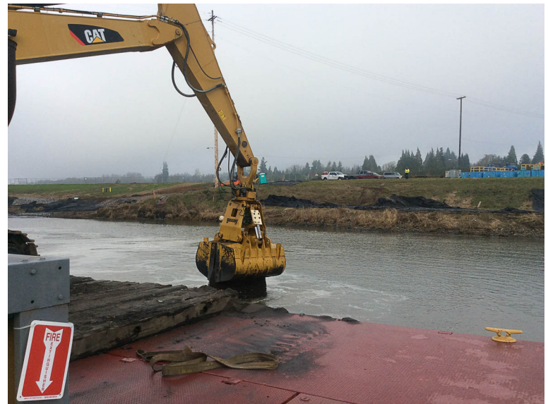
In-water ENR Sand Placement
