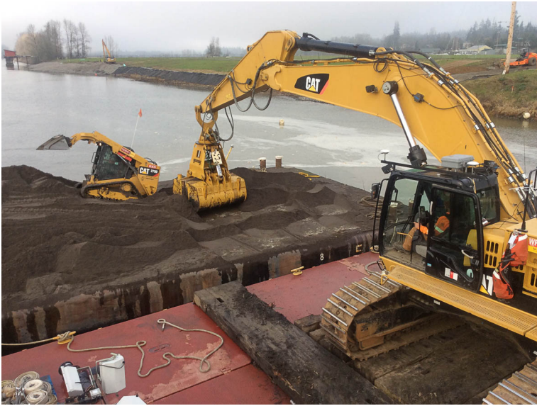
Young's Bucket picking up sand from a materials barge.
