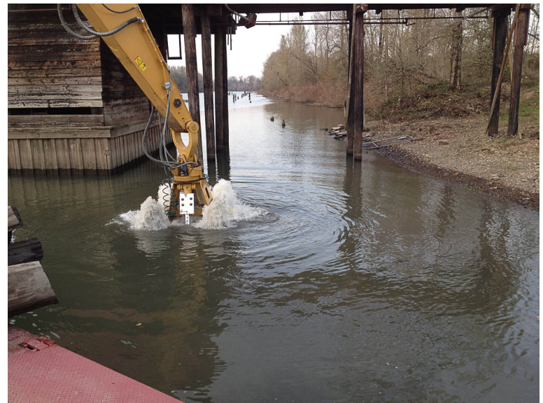
Dredging in shallow water.
