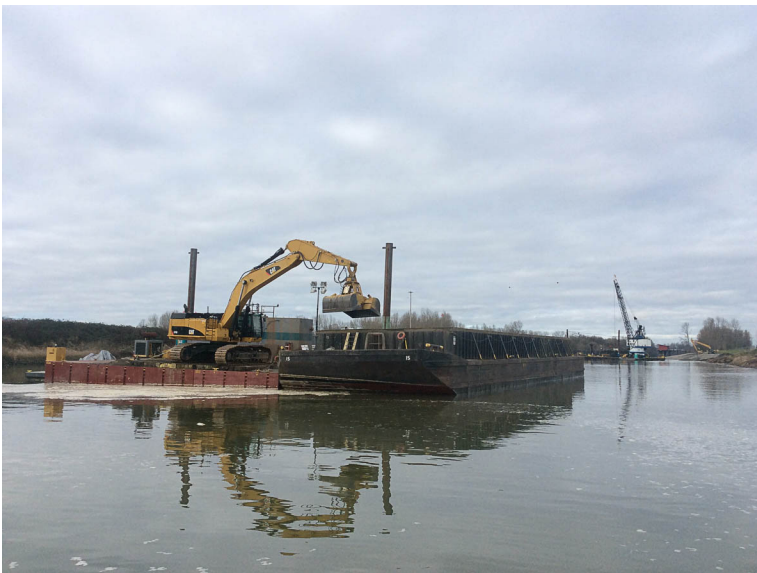
In-water ENR Sand Placement with Young's Bucket.
