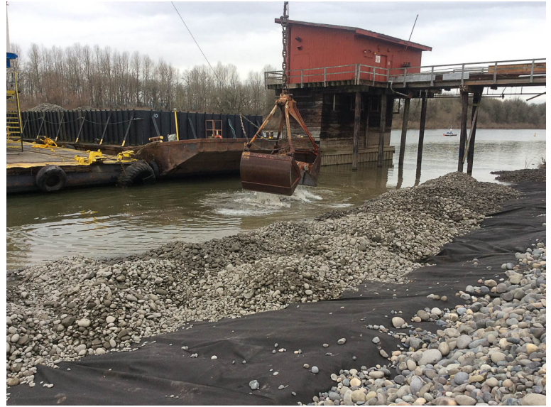
Fish Mix Placement from in-water.
