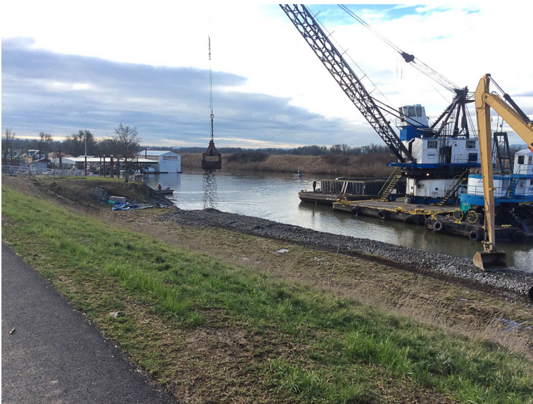
Upstream Fish Mix Placement.
