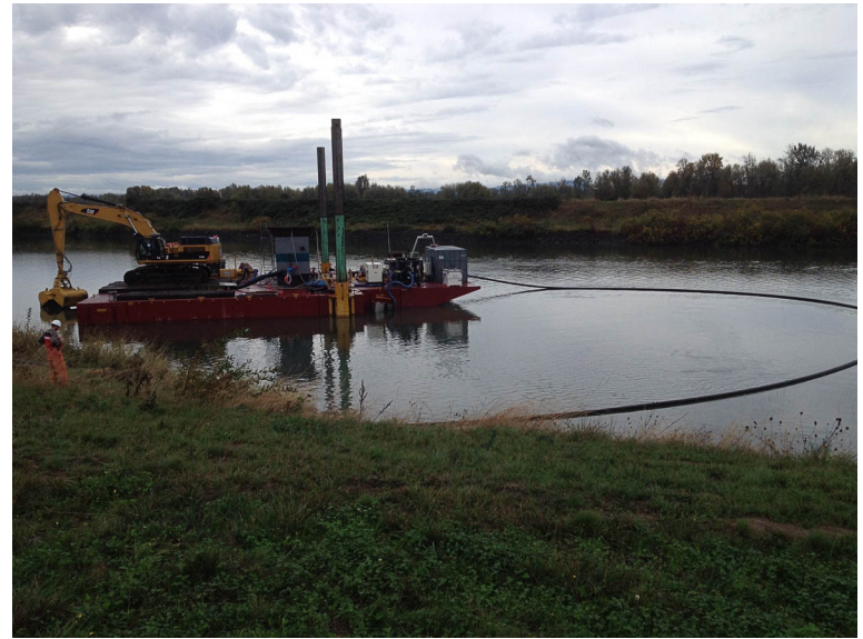
Dredge barge and pipeline
