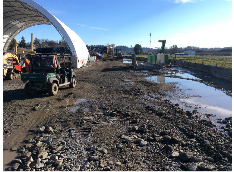
Rock removed from MHA exit.
