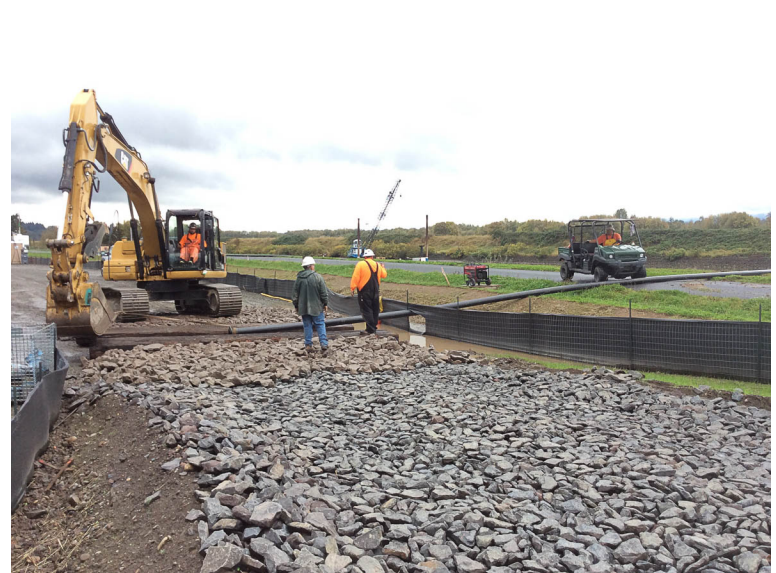
Constructing pathway for pipeline in MHA.
