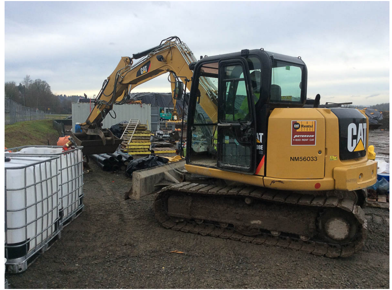
Demobilization of materials in MHA.
