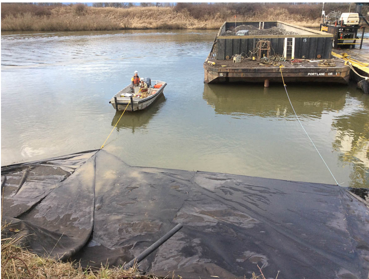
Laying out filter fabric before fish mix placement.
