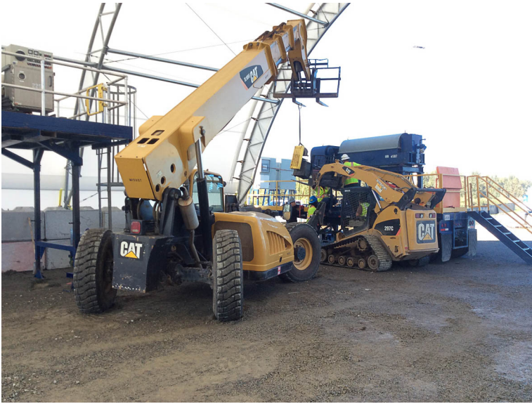
Assembling the water treatment system in the MHA.
