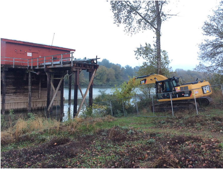
Vegetation removal on northern boundary shoreline using excavator.
