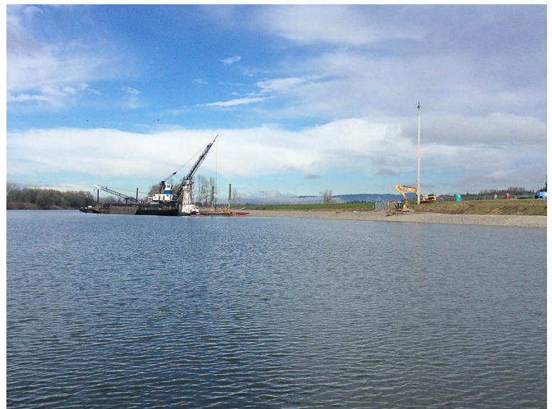
Fish Mix Placement in low spots downstream.
