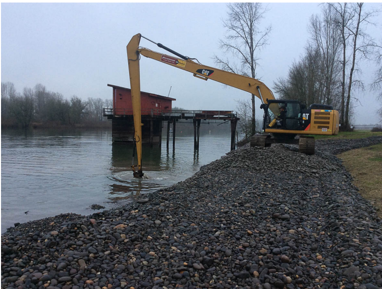
Excavator grading fish mix in water.
