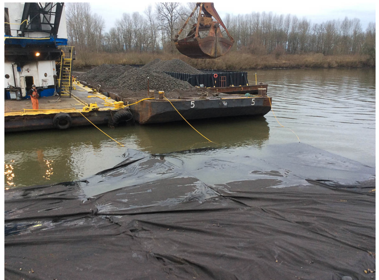
Fish Mix Placement on filter fabric.
