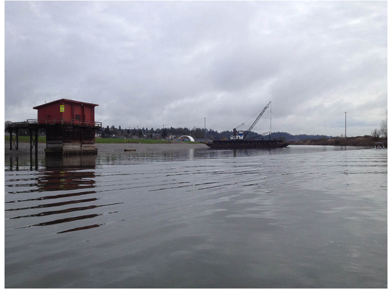
Fish mix rock along shoreline near pump house.
