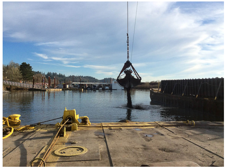
ENR sand placement between Division Street and Mill Street.
