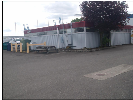
EXTERIOR VIEW - NORTHEAST CORNER
