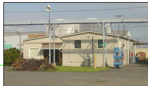
EXTERIOR VIEW - WEST SIDE
