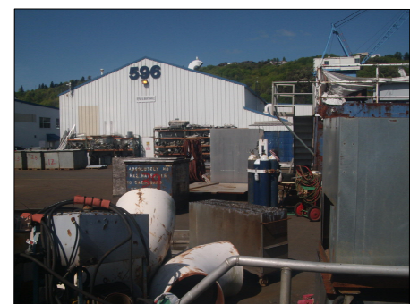
EXTERIOR VIEW - WEST SIDE
