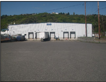
EXTERIOR VIEW - WEST SIDE
