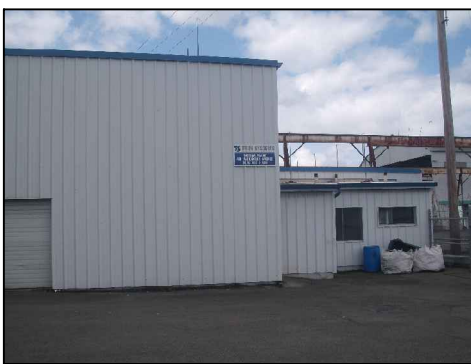
EXTERIOR VIEW - SOUTH SIDE
