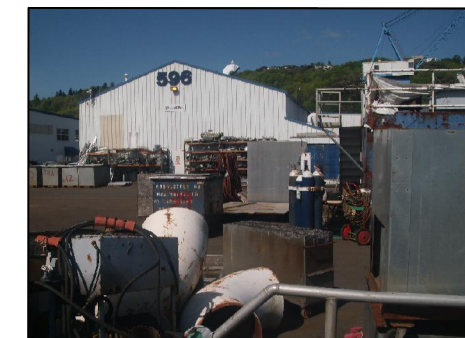
EXTERIOR VIEW - WEST SIDE
