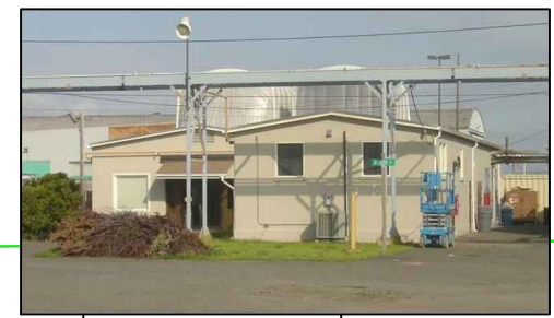
EXTERIOR VIEW - WEST SIDE
