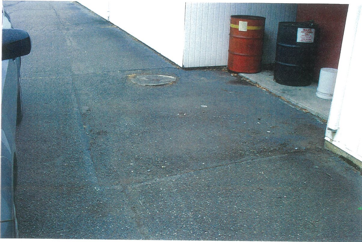
1989 WASTE OIL TANK EXCAVATION AREA AND WATER SAMPLING WELL
