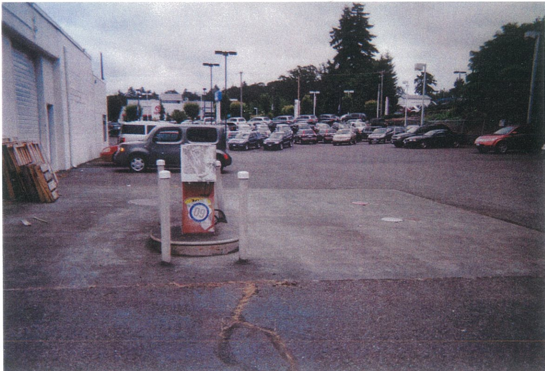
4,000 GALLON GASOLINE UST, 500 GALLON WASTE OIL UST, AND FUEL DISPENSING ISLAND
