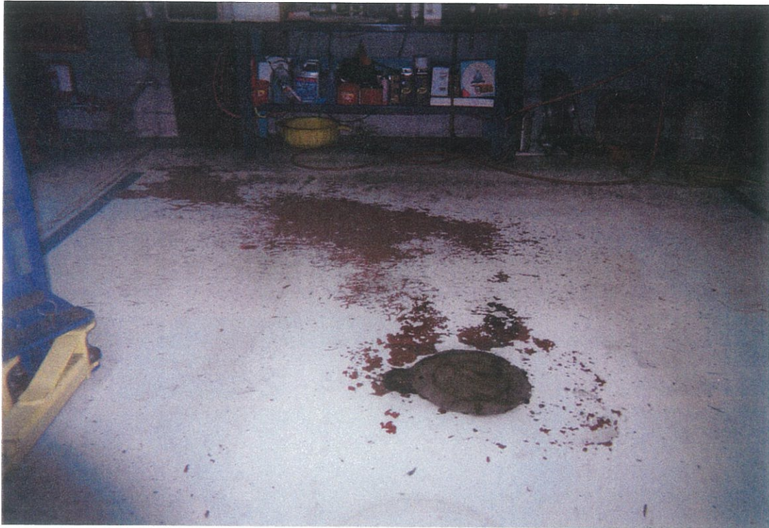
ABANDONED SINGLE POST UNDERGROUND HYDRAULIC LIFT IN MAINTENANCE/SERVICE AREA
