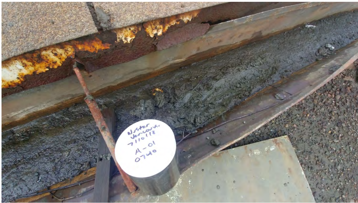
Photo 1 (top) Roof of NuStar Building #2655. Facing south.
