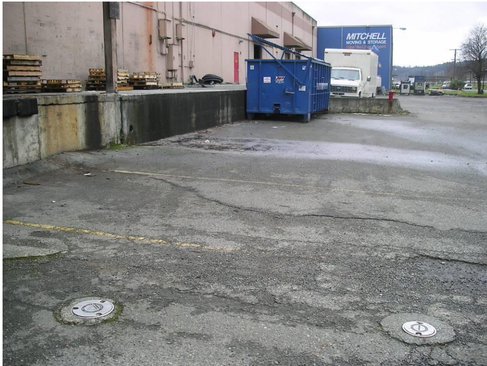
Photo 3: Former Tank Area – from the north.
