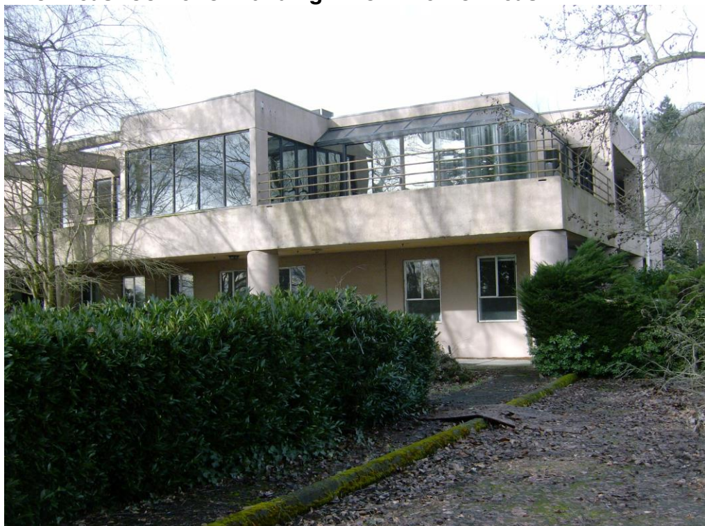
Photo 2: Northeast Corner of Building – from the Northeast
