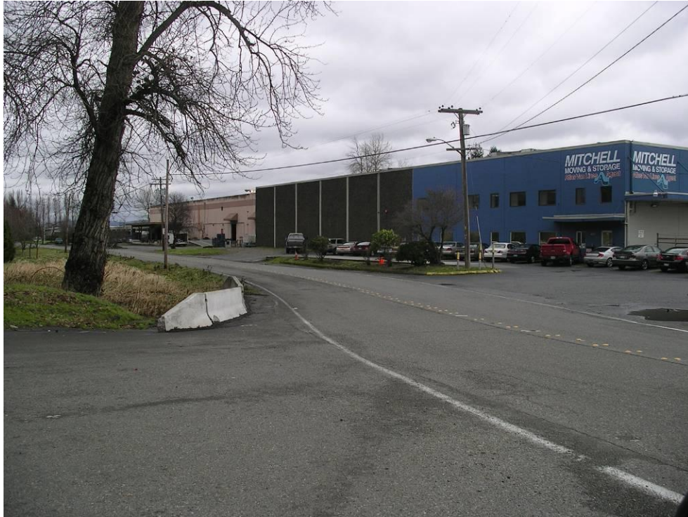
Photo 1: Southwest Side of Building - from the southwest
