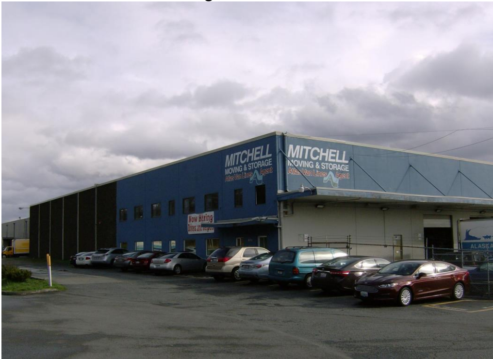
Photo 1: Southwest Side of Building - from the southwest
