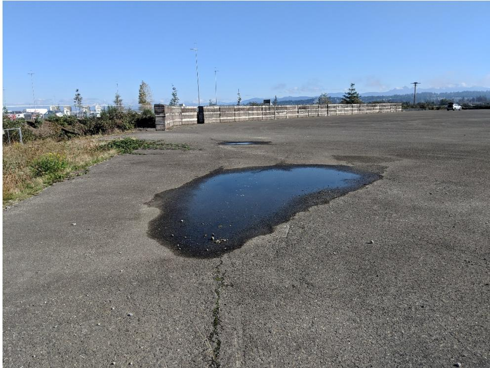
Photograph 1. Crack in asphalt and ponding on northwest side of the cap (looking north).
