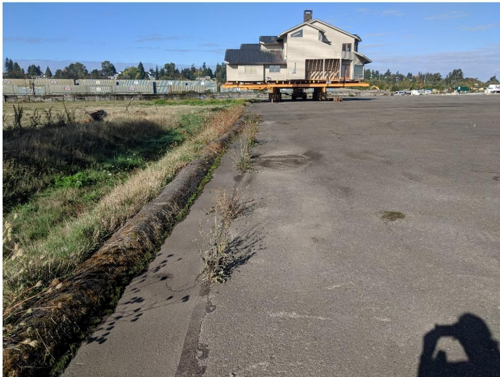
Photograph 4. Crack in the asphalt with growing vegetation along the south edge of the cap (looking west).
