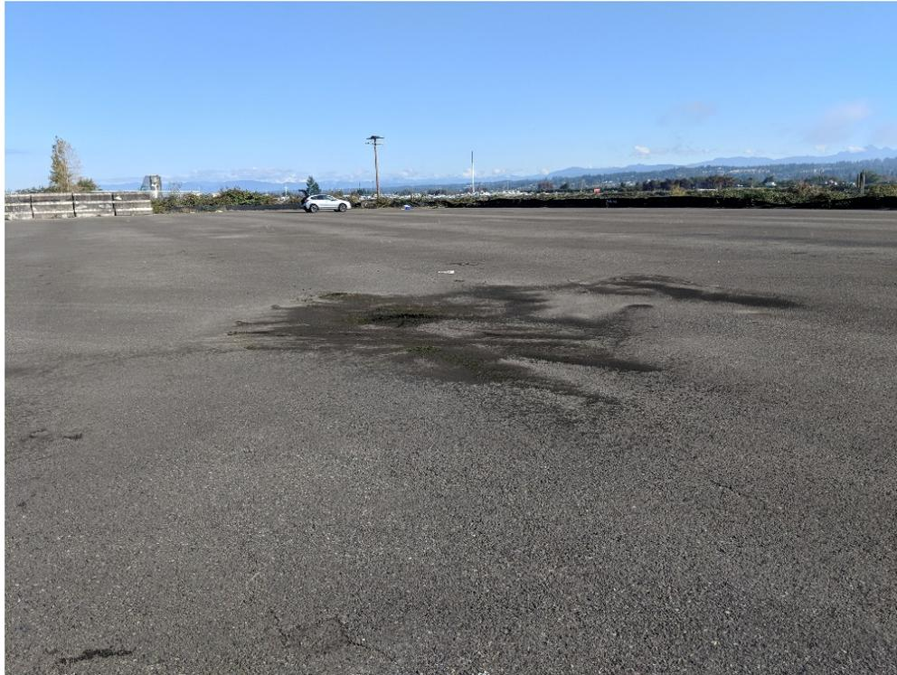
Photograph 3. Settled area with deposited dust and debris (looking northeast).
