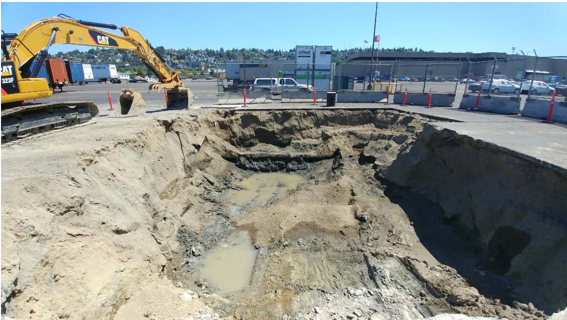
Excavation at conclusion of remediation, with view looking E. July 16, 2018.
