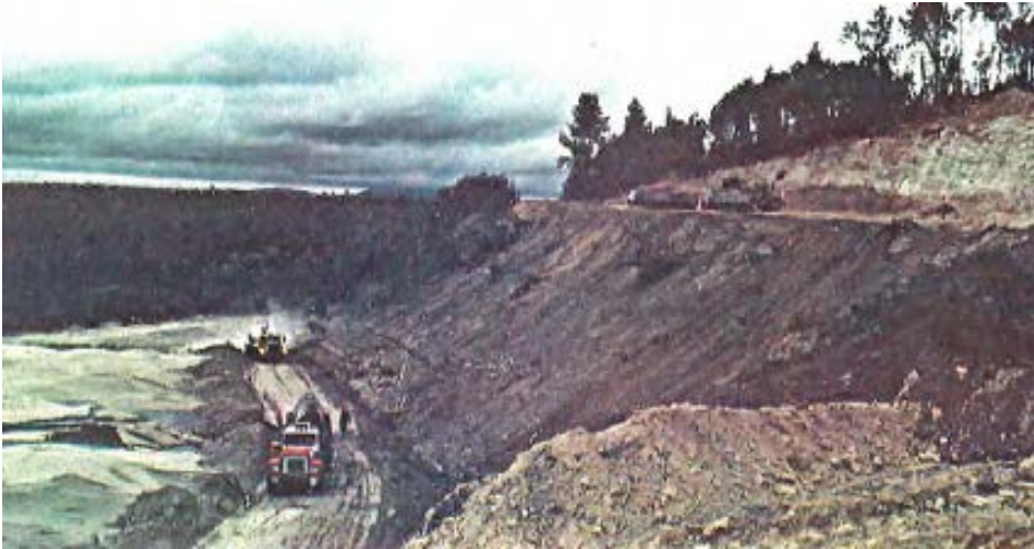
1982 Cement kiln dust Lower Disposal Area
