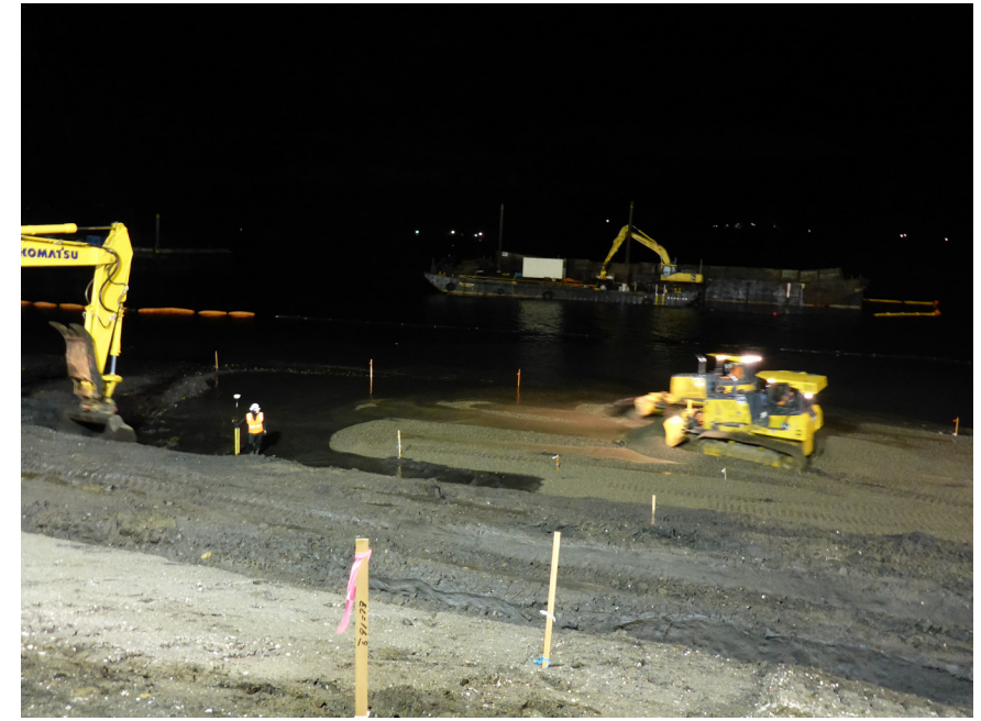
Intertidal excavation and placement of filter material
