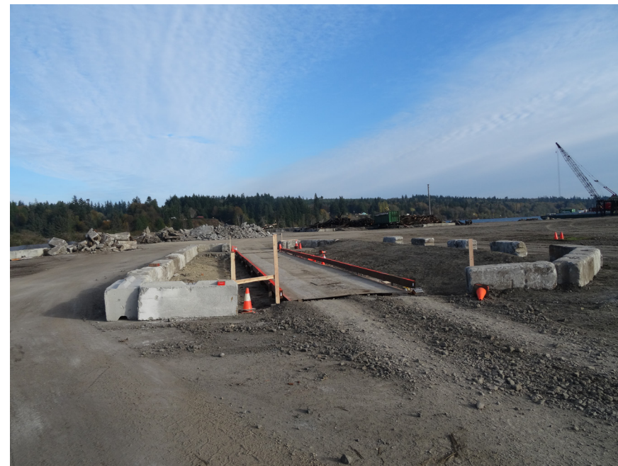
On-site truck scale
