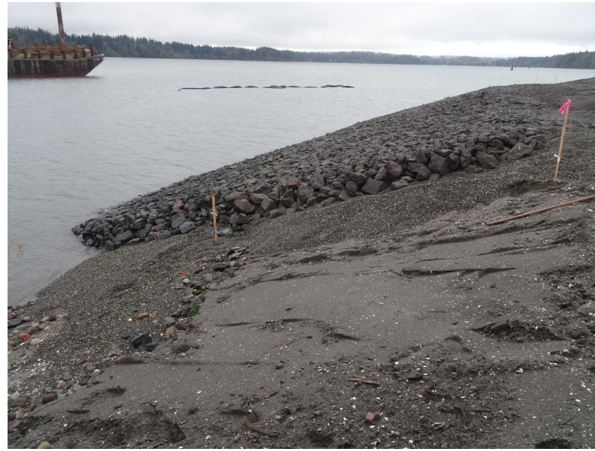
Section of completed SMA-2 intertidal cap
