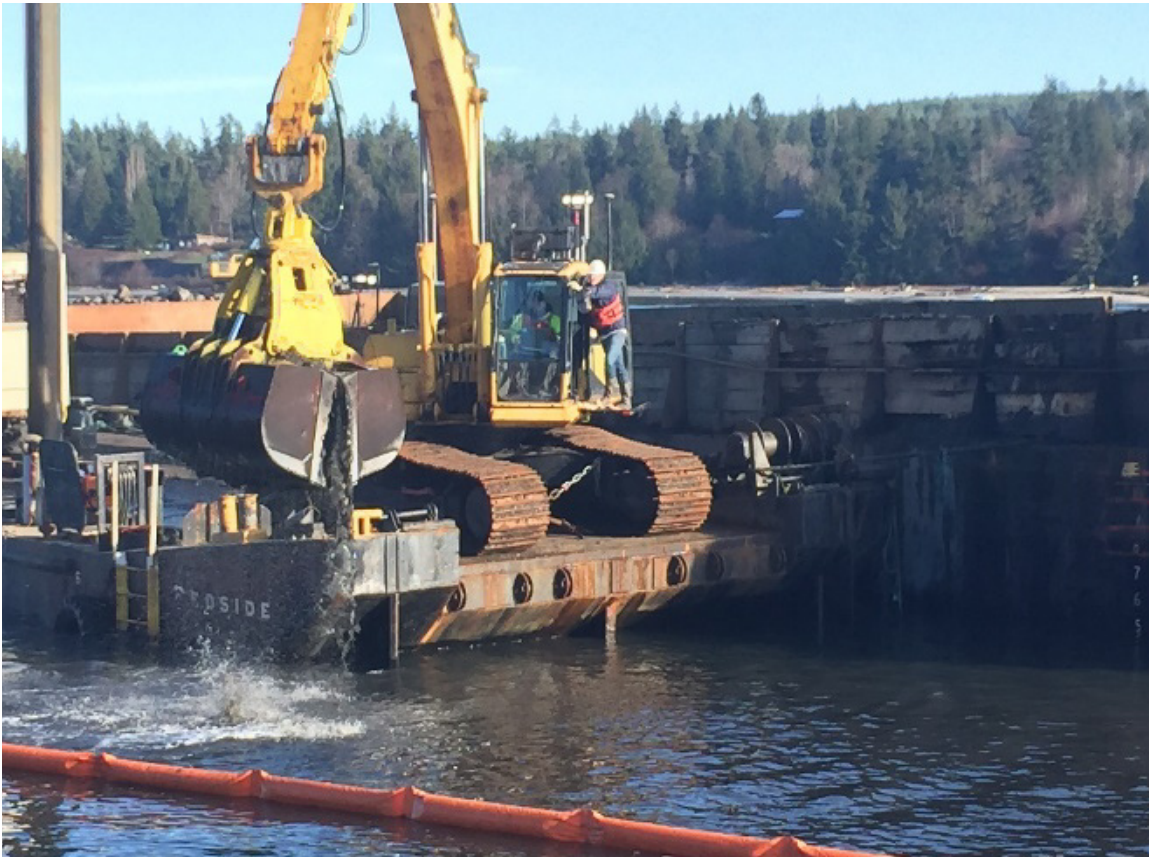
Figure ES-3 – Subtidal Dredging in SMA-2
