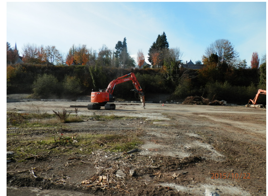
Perforating stockpile area
