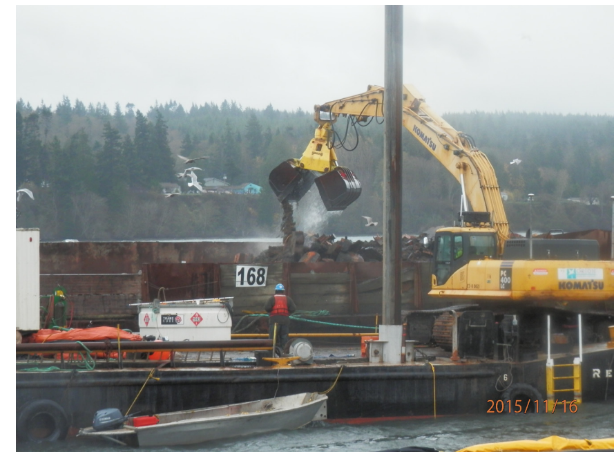
Subtidal dredging in area with larger wood debris
