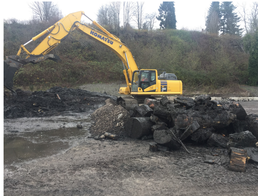
Removing large wood debris from subtidal dredge material stockpiles
