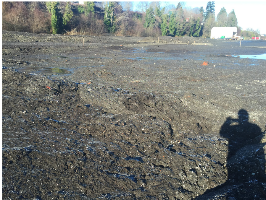
Subtidal dredging stockpiles
