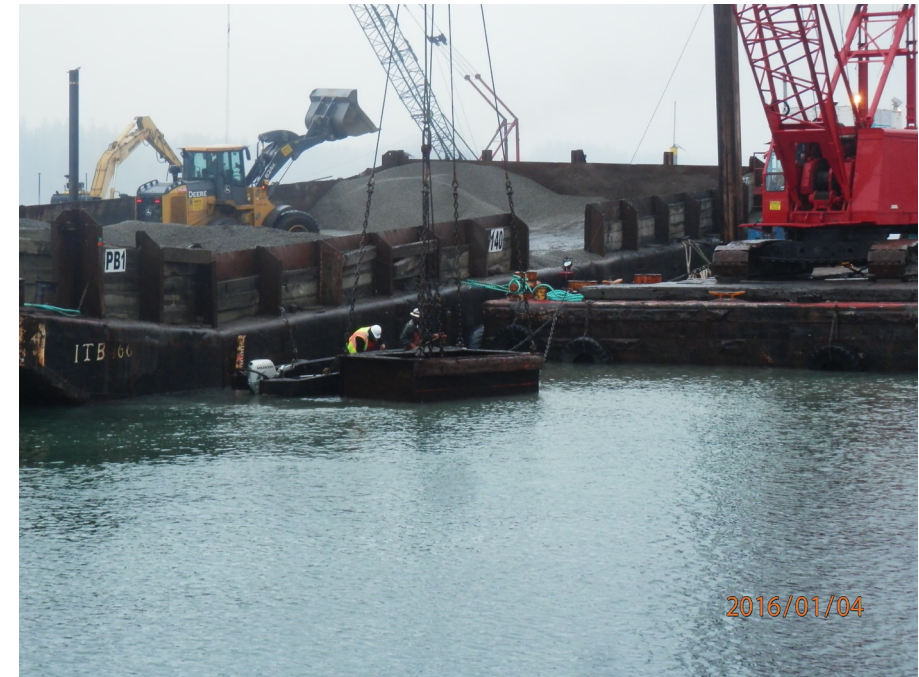
Placing shallow subtidal cap filter material layer
