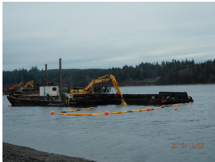
Subtidal dredging with the PC400 Komatsu excavator in SMA-2
