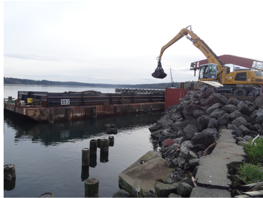
Dredge material barge moored at transload bulkhead
