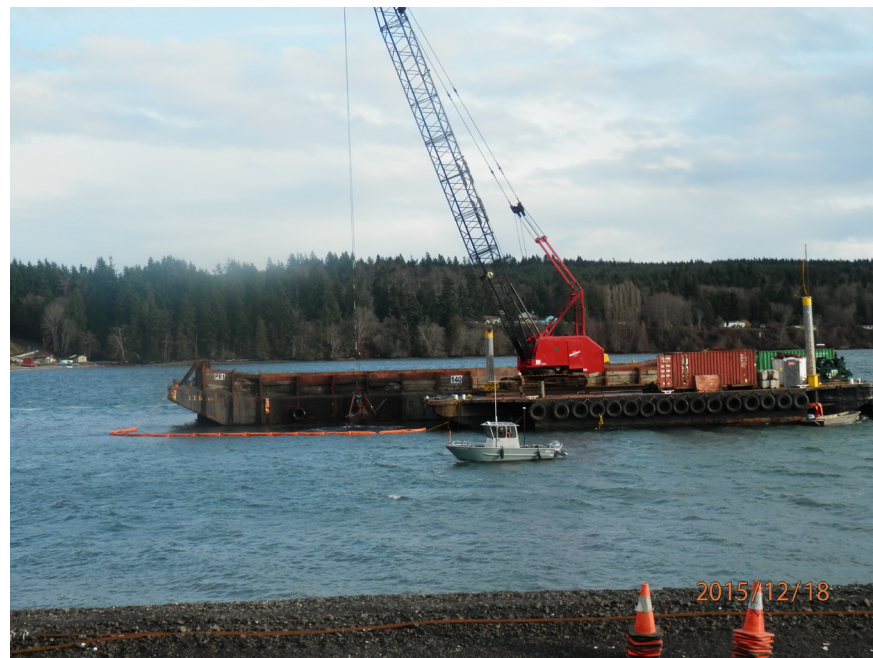
Subtidal dredging with the Maniwoc 3900 crane and clamshell bucket in SMA-2
