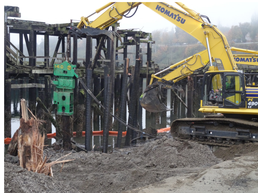
Intertidal pile removal
