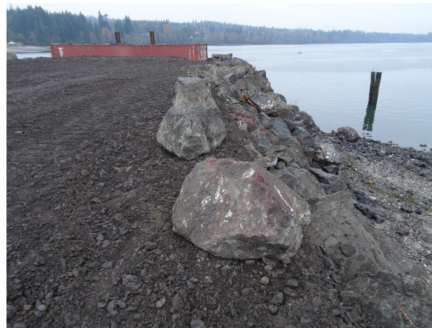
Temporary transload bulkhead
