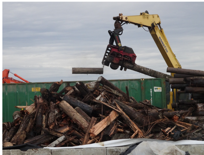
Creosote pile processing
