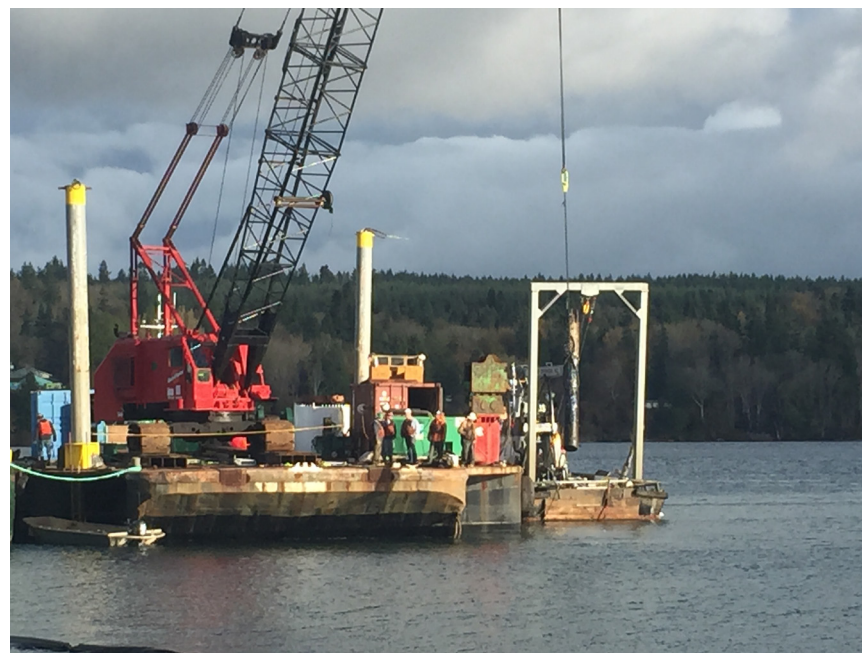
Diver assisted submerged subtidal pile removal
