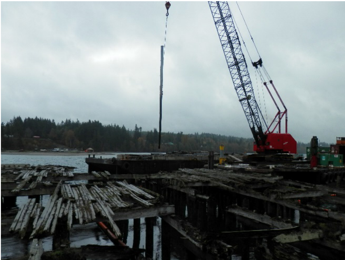
Figure ES-2 – Demolition of Eastern Wharf
