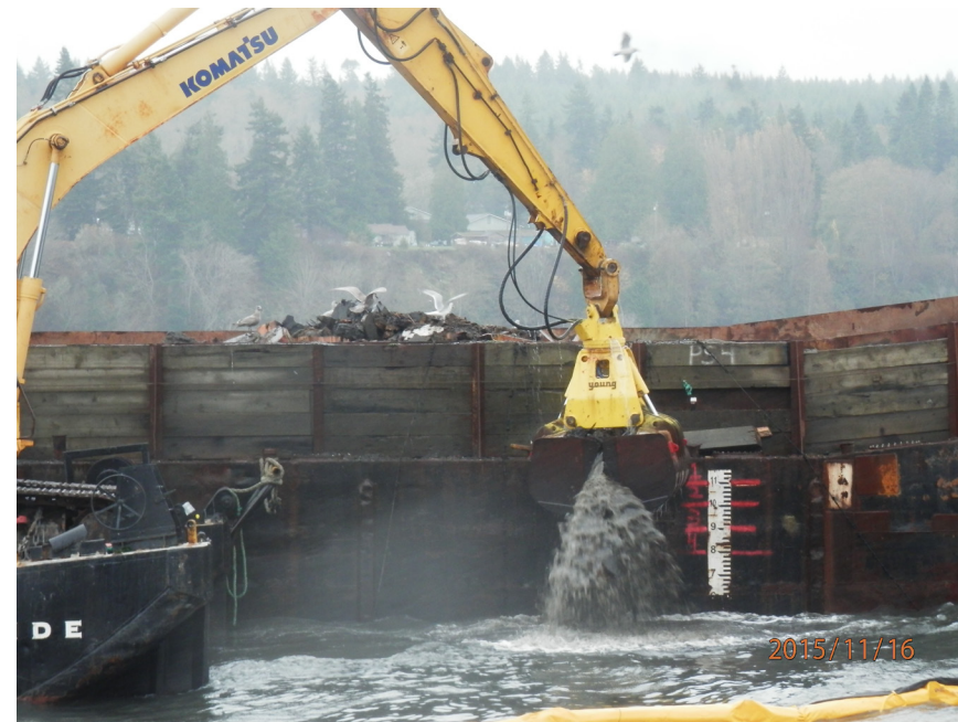
Hydraulic Young bucket used on the PC400 excavator
