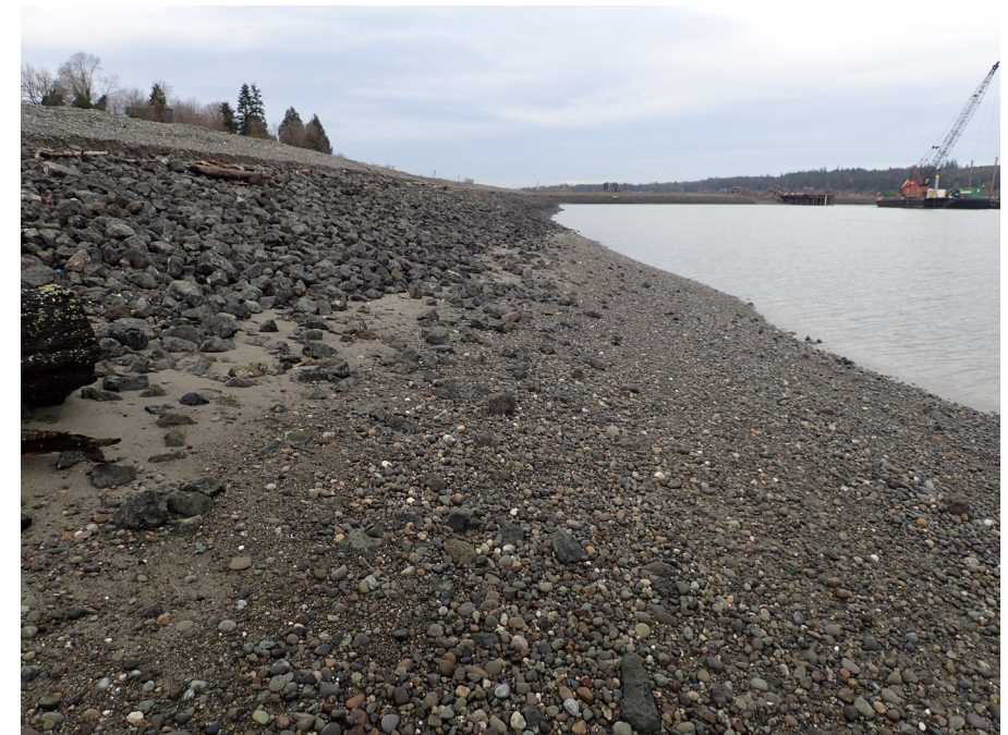
Completed intertidal cap area in SMA-2
