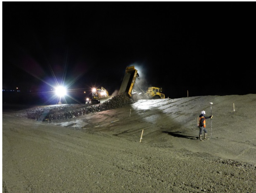
Placement of Type 2 armor layer in SMA-2 intertidal cap
