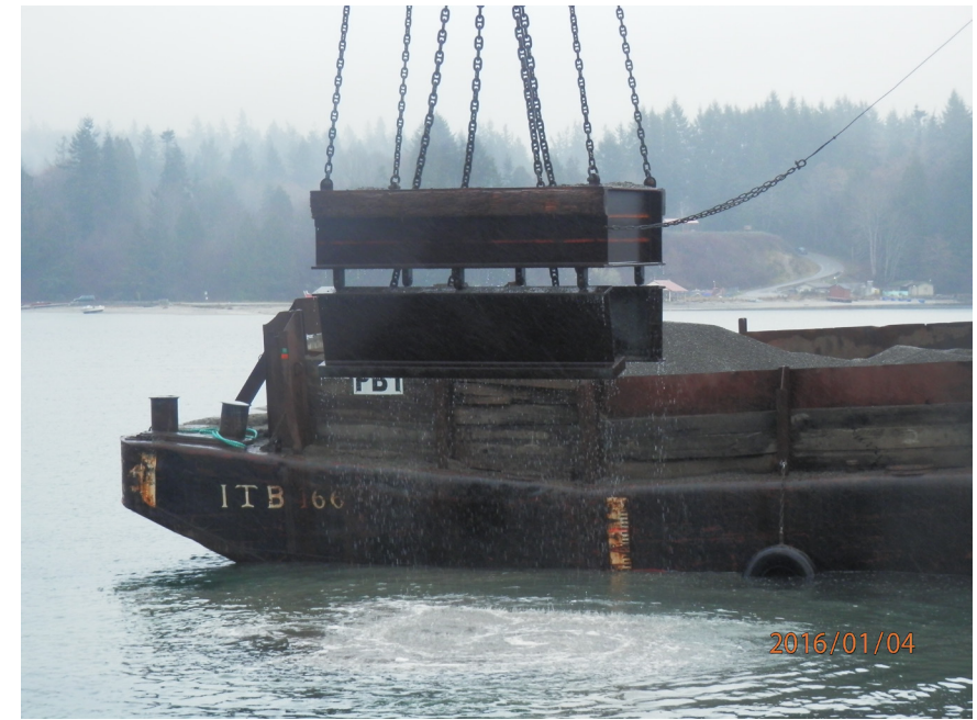
Placing SMA-2 subtidal cap using the Bombay box
