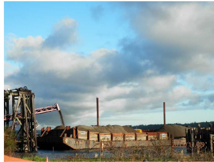
Loading sand cap material for capping in SMA-2
