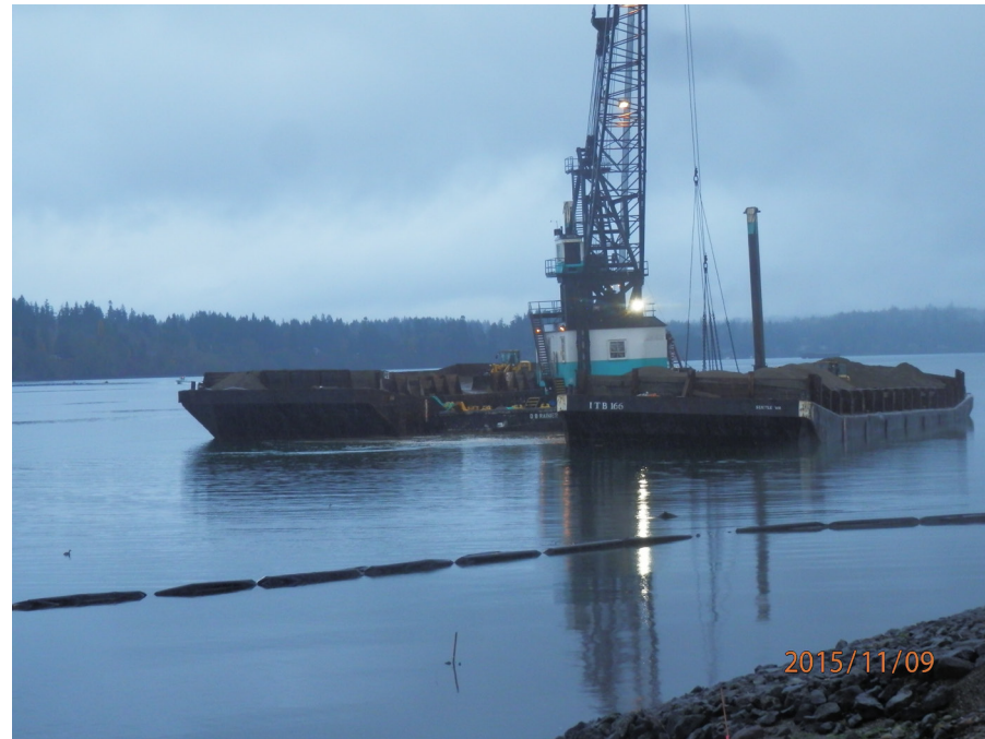
Placing SMA-2 subtidal cap with the DB Rainier and Bombay box
