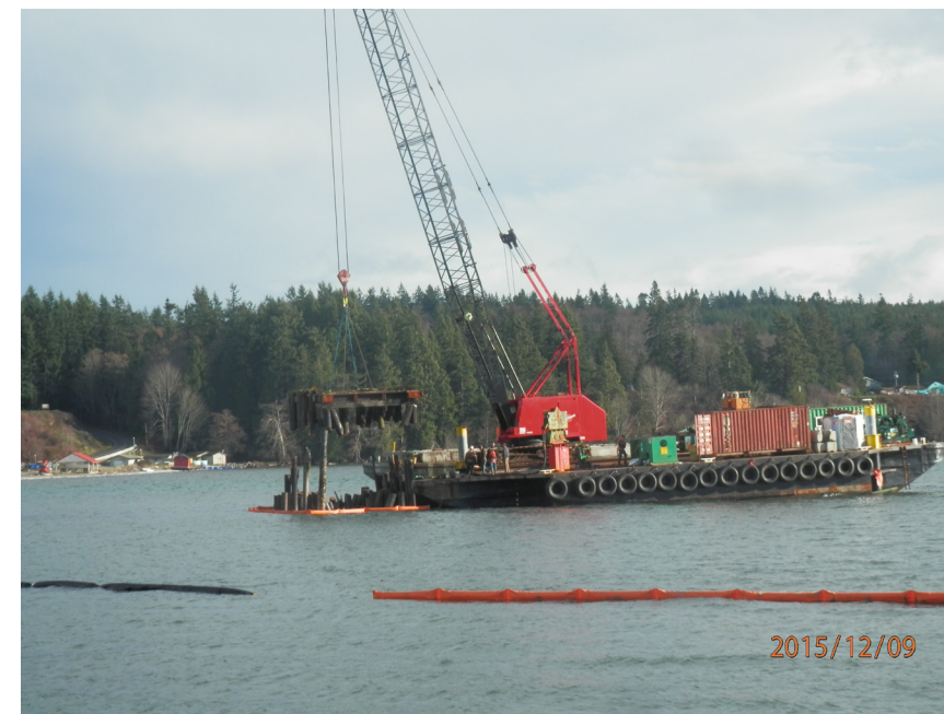
Offshore Alder Chip Pier demolition
