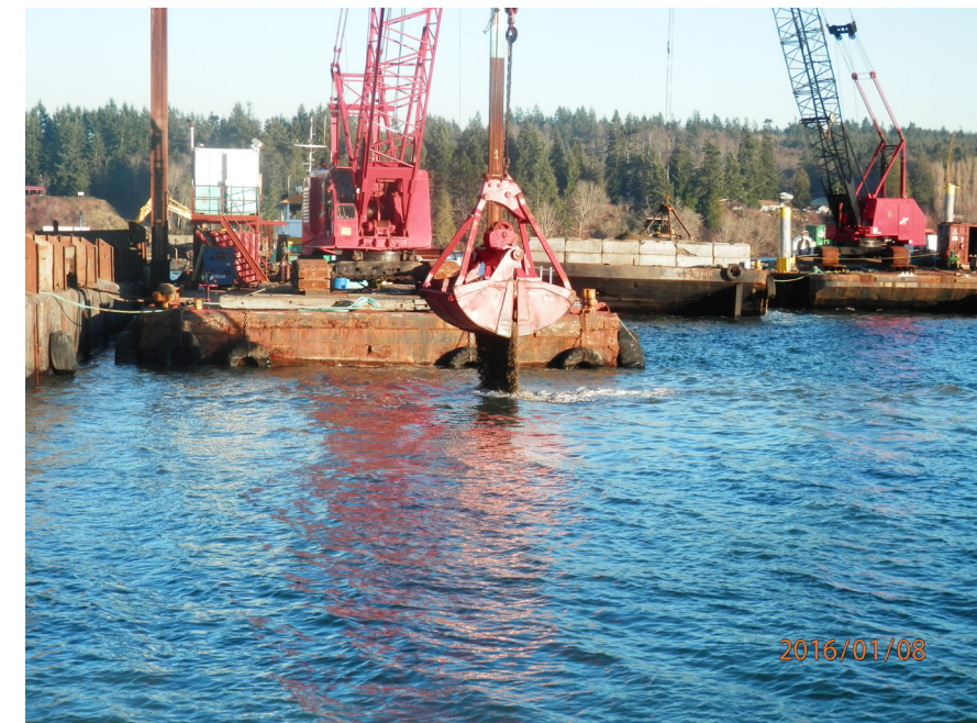
Placement of post-dredging RMC in SMA-2
