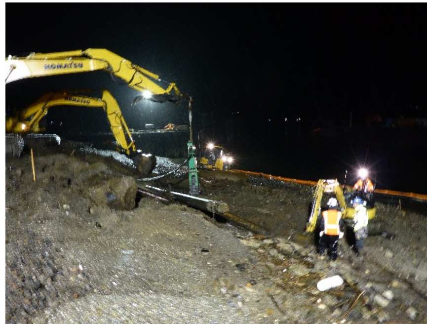
Removal of piles encountered during intertidal excavation
