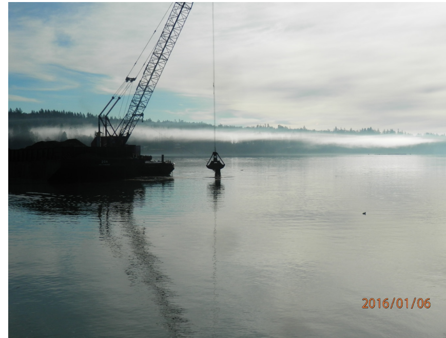
Placing EMNR material with the Manitowoc 3900 crane and clamshell bucket
