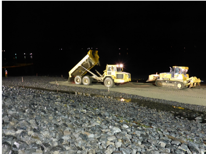
Placing habitat substrate over Type 3 armor
