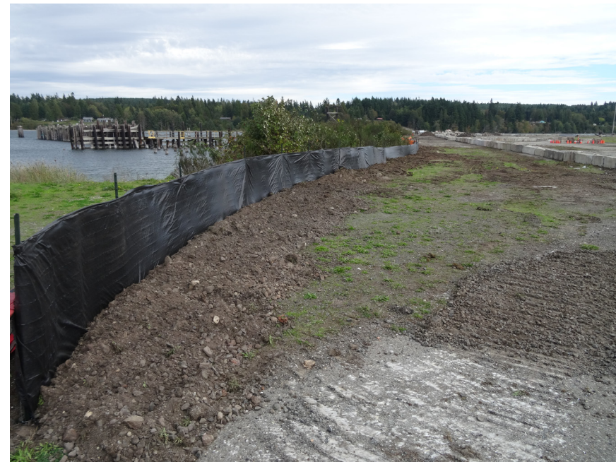
Perimeter silt fence installation
