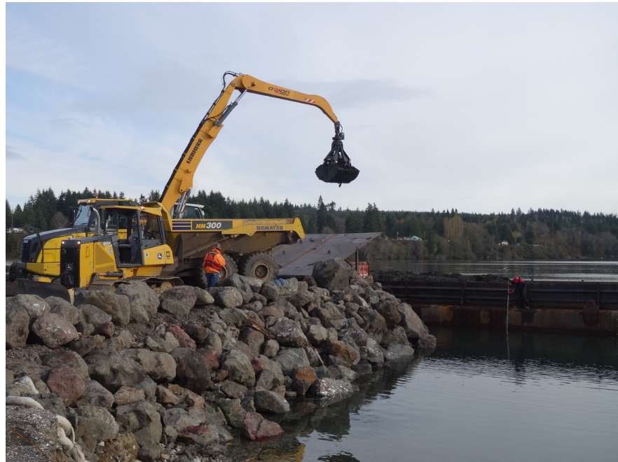
Offloading a dredge material barge at the transload facility
