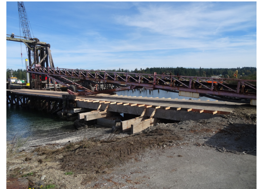
Installation of clean capping material barge loading conveyor
