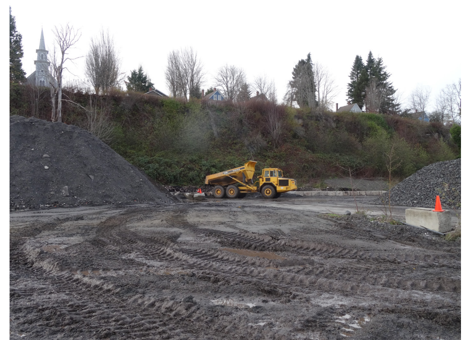
Transporting dredge material to stockpiles
