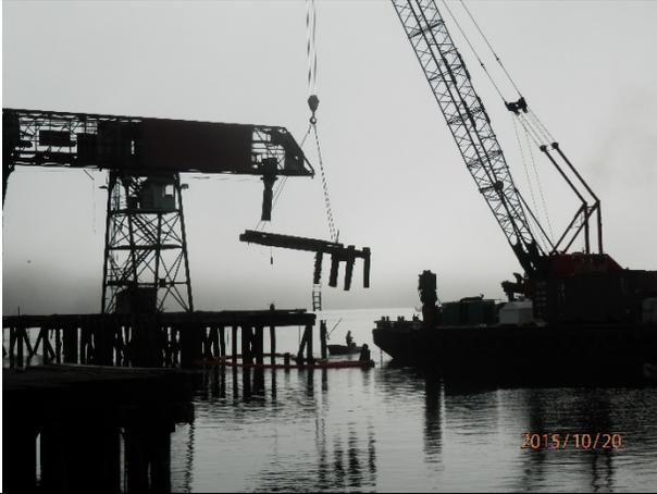
Description: Removing pier sections in subtidal area in SMA-2.
