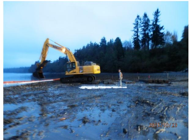
Description: Grading intertidal pile removal area in SMA-2.
