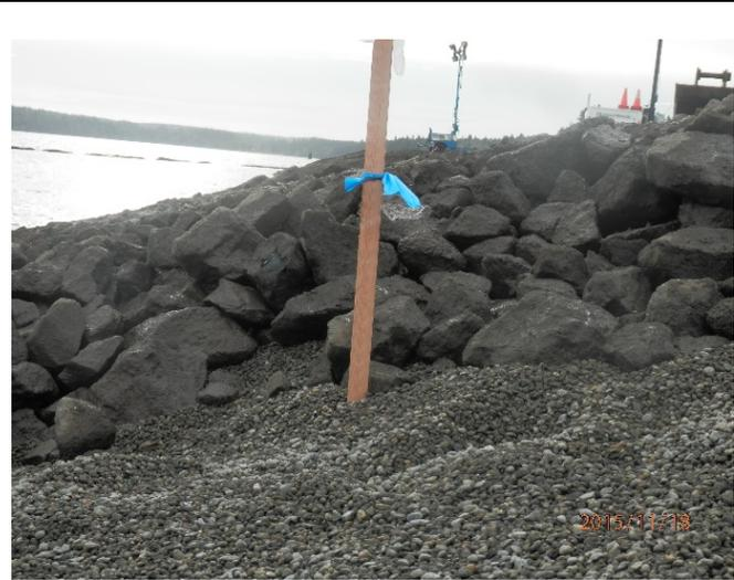
Description: Edge of intertidal cap placement area showing completed armor thickness and grade stake.
