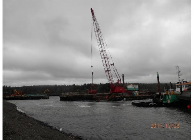
Description: Placement of interim sand cover in south portion of SMA-2 northern dredge prism.
