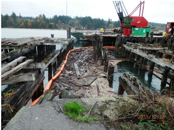
Description: Eastern Wharf area pier demolition and debris boom.
