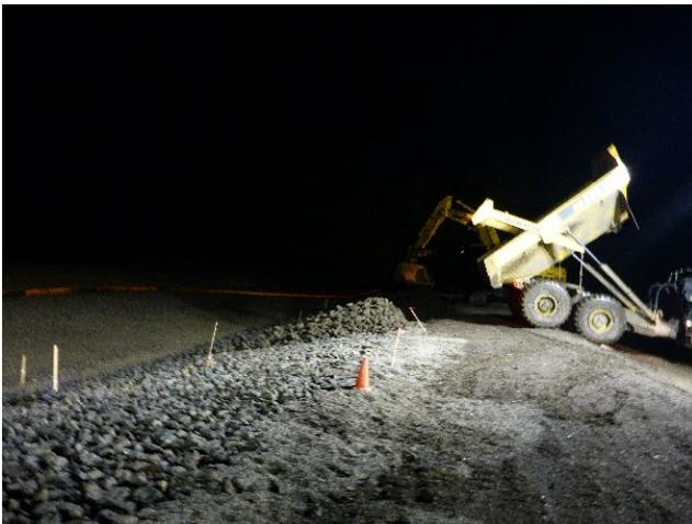
Description: Unloading and spreading Type 2 cap armor.
