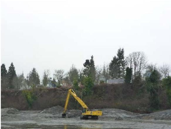
Description: Sorting and consolidating dredge material with excavator.
