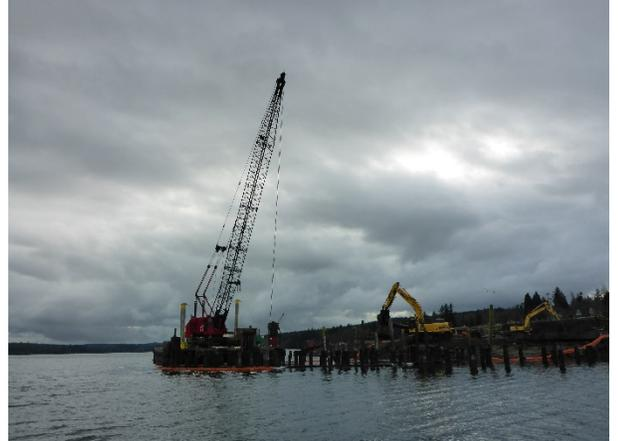
Description: Pile and debris removal in Eastern Wharf with crane and excavator.
