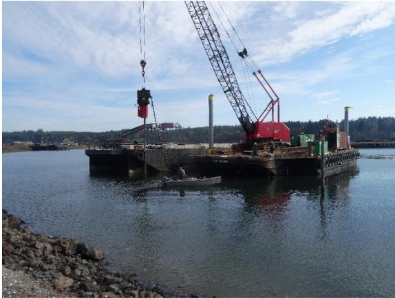
Description: Removing the last row of individual subtidal piles within SMA-2.
