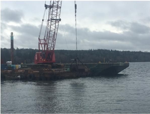
Description: Pile extraction attempt with clamshell digging bucket from dredge area near former Pier 5 location.
