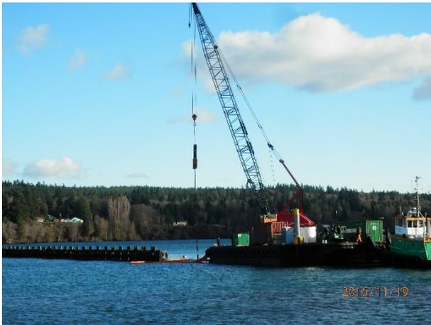
Description: Demolition of breakwater structure in SMA-2.
