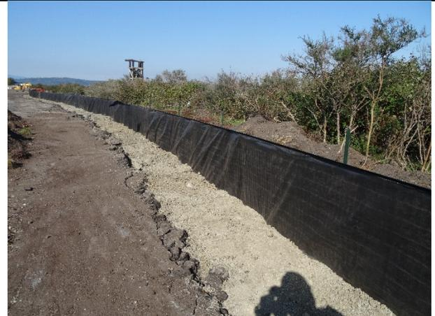
Description: Silt fence installation at creosote processing area.
