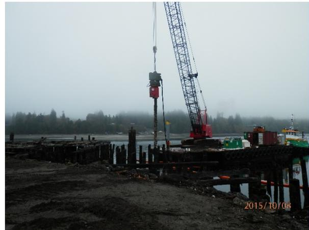
Description: Subtidal pile removal with crane from barge at Station 18+00.
