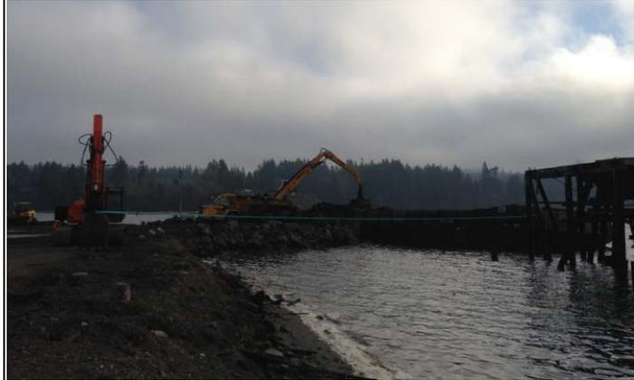
Description: Offloading dredge sediment barge at temporary offload facility and installation of rigging for conveyor structure demolition.
