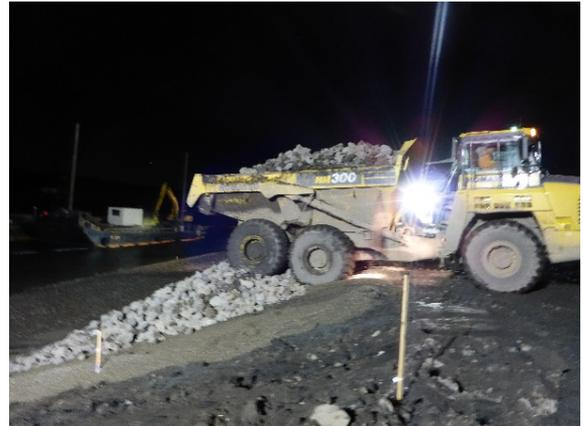
Description: Intertidal capping with Type 2 armor capping material.
