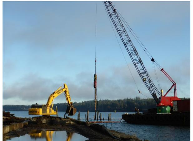
Description: Pile and debris removal in Eastern Wharf area with vibratory hammer from barge and excavator from shoreline.
