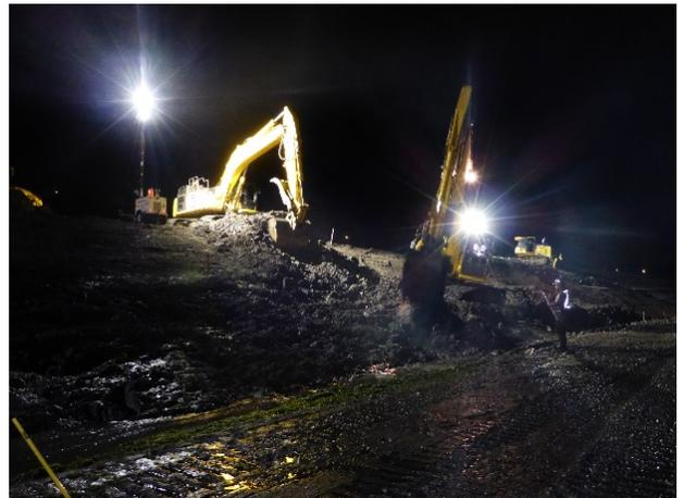
Description: Excavators clearing and grading excavation work area.
