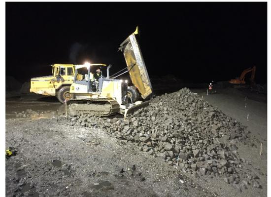
Description: Placement of Type 2 armor material on 3:1 slope.
