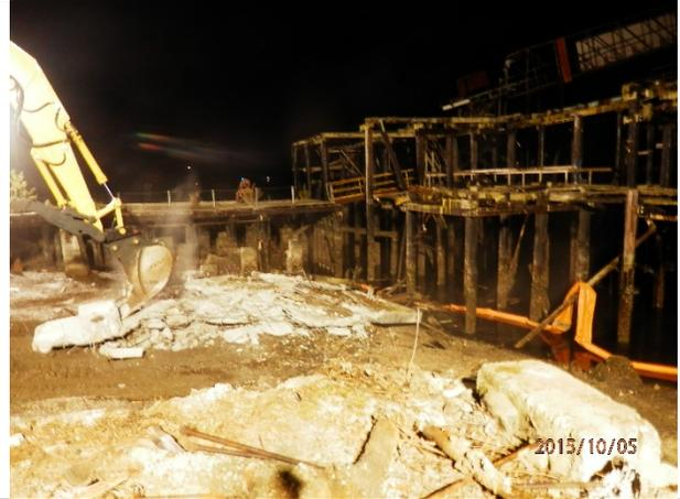
Description: Demolished elevated concrete portion of nearshore Alder Chip Mill Pier.
