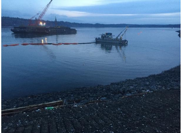
Description: Capping in SMA-2 and collecting confirmatory post-dredge sediment cores.
