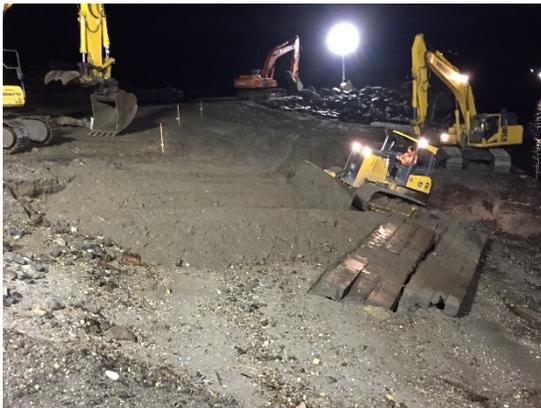
Description: Excavating and grading intertidal bank to 3:1 slope.
