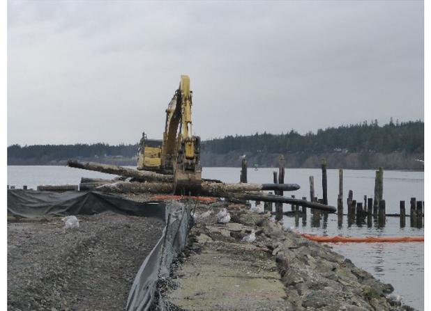
Description: Pile removal in Eastern Wharf with excavator from shoreline.
