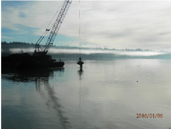
Description: RMC placement with crane and clamshell in SMA-2.
