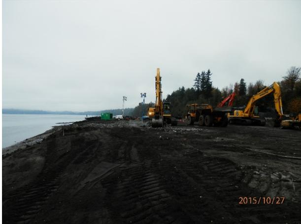
Description: Removal of concrete bulkhead structure at approx.. Station 5+00.
