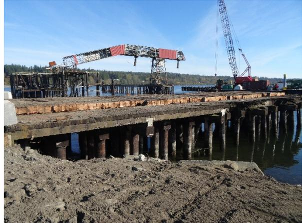
Description: Crane mats added to Pier 4 for offloading of creosote piles.
