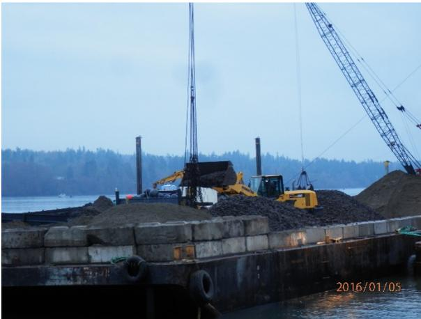
Description: Type 3 armor and habitat substrate material loaded on material barge for Type 3 cap placement in shallow subtidal areas.
