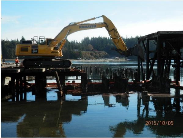
Description: Removing section of nearshore Alder Chip Mill Pier
