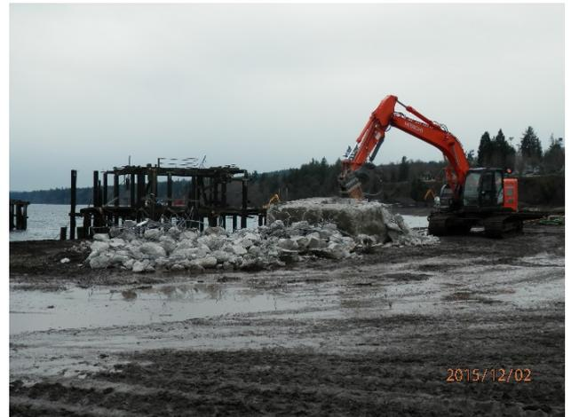
Description: Processing concrete from Alder chip pier demolition.
