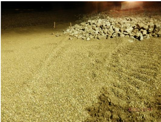
Description: Placement of Type 2 armor and filter capping material at 10+00.
