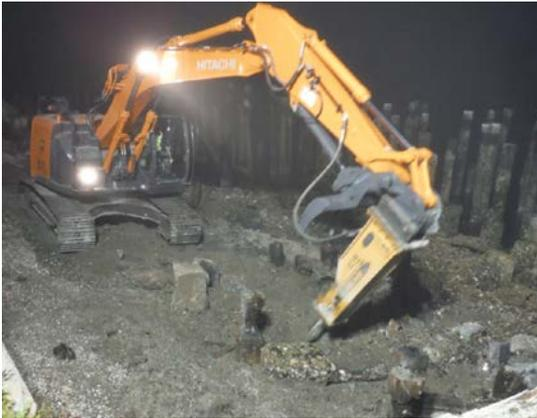
Description: Concrete sizing and removal from intertidal areas in the dry.
