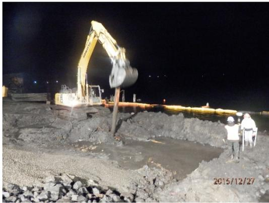
Description: Intertidal excavation and pile pulling in north SMA-2.
