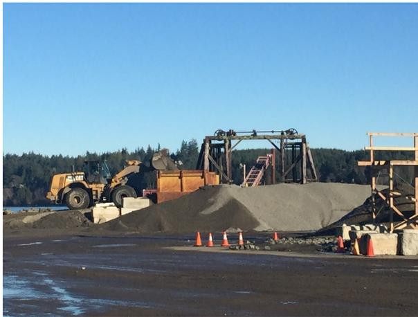
Description: Loading filter material onto a barge for intertidal capping with marine equipment below El. +0 MLLW.
