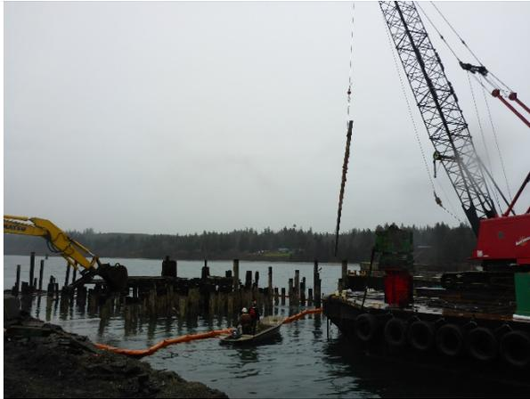
Description: Pile removal in Eastern Wharf with excavator from shoreline and crane from barge.
