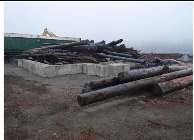
Description: Treated and untreated piles removed and ready for processing.
