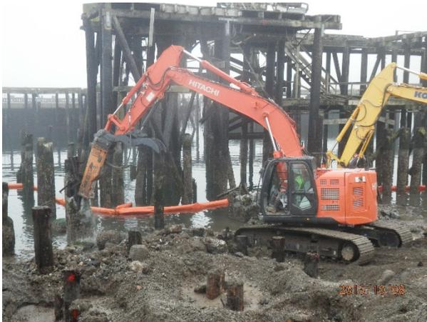
Description: Demolition of concrete pads on piles in intertidal area at Station 17+00
