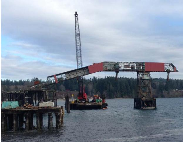
Description: Installation of demolition rigging on overhead conveyor.
