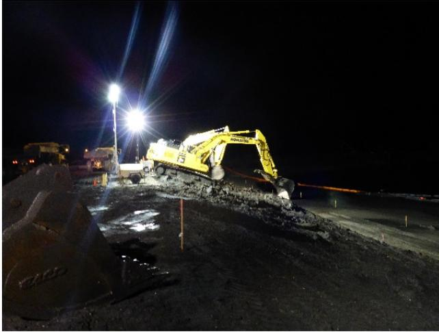
Description: Placement and grading of pea gravel filter material.
