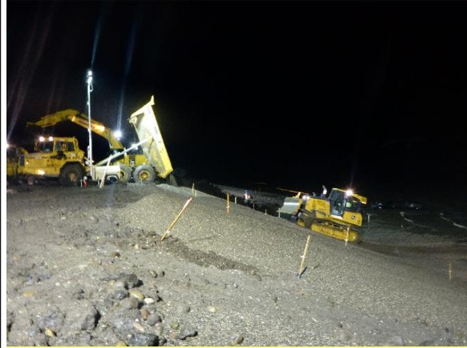
Description: Placement and spreading of intertidal cap filter material.
