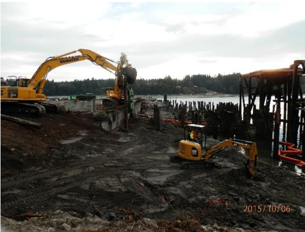
Description: Intertidal pile removal with excavator and excavator clearing and grading pile removal site.
