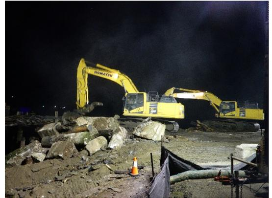
Description: Removal of concrete encased piles at Eastern Wharf.
