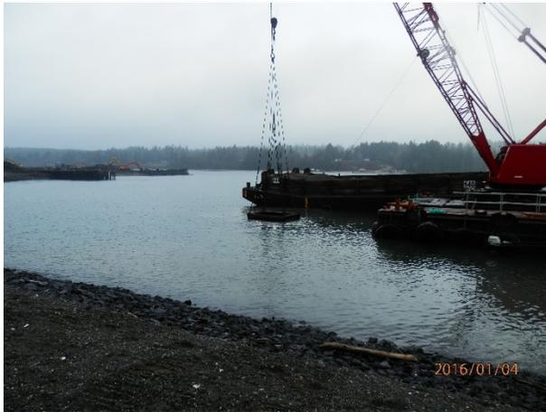
Description: Placement of shallow subtidal Type 3 cap filter material using Bombay box.
