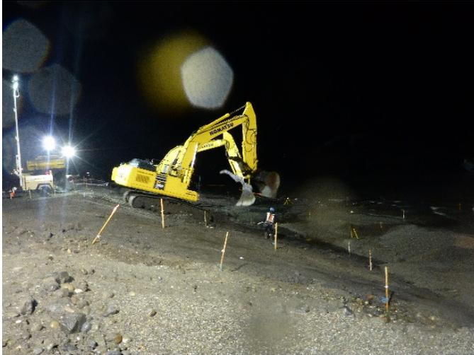
Description: SMA-2 intertidal excavation of 3H:1V slope on shoreline bank.
