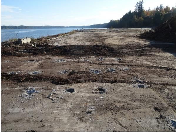
Description: Demolition of upland concrete slab within bank excavation footprint.
