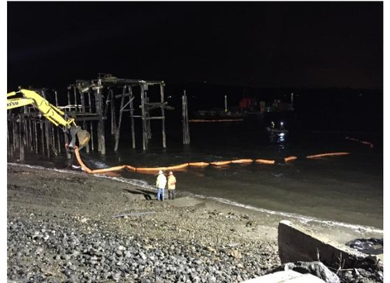
Description: Installation of boom around demolition work area.
