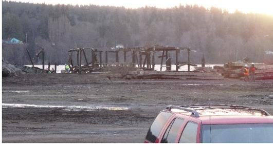
Description: Overhead conveyor immediately following demolition by rigging and pulling structure down.
