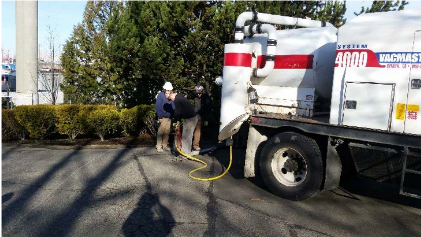
Air knifing B-03 looking to the north.
