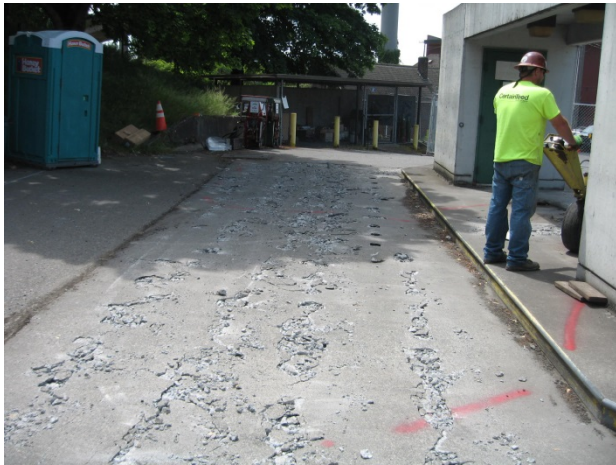
Pump Island and eastern extent of UST excavation
