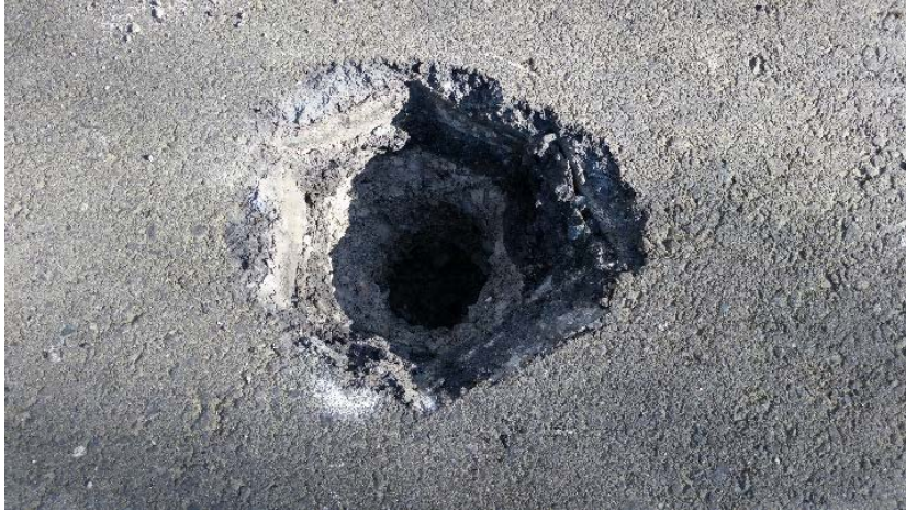
View of air knifed location prior to direct push drilling activities.
