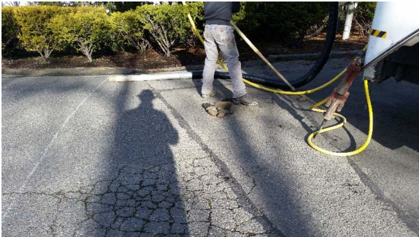
Air knifing B-03 looking to the north.
