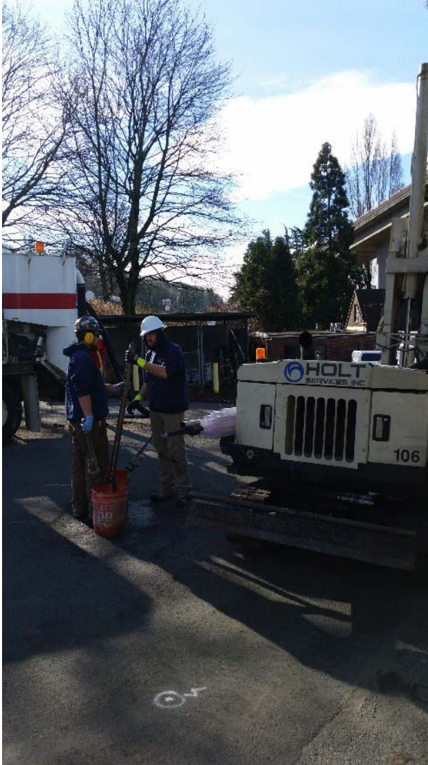
Decontamination of drill rods near B-02.
