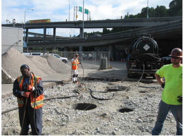
Marine Vacuum Inc. Pumping and Rinsing Tanks; Marine Chemist Inerting Tanks
