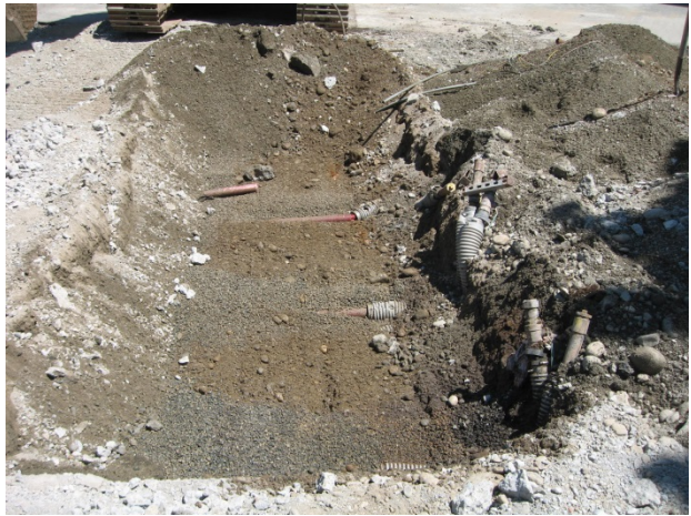
Piping system leading from island to tanks
