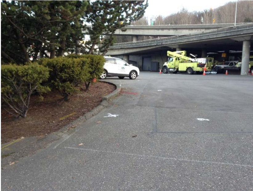
Utility locate, B-03 location in foreground, looking to the northeast.
