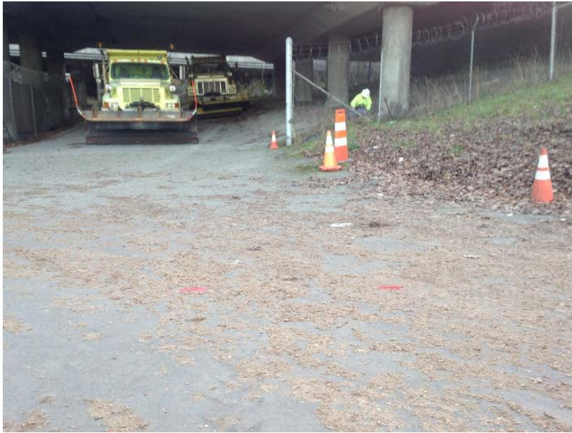
Utility locate, south end of the site, view of I-5 overpass and WADOT truck storage looking to the east.
