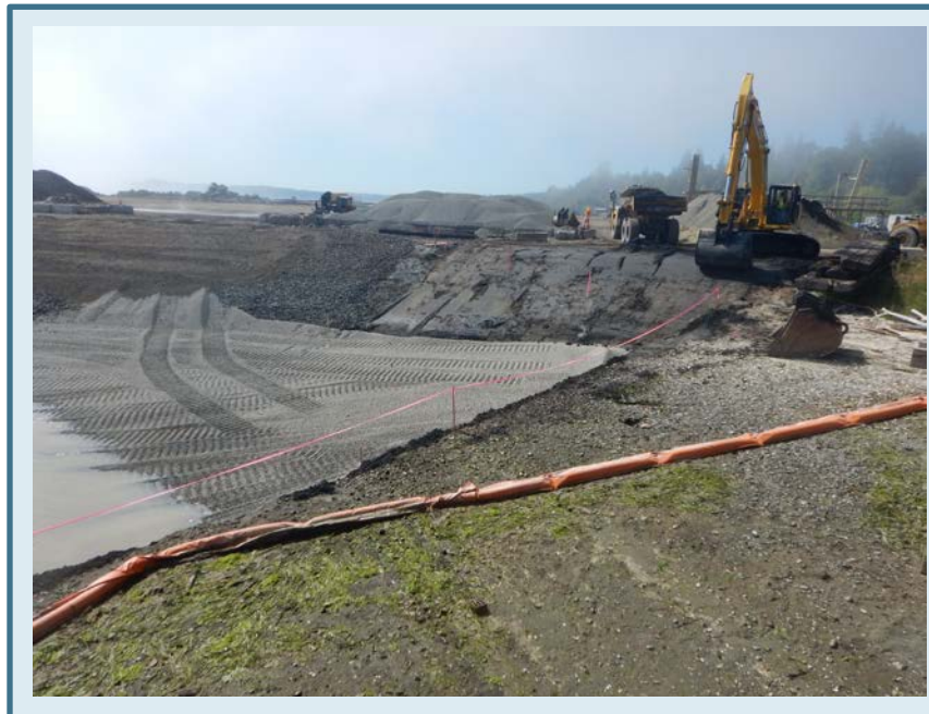
During Construction SMA-1 Shoreline
