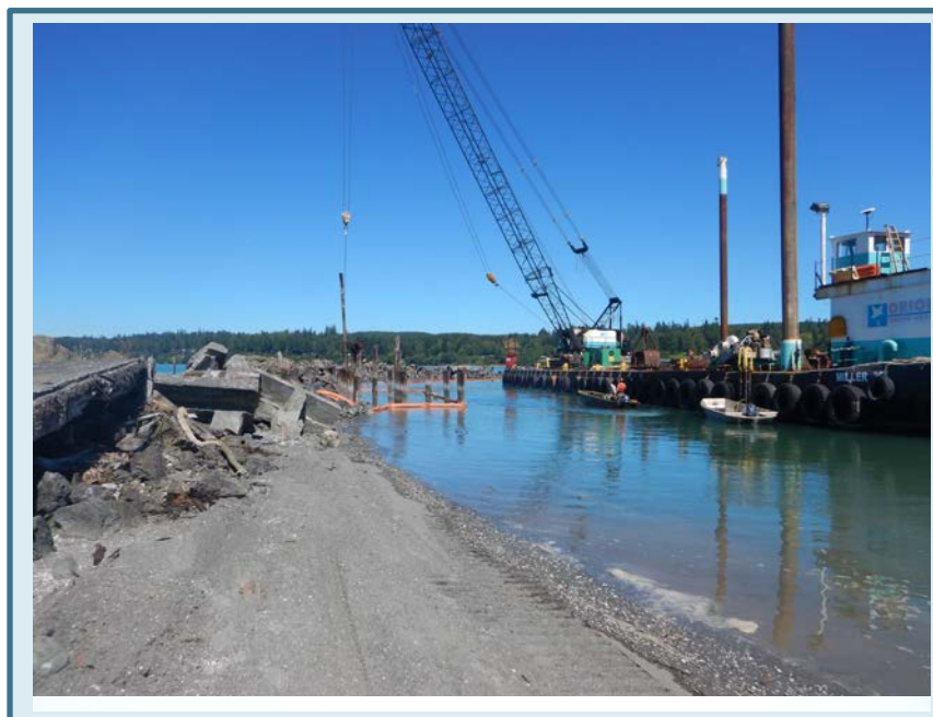
During Construction Jetty
