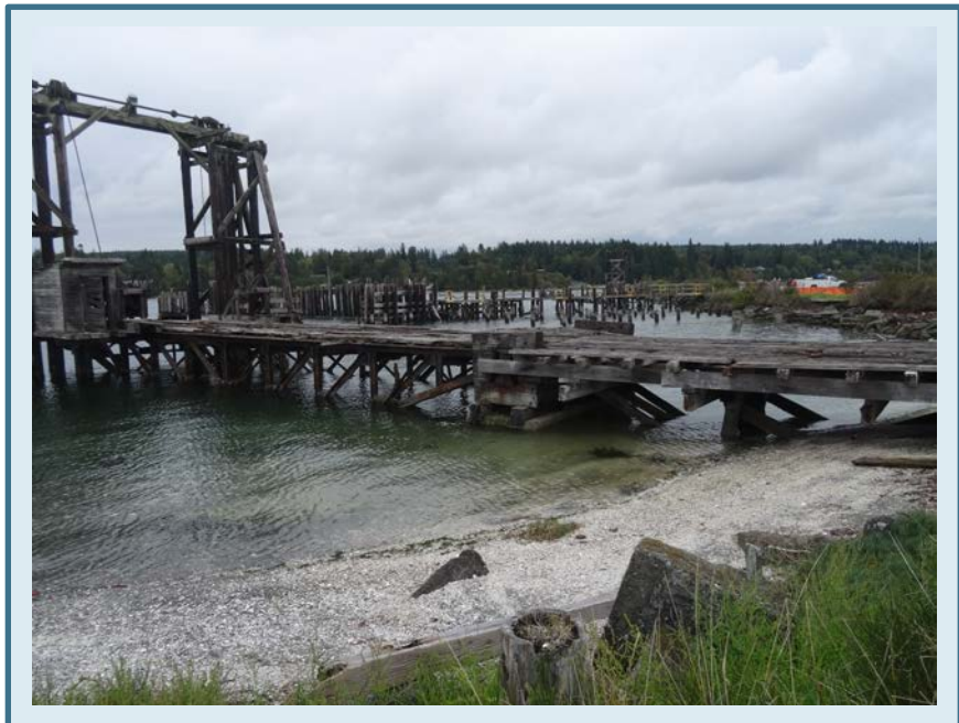
Pre-Construction SMA-1 Shoreline
