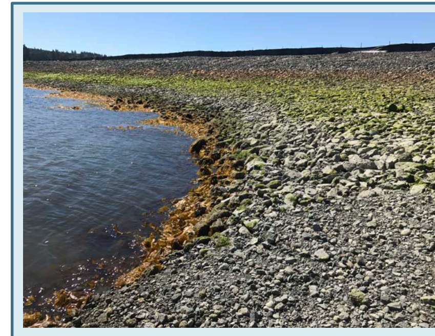
Post Construction SMA-1 Shoreline
