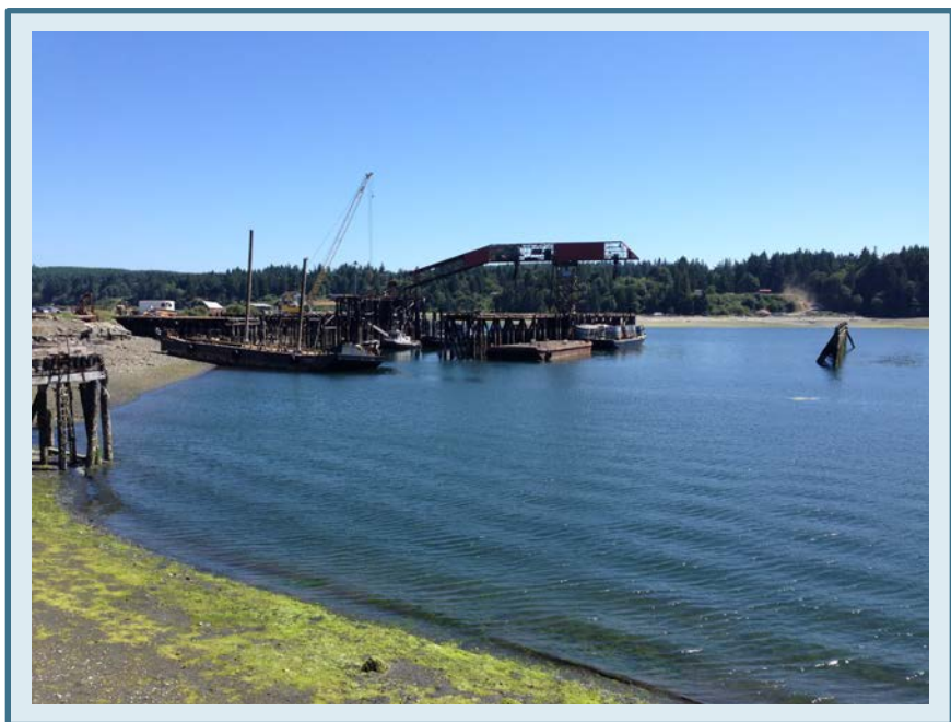
Pre-Construction SMA-2 Shoreline
