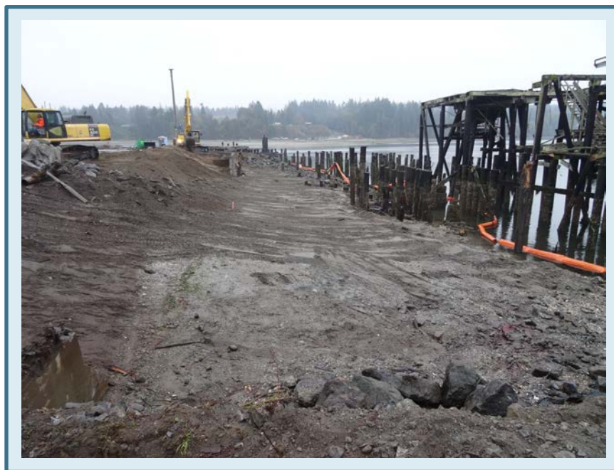
During Construction SMA-2 Shoreline
