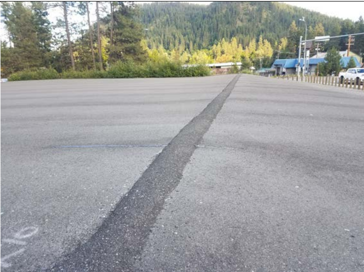
Photo 1: View looking south along western edge of cap, along slope break (post-crack fill).
