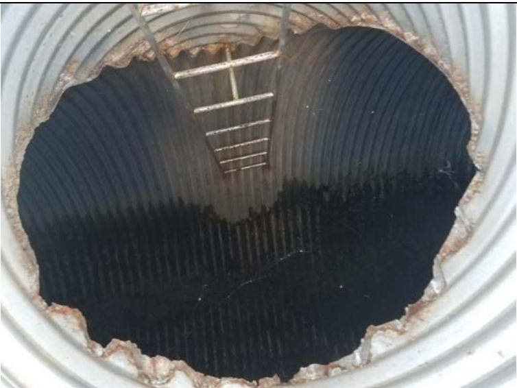
Photo 7: View inside vault.
