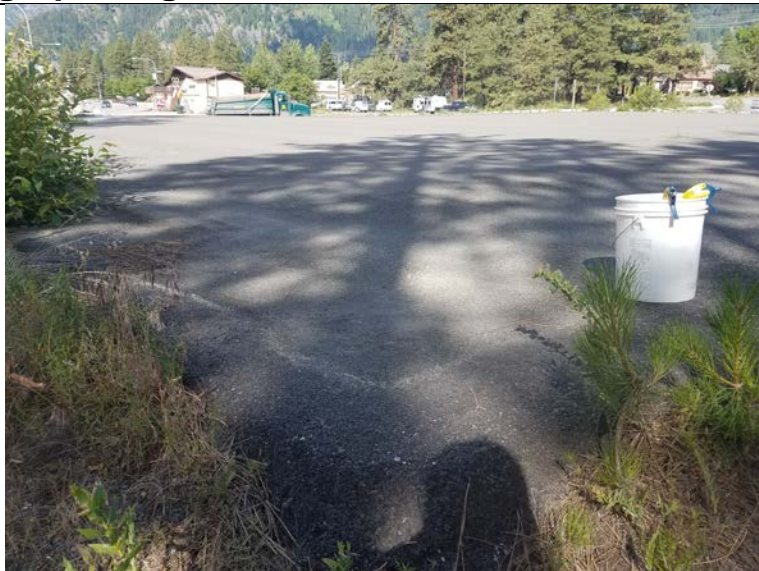
Photo 10: View looking northeast in northeast corner of cap (pre-crack fill).
