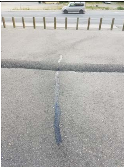
Photo 12: View looking east in towards slope in northeast corner of cap (post-crack fill).
