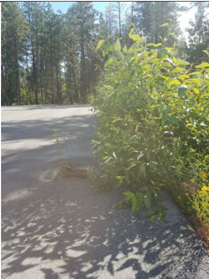
Photo 2: View looking east along southern edge of cap (post-crack fill).
