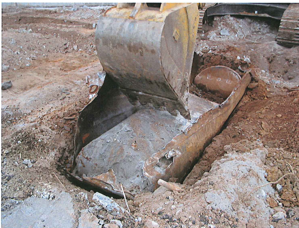
Photo #6: Removing contents of UST from former abandonment
