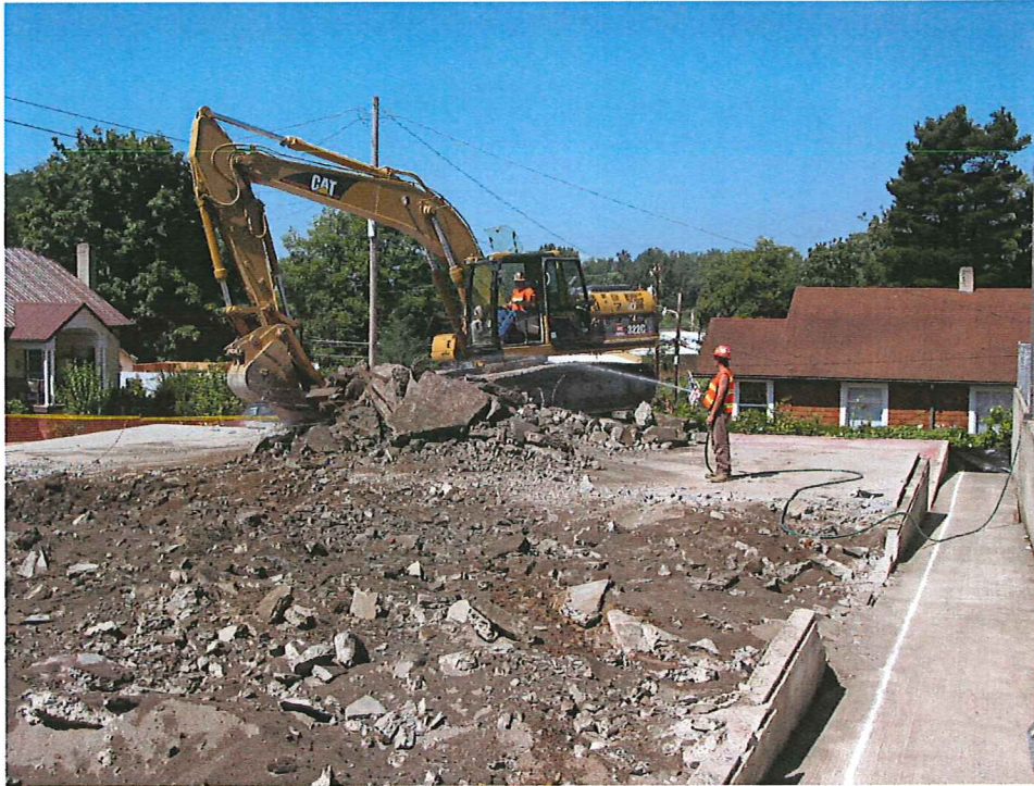
Photo #3: Slab demolition
