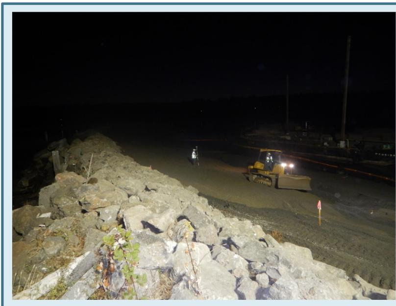
SMA-1 Jetty Area Intertidal Cap Filter Layer Placement
