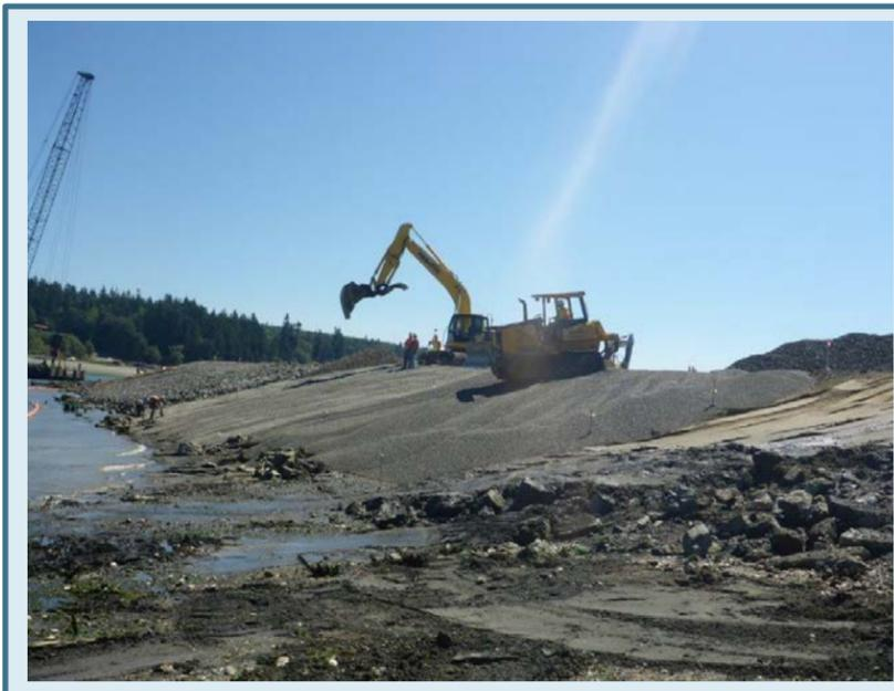
SMA-1 Intertidal Cap Filter Layer Placement
