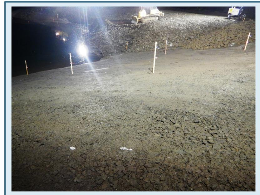
3" Minus Backfill Placement – Former Pier 4 Area Cap
