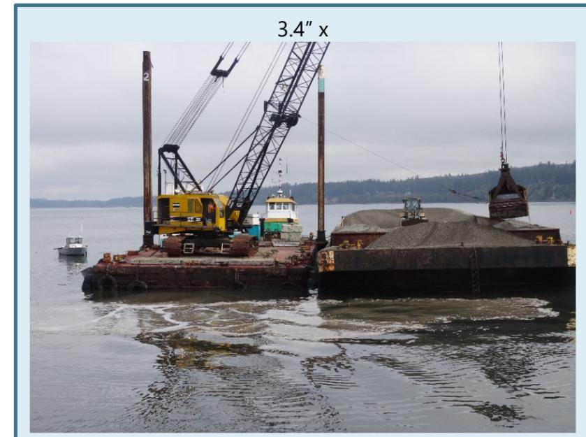
Subtidal Cap Placement in SMA-1 and Water Quality Monitoring
