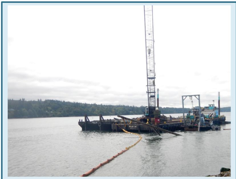
Diver-assisted Removal of Submerged Piling at the Eastern Wharf
