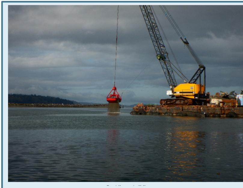
Subtidal Cap Filter Layer Placement in SMA-1
