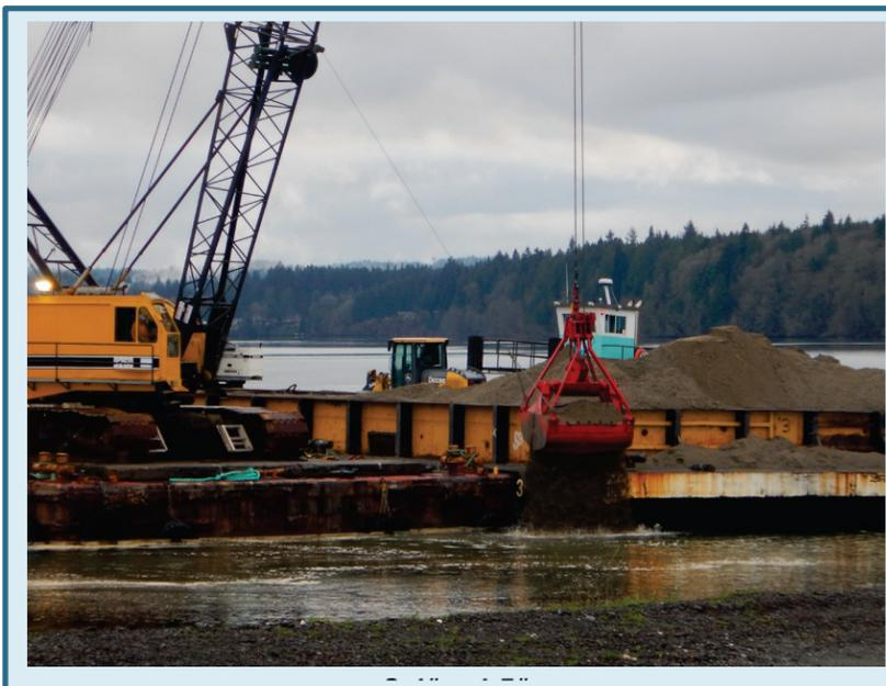
Post-dredging RMC Placement with 9260 Crane and Clamshell Bucket
