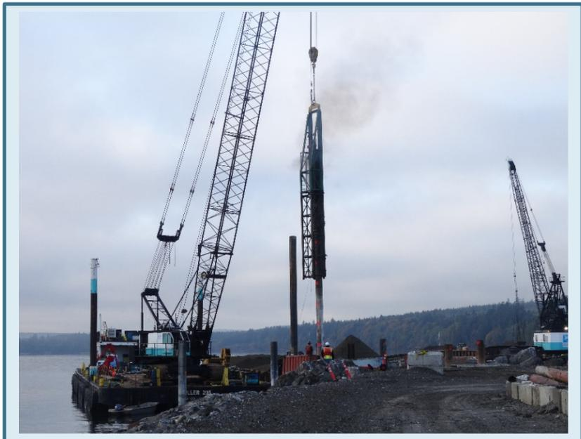
Installation of Temporary Pilings for Transload Extension
