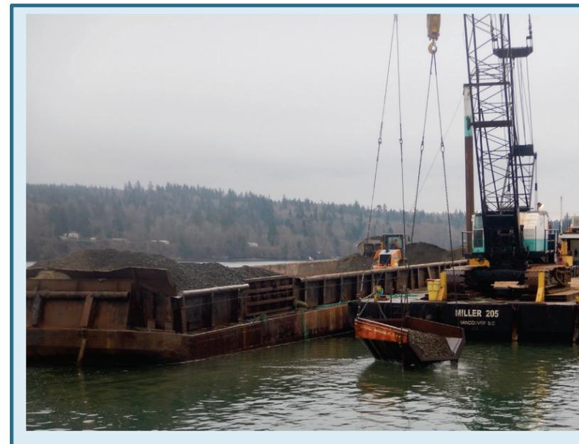
Placement of Angular Gravel Backfill Buttress Material in SMA-2 with 9299 Crane and Skip Box
