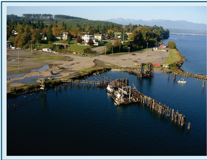
SMA-1 Conveyor/Pier and Log Transfer Dock (Pre-demolition)
