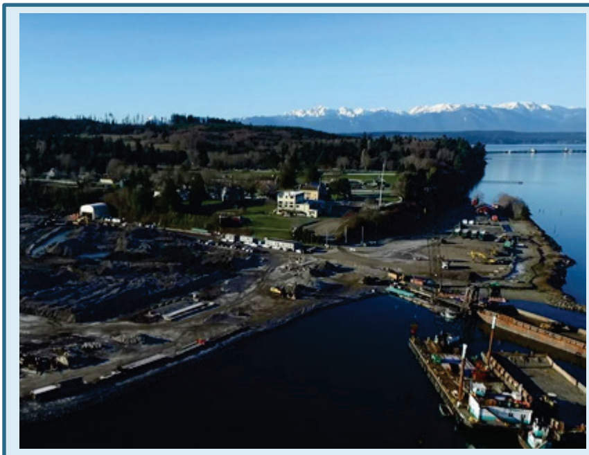
SMA-1 Conveyor/Pier (Post-demolition), Log Transfer Dock (Pre-demolition)
