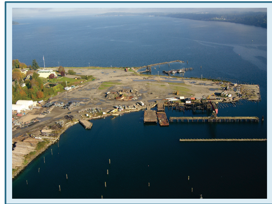
SMA-2 and Mill Site (Pre-construction)
