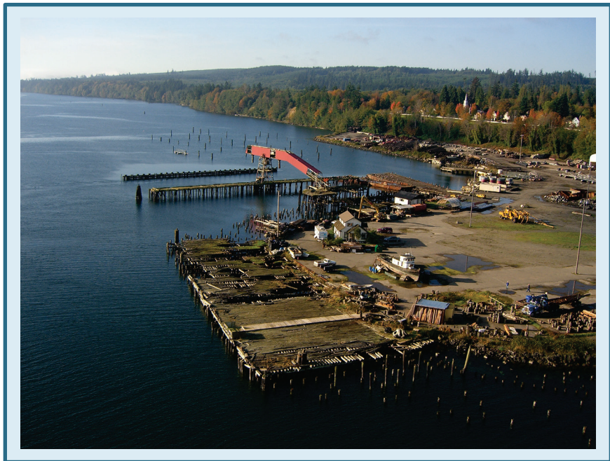
Eastern Wharf and Alder Chip Mill (Pre-demolition)
