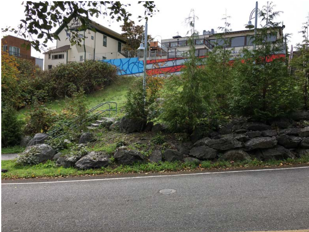
Photo 3: The cap includes pavement, soil, trees, and a rockery retaining wall.
