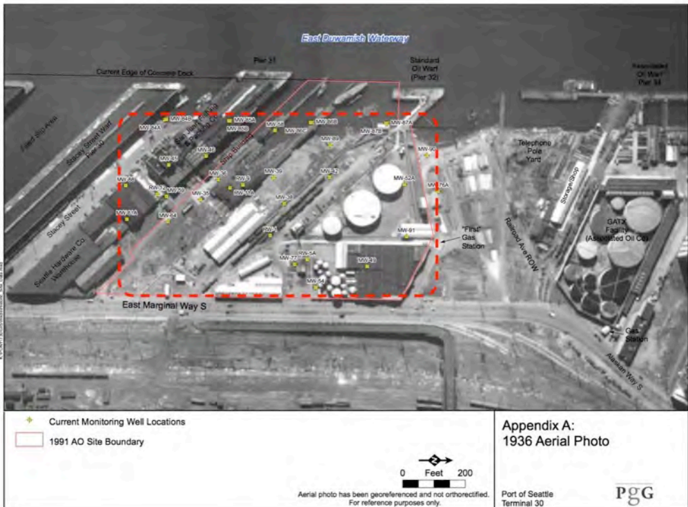
Figure 11. 1936 aerial photograph depicting the project location in red (Pacific Groundwater Group 2016: Appendix A).
