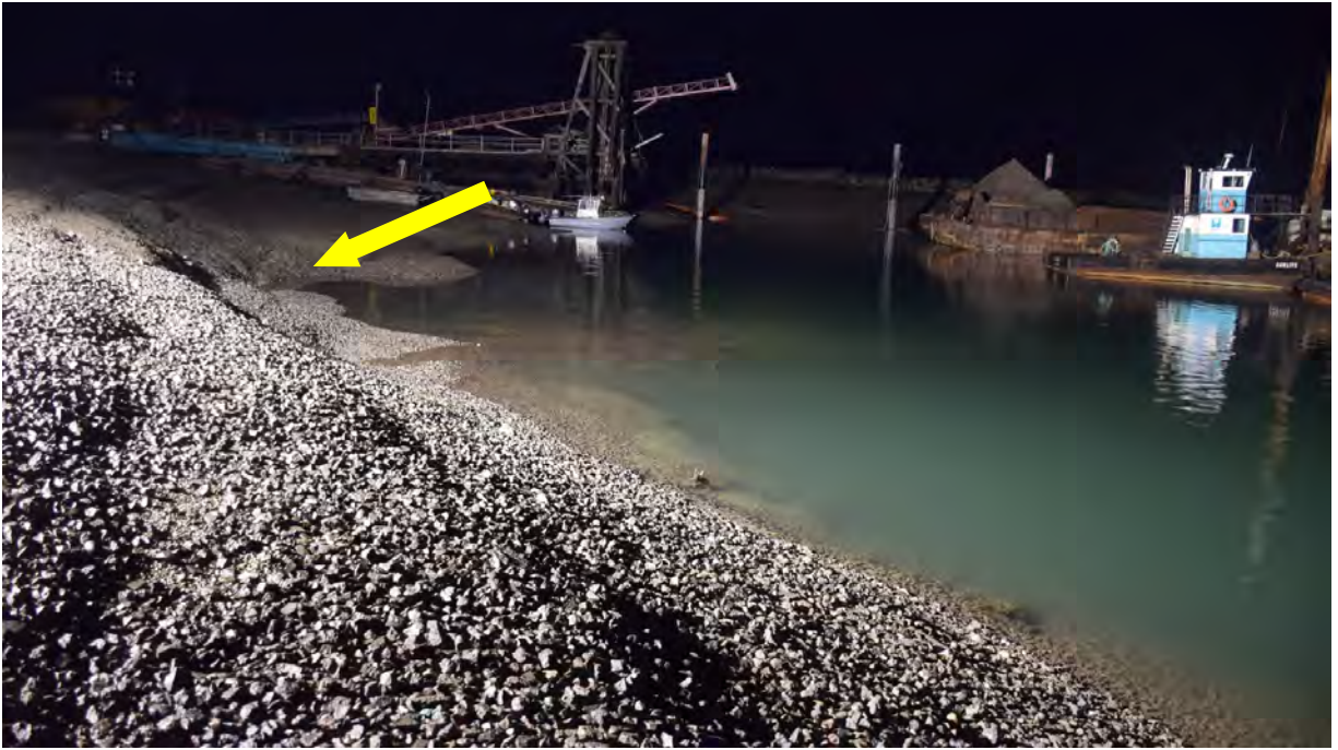
Photo 2 Potential Propwash Scour Area
