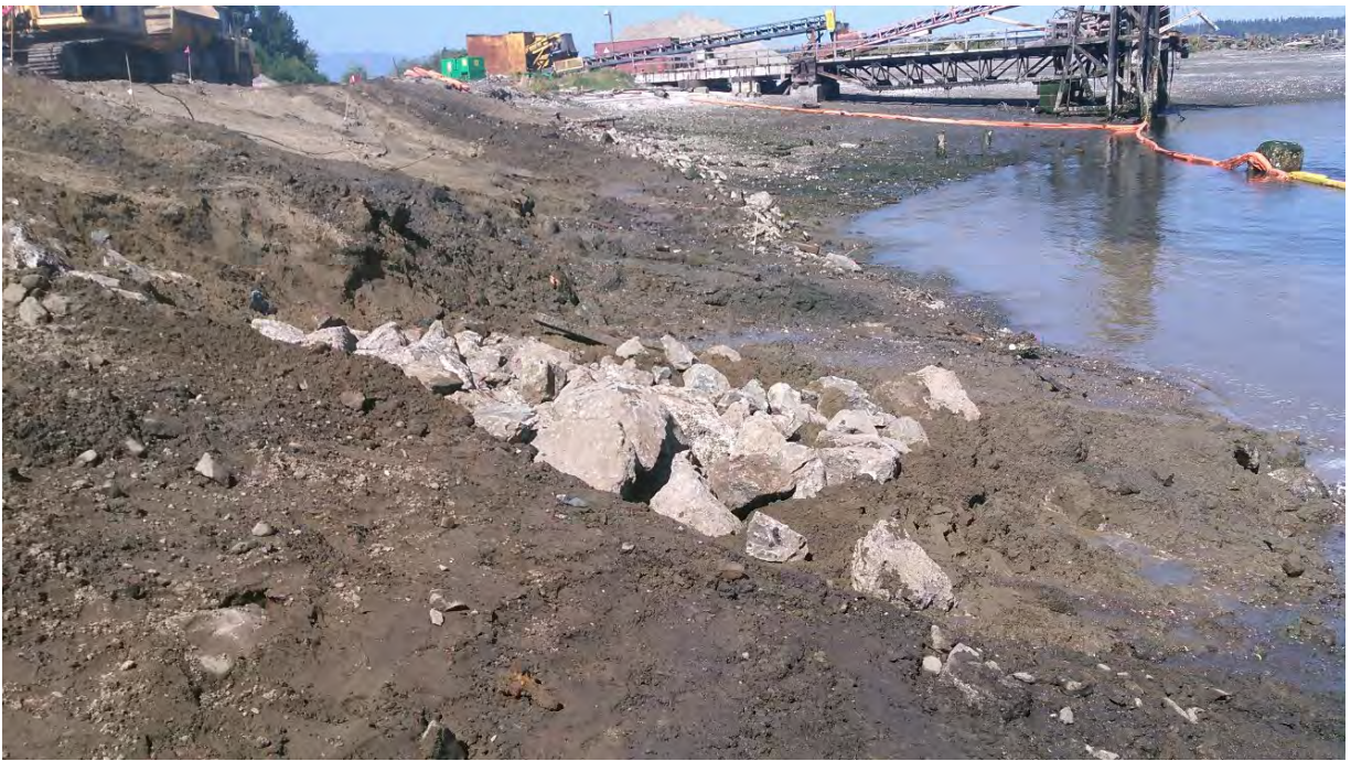
Photo 1 Seep Backfilled with Salvaged Armor Rock (August 2016)
