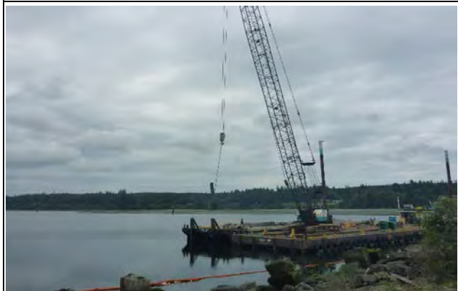
Comment: Pile removal SMA-1, pile with concrete base
