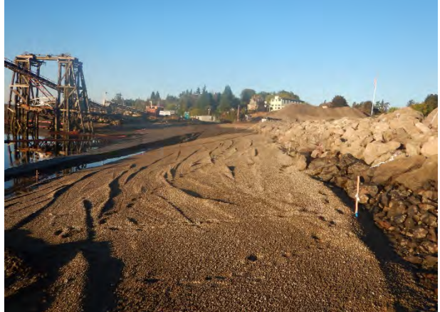
Comment: Placement of filter material along SMA-1 jetty intertidal cap area
