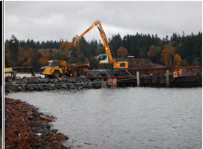
Comment: Offload setup with new piles and platform
