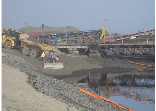
Comment: Placing habitat substrate over armor layer Sta. 25+00
