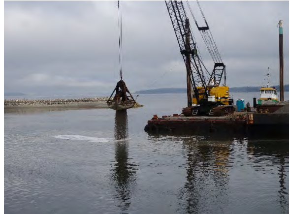
Comment: Placing subtidal cap in SMA-1
