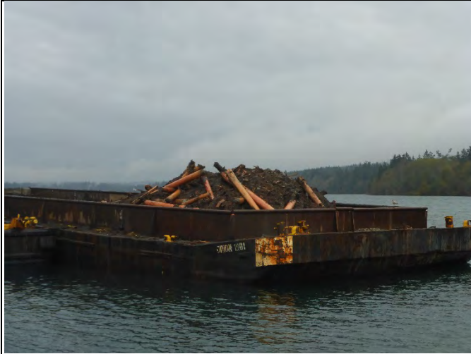
Comment: Dredge material barge and removed pilings in SMA-2
