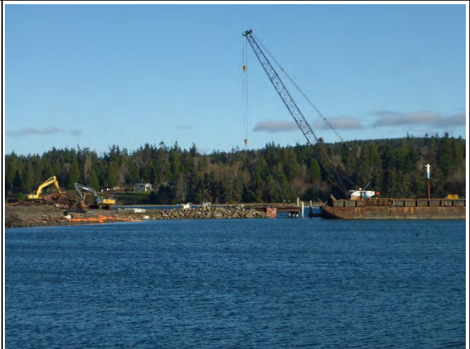
Comment: Transload facility demolition
