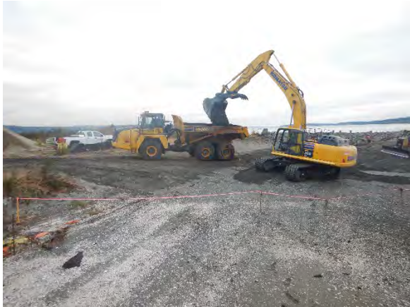
Comment: Intertidal excavation at nearshore end of SMA-1 jetty
