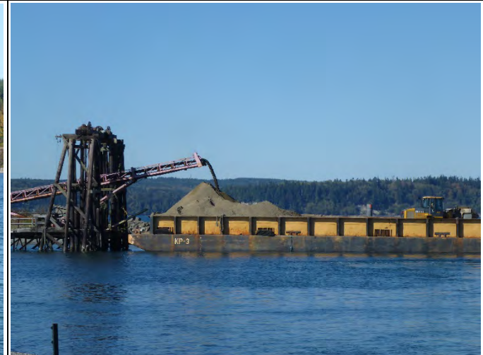
Comment: Loading barge with sand material for placement in SMA-2.
