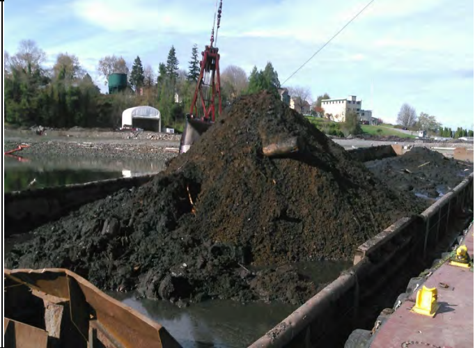
Comment: Wood waste material placed in dredge material barge
