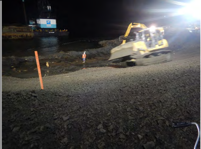
Comment: Placing initial lift of 3" minus backfill on 3h:1v slope
