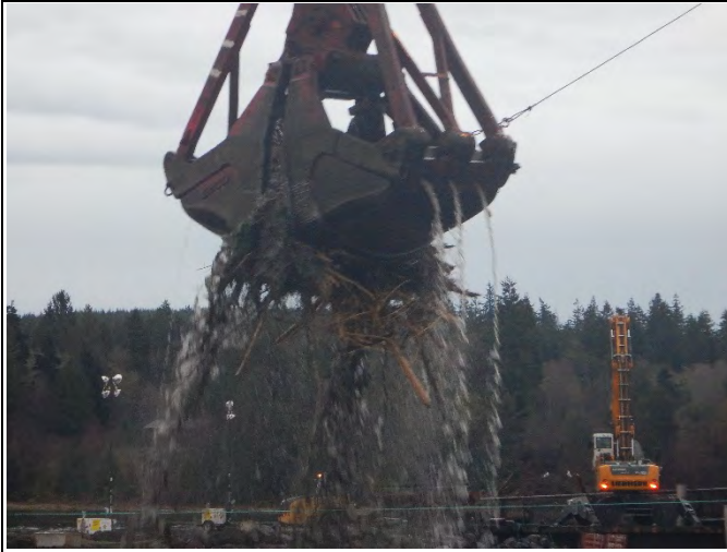
Comment: Wood waste material dredged from SMA-2
