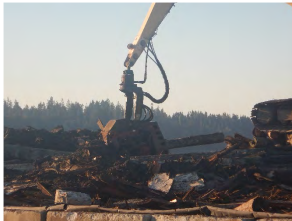
Comment: Processing creosote piles in the processing area
