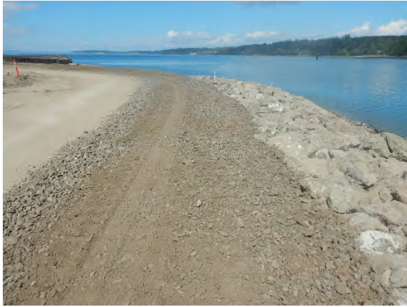
Comment: Perimeter containment berm at the Eastern Wharf
