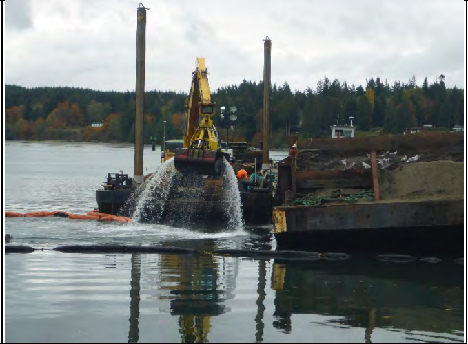
Comment: PC400 Dredging in SMA-1
