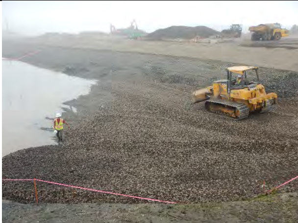
Comment: Placing armor layer Sta. 25+00
