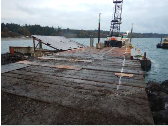
Comment: Completed offload facility platform
