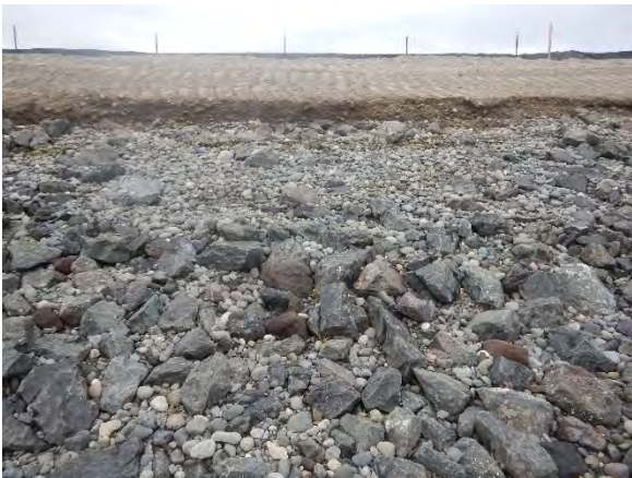
Comment: Habitat substrate on SMA-1 3:1 slope looking up from toe
