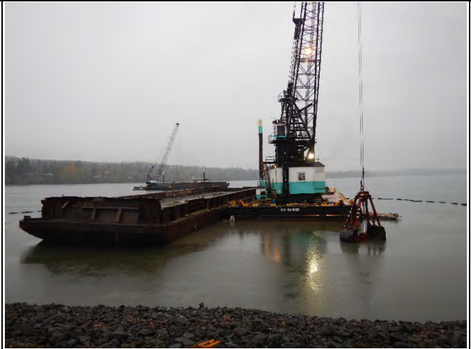
Comment: DB Rainier dredging in SMA-2
