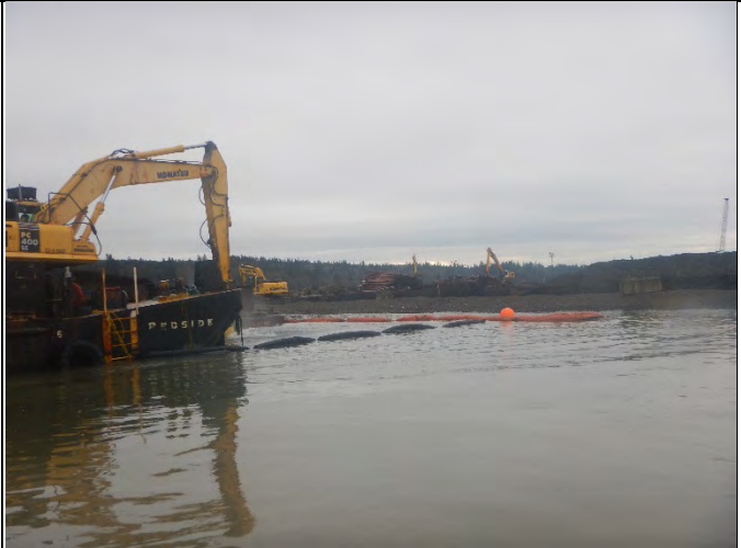
Comment: SMA-1 dredging
