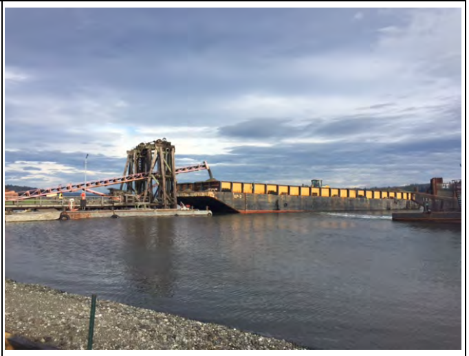
Comment: Loading sand for continued subtidal capping in SMA-2
