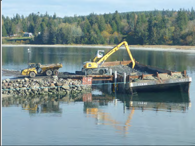
Comment: Dredge material offloading - ITB 166 material barge
