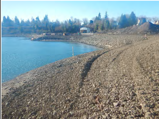
Comment: Pier 4 excavation/dredging area looking west
