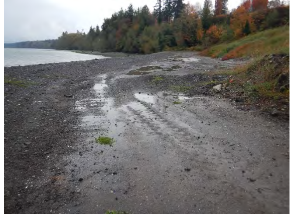
Comment: South end of SMA-2 perimeter berm
