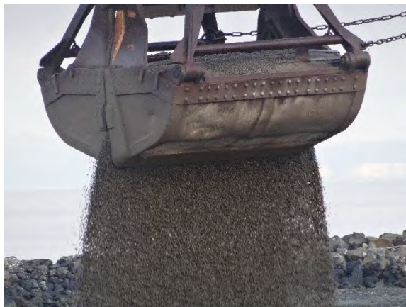
Comment: SMA-1 subtidal cap filter layer placement
