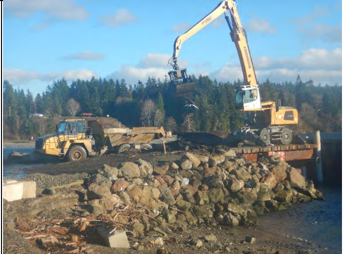
Comment: Offloading dredge material from SMA-2
