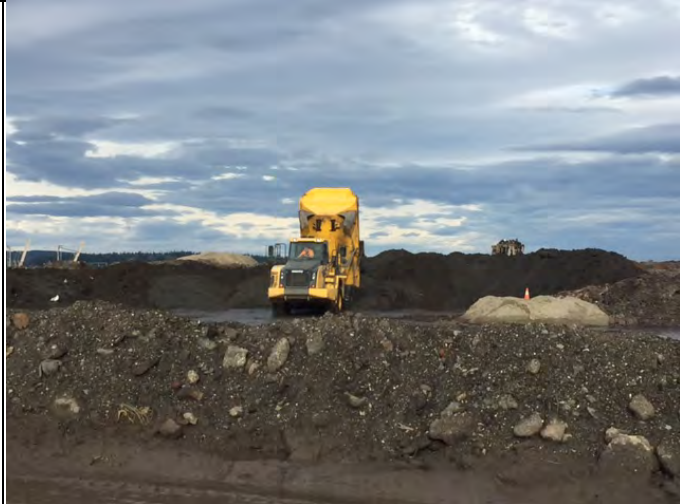
Comment: Stockpiling offloaded dredge material barge
