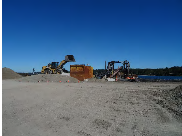
Comment: SMA-3 EMNR material loading to conveyor
