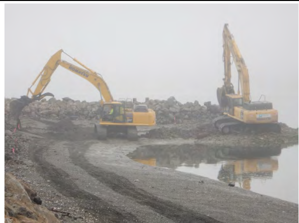
Comment: SMA-1 intertidal excavation at Sta. 34+69
