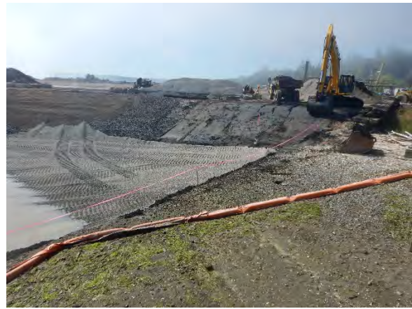
Comment: Filter material placed on lower area of excavation
