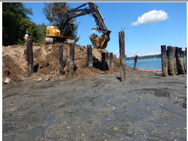
Comment: FLTF bulkhead removal, pilings remain.
