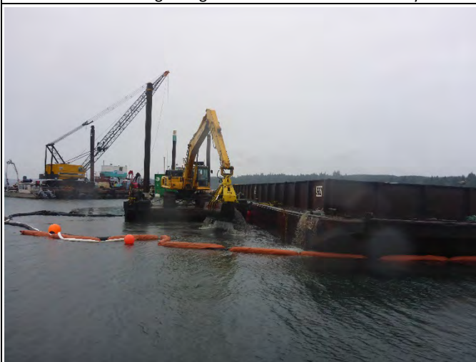
Comment: PC400 dredging in SMA-1
