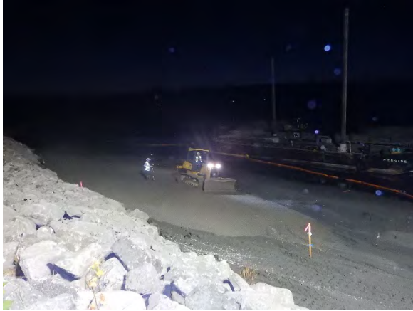
Comment: Filter layer placement along SMA-1 jetty
