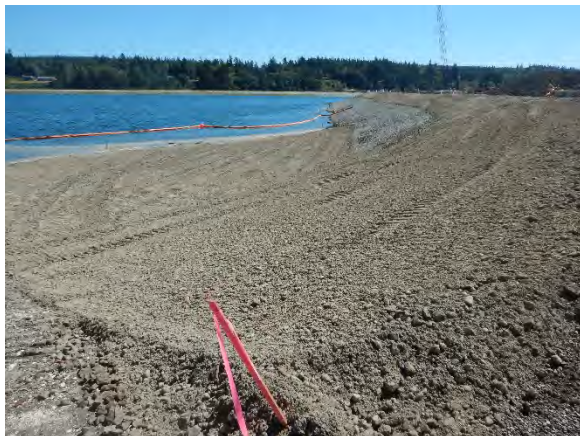
Comment: Completed habitat substrate area Sta. 25+00
