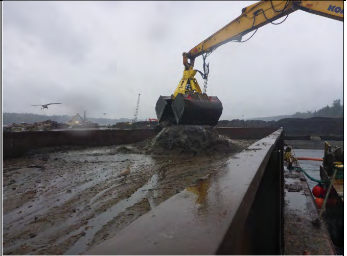
Comment: SMA-1 dredge material on barge
