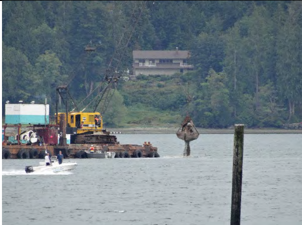
Comment: EMNR material placement in SMA-3
