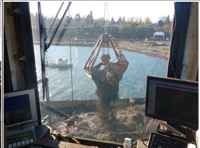
Comment: DB Rainier dredging in SMA-2
