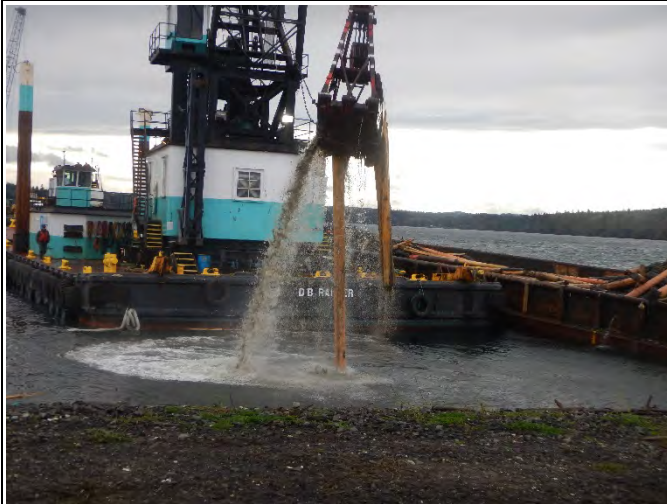
Comment: Piling removed during SMA-2 dredging
