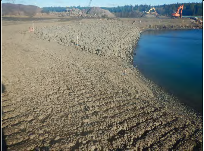
Comment: Pier 4 excavation/dredging area looking east
