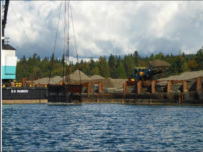
Comment: Sand placement in SMA-2 viewed from Water Quality Boat
