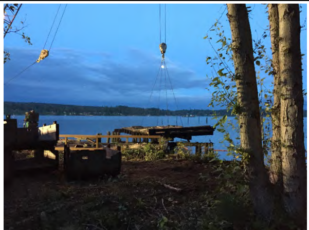
Comment: Removing decking from FLTF pier with barge-mounted crane
