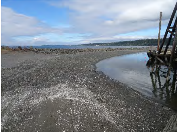
Comment: Completed intertidal excavation and capping at SMA-1 jetty
