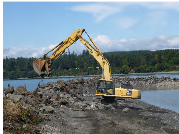
Comment: Concrete removal from SMA-1 jetty
