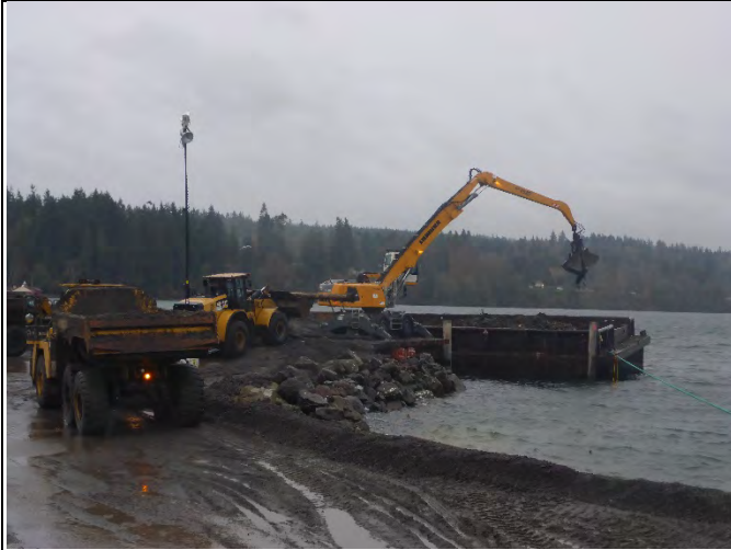
Comment: Offloading dredge material at Transload Facility
