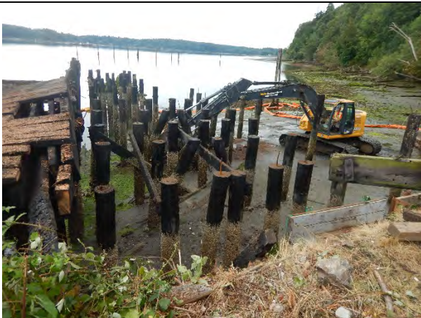
Comment: FLTF pier demolition progress
