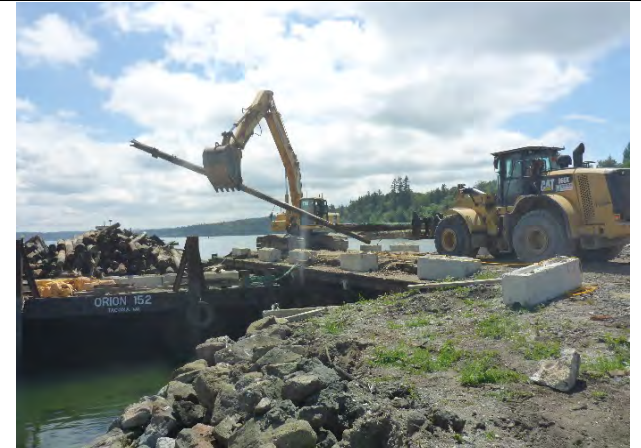
Comment: Pile offloading at Pier 4
