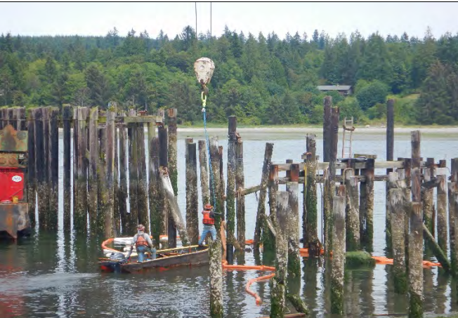
Comment: Removing partially extracted pilings with choker chain
