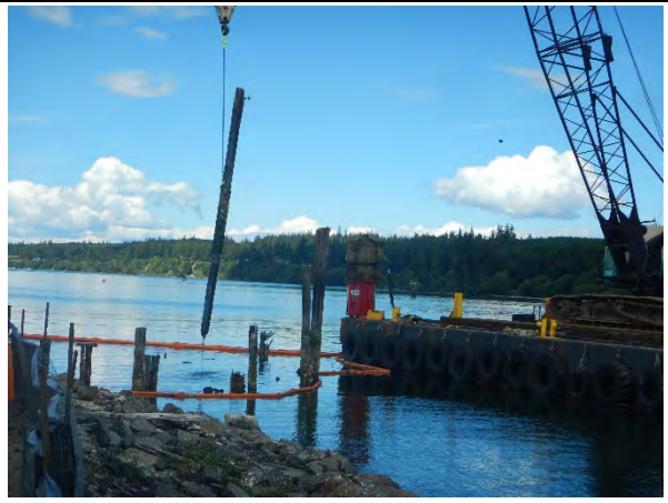
Comment: Pile removal north of Eastern Wharf
