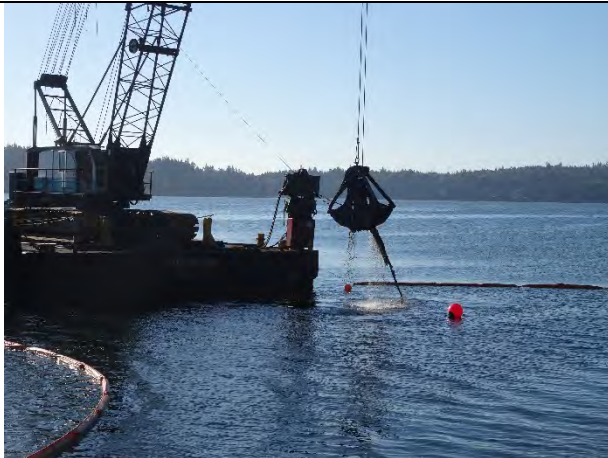
Comment: Removing derelict vessel at the FLTF
