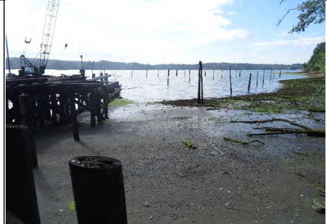
Comment: Pile removal in SMA-5 at the FLTF
