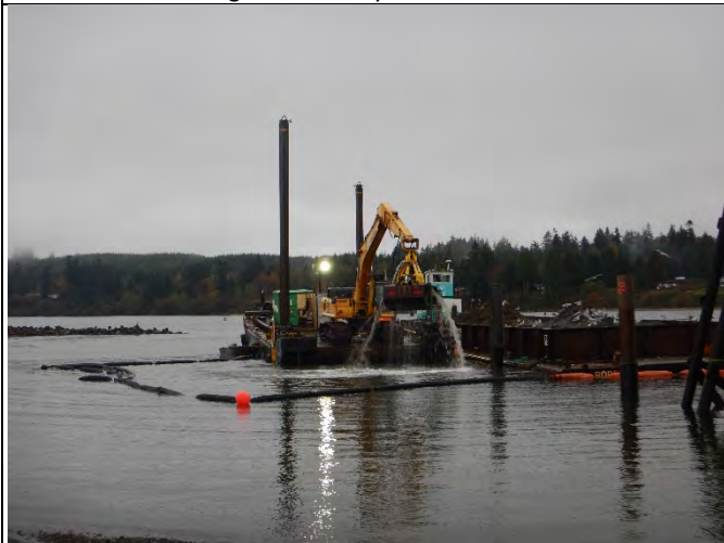
Comment: Dredging with the PC400 in SMA-1
