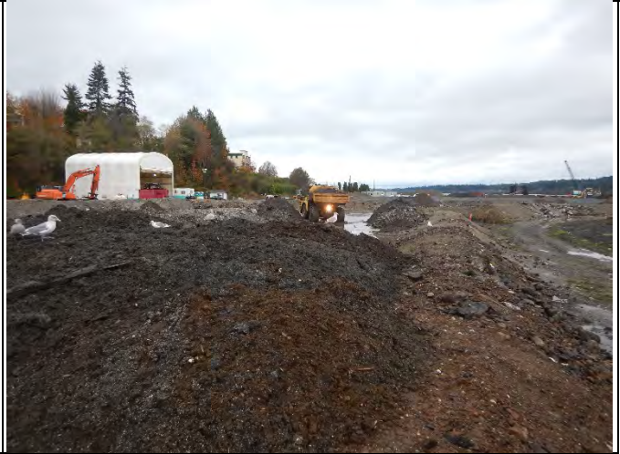
Comment: Dredge sediment offloaded and placed in cell #5
