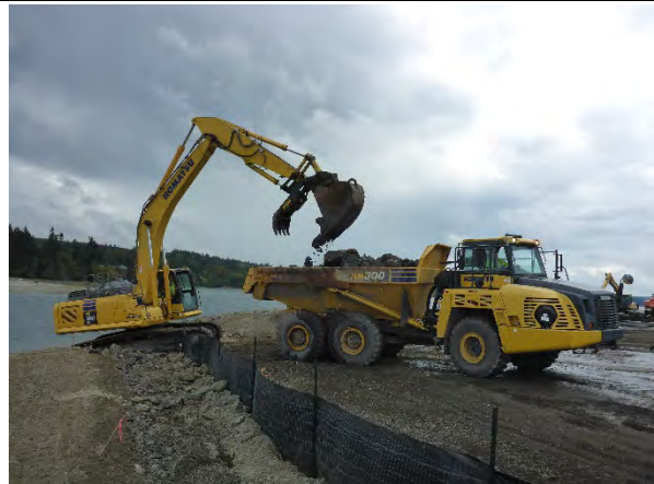
Comment: Intertidal excavation at southern end of SMA-1 jetty
