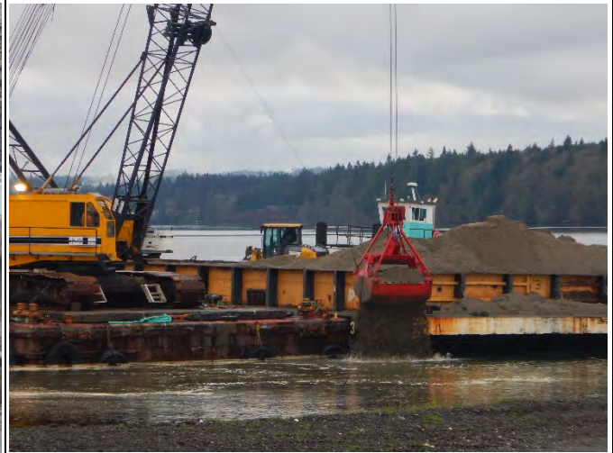
Comment: RMC placement in SMA-2
