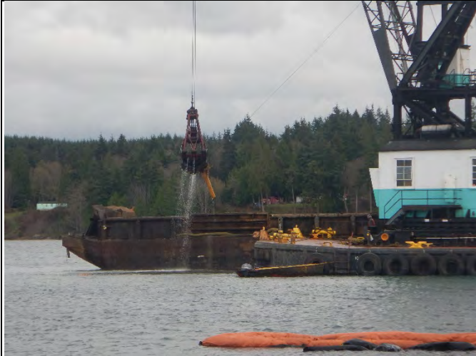
Comment: SMA-1 pile removal using the DB Rainier
