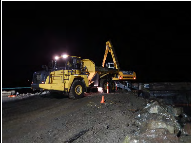
Comment: Offloading dredge spoil barge
