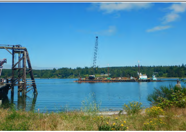
Comment: Pile removal at Dolphin offshore of Convey/Pier
