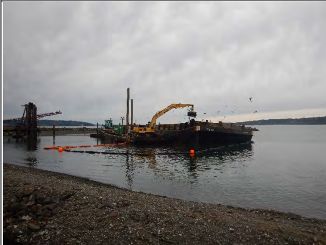
Comment: Dredging in SMA-1, filling the ITB 166
