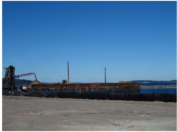
Comment: SMA-3 EMNR material barge loading
