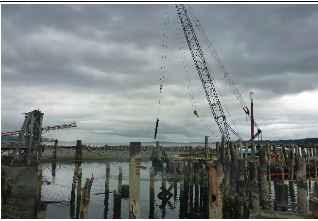
Comment: Piling removal near floating dock area (floating dock removed)
