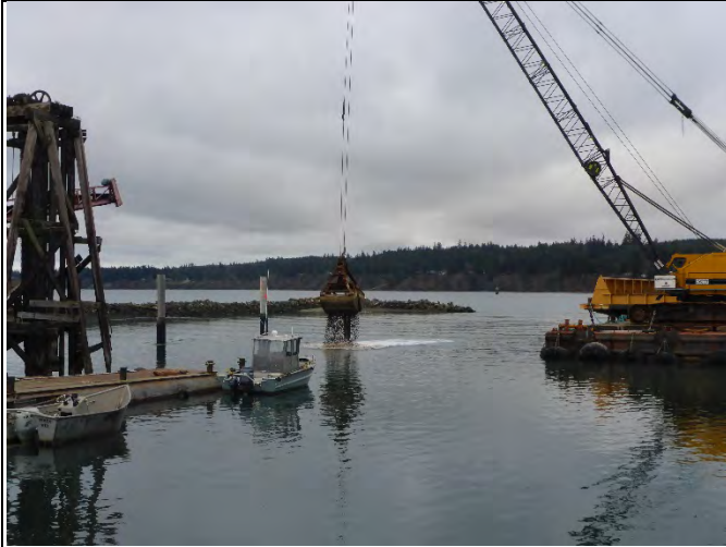
Comment: Placing SMA-1 subtidal cap – armor layer
