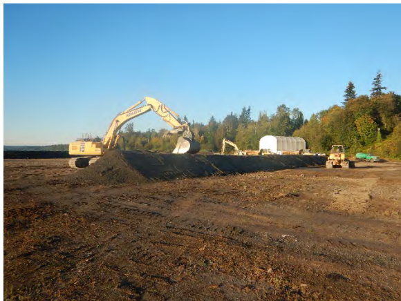
Comment: Building containment berms
