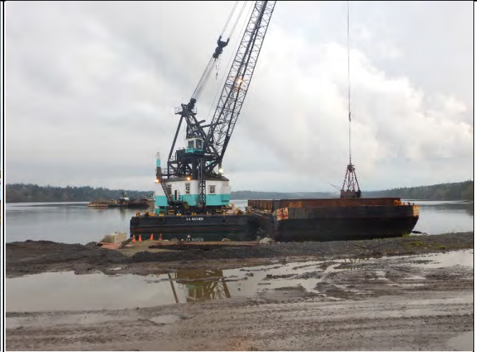
Comment: SMA-2 dredging
