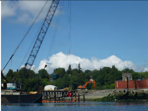
Comment: Removing piles with vibratory hammer at Station 17+00 in SMA-2
