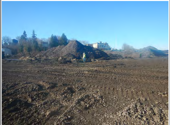
Comment: Stockpiles stacked higher to make room for additional dredge material
