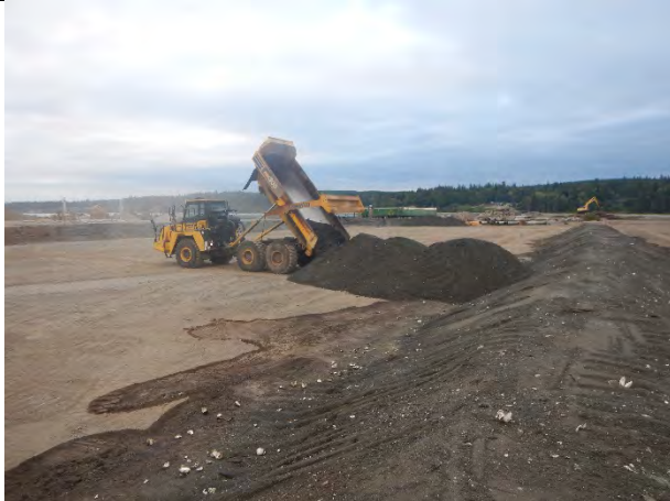
Comment: Placing intertidal excavation material for containment berms
