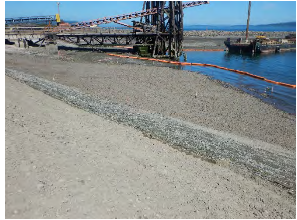
Comment: Completed armor layer Sta. 25+00 to 27+00
