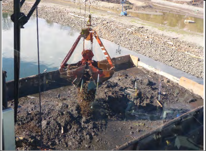
Comment: DB Rainier filling material barge – wood waste
