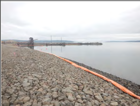
Comment: Completed portion of SMA-1 intertidal cap
