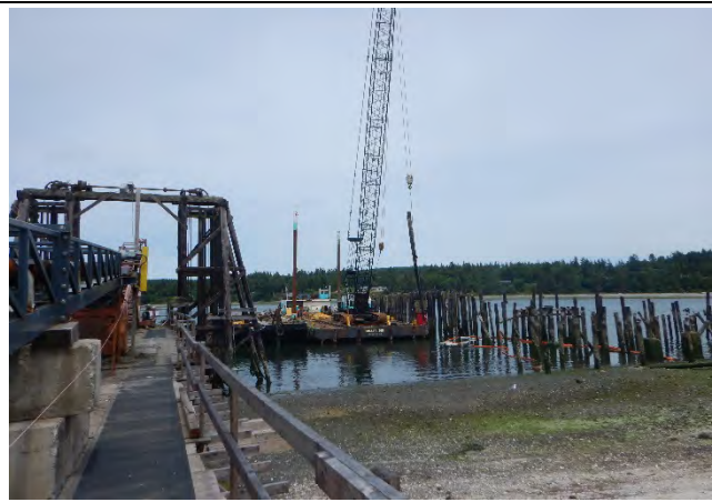
Comment: Piling removal near material loading conveyor
