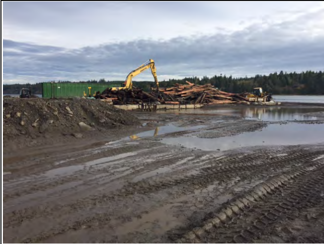
Comment: Pilings in processing area
