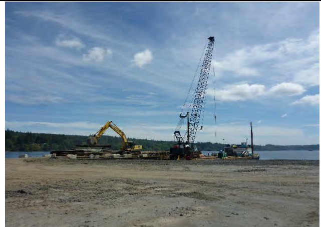
Comment: Offloading 152 material barge to upland containment and processing area
