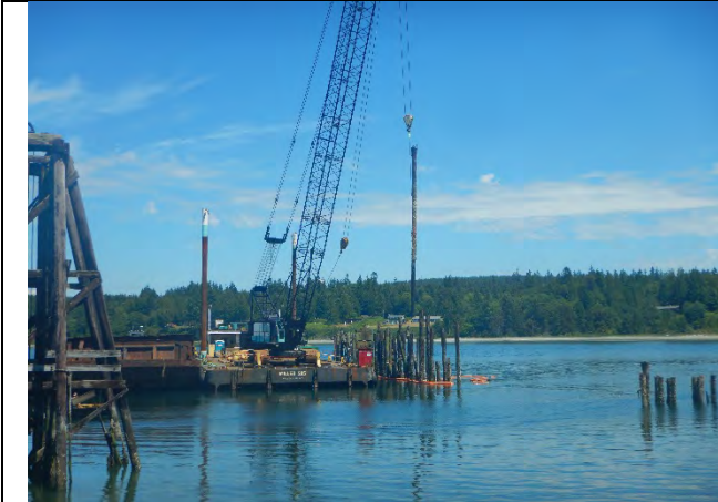
Comment: SMA-1 pile removal
