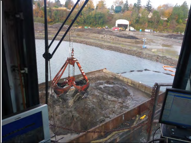
Comment: Dredge material in SMA-2 viewed from crane
