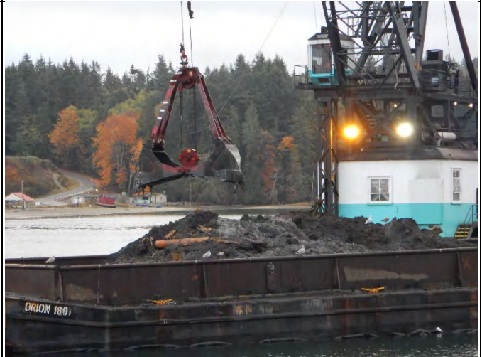
Comment: DB Rainier filling 1801 material barge
