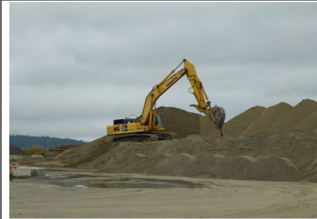
Comment: Stockpiled sand
