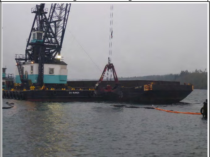
Comment: DB Rainier dredging in SMA-2
