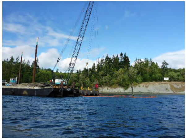
Comment: SMA-5 pile removal
