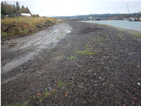
Comment: SMA-2 perimeter berm looking north
