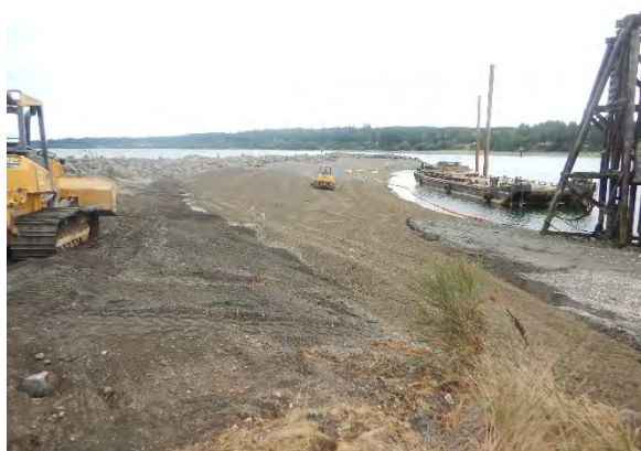
Comment: Habitat substrate placement at nearshore end of SMA-1 jetty
