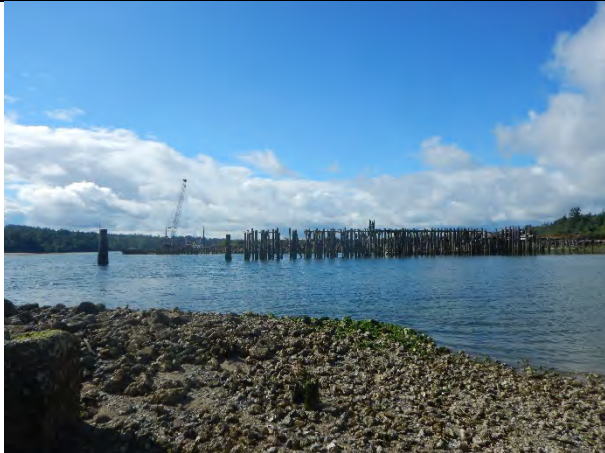
Comment: Season 2 pile removal starting in south end of SMA-1
