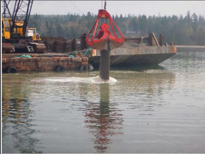
Comment: Placing filter layer for SMA-1 subtidal cap
