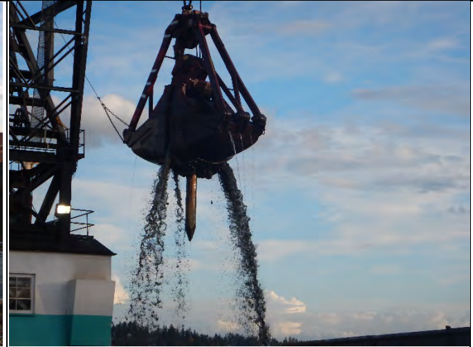
Comment: Numerous piles removed during dredging in SMA-2
