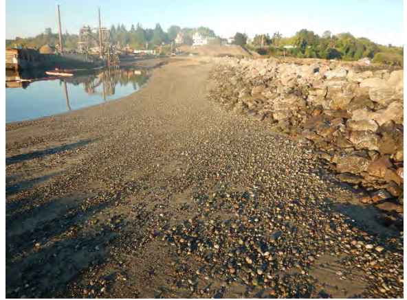
Comment: Completed intertidal cap along the SMA-1 jetty
