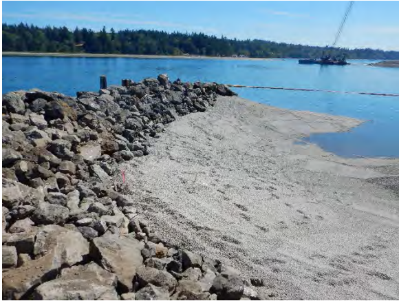
Comment: Filter layer placement at end of SMA-1 jetty
