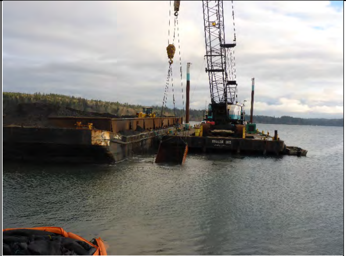
Comment: Placing 3" minus backfill in SMA-2
