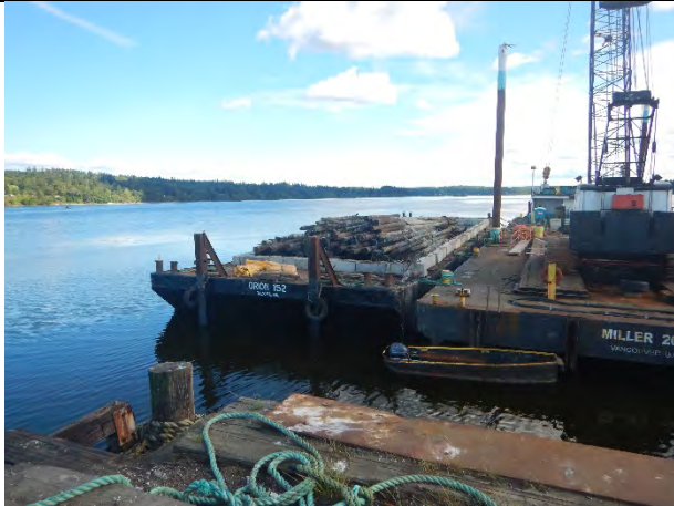
Comment: Piling staged on the 152 material barge
