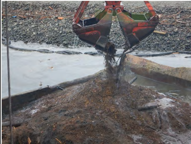
Comment: Wood waste material dredged in SMA-2
