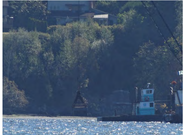
Comment: EMNR material placement in SMA-3 with 4 CY re-handling bucket
