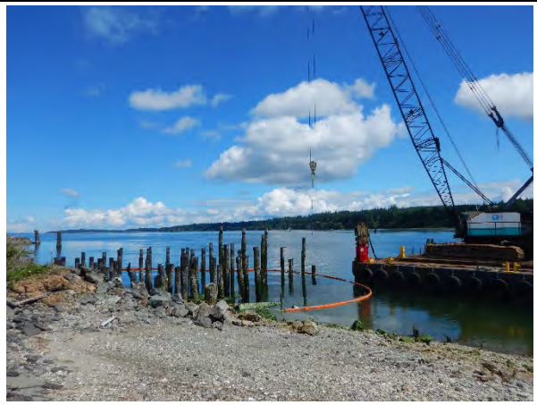
Comment: Pile removal at Sta. 21+00
