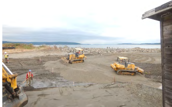
Comment: Filter layer placement at nearshore end of SMA-1 jetty
