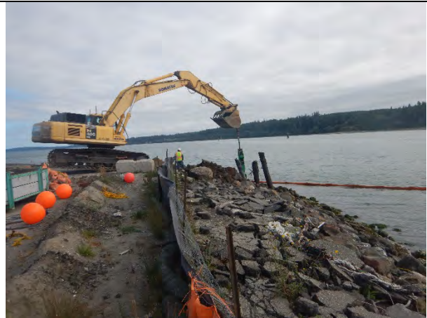
Comment: Pulling intertidal pilings from upper portion of Eastern Wharf bank
