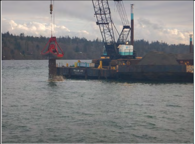
Comment: Placing EMNR in SMA-2
