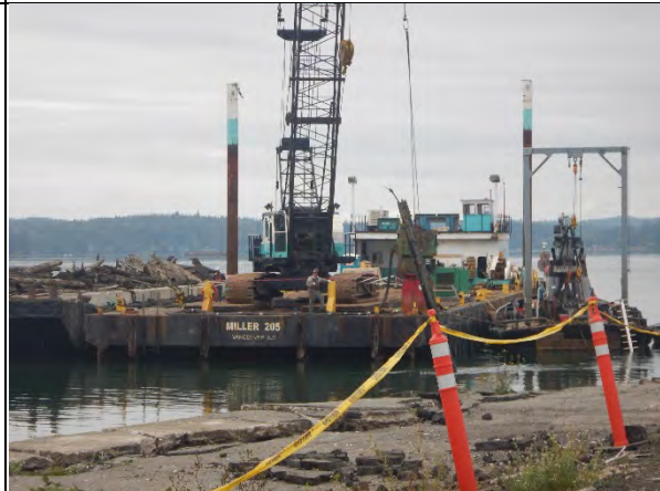
Comment: Diver assisted pile removal
