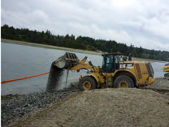
Comment: Intertidal capping southern at end of SMA-1
