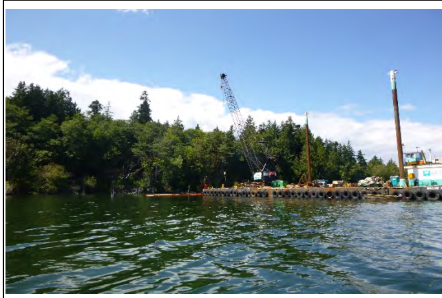
Comment: Pile removal in SMA-5 north of the FLTF
