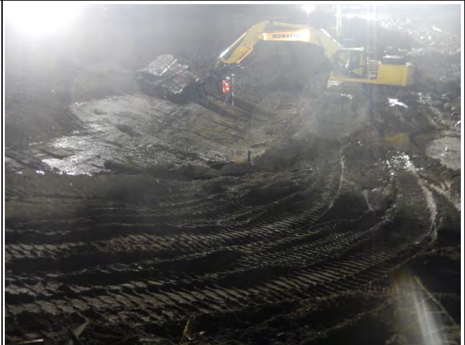
Comment: Upland excavation in SMA-2 bank adjacent to former Pier 4 area.
