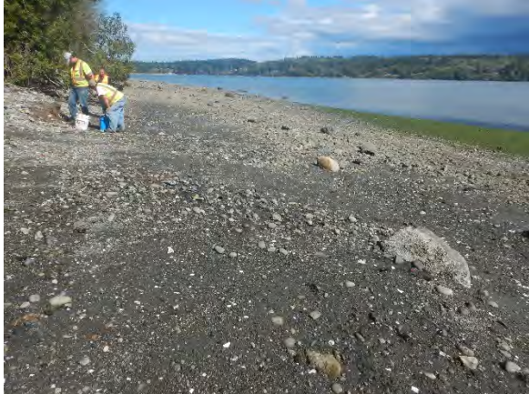
Comment: Additional cleanup of asphalt and brick at Area 4
