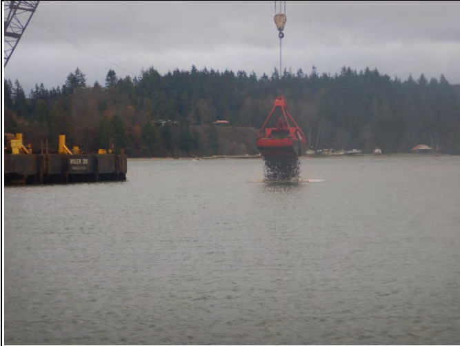
Comment: Placing SMA-1 subtidal cap
