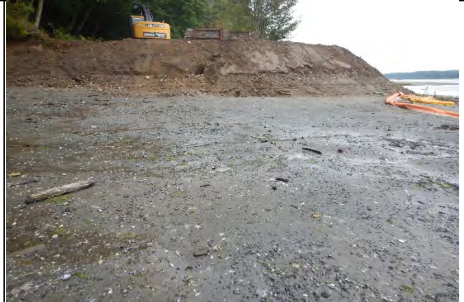
Comment: FLTF area after bulkhead and piling removal
