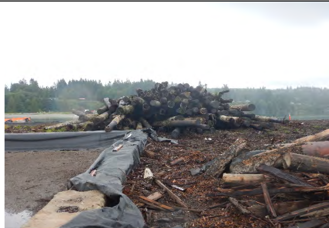
Comment: Piling stockpiled in containment/processing area
