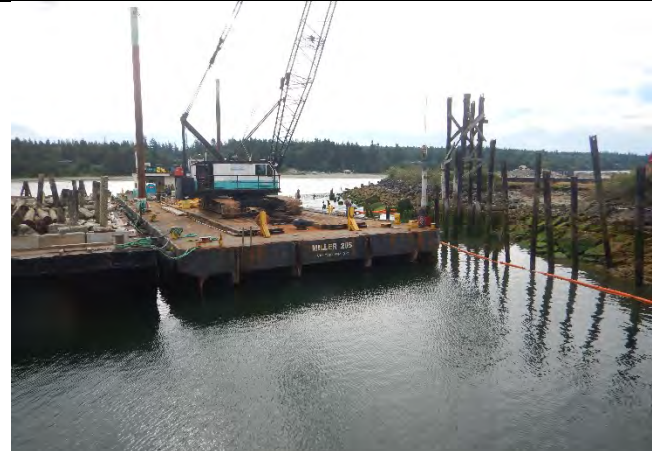
Comment: SMA-1 pile removal
