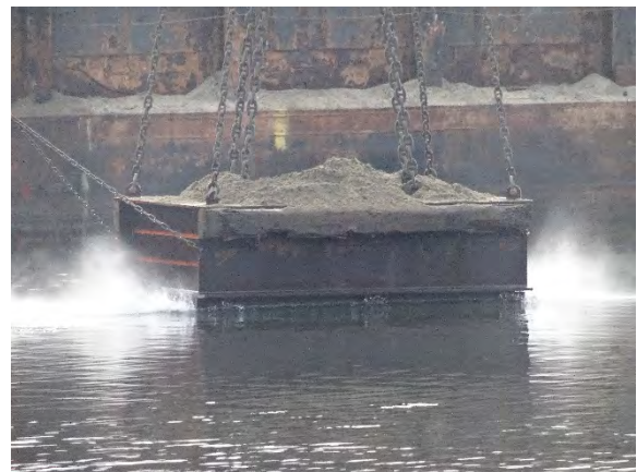
Comment: SMA-2 subtidal cap placement with Bombay Box
