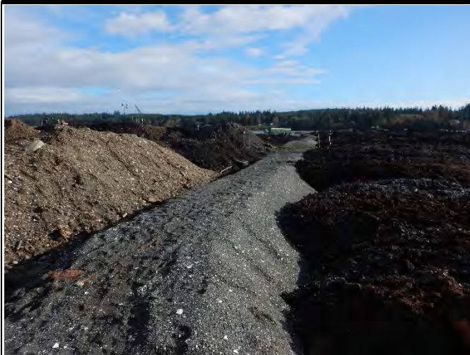
Comment: Dredge stockpiles and interior containment berms
