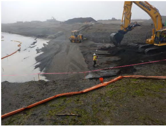
Comment: Placing filter material in completed areas and excavating 2-foot cut
