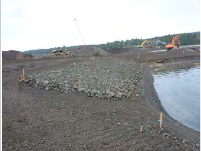
Comment: Type 2 armor rock placed on 5h:1v backfilled slope at dredging area adjacent to former Pier 4
