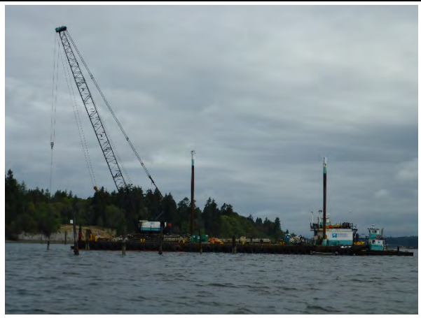
Comment: Removing piles with vibratory hammer in SMA-5
