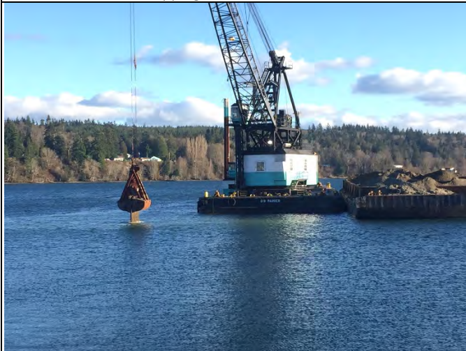
Comment: Subtidal capping in SMA-2 with DB Rainier
