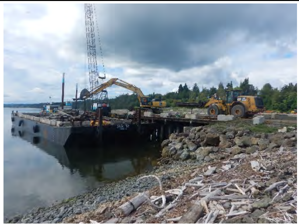
Comment: Offloading piles and transferring to upland containment/processing area
