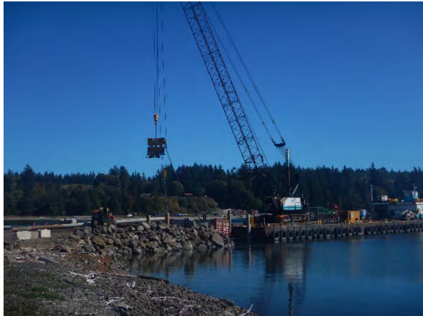
Comment: Installing temporary pilings at the transload area
